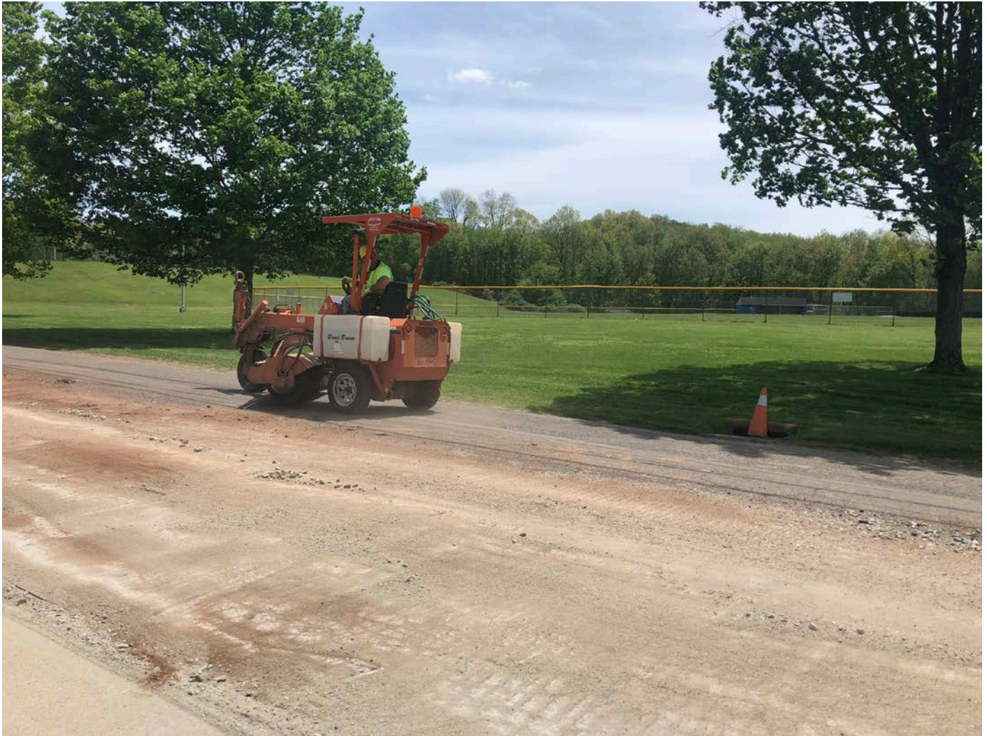
Picture 7: Ludlow cleaning up Pickett Lane with the Bocce Broom. Durham, CT.
