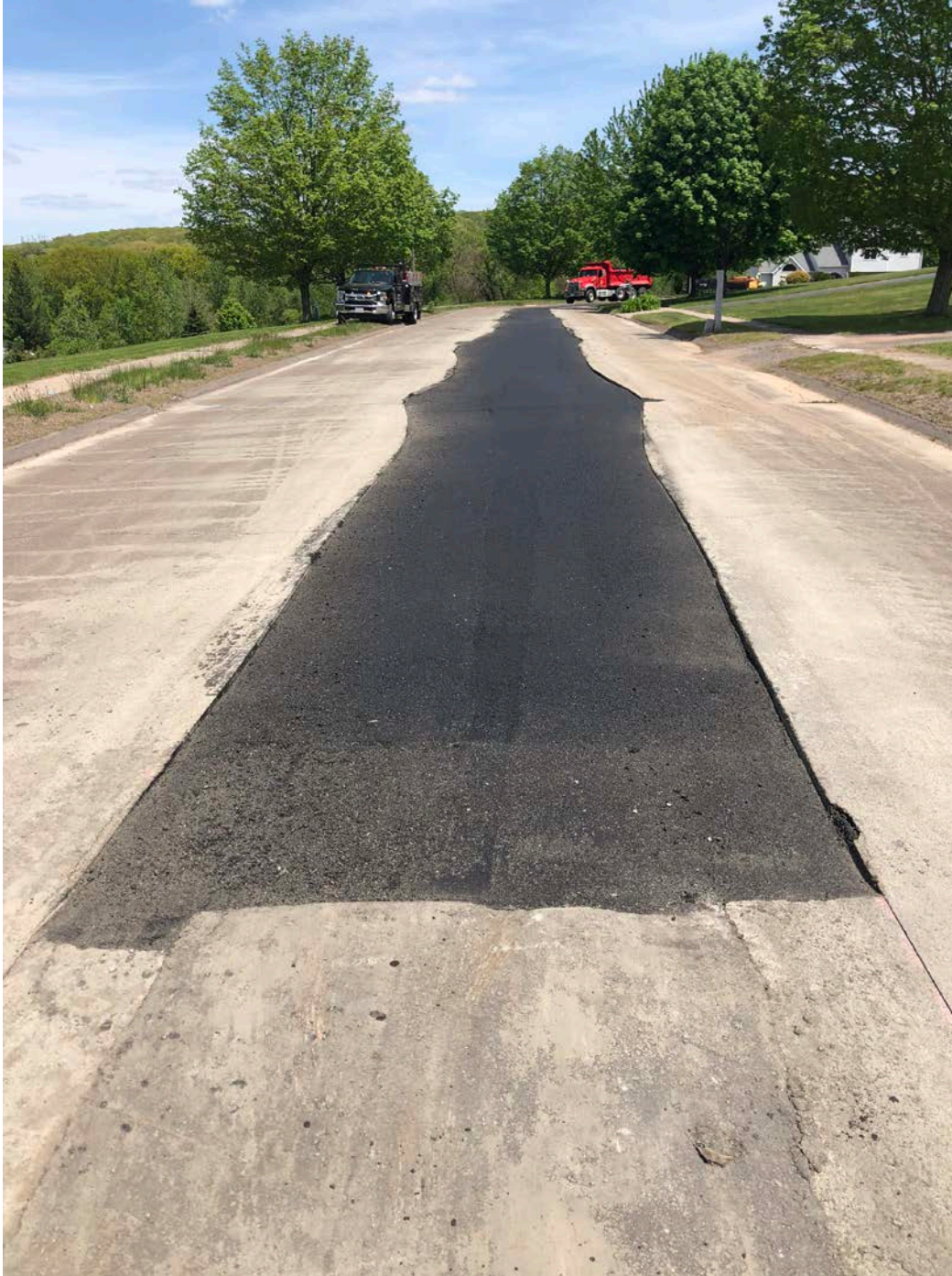
Picture 8: The first of two lifts of asphalt placed and compacted on 12" cut backs from edge of patch on Talcott Ridge Drive, Middletown, CT. Station 42+50 in the foreground.
