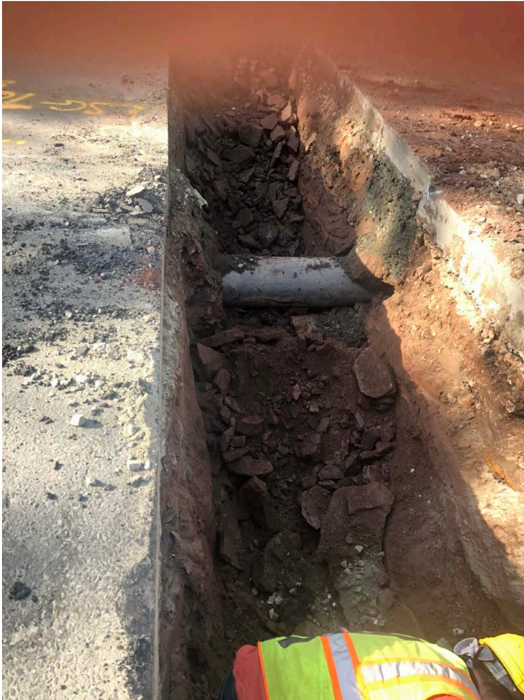
Picture 2: High-pressure gas line at the intersection of Route 68 and Main Street. Ludlow had to hammer rock around the pipe. View to the south. Durham, CT.
