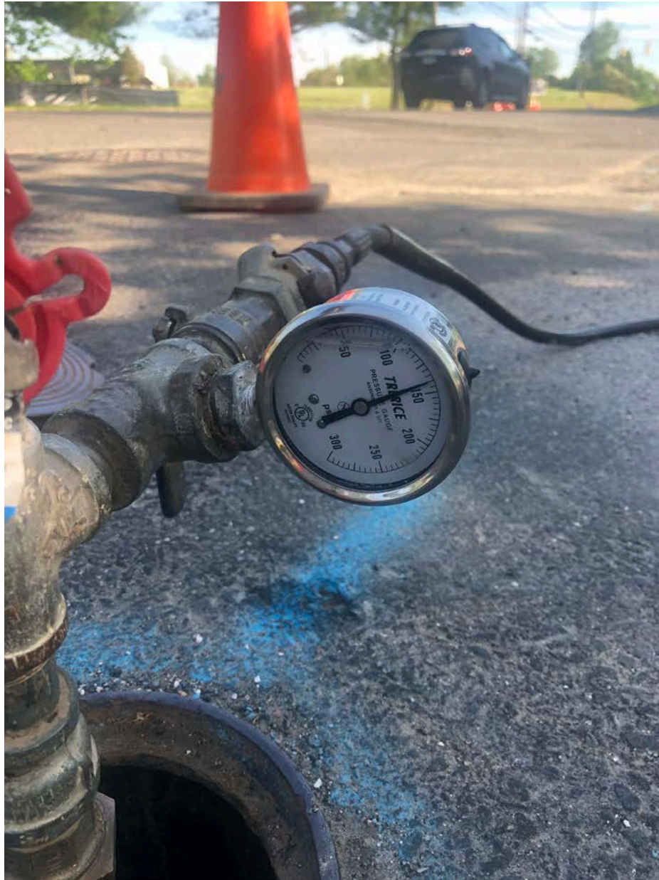
Picture 3: Pressure gauge for the pressure test performed on the water line located at the intersection of Talcott Ridge Drive and South Main Street. Middletown, CT. View to the north.
