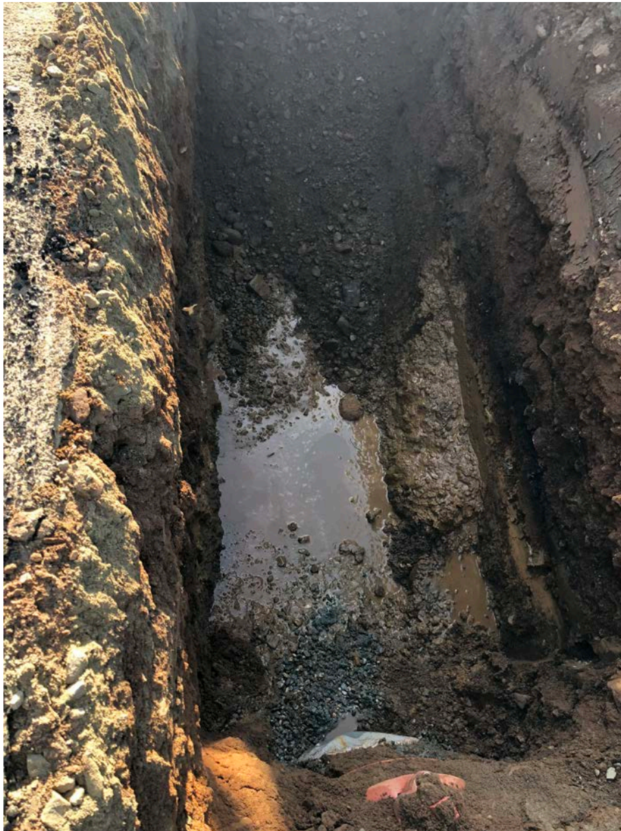
Picture 1: Water observed in bottom of trench on Pickett Lane at ~ Station 518+38. View to the southeast. Middletown, CT).
