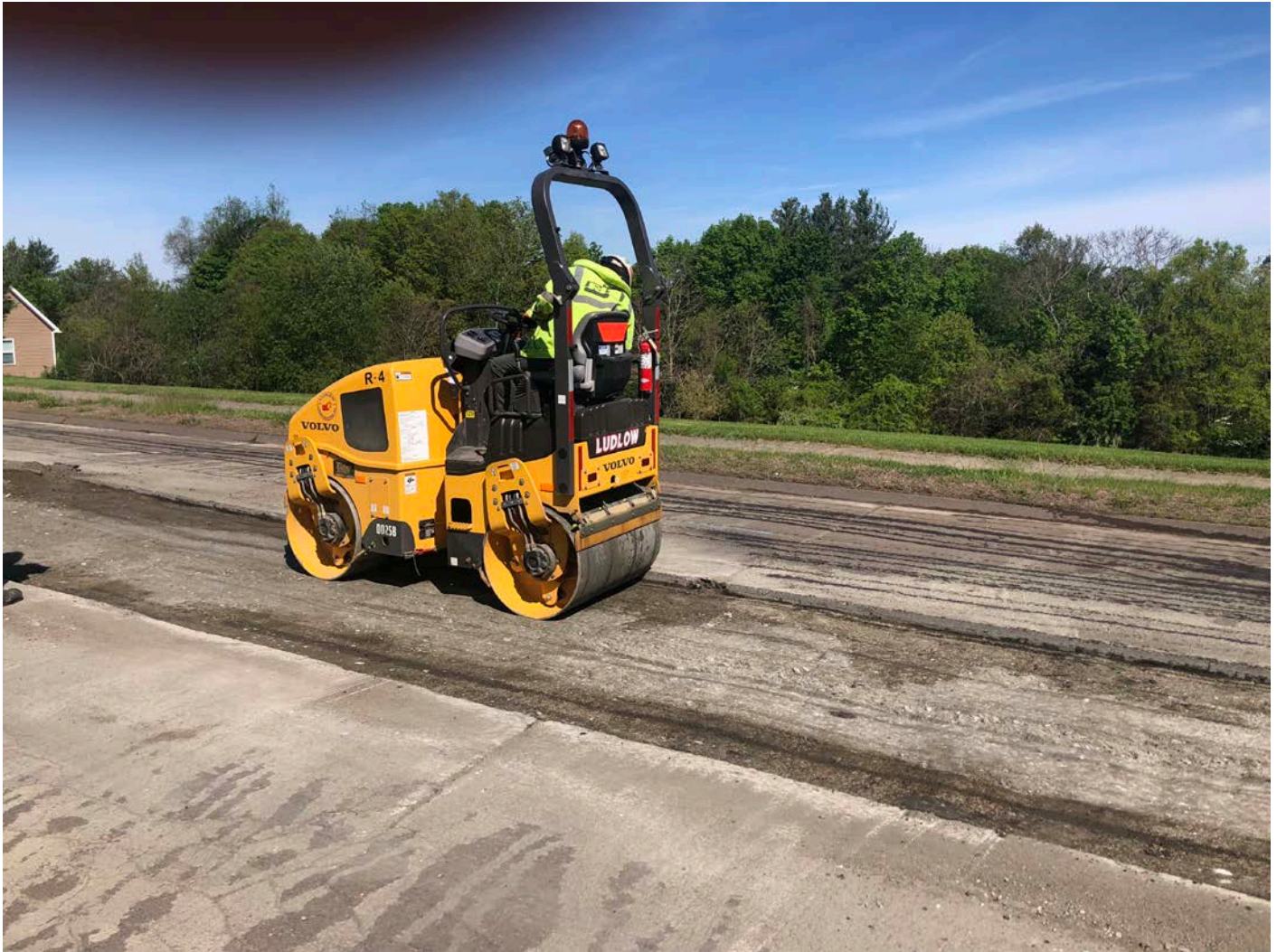
Picture 5: Ludlow compacting road base after having removed asphalt patch. Talcott Ridge Drive, Middletown, CT.
