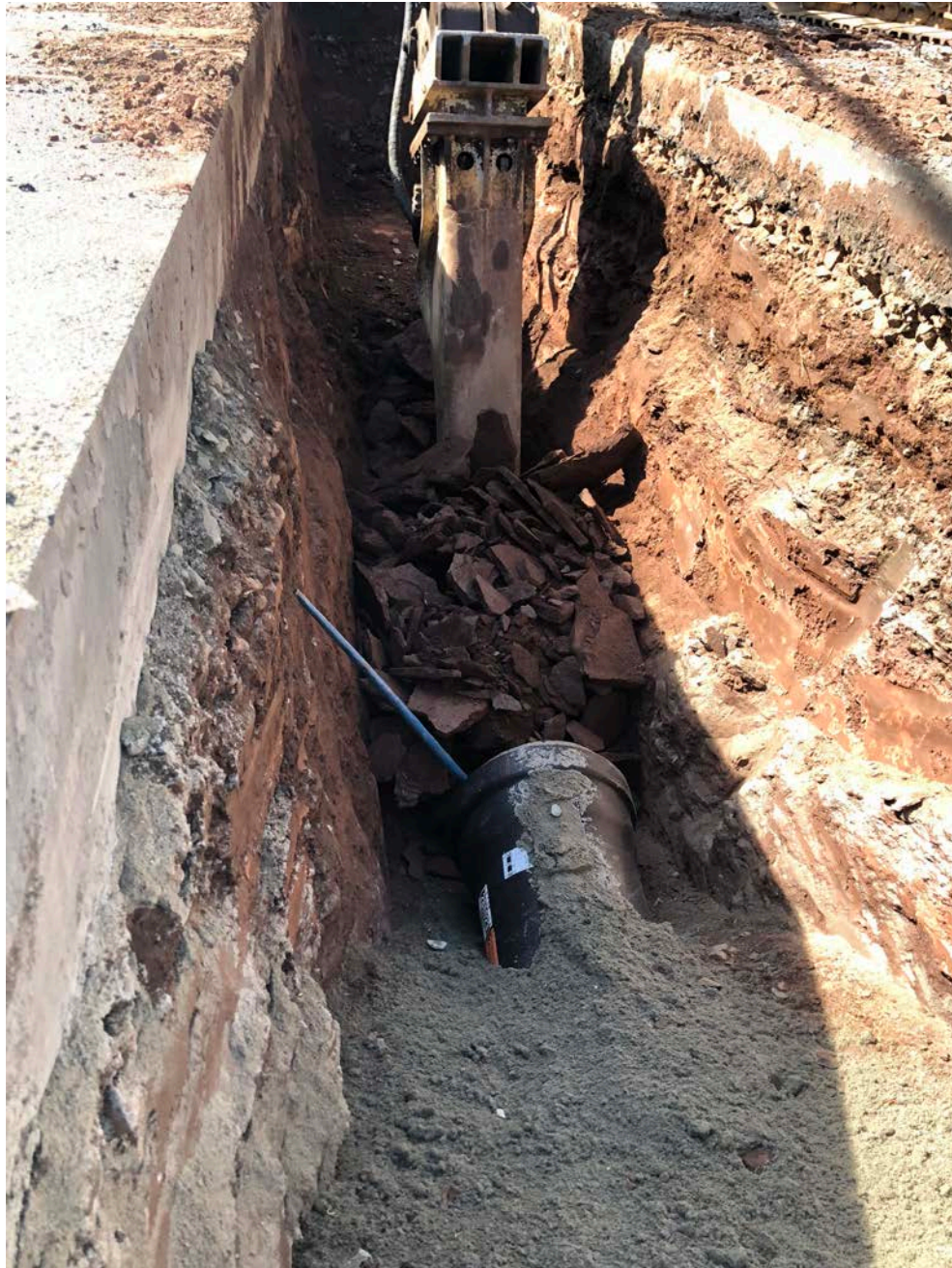
Picture 6: Ludlow hammering rock in the trench at Station 195+65 (intersection of Route 68 and Main Street). View to the south. Main Street, Durham, CT.
