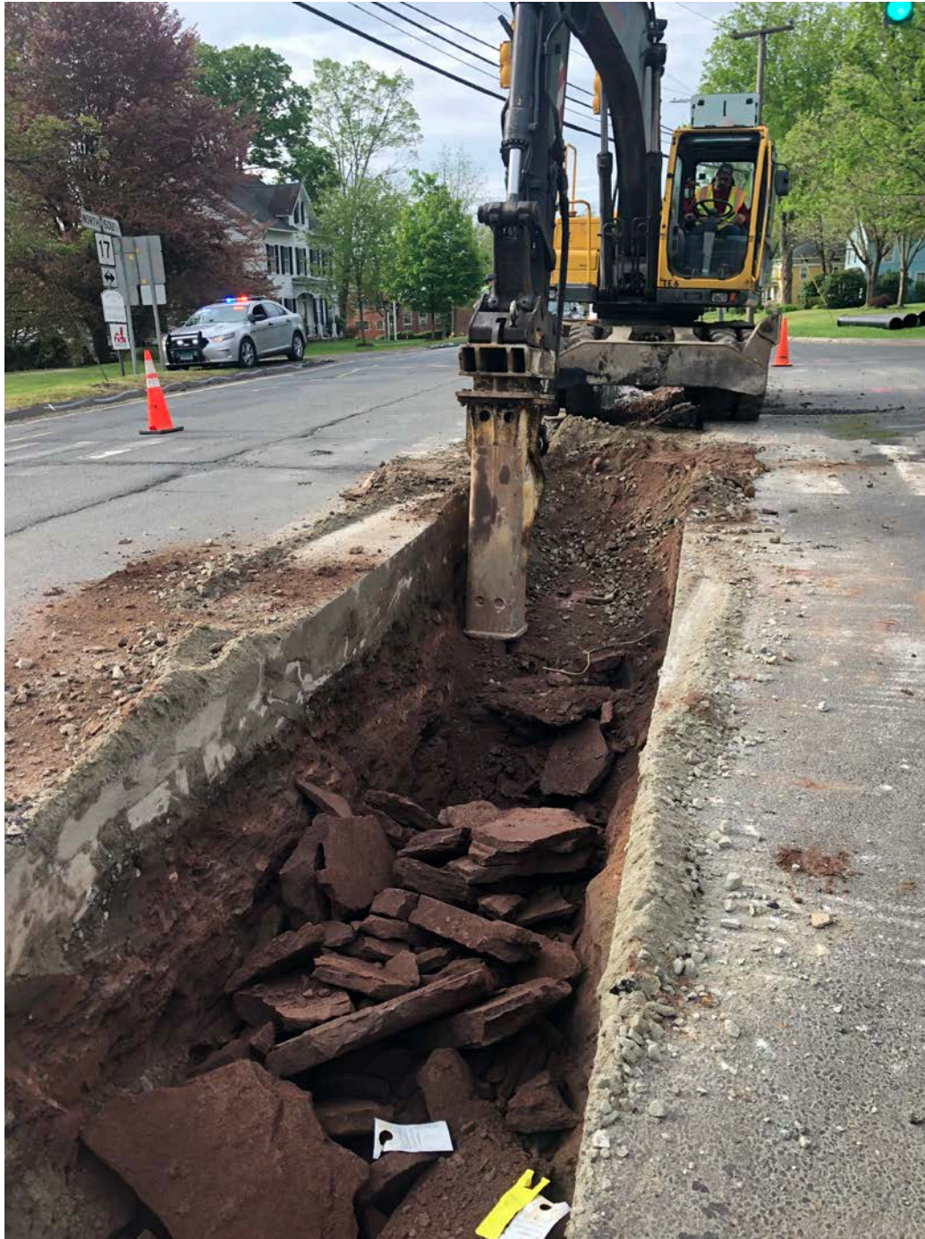
Picture 4: Ludlow hammering rock encountered beginning at Station 194+78. View to the south. Durham, CT.
