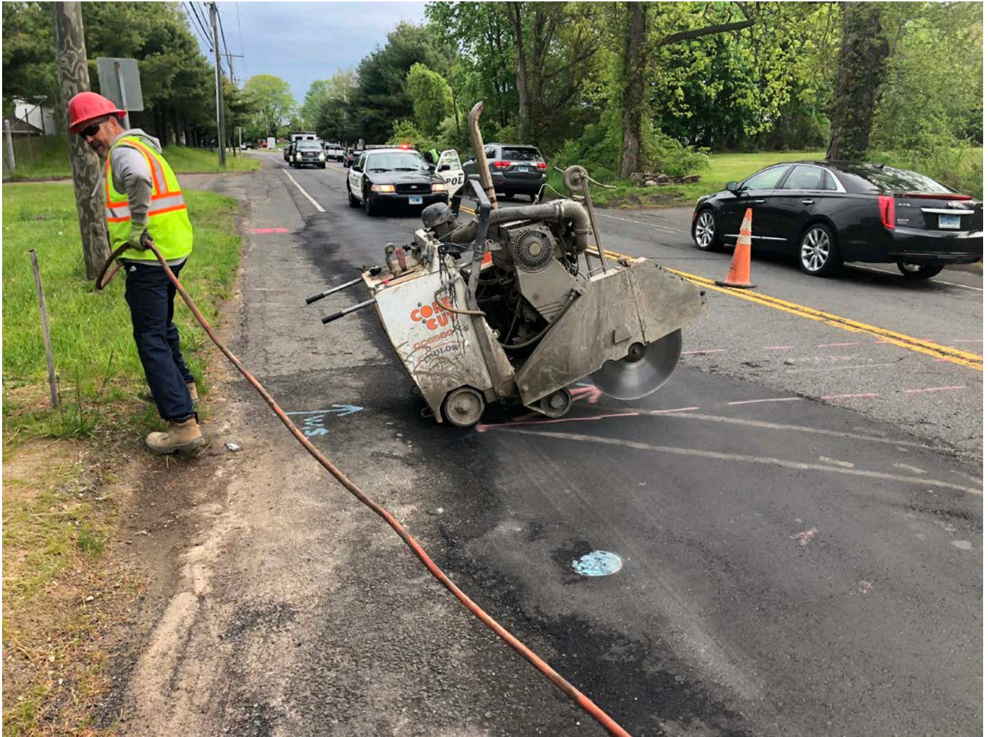
Picture 3: Ludlow saw cutting pavement on the southbound side of South Main Street in Middletown, CT. View to the north.
