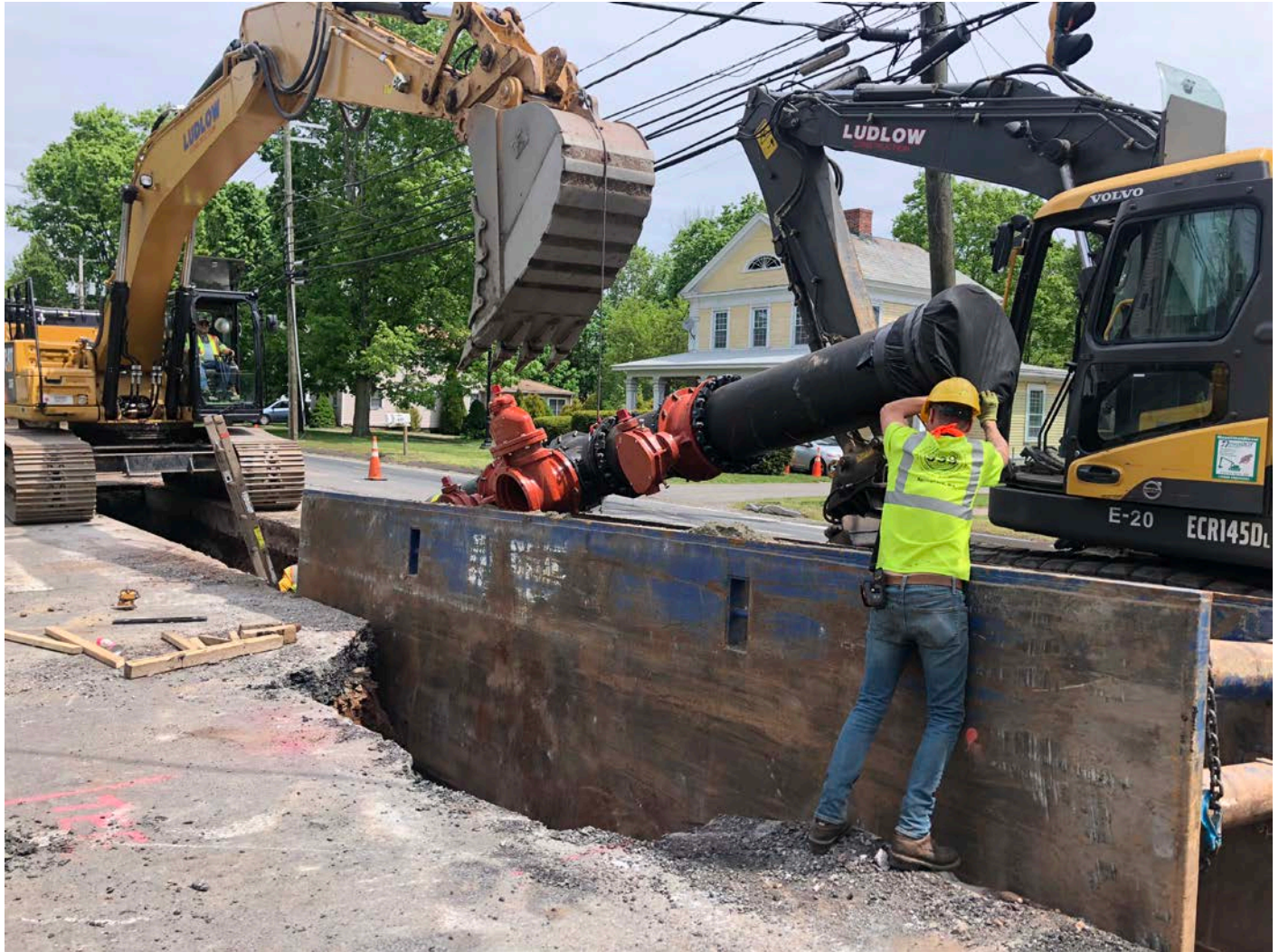
Picture 6: Ludlow placing 16"x16"x12" M.J. C.L.D.I. TEE with two 16" M.J. butterfly valves and a 12" M.J. gate valve and gate box at Station 195+26. View to the northeast. Durham, CT.
