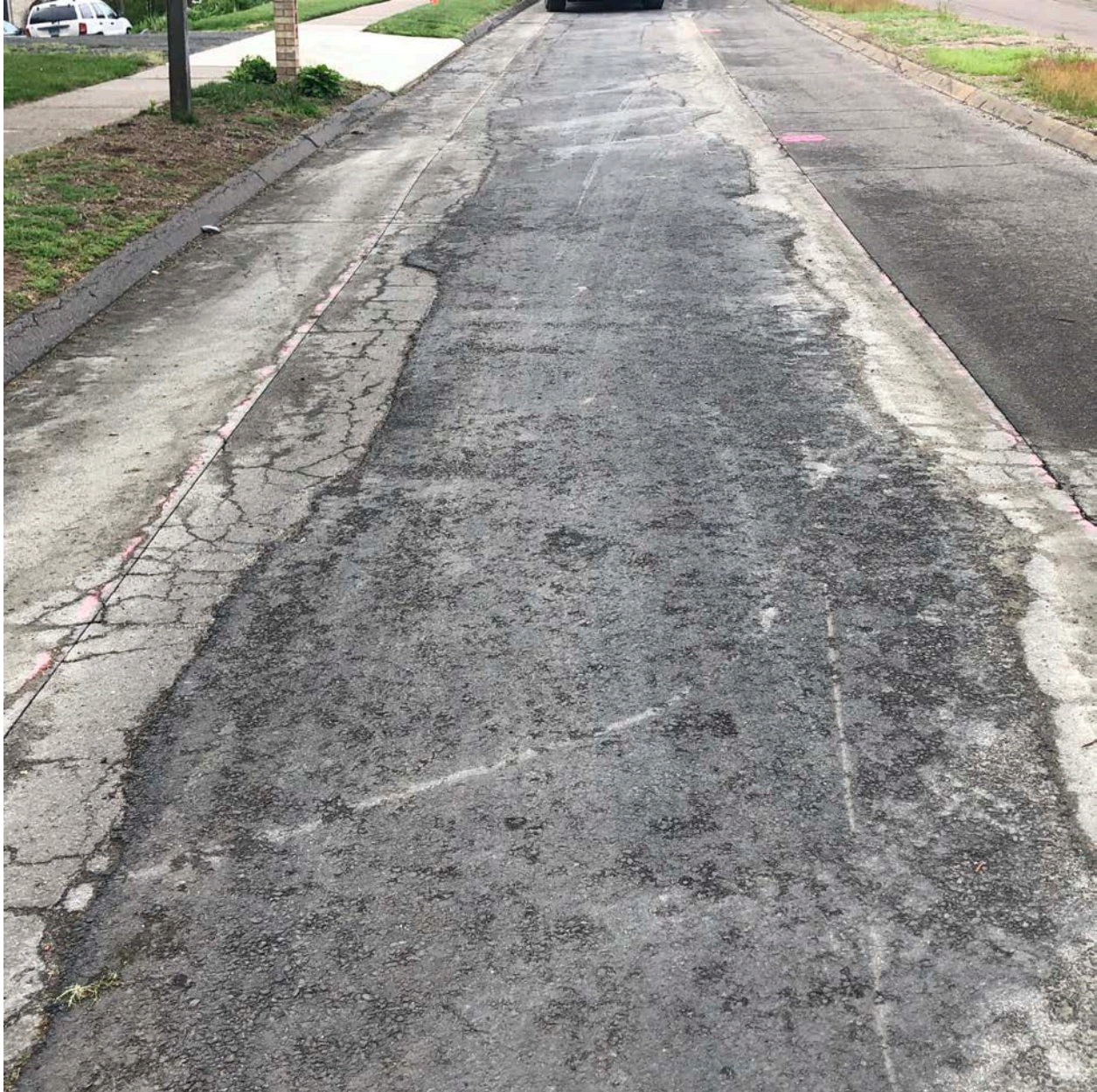
Picture 2: Cut pavement on either side of patched trench on Talcott Ridge Drive. View to the southeast. Middletown, CT.
