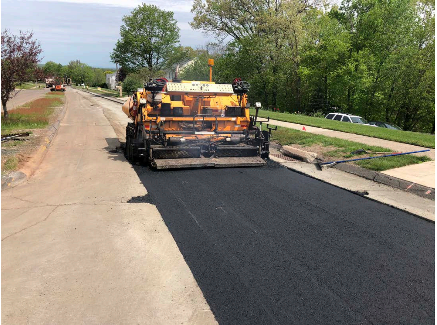
Picture 5: Ludlow placing first lift of hot patch on Talcott Ridge Drive at ~Station 36+00. View to the northwest. Middletown, CT.
