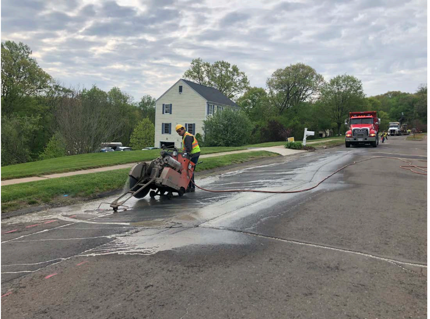
Picture 1: Ludlow saw cutting pavement on Talcott Ridge Drive at ~Station 36+50. View to the southeast. Middletown, CT).
