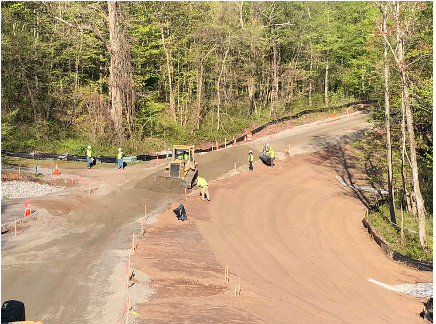
Picture 2: Ludlow filling and grading between stations 16+00 and 14+40 in preparation to place plastic soil stabilization grid. View to the west. Middletown, CT
