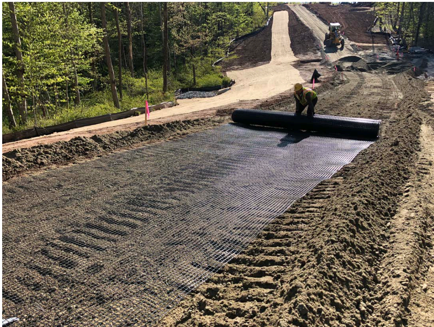
Picture 3: Ludlow places plastic soil stabilization grid between stations 16+00 and 14+40. View to the east. Middletown, CT.
