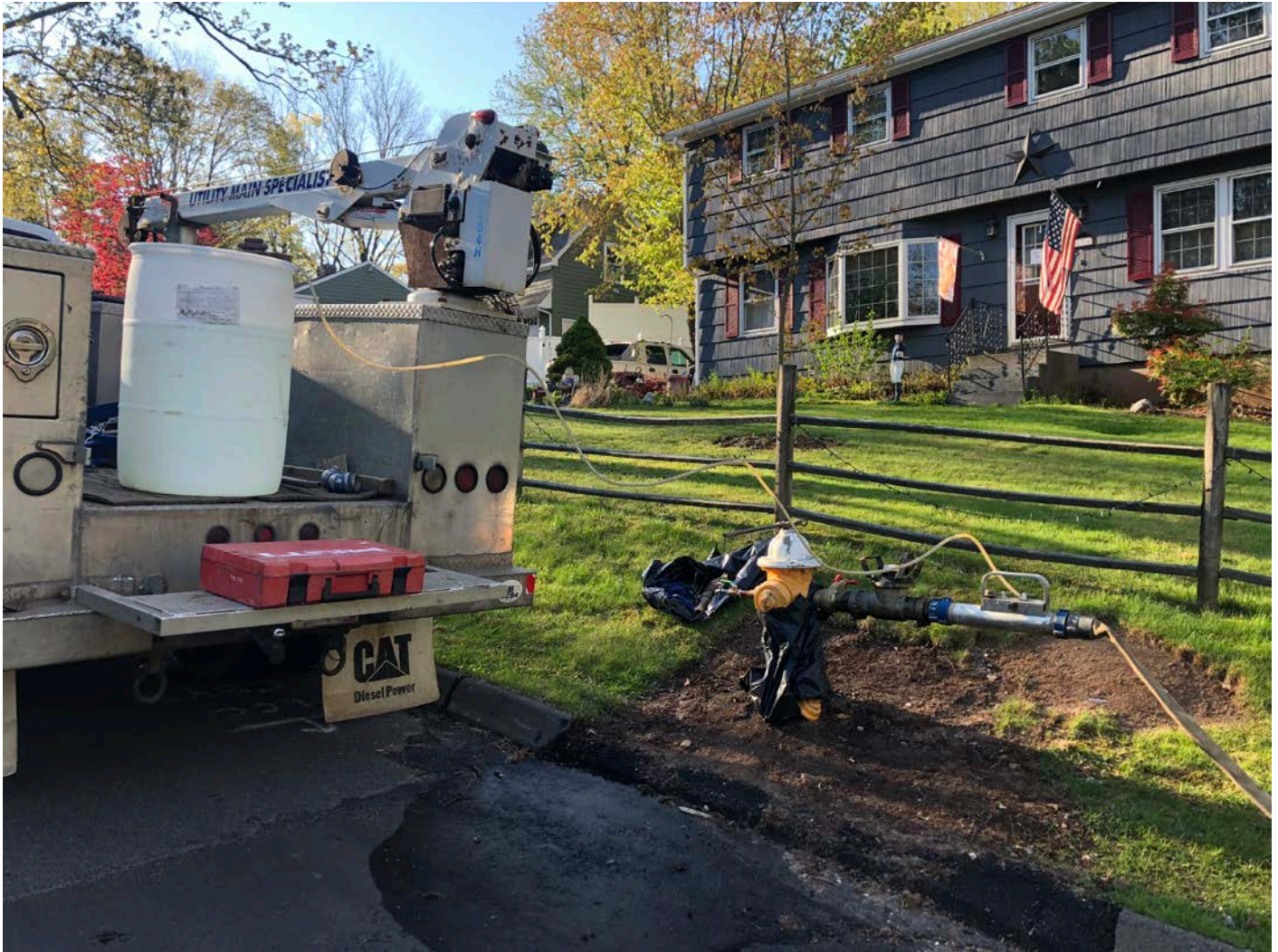
Picture 1: Disinfection of water line running from the intersection of Main Street and Talcott Ridge Drive to the intersection of Main Street and Oak Terrace.
