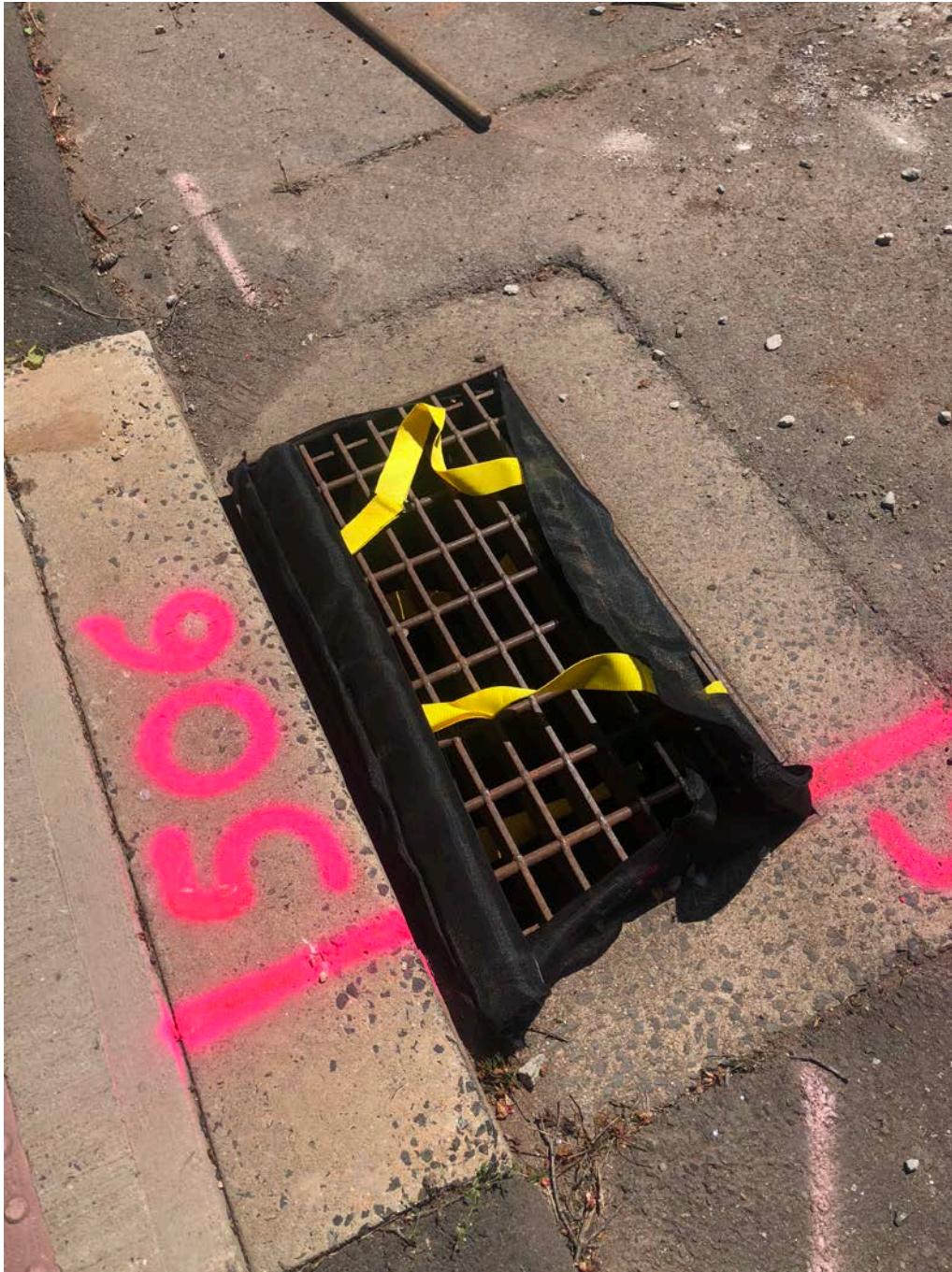
Picture 5: Silt sock placed in catch basin at Station 506+00. Picket Lane, Durham CT.
