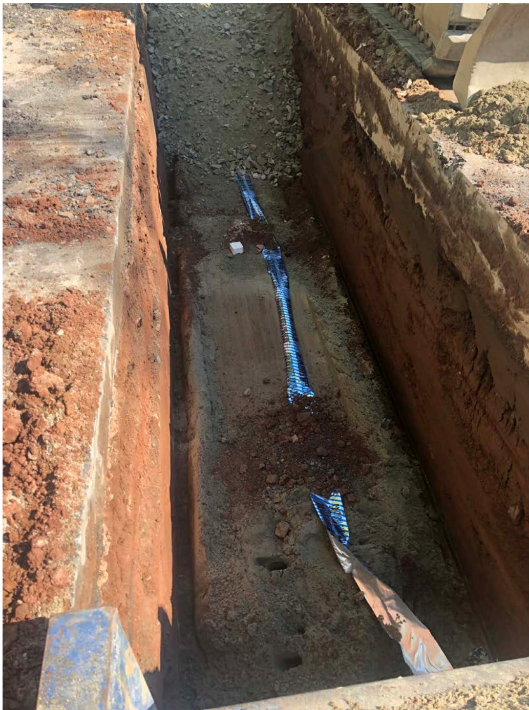
Picture 4: Caution tape placed over 16" DIP in trench on Main Street at Station 190+00. View to the north. Durham CT.
