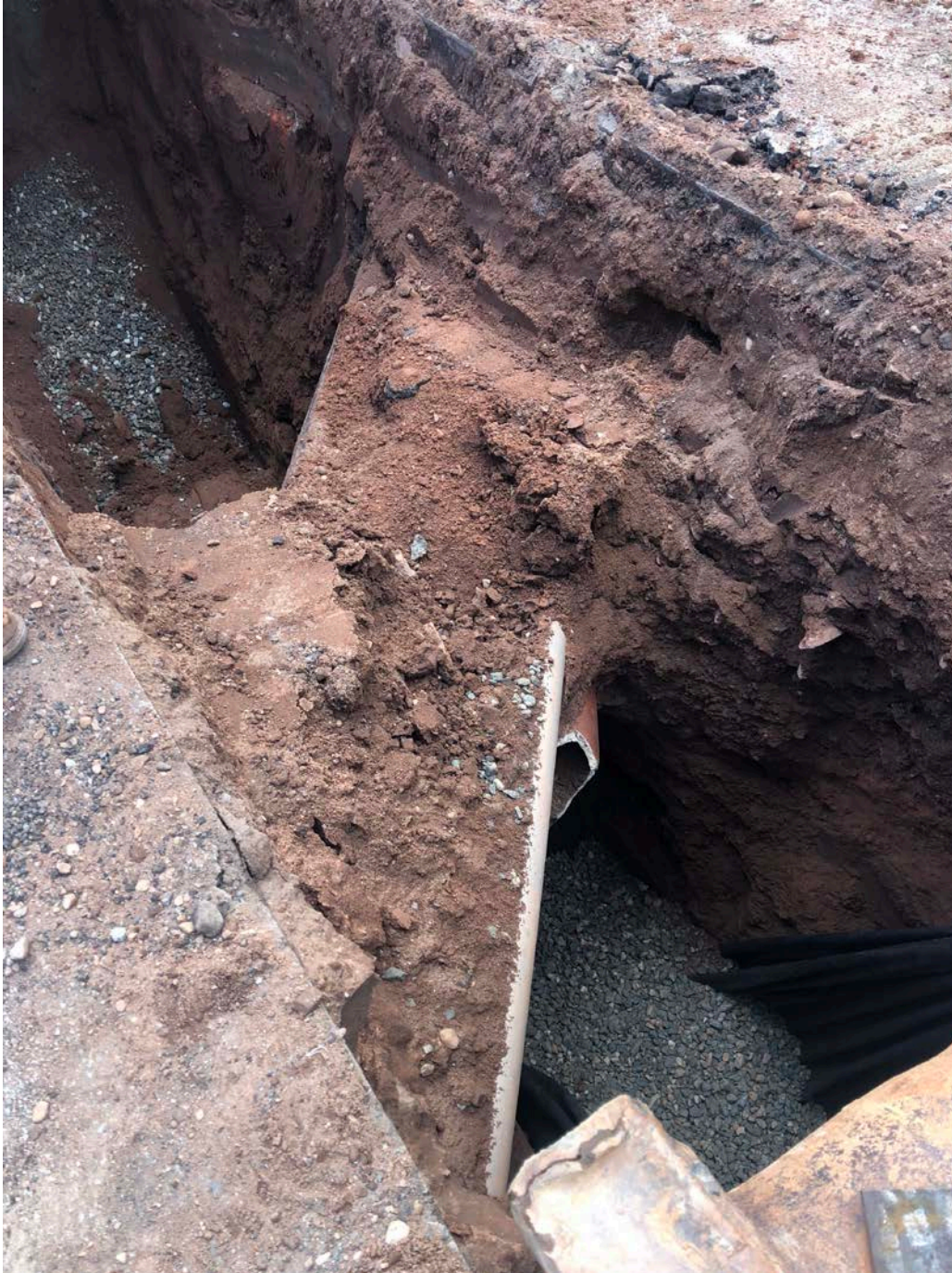
Picture 5: Utilities daylighted at Station 503+50: two conduits of 4" PVC and an 8" clay pipe beneath the PVC that was damaged during excavation. Durham, CT.
