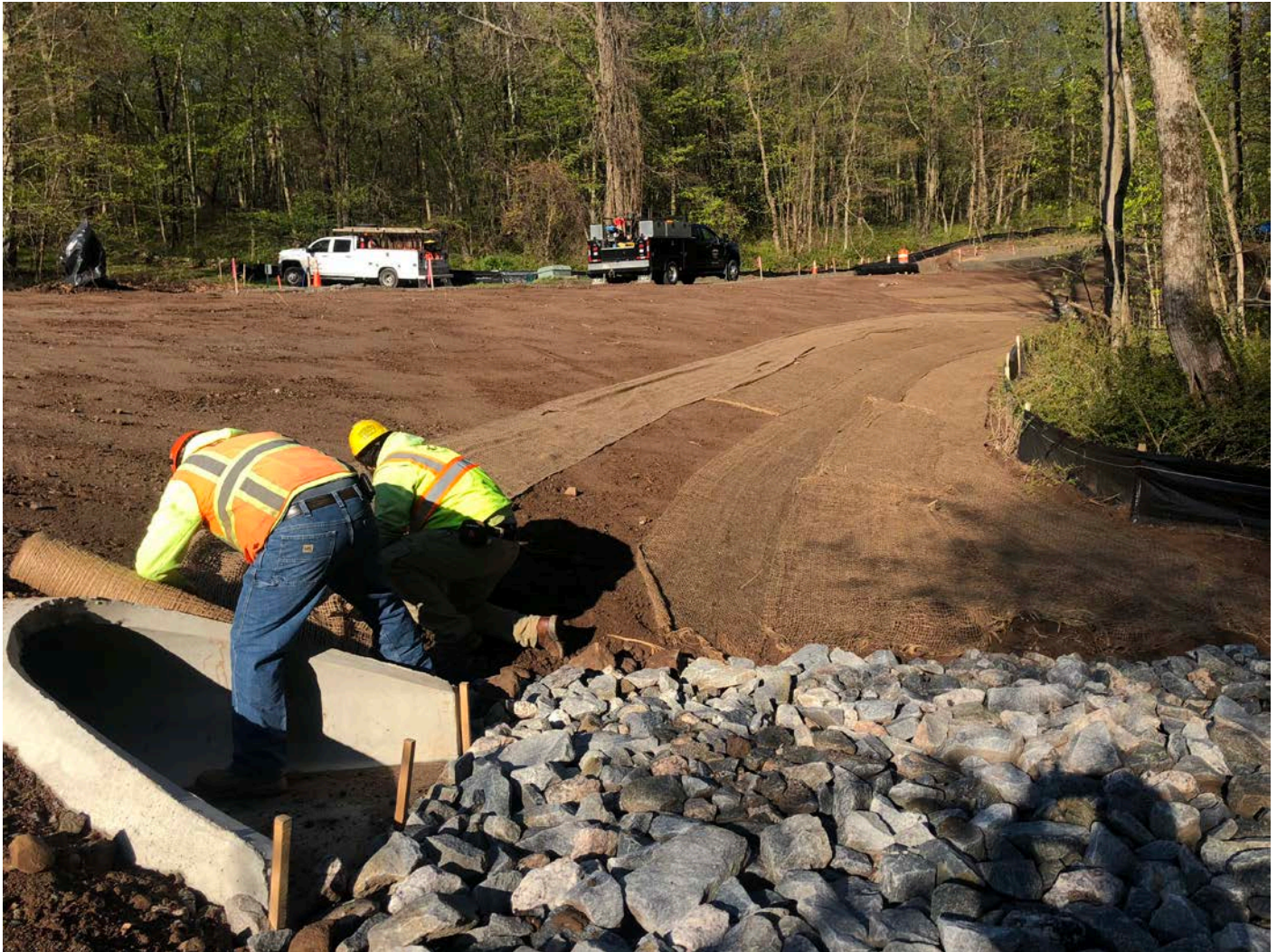
Picture 1: Ludlow placing jute erosion control cloth on the north side of the shared access road at ~Station 14+40. View to the west. Middletown, CT.
