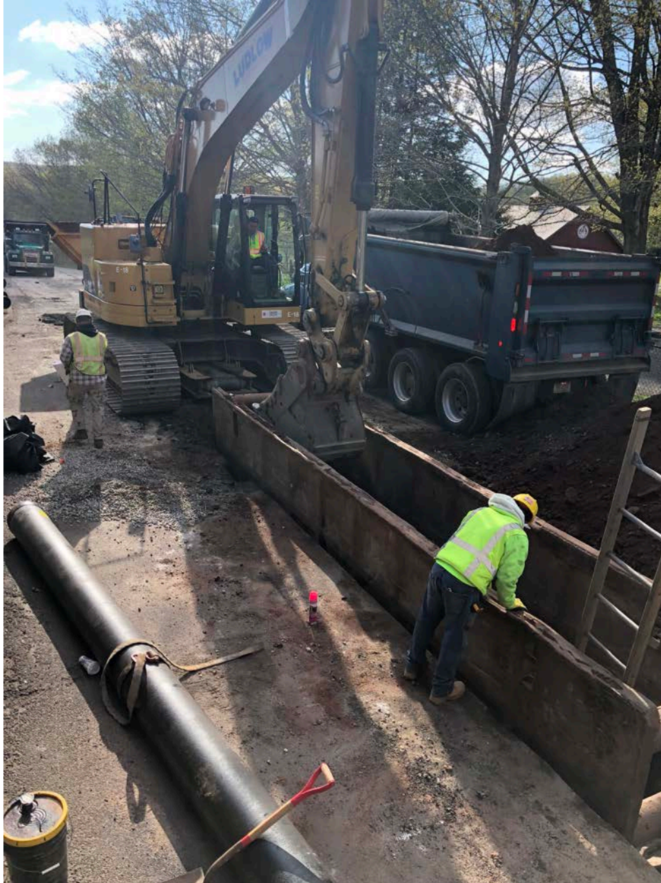
Picture 3: Ludlow placing 12" DIP. View to the southeast. Pickett Lane, Durham, CT.
