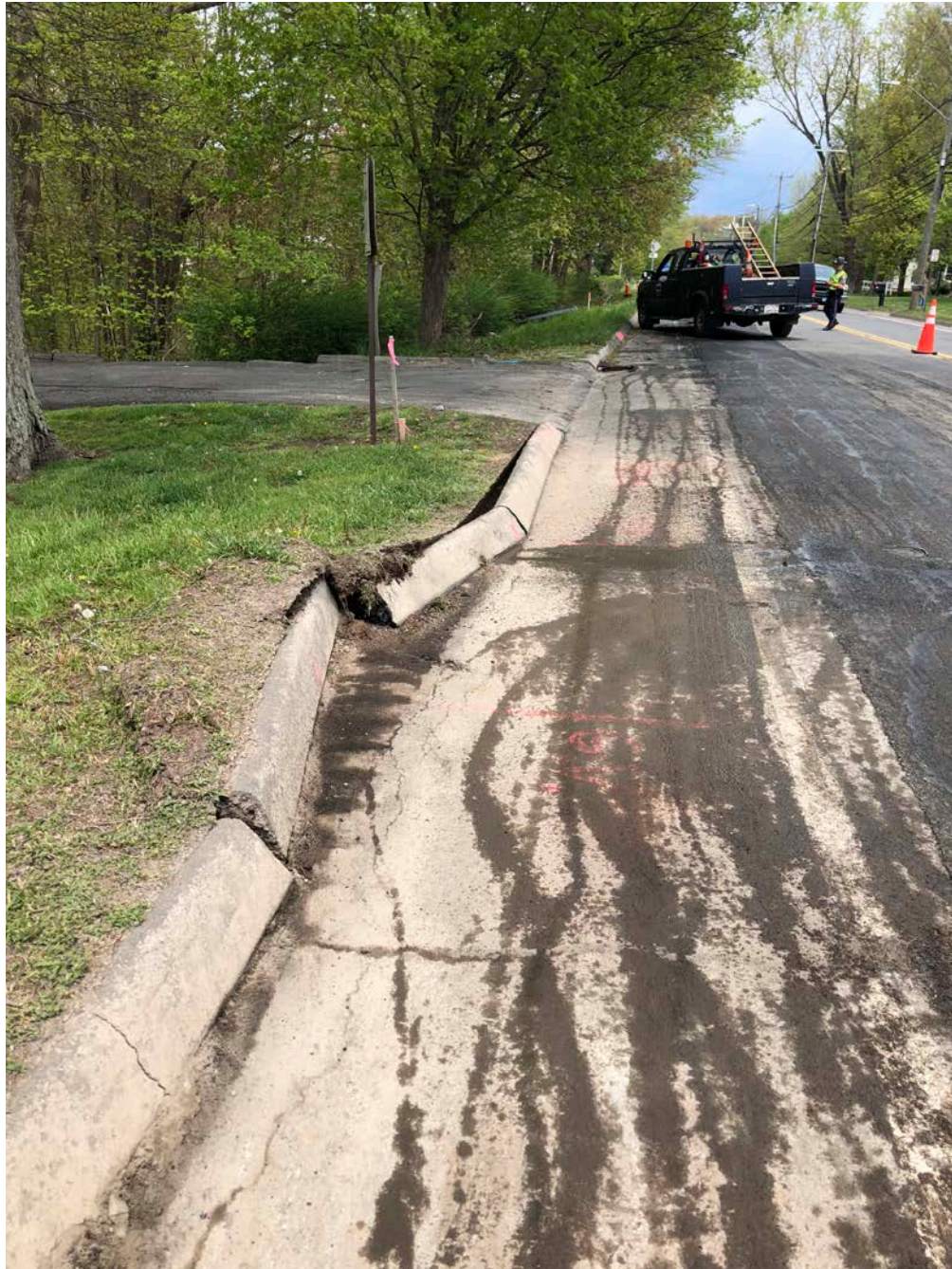
Picture 8: Damage to curbing at Station 185+20. View to the north. Main Street, Durham, CT.
