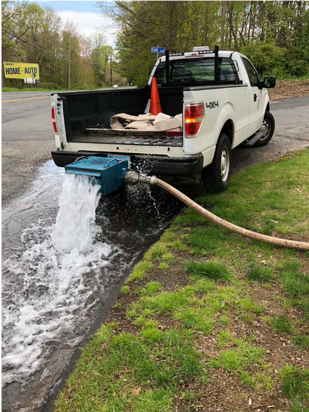
Picture 2: Hydrant/waterline being flushed at Oak Terrace. View to the north. Durham, CT.
