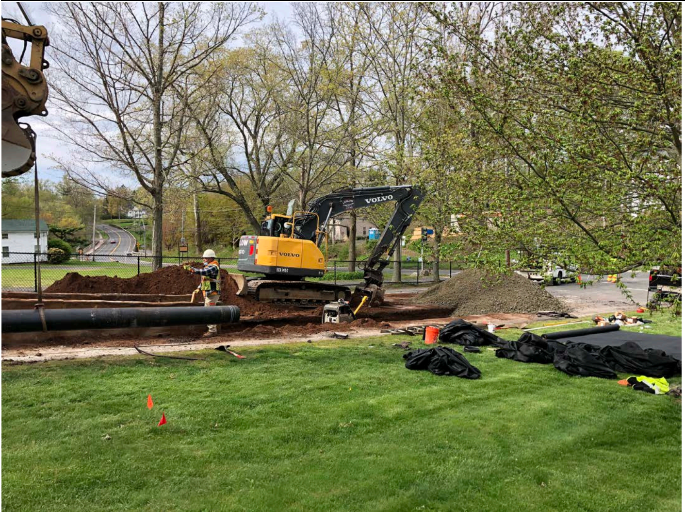
Picture 5: Ludlow placing 12" DIP on Pickett Lane at ~Station 501+40. View to the southwest. Durham, CT.
