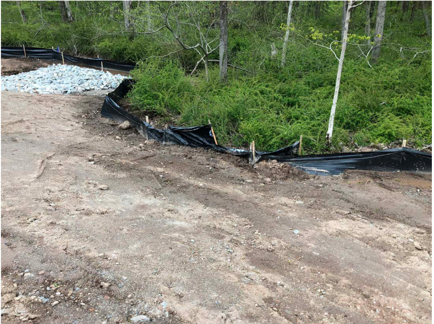
Picture 6: Minor break in silt fence north of 14+40. View to the northwest. Middletown, CT.
