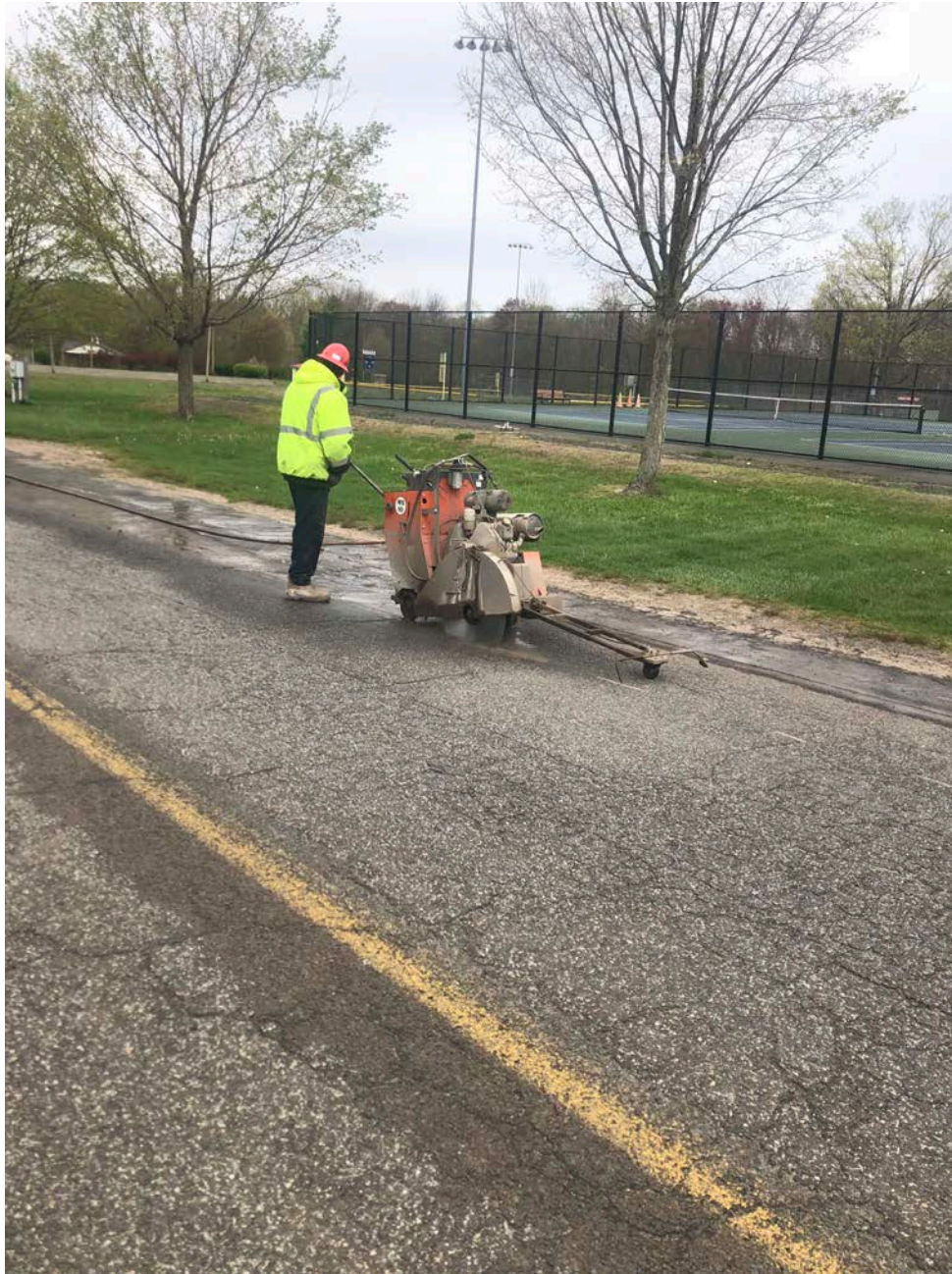
Picture 2: Ludlow saw cutting pavement at Station 521. View to the northwest. Pickett Lane, Durham, CT.
