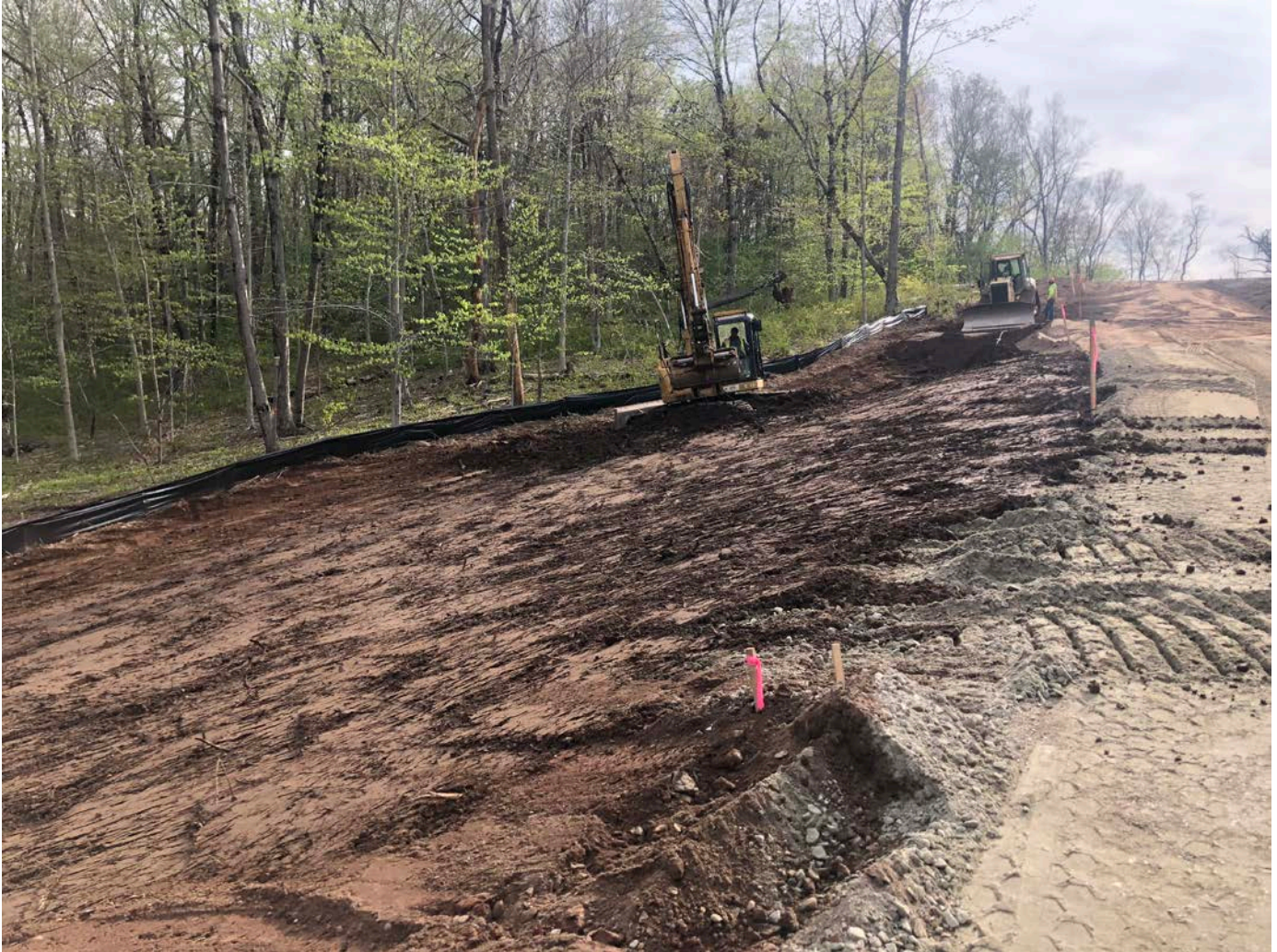
Picture 1: Ludlow filling and grading along the north side of the shared access road. View to the east. Middletown, CT.
