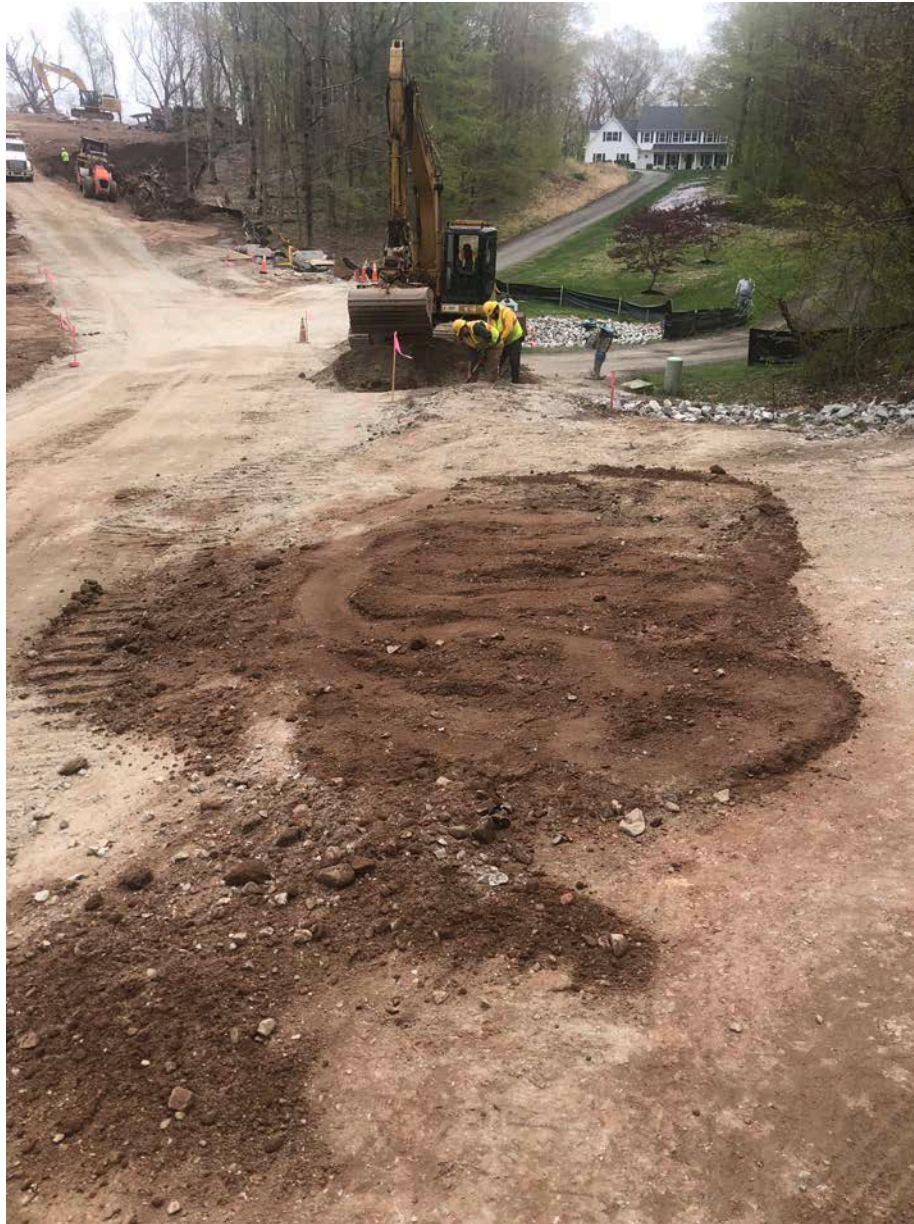
Picture 4: Ludlow digging test pits in front of the driveways for 216 and 224 Talcott Ridge Drive to locate utilities. View to the east. Middletown, CT.
