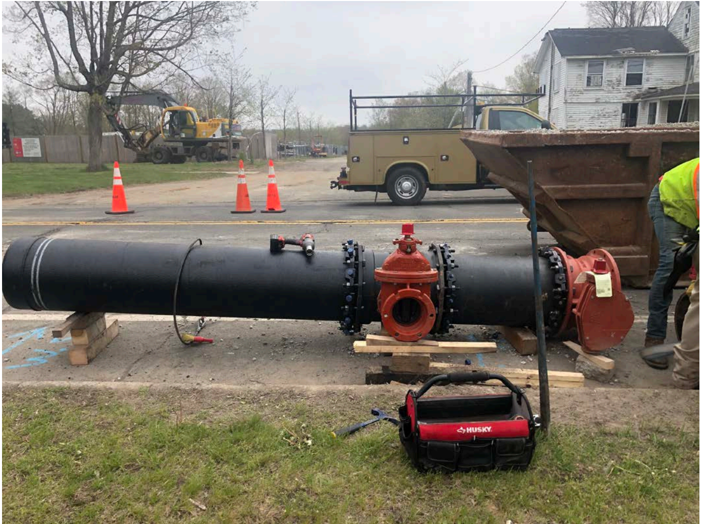
Picture 3: 16" x 6" M.J. C.D.L.I. hydrant Tee with a 6" gate valve and valve box and a 16" M.J butterfly valve and valve box being assembled to place at Stations 183+57.5 and 183+61, respectively. Main Street, Durham, CT.
