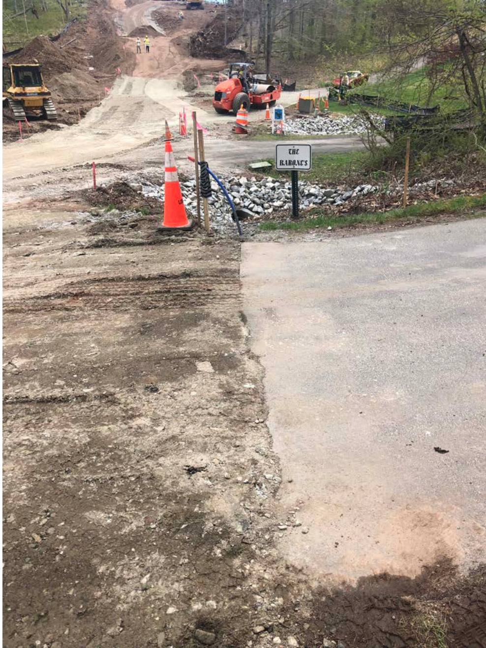
Picture 5: Driveway for 224 Talcott Ridge Drive after end was saw cut to make a clean transition to the shared access road. View to the east. Middletown, CT.
