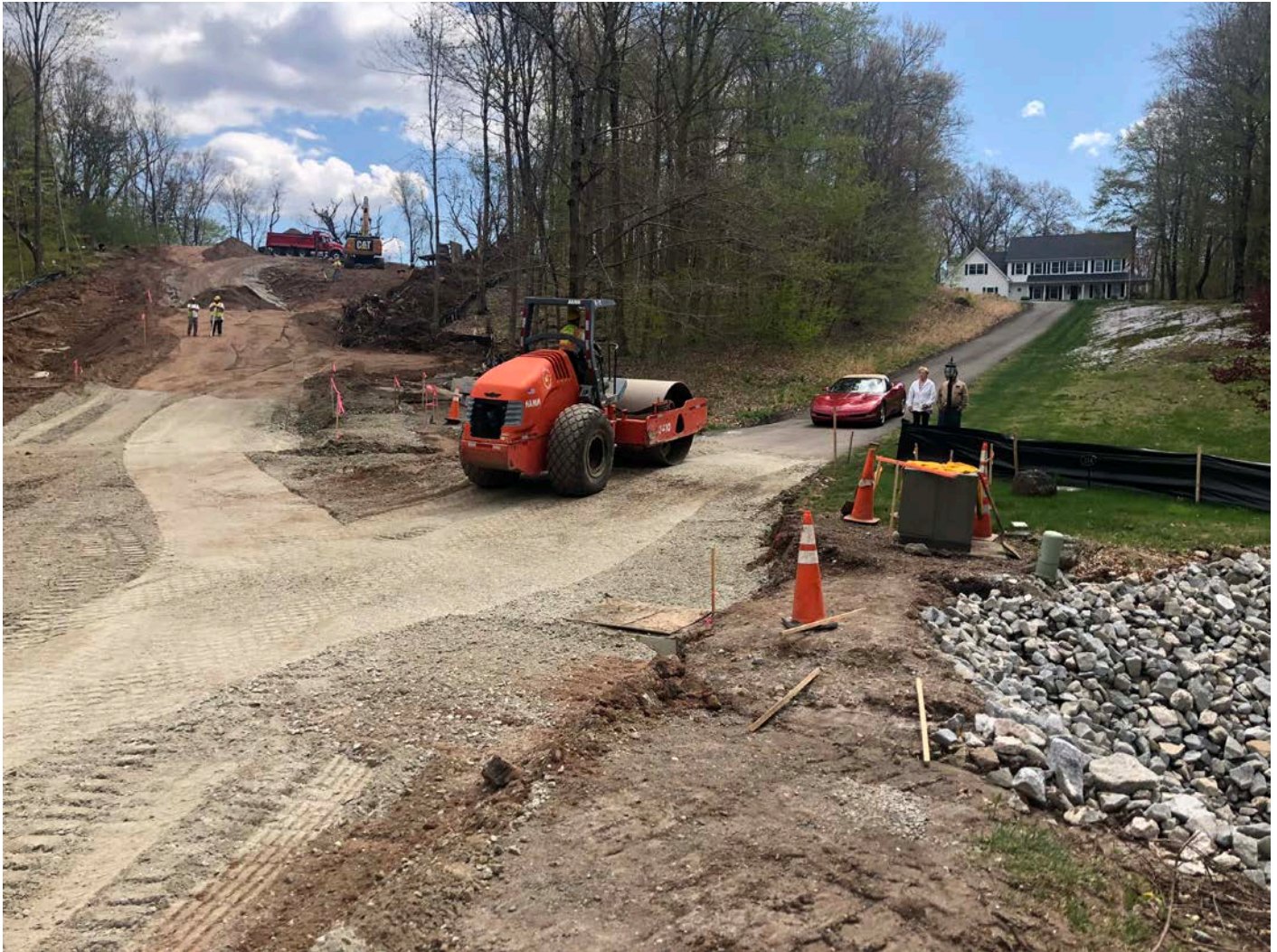
Picture 7: Ludlow compacting fill adjacent to the driveway for 214 Talcott Ridge Drive. View to the southeast. Middletown, CT.
