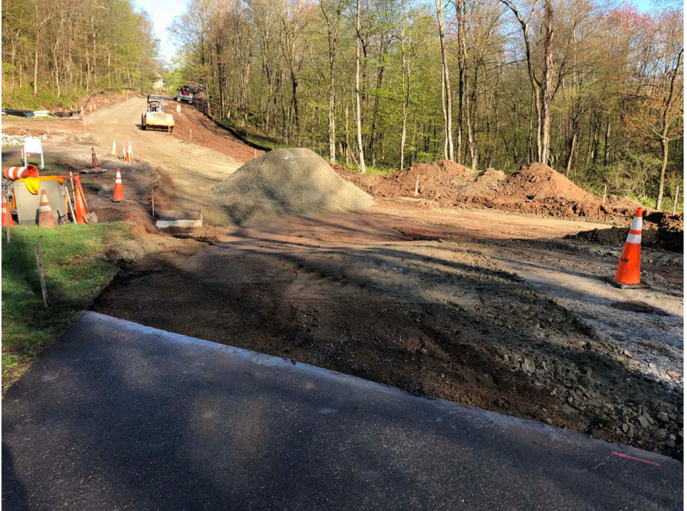
Picture 2: Driveway for 214 Talcott Ridge Drive after end was saw cut to make a clean transition to the shared access road. View to the northwest. Middletown, CT.
