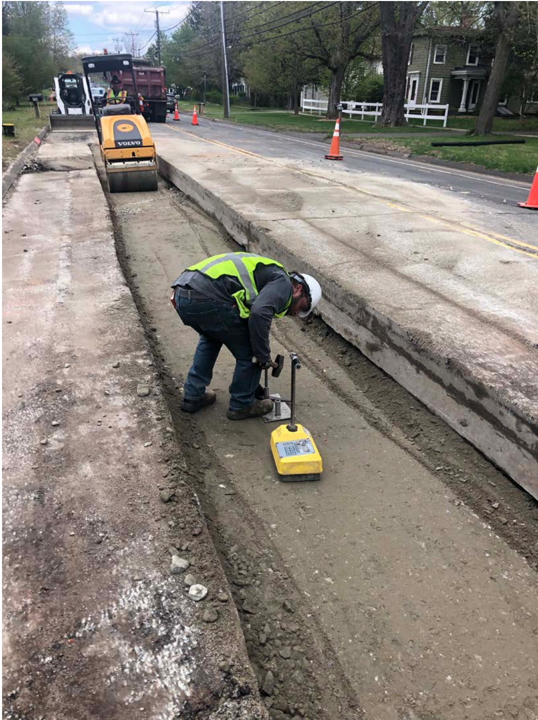
Picture 8: JTC performing compaction testing along the southbound lane of Main Street. View to the northeast. Middletown, CT.
