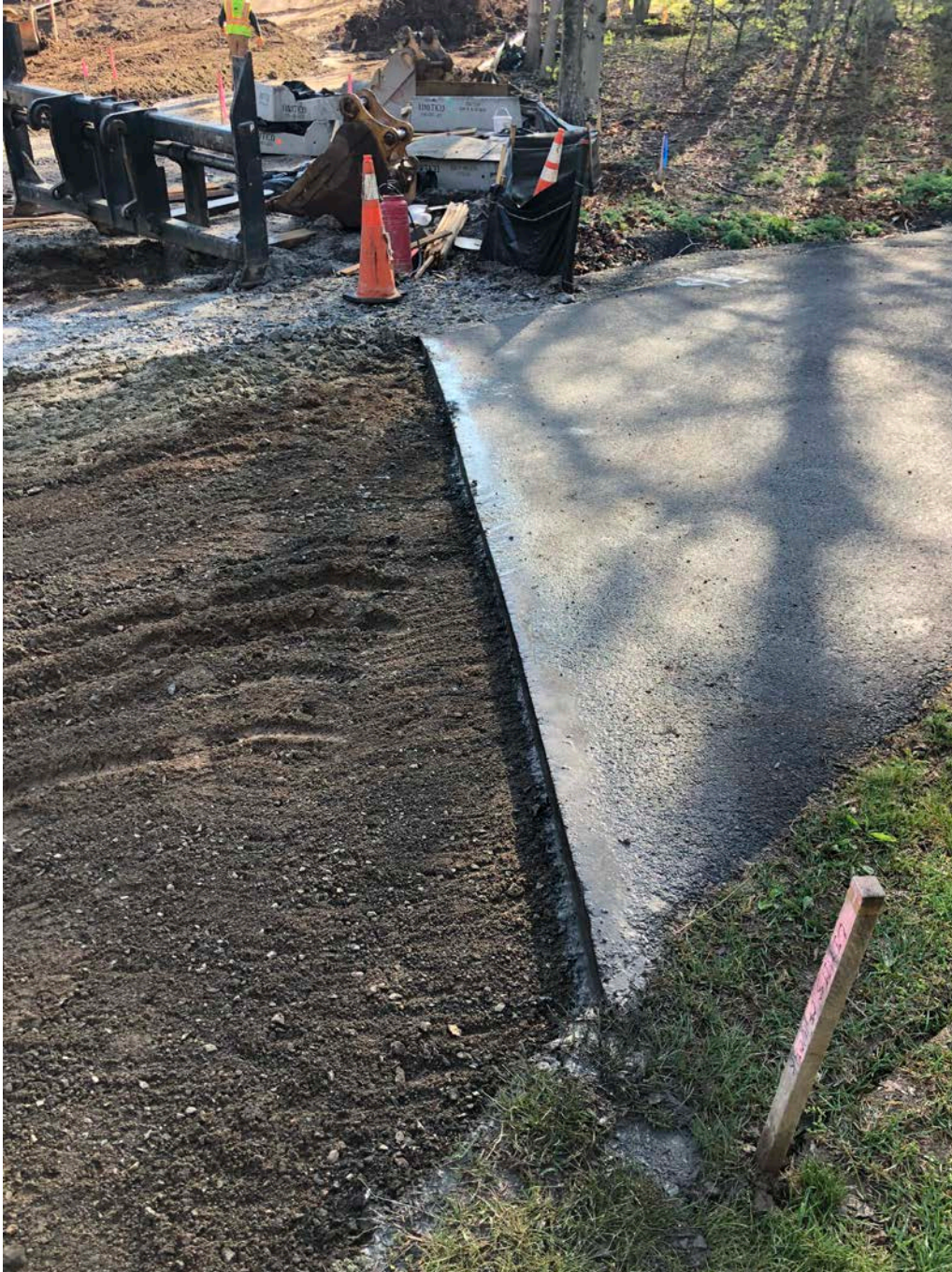
Picture 3: Driveway for 214 Talcott Ridge Drive after end was saw cut to make a clean transition to the shared access road. View to the east. Middletown, CT.
