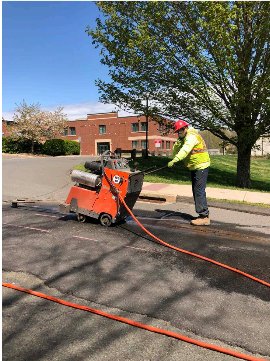
Picture 5: Ludlow saw cutting on Pickett Lane. View to the north. Durham, CT.
