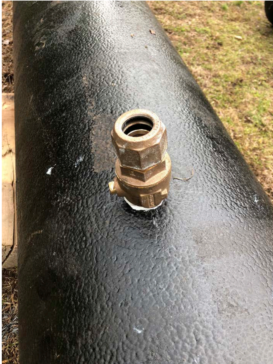
Picture 2: 1" corporation stop placed onto 16" DIP. Main Street, Durham, CT.
