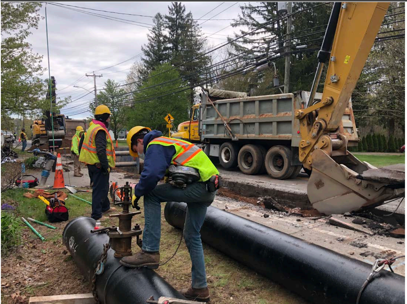
Picture 1: Ludlow tapping 16" DIP for the placement of a corporation stop. Main Street, Durham, CT.
