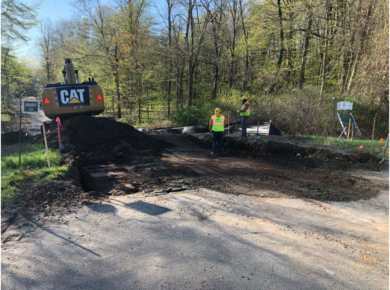
Picture 1: Ludlow begins to excavate the shared access driveway to place processed stone base for the new driveway. View to the southeast. Middletown, CT.
