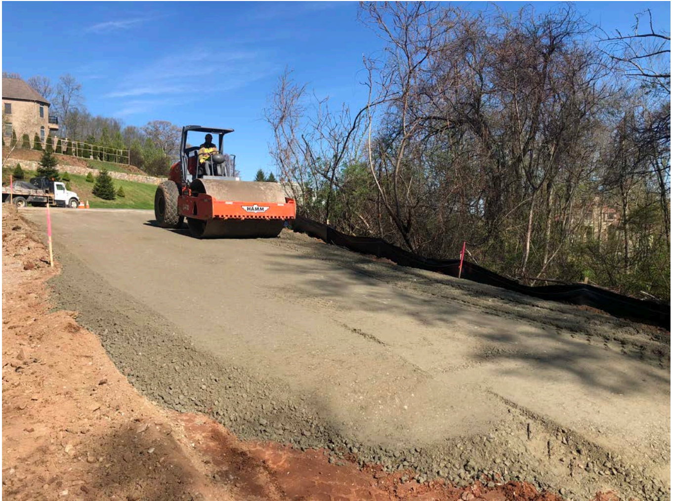
Picture 2: Ludlow rolling 1 1/4" processed stone as part of upgrade activities on the shared access road. View to the northwest. Middletown, CT
