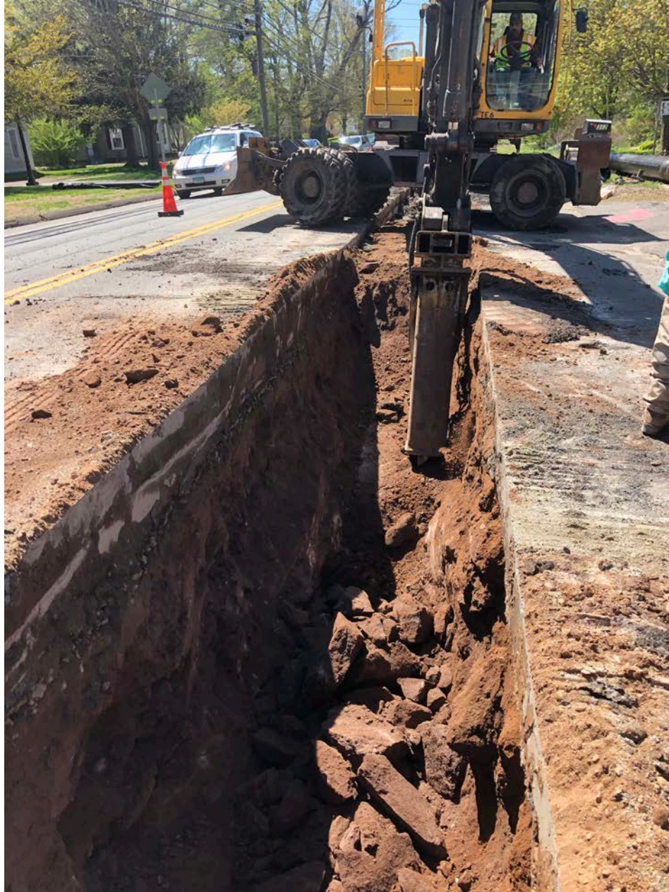
Picture 4: Ludlow hammering bedrock in trench at Station 177+25. View to the south. Durham, CT.
