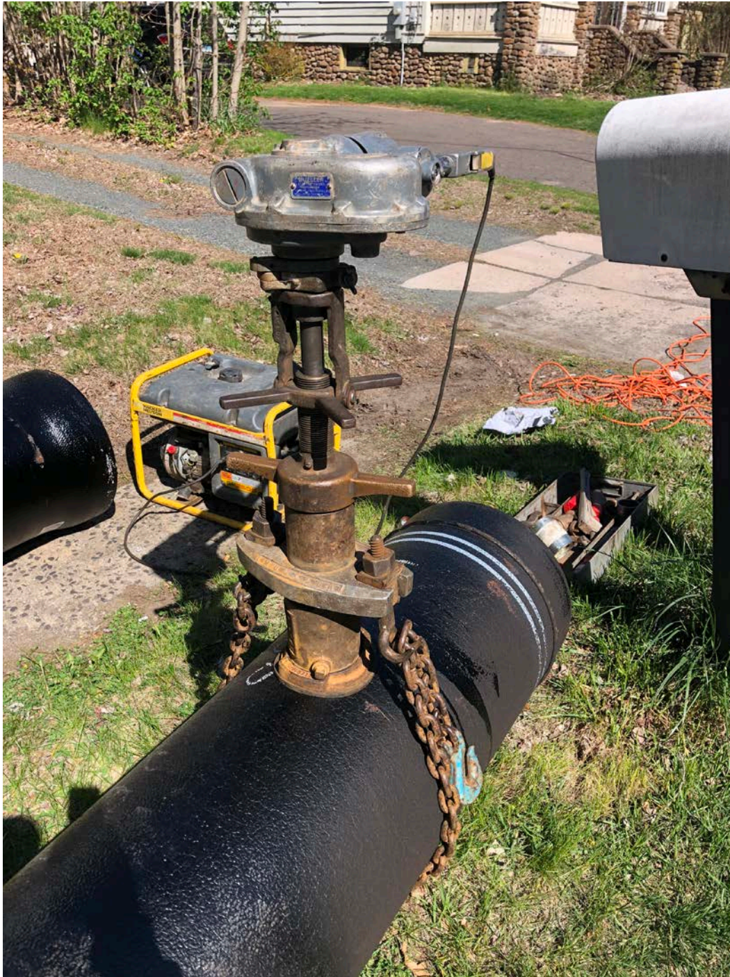
Picture 3: Ludlow in the process of tapping 16" DIP to place a 1" corporation stop. Main Street, Durham, CT.
