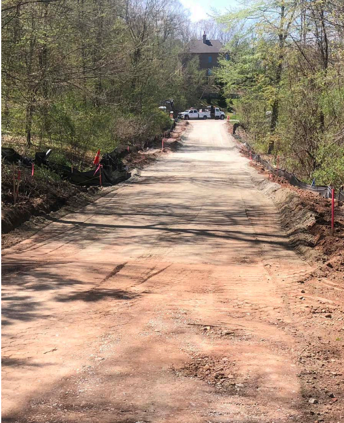
Picture 6: Shared access driveway after cutting, filling, grading, and compaction. View to the west. Middletown, CT.
