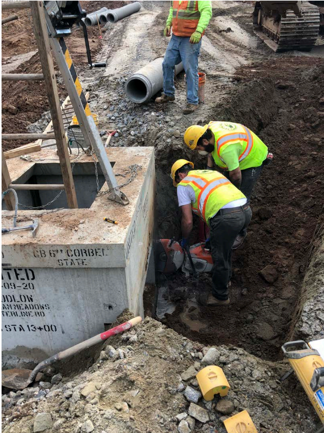
Picture 1: Ludlow cutting a hole in the south side of the catch basin located at Station 13+00 in order to connect 12" RCP. View to the east. Middletown, CT.
