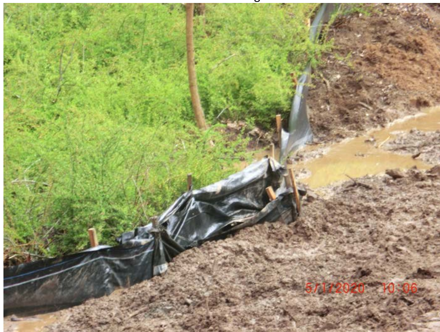
Figure 8: Potential issue Location A: Facing northeast. Approximately 50 feet east of large culvert. Small silt ponding behind silt fence. Trouble area reported by Ludlow and repaired/reinforced over last two days.
