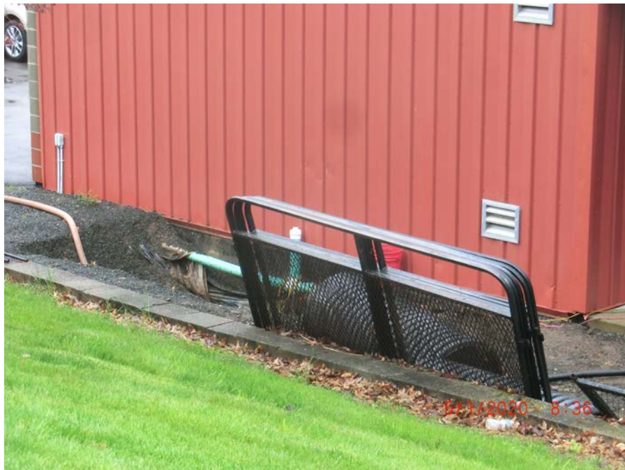
Picture 2: Durham Auto Center 4" Sch35 Perforated PVC drainpipe being installed or repaired along north side of building. Drain hose seen to left, not currently flowing.
