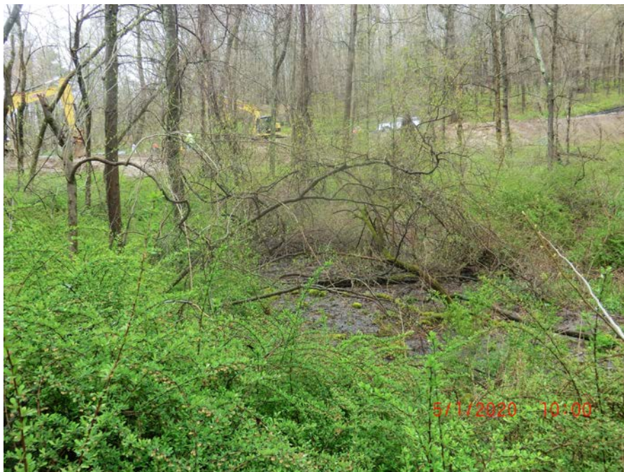
Figure 10: Facing south. Water flowing in drainage swale approximately 100 feet north of the Large culvert. Water is running clean with no indication of silt transport.
