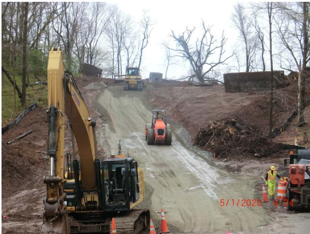
Picture 4: View facing east on shared access road. Laying road base and compaction on slope up to water tower.
