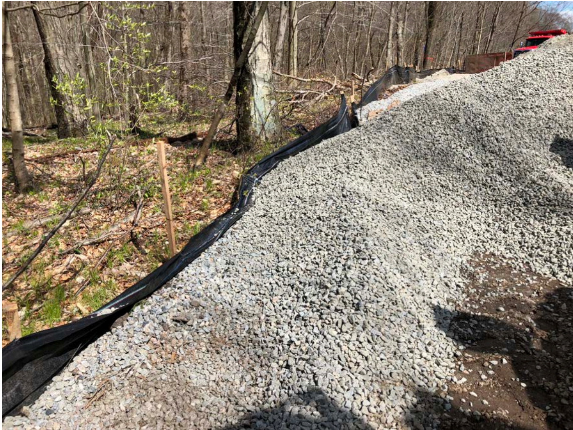
Picture 8: 3/4" stone crowding silt fence located on the north side of the shared access road. View to the northeast. Middletown, CT.
