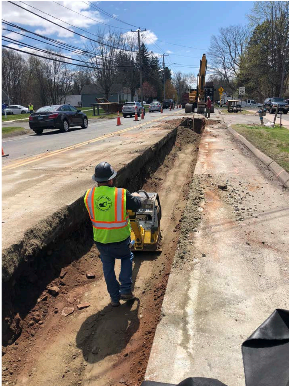
Picture 6: Ludlow compacting -3" gravel along the southbound lane of Main Street. View to the south. ~Station 171+50. Durham, CT.
