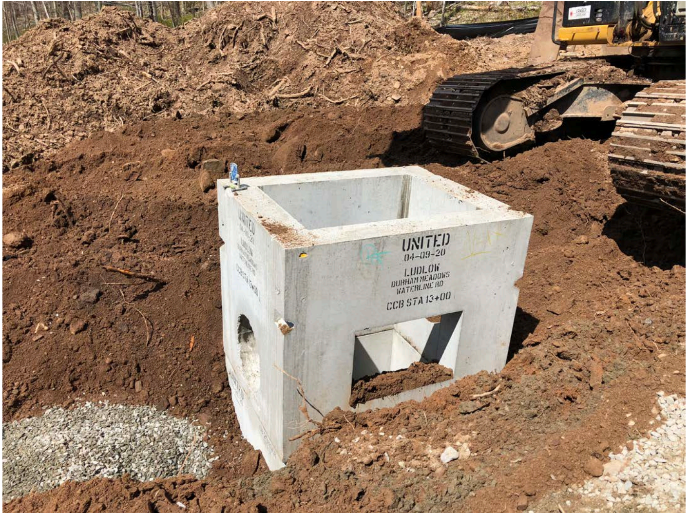
Picture 7: Type C catch basin Ludlow placed at Station 13+00. View to the north. Middletown, CT.
