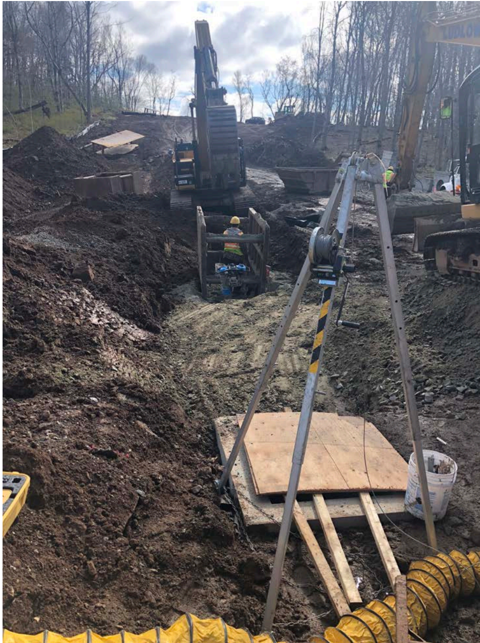
Picture 3: Ludlow placing 15" RCP east of the catch basin located on the north side of the shared access road at Station 14+40. View to the east. Middletown, CT.
