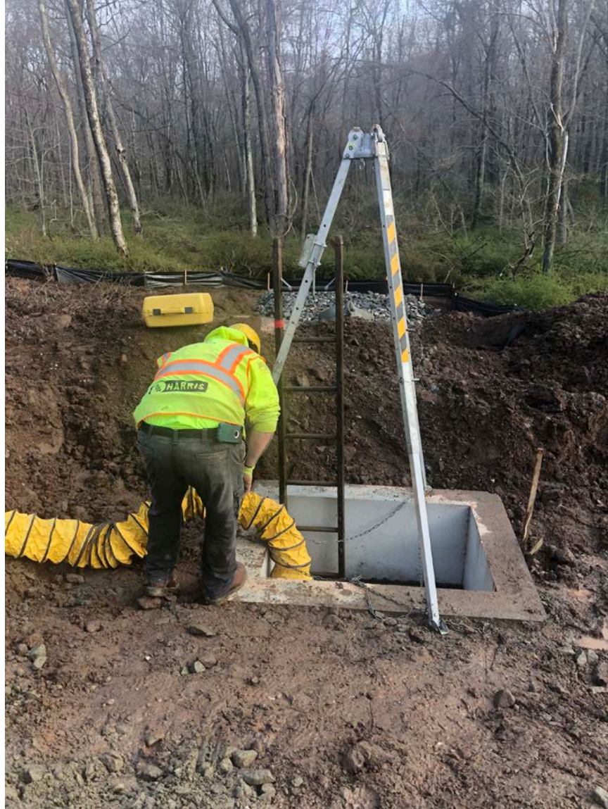
Picture 1: Ludlow preparing to make a confined space entry into the catch basin located on the north side of the shared access road at Station 14+40. View to the north. Middletown, CT.
