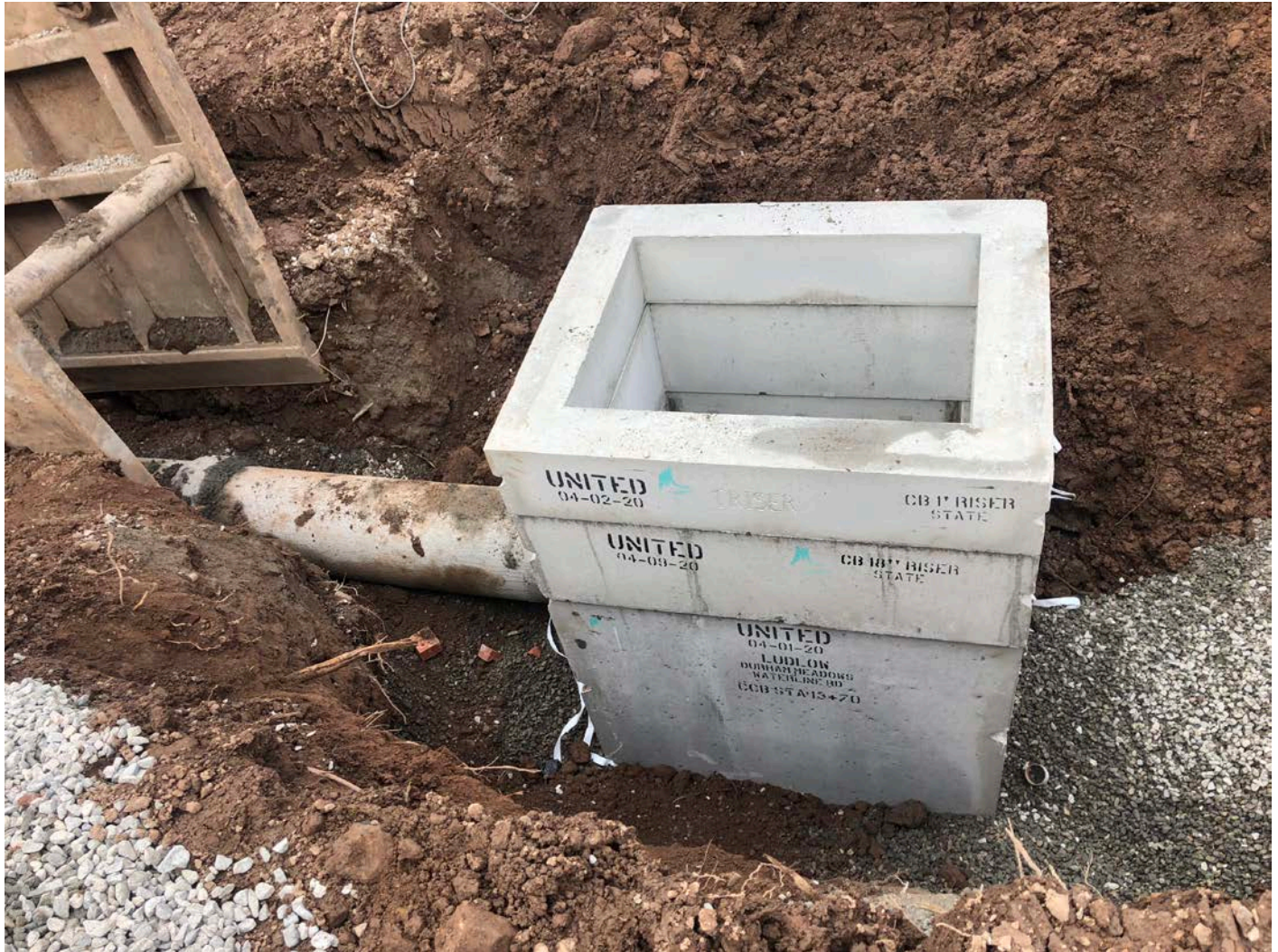
Picture 5: Type C catch basin Ludlow placed at Station 13+70. View to the north. Middletown, CT.
