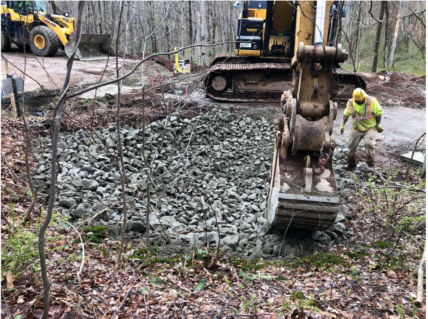
Picture 8: Ludlow placing riprap in the plunge bowl located between the driveways for 224 and 216 Talcott Ridge Drive. View to the north. Middletown, CT.
