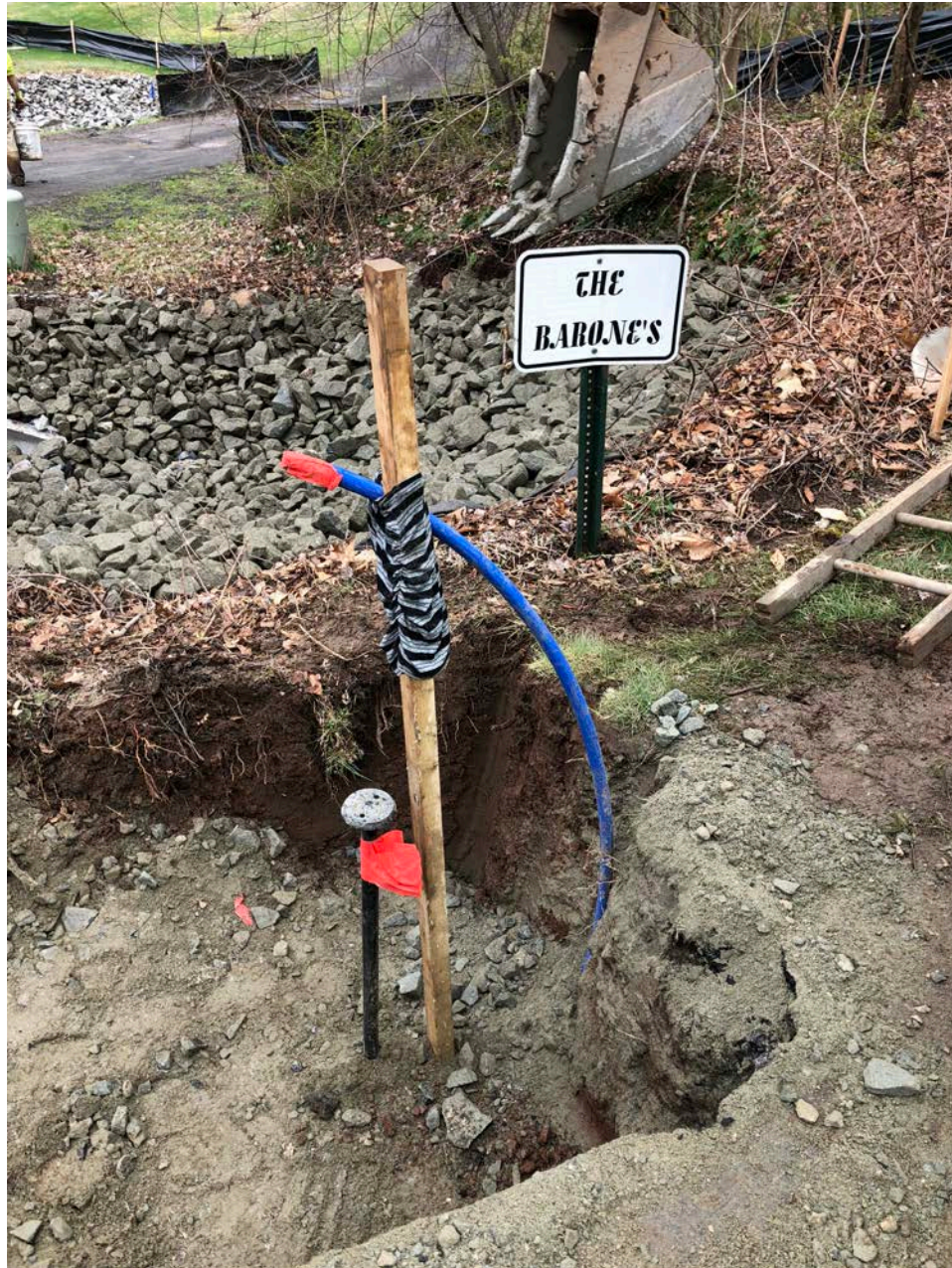
Picture 7: Valve stem associated with the curb stop installed for 224 Talcott Ridge Drive. View to the southeast. Middletown, CT.
