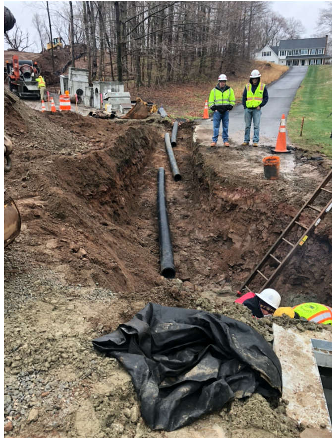
Picture 1: 8" corrugated black plastic pipe from the east edge of the driveway for 214 Talcott Ridge Drive into the catch basin located at Station 14+40 on the south side of the shared access road. Placement of 8" View to the southeast. Middletown, CT.
