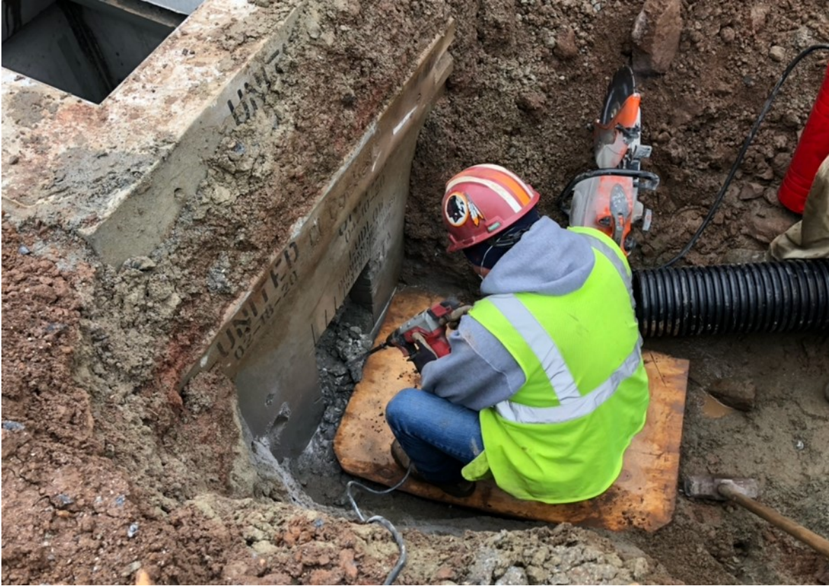
Picture 2: Ludlow cutting hole in side of catch basin to receive 8" corrugated black plastic pipe from the east edge of the driveway for 214 Talcott Ridge Drive. Middletown, CT.
