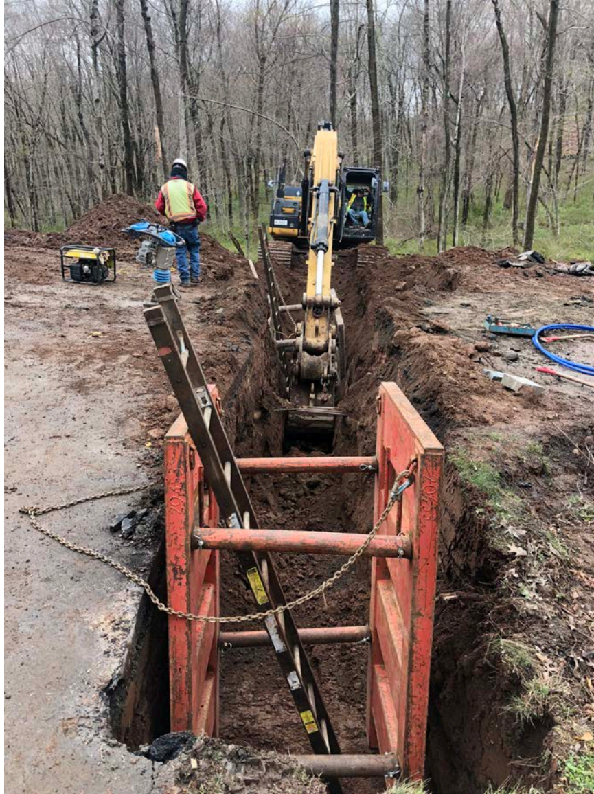
Picture 6: Ludlow trenching across the shared access road adjacent to the driveway for 224 Talcott Ridge Drive in order to tap the 20" water line to add a corporation stop. View to the north. Middletown, CT.
