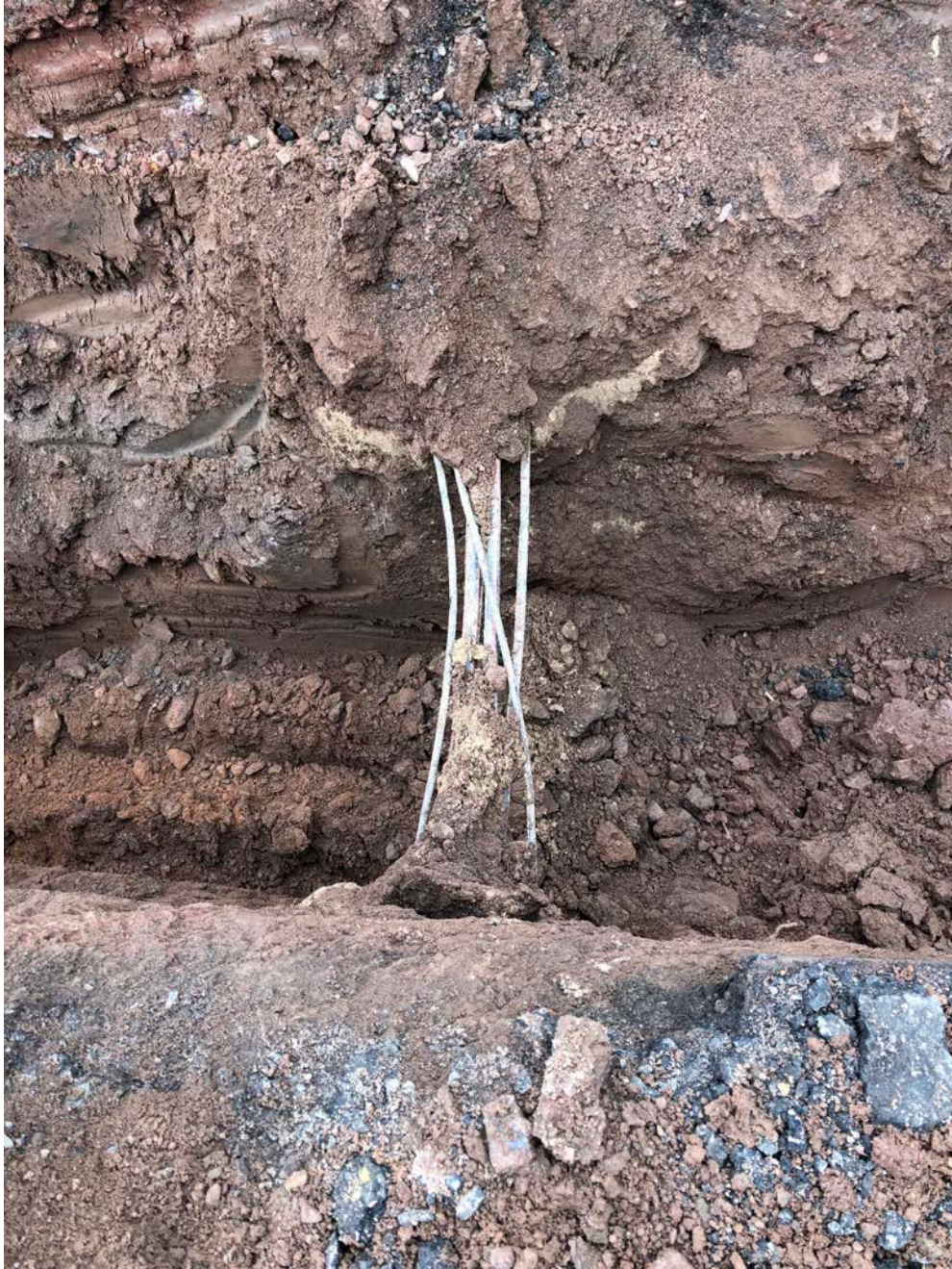
Picture 5: Communication and power lines daylighted by Ludlow adjacent to the driveway for 224 Talcott Ridge Drive. Middletown, CT.
