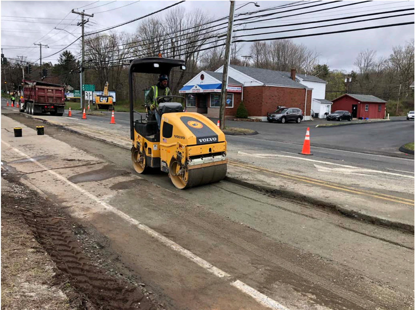
Picture 9: Ludlow compacting backfill at ~Station 168+00. View to the northeast. Durham, CT.
