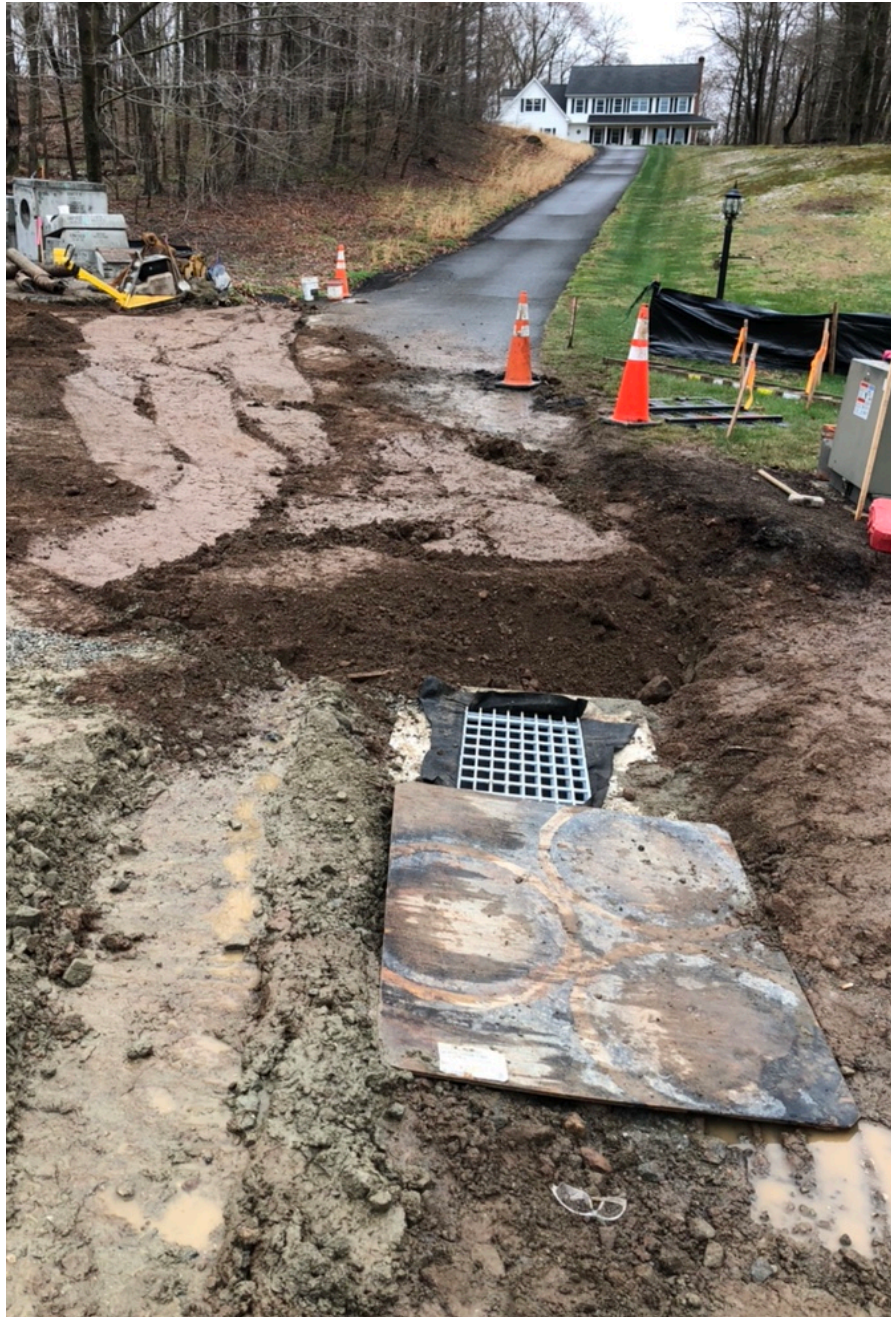
Picture 3: Trench closed up after installation of 8" corrugated black plastic pipe from the east edge of the driveway for 214 Talcott Ridge Drive into the catch basin located at Station 14+40. View to the southeast. Middletown, CT.
