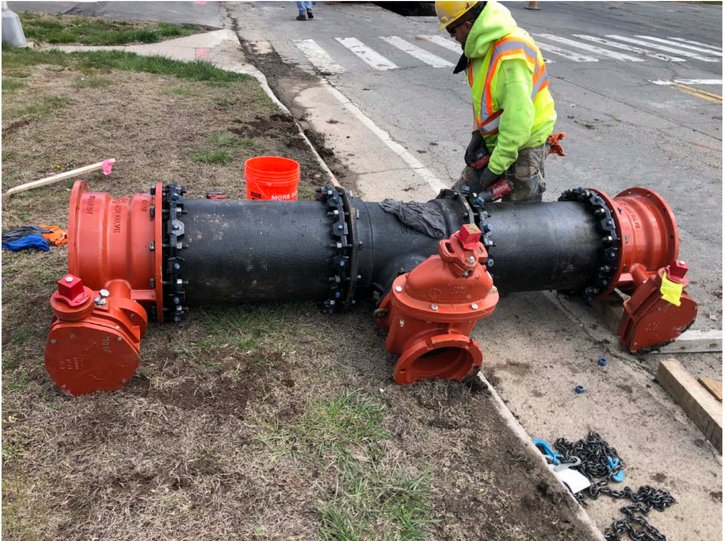
Picture 6: 16"x16"x8" M.J. C.L.D.I. Tee with two 16" butterfly valves and one 8" gate valve and a valve box that was placed at Station 166+32 (Haddam Quarter Road intersection).
