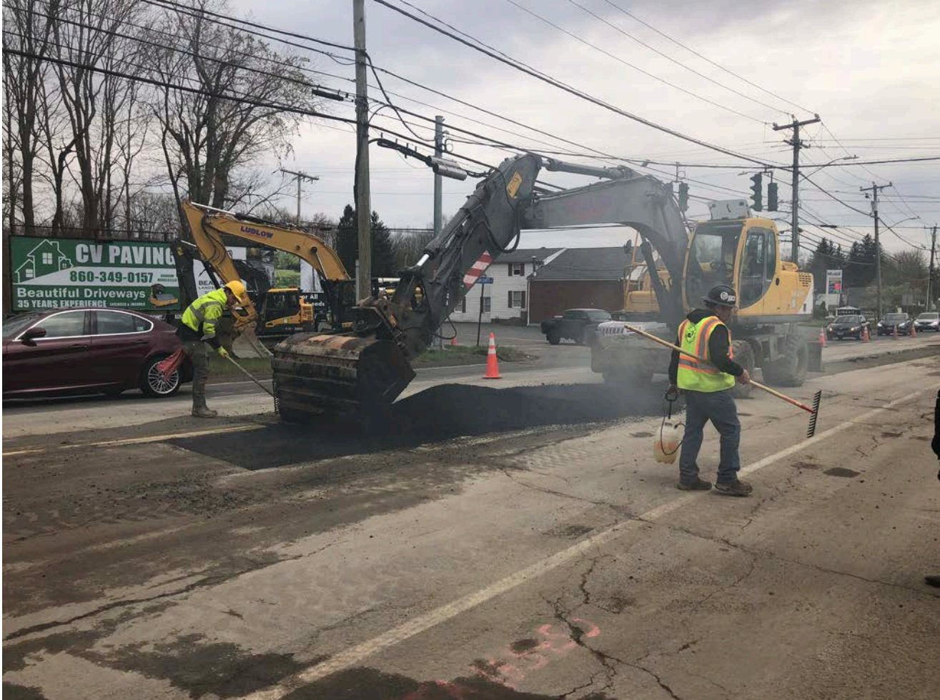
Picture 8: Ludlow placing hot patch over compacted soil on Main Street. View to the southeast.
