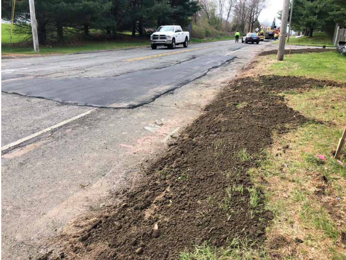
Picture 4: Newly placed loam and shim coating of asphalt on South Main Street, just south of the intersection with Talcott Ridge Drive. View to the south.
