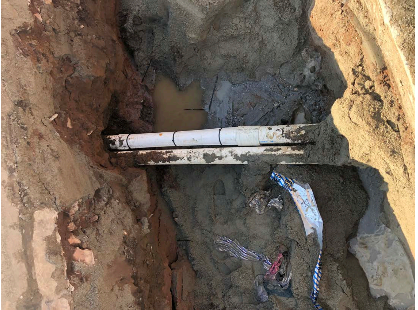
Picture 2: Communications cable conduit repaired by Ludlow at Station 165+78.
