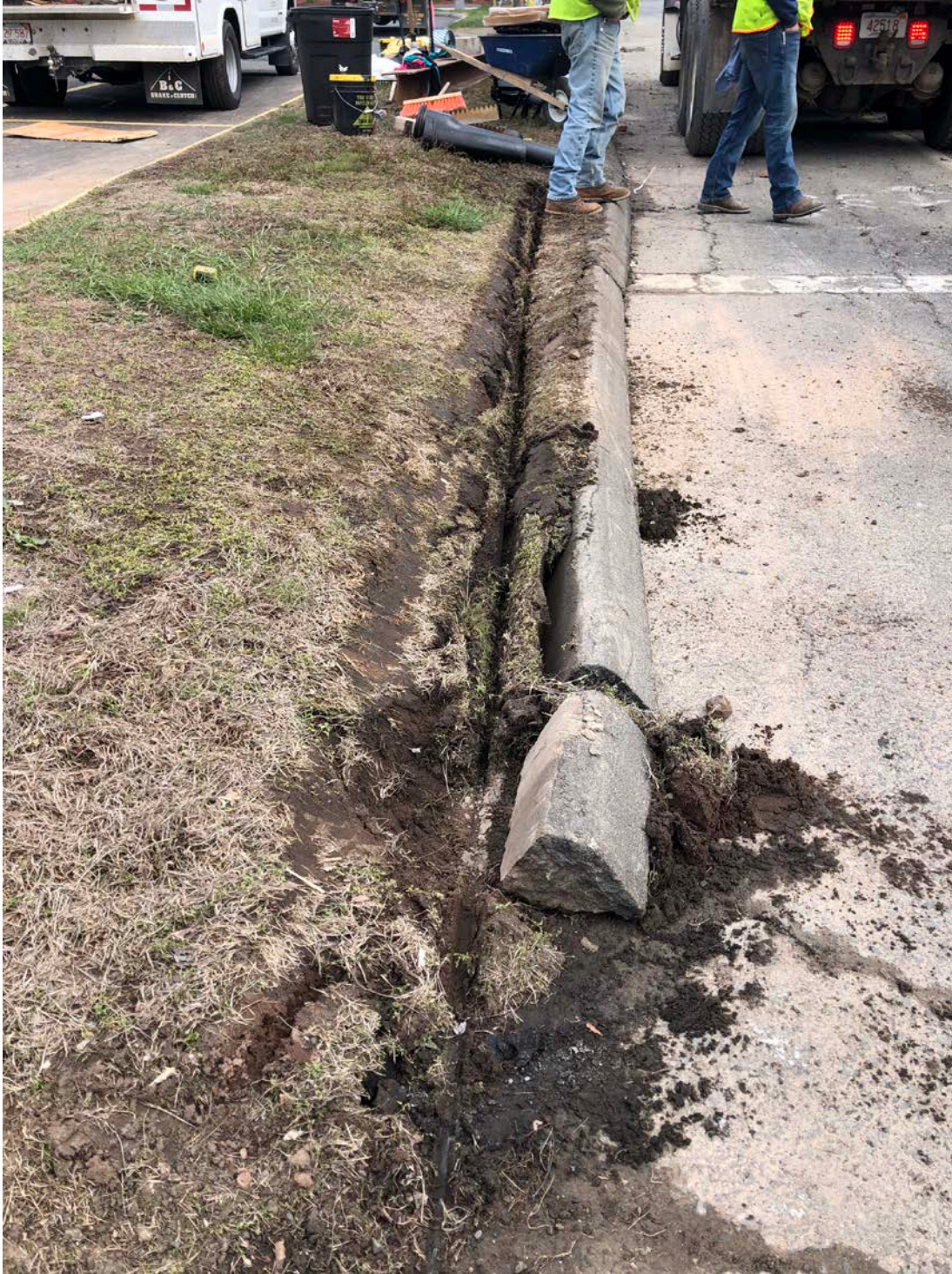
Picture 5: Damage to curbing at ~Stations 166+20 to 166+35. View to the north.
