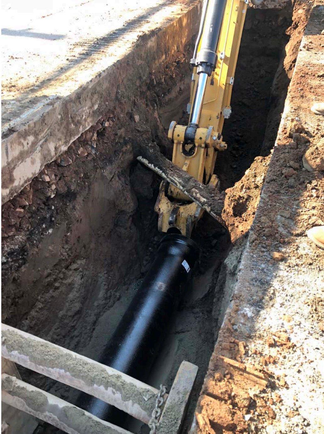
Picture 3: 16" DIP placed below communications cable located at ~Station 166+05. View to the south.
