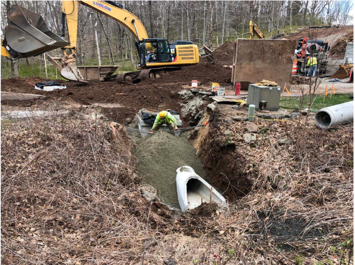
Picture 7: Ludlow placing sand over 18" RCP at Station 14+40. View to the north.
