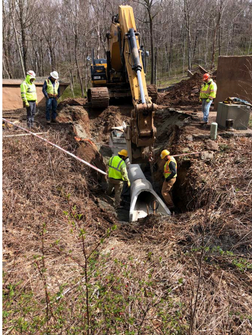
Picture 5: Ludlow placing 18" RCP into Type CL catch basin they installed earlier today. View to the north.
