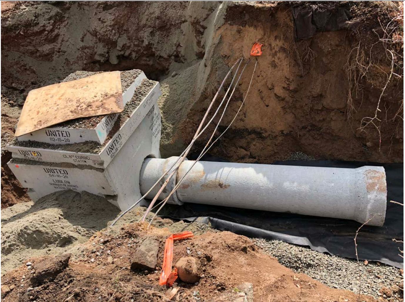
Picture 4: Type CL catch basin placed at Station 14+40, with 18" RCP placed to the right. Note exposed power, telephone and CATV cables. View to the east.
