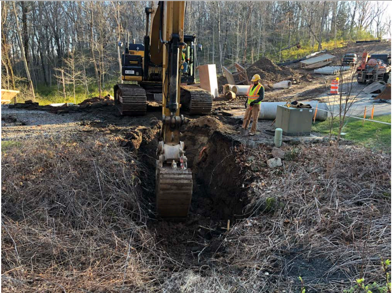
Picture 1: Ludlow begins excavation for Type CL catch basin that will be installed at ~Station 14+40. View to the northeast.
