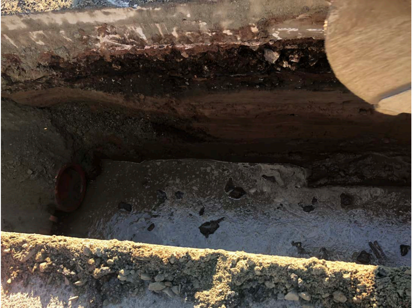
Picture 3: Water observed in trench at Station 164+19 after Ludlow daylighted the southern end of yesterday's pipe placement.
