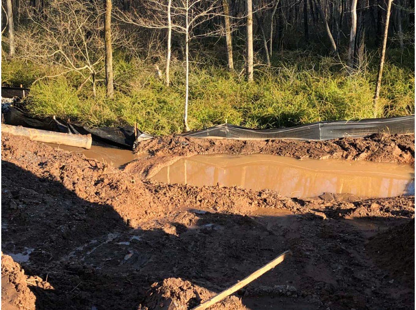
Picture 2: Water and soil accumulated against the silt fence located east of Station 14+40, prior to Ludlow cleaning along the silt fence. View to the north.
