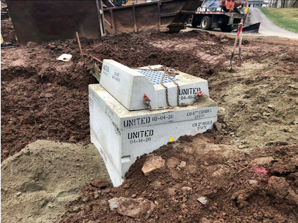
Picture 1: Type C catch basin that was installed at Station 14+40 on April 20, 2020. View to the southeast.
