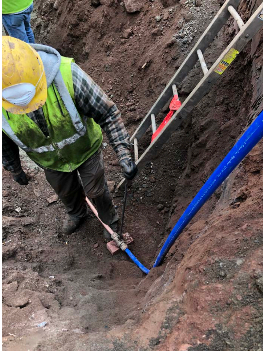
Picture 7: 1" plastic pipe connected to 1" copper pipe for service connection to 216 Talcott Ridge Drive.
