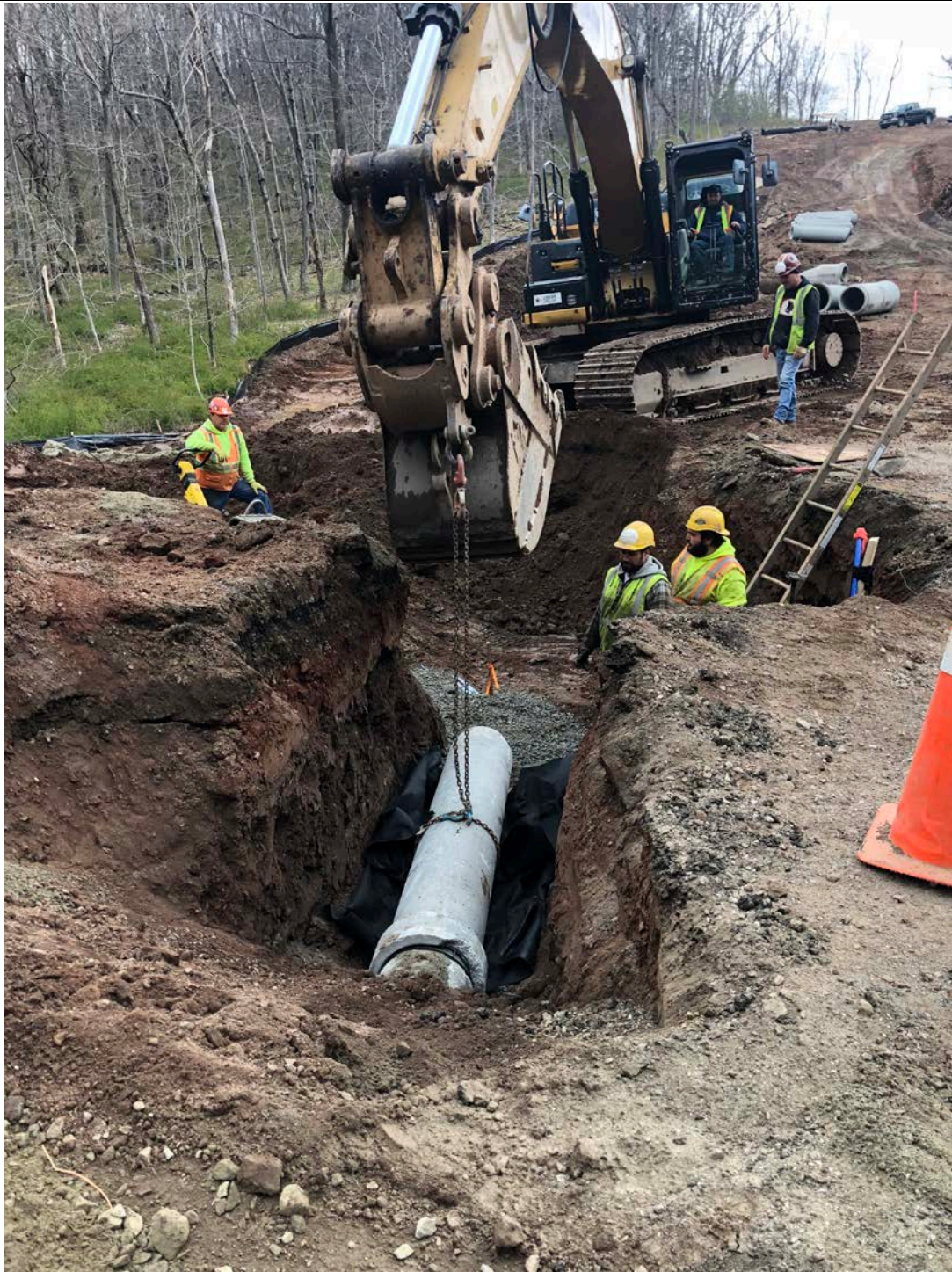
Picture 8: Placing RCP storm drain culvert at ~Station 15+00. View to the northeast.
