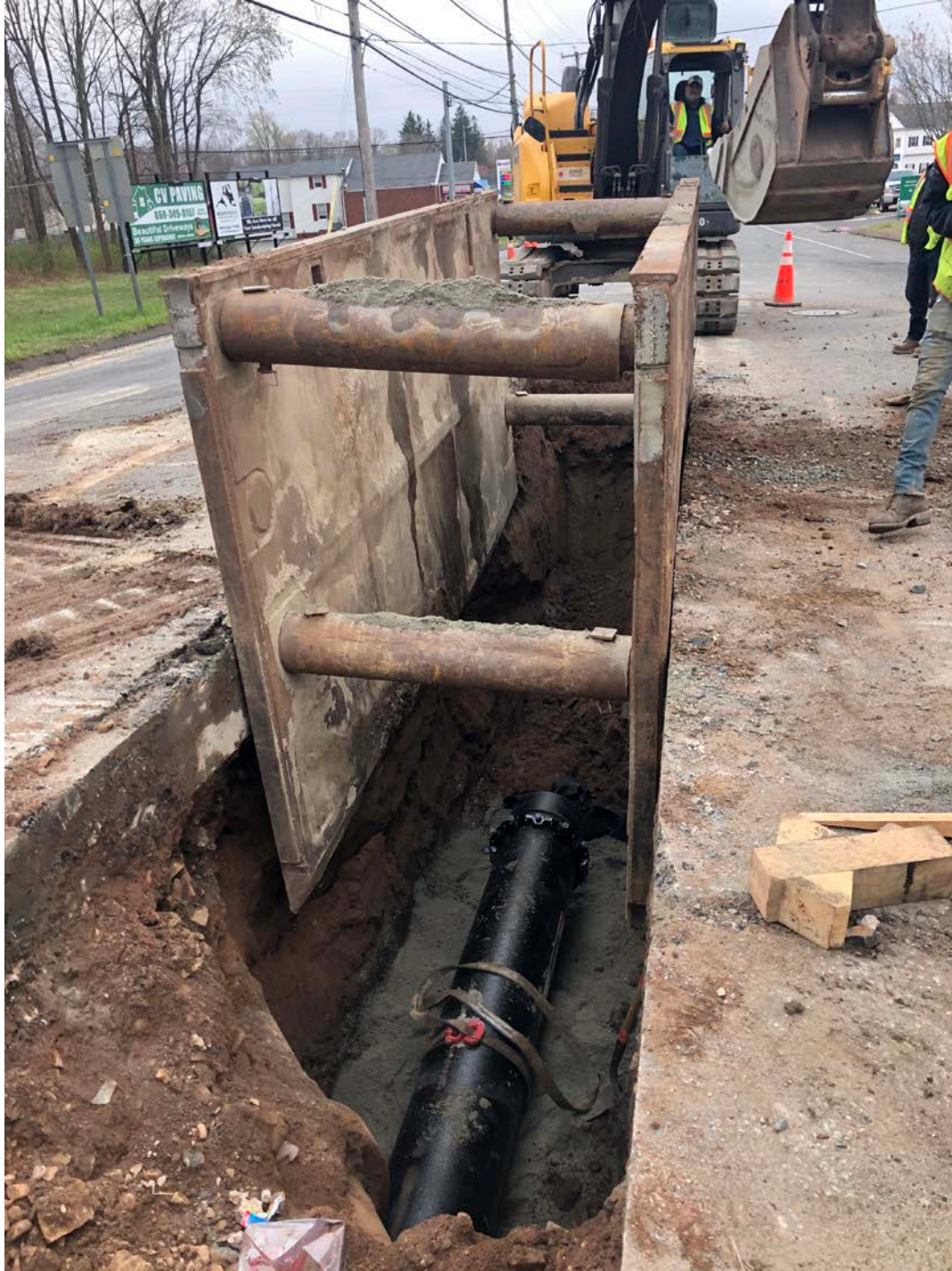
Picture 3: Position of trench box just after the USACE representatives directed Ludlow personnel out of the trench so the box could be placed deeper and provide more safety. View to the south.
