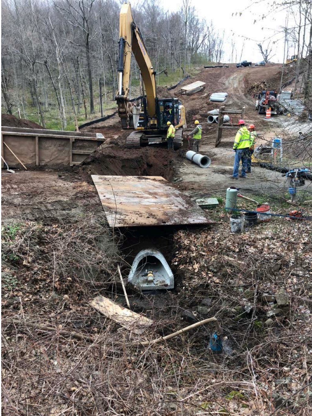
Picture 2: Culvert placed on the south side of the tank access road between the driveways for 224 and 216 Talcott Ridge Drive at ~Station 15+10. View to the northeast.
