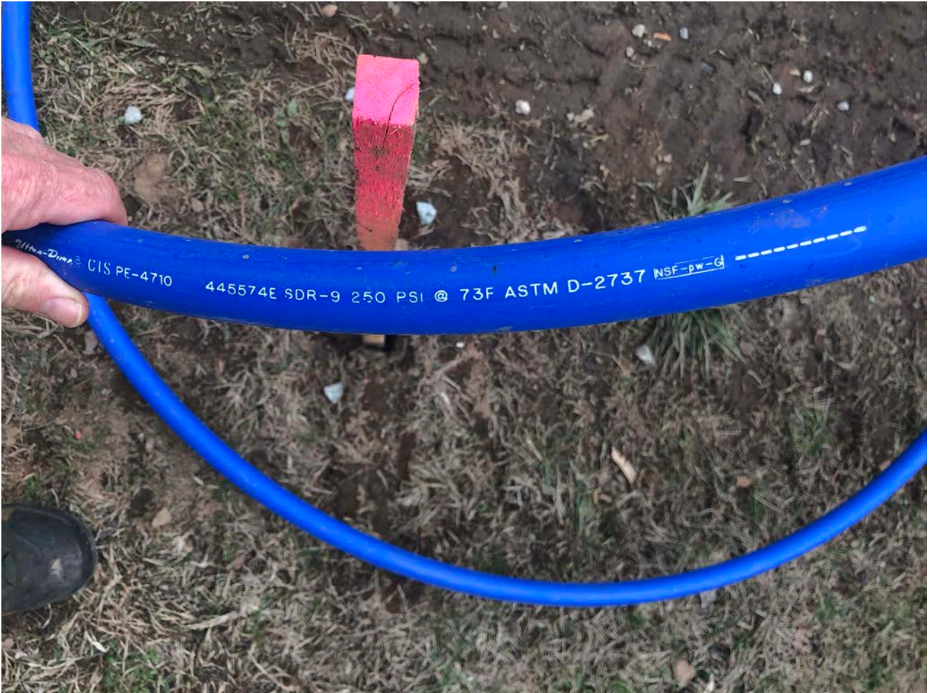
Picture 6: 1" plastic pipe used in conjunction with 1" copper pipe for service connection to 216 Talcott Ridge Drive.
