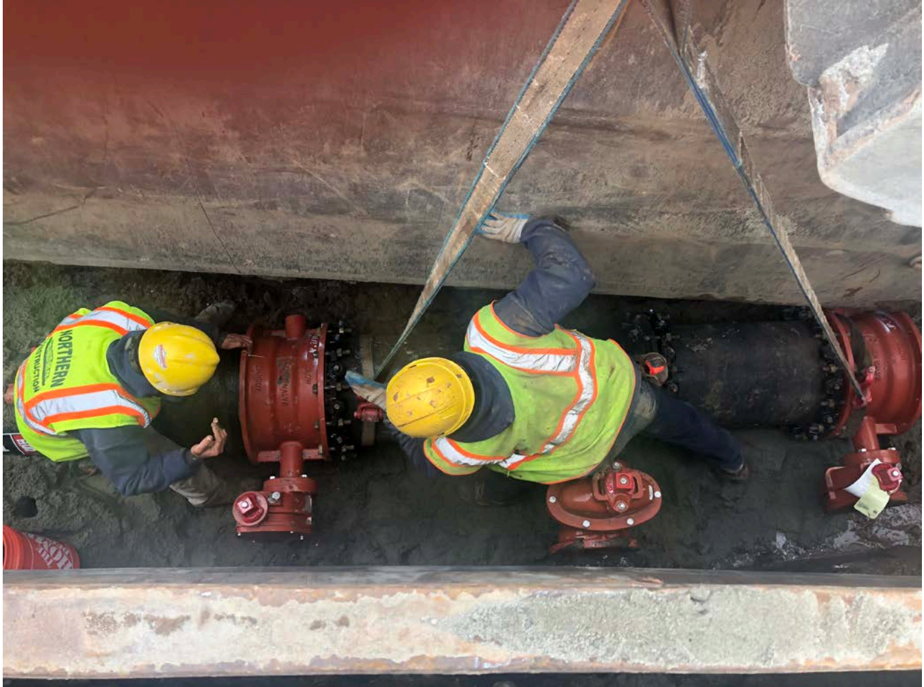
Picture 5: Ludlow installing two sections of 16" DIP that connect two 16" M.J. butterfly valves and a 16"x16"x8" M.J. C.L.D.I.
