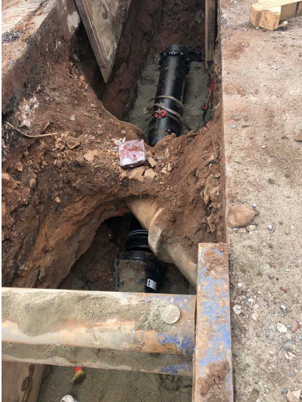
Picture 4: 16" DIP placed beneath storm drain pipe at the intersection of Main Street and Route 147 West. View to the south.
