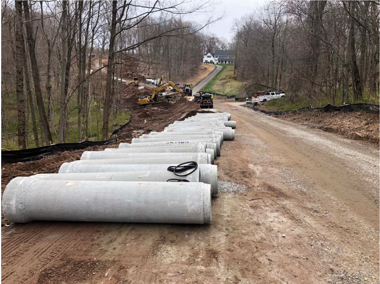
Picture 3: RCP staged along the tank access road. View to the east.
