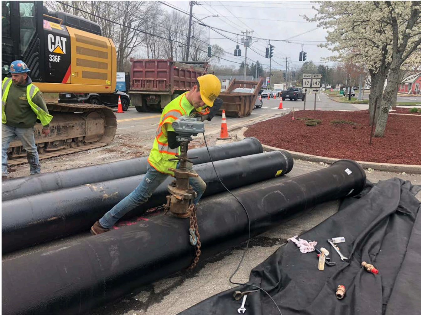
Picture 6: Ludlow tapping holes for curb stops on pipe that will be installed near Station 163+00.
