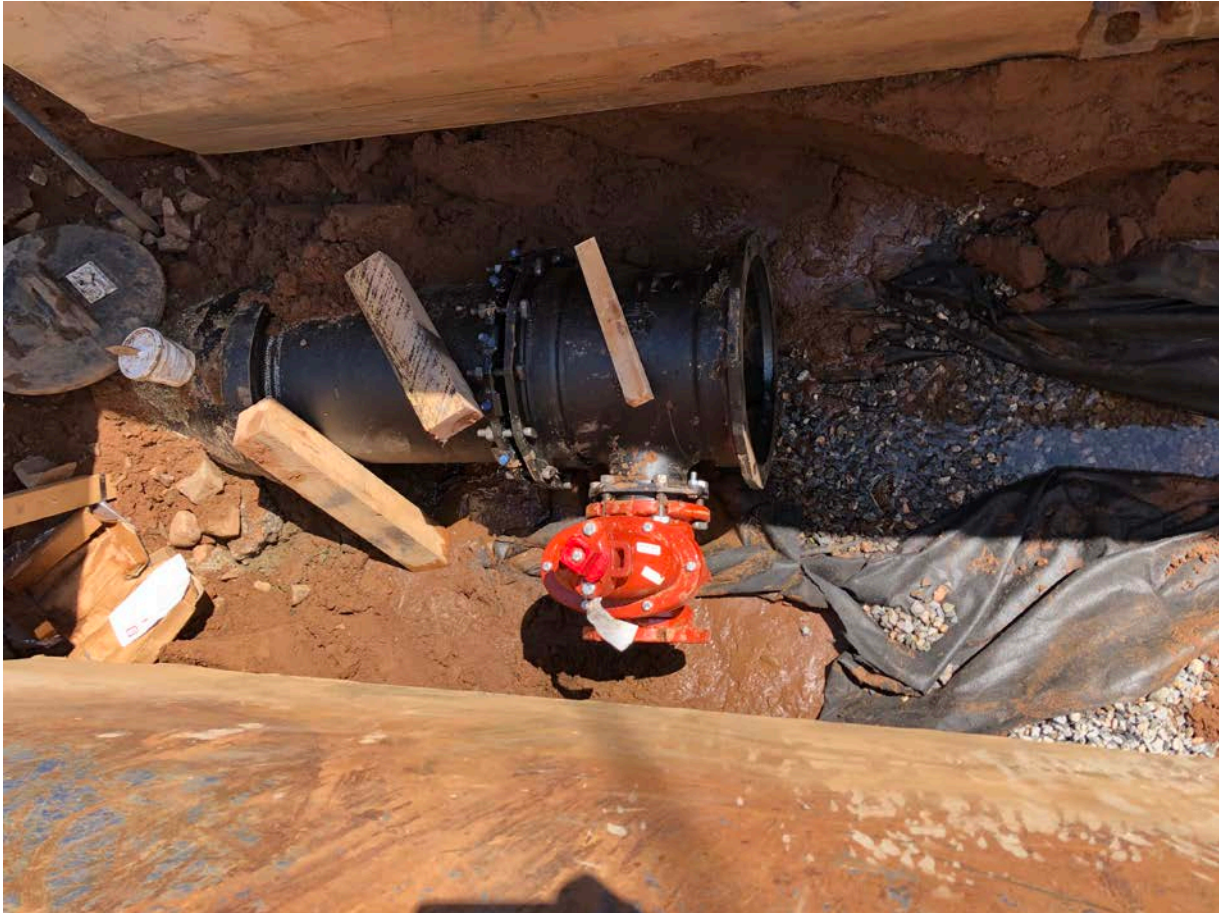
Picture 9: Tee and valve box installed at Station 160+90 for future installation of fire hydrant assembly.
