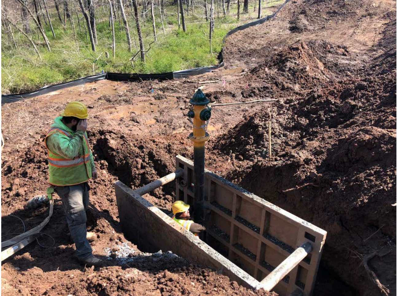
Picture 4: Ludlow preparing to install a hydrant assembly today at Station 14+69. View to the southeast.
