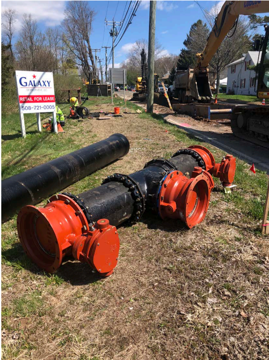
Picture 6: Butterfly valves and piping that were installed from Station 161+10 to Station 161+18.
