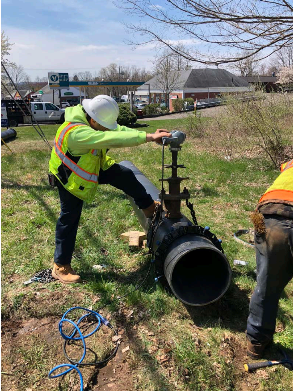
Picture 8: Ludlow tapping 16" DIP to install fitting for curb stop at ~Station 161+05.
