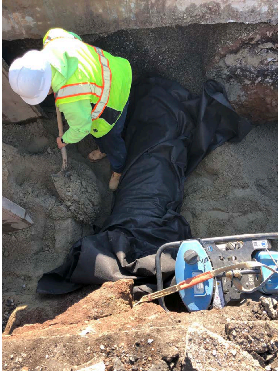
Picture 3: Section of metal storm drain pipe with holes corroded through its walls that Ludlow has wrapped in filter fabric prior to backfilling at ~Station 160+20.
