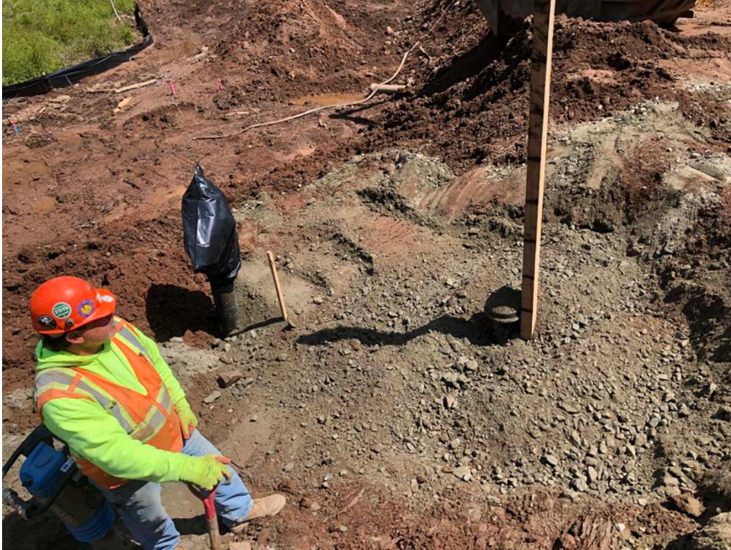
Picture 10: Hydrant assembly being backfilled at Station 14.69.
