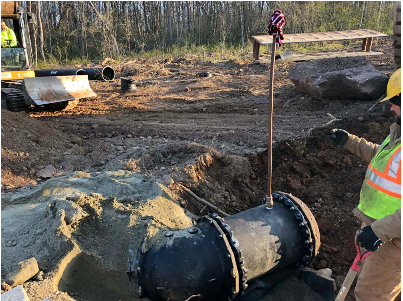
Picture 1: Ludlow placing temporary air release on 20" DIP at the top of the tank access road in order to perform pressure test.
