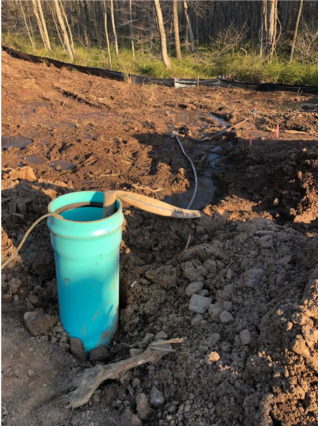
Picture 2: Ludlow pumping water from a temporary dewatering well placed at ~Station 15+00.
