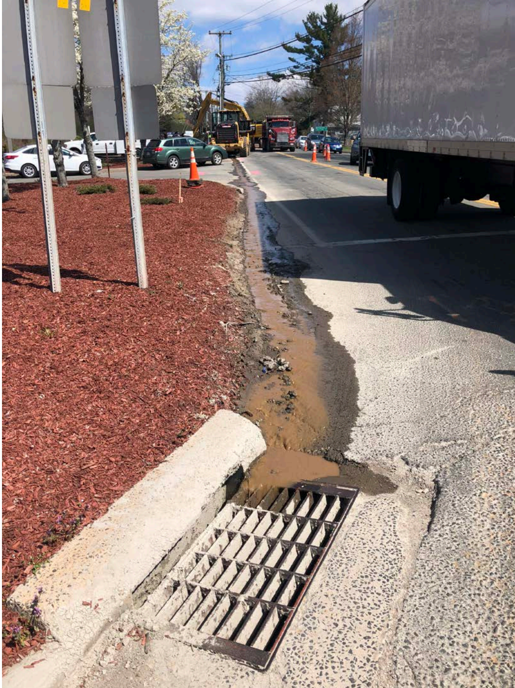
Picture 7: Water being pumped from excavation at ~Station 160+90 and being discharged to catch basin on the corner of Main Street and Route 147.
