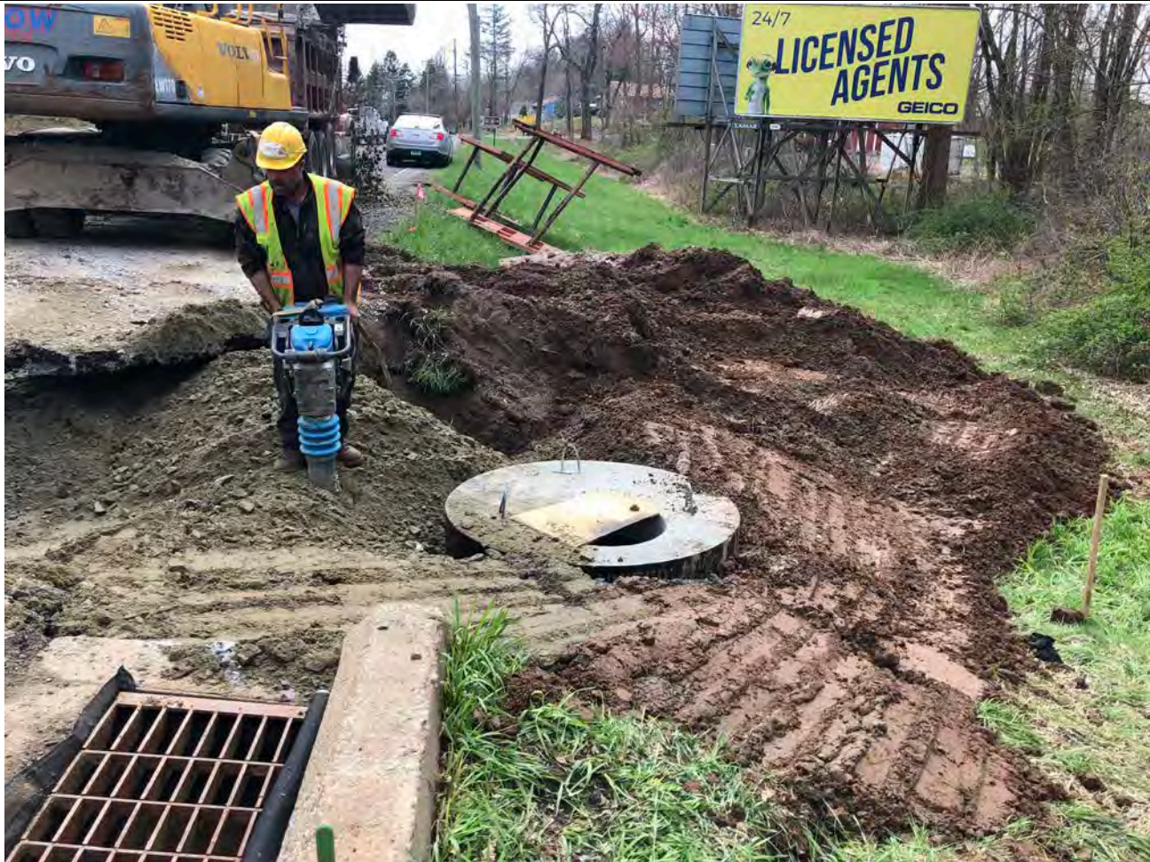
Picture 11: Compacting soil around the Manual Water Main Drain. View to the south.
