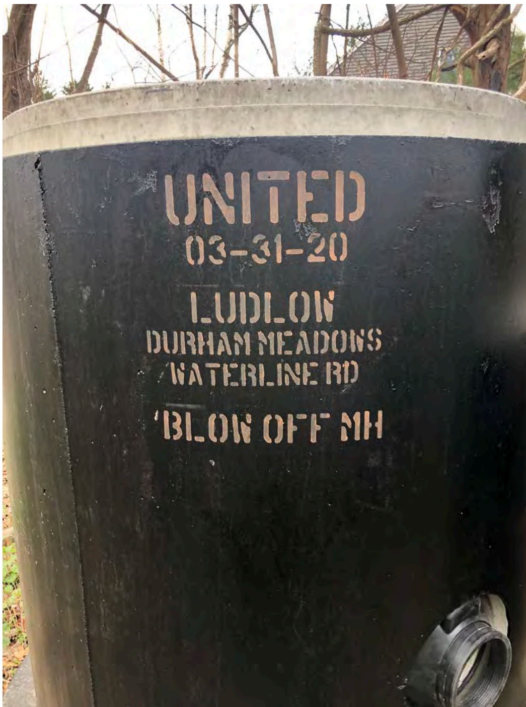
Picture 3: Lower section of Manual Water Main Drain that was installed at Station 137+73.
