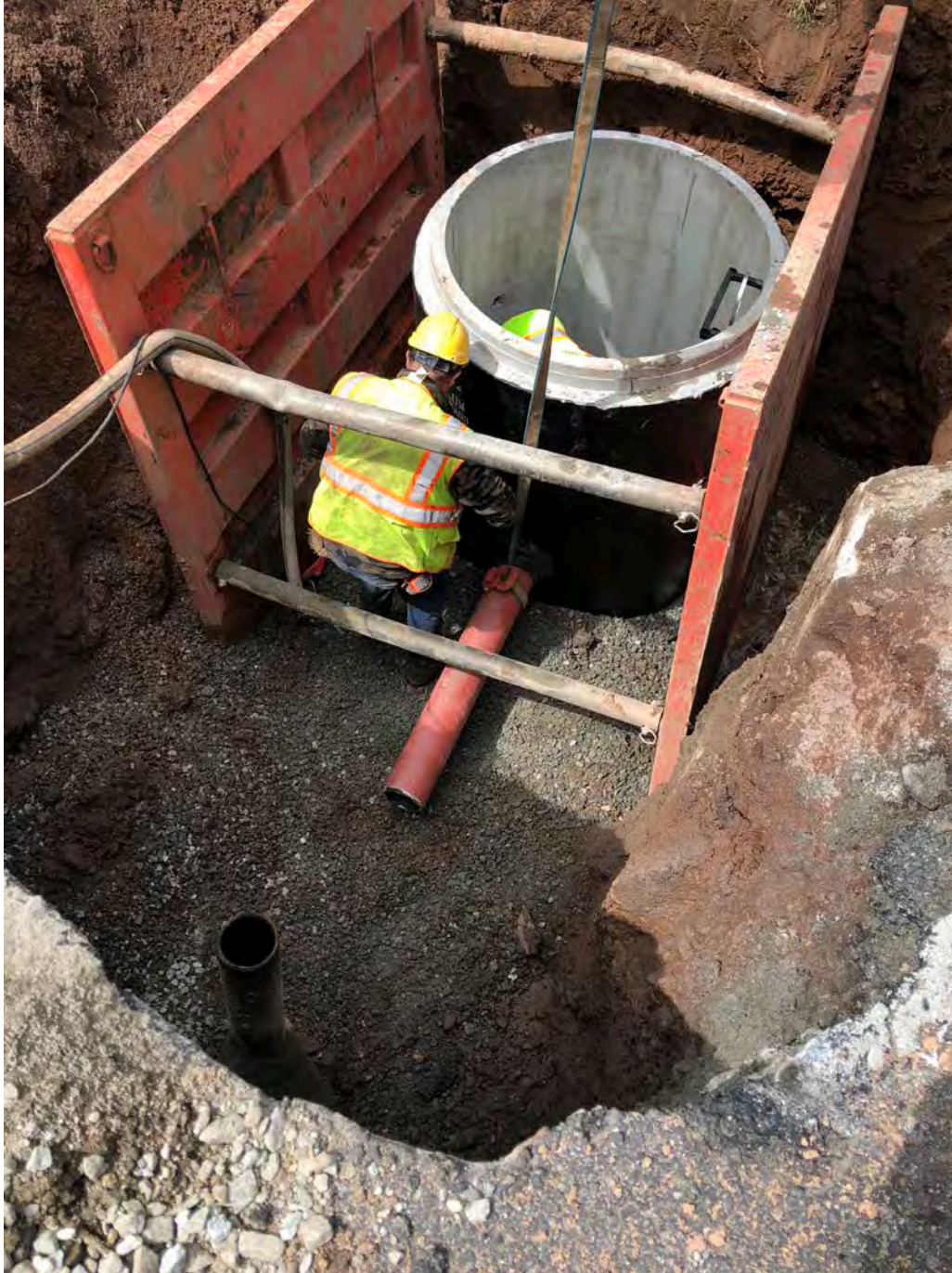
Picture 9: 6" DIP being placed to connect the lower portion of the Manual Water Main Drain to the valve box.
