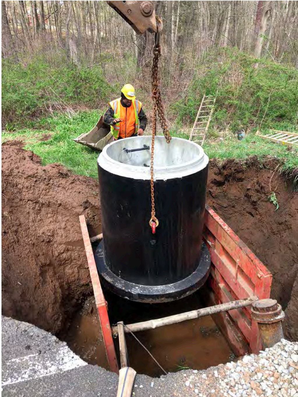
Picture 8: Lower portion of the Manual Water Main Drain being placed. View to the west.
