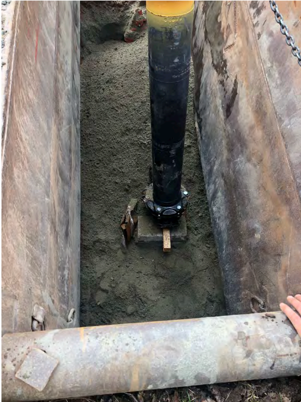
Picture 2: Blocks placed beneath hydrant assembly at Station 128+50.
