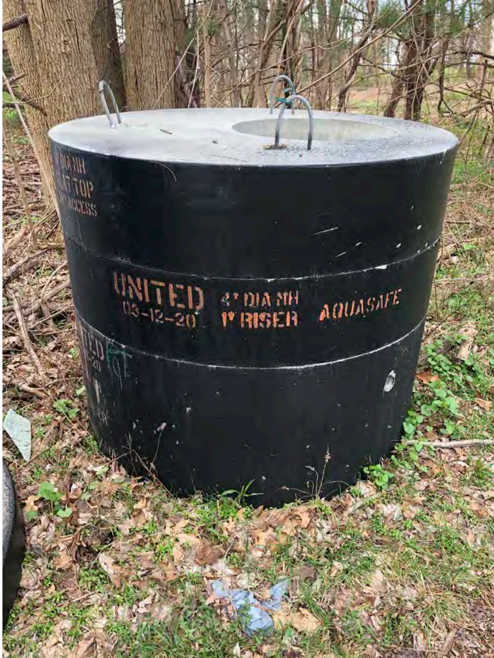
Picture 4: Upper sections of Manual Water Main Drain that was installed at Station 137+73.
