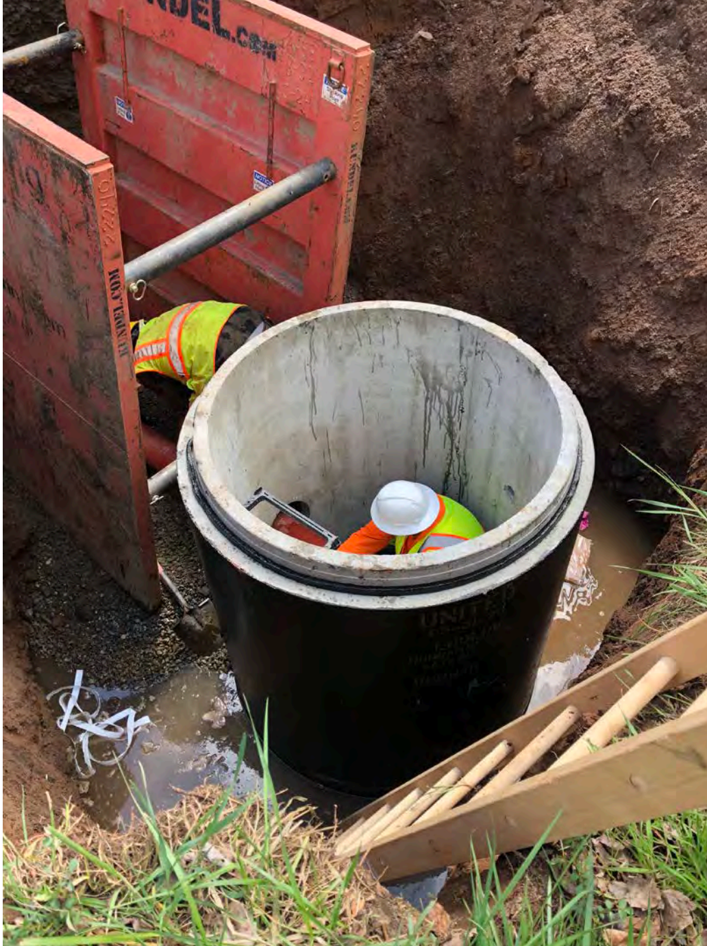
Picture 10: Chemseal gasket placed along the top rim of the lower portion of the Manual Water Main Drain.
