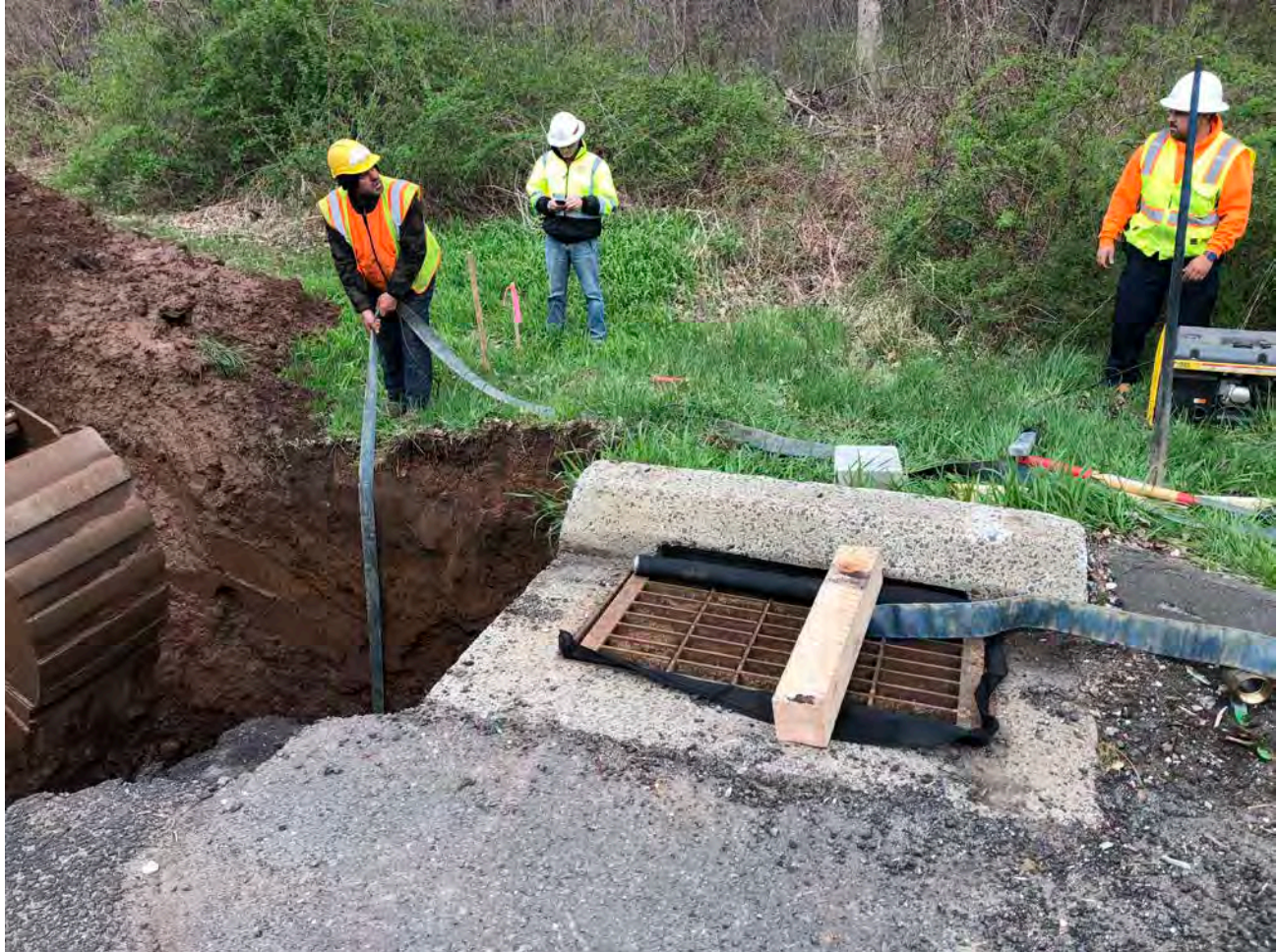
Picture 6: Ludlow pumping water from excavation at Station 137+73 into adjoining catch basin.
