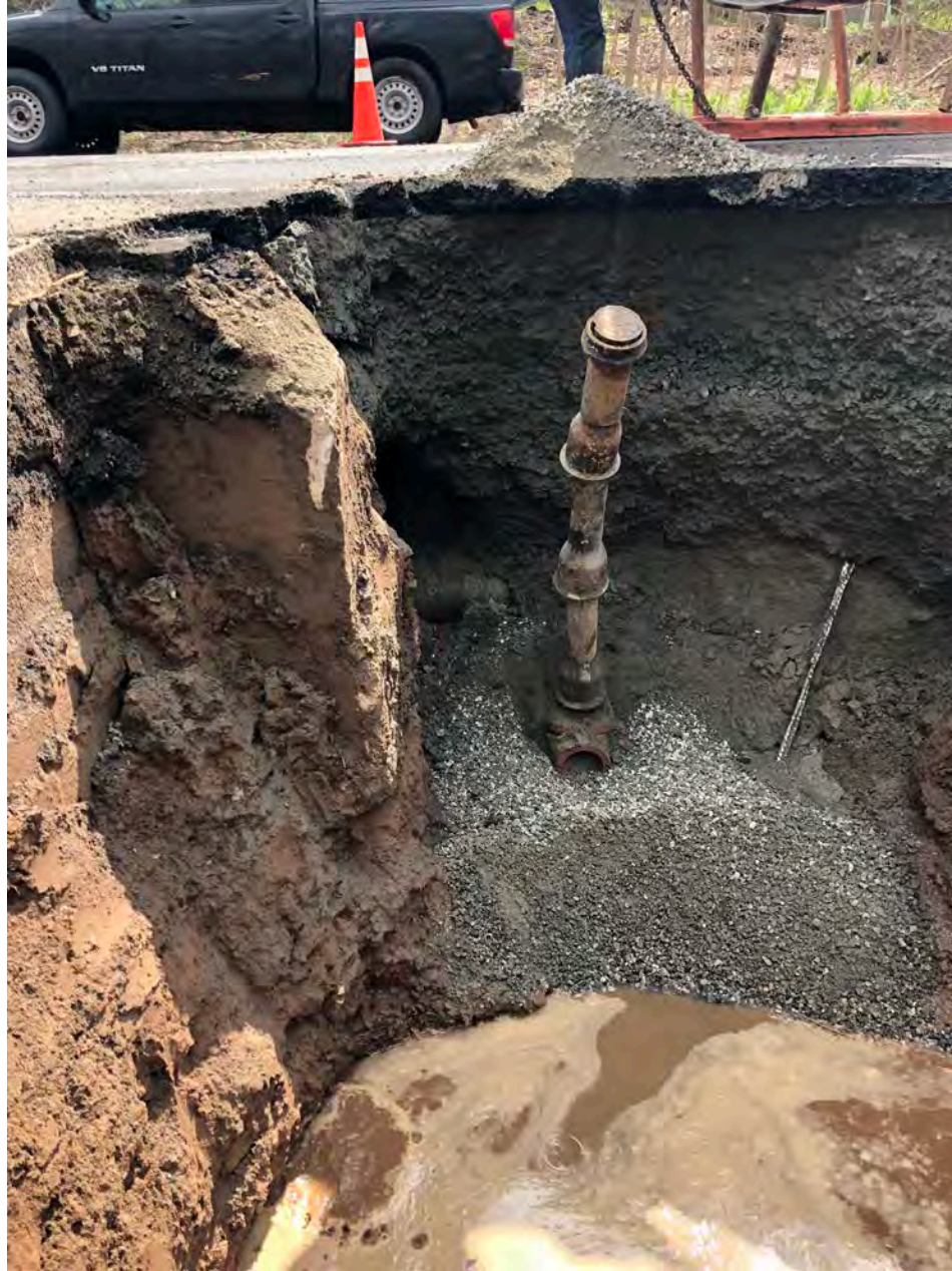
Picture 7: Valve box exposed by excavation activities at Station 137+73. View to the east.
