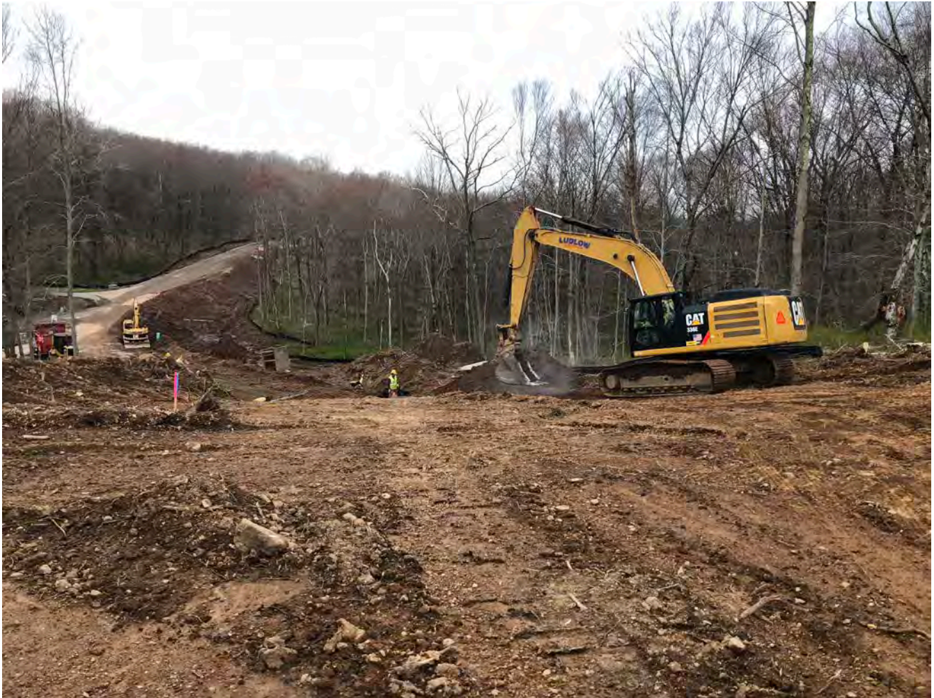
Picture 1: Ludlow placing 20" DIP at the tank access road; approaching the tank pad. View to the northwest.
