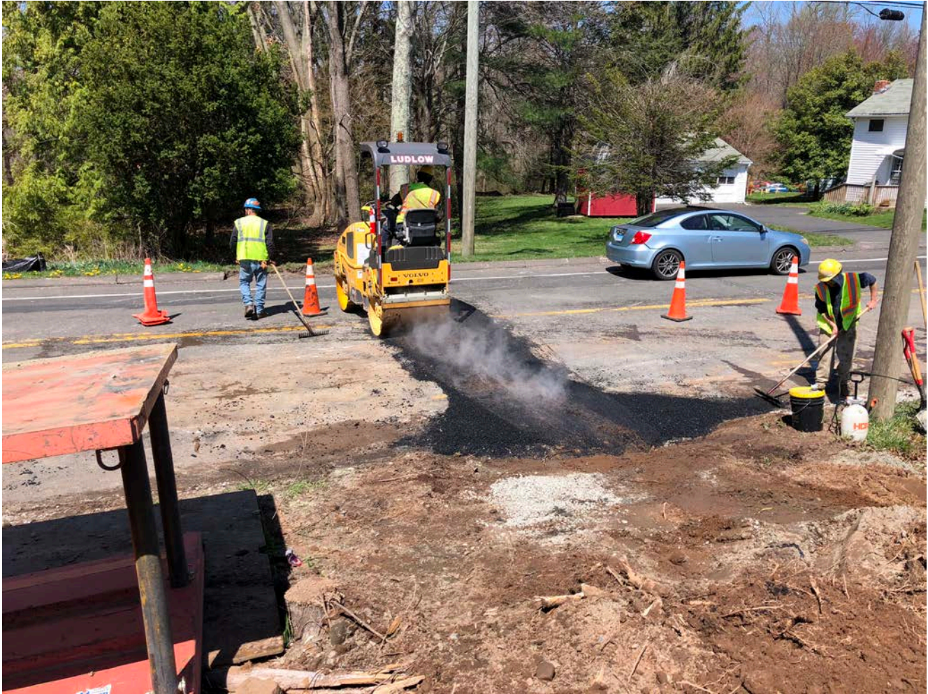
Picture 5: Ludlow placing hot patch at Station 124+71.
