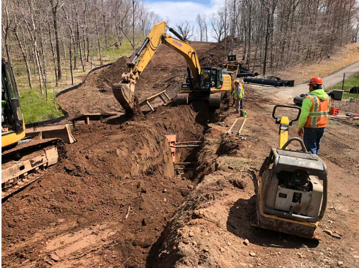
Picture 9: Overview of 20" DIP installation on the tank access road. View to the south.
