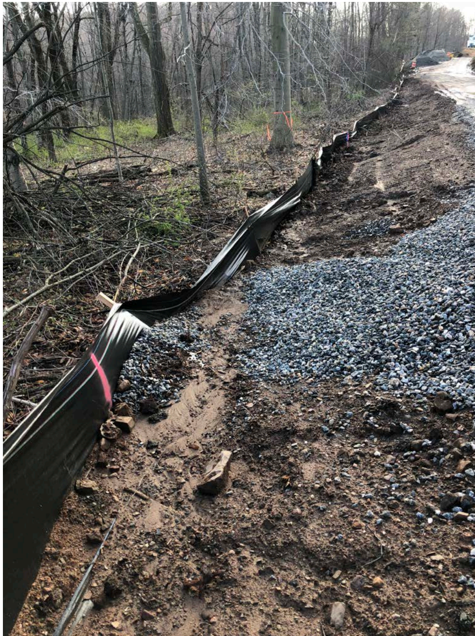
Picture 2: Silt collected on the up-slope side of silt fence that runs along the tank access road. View to the south/southeast.
