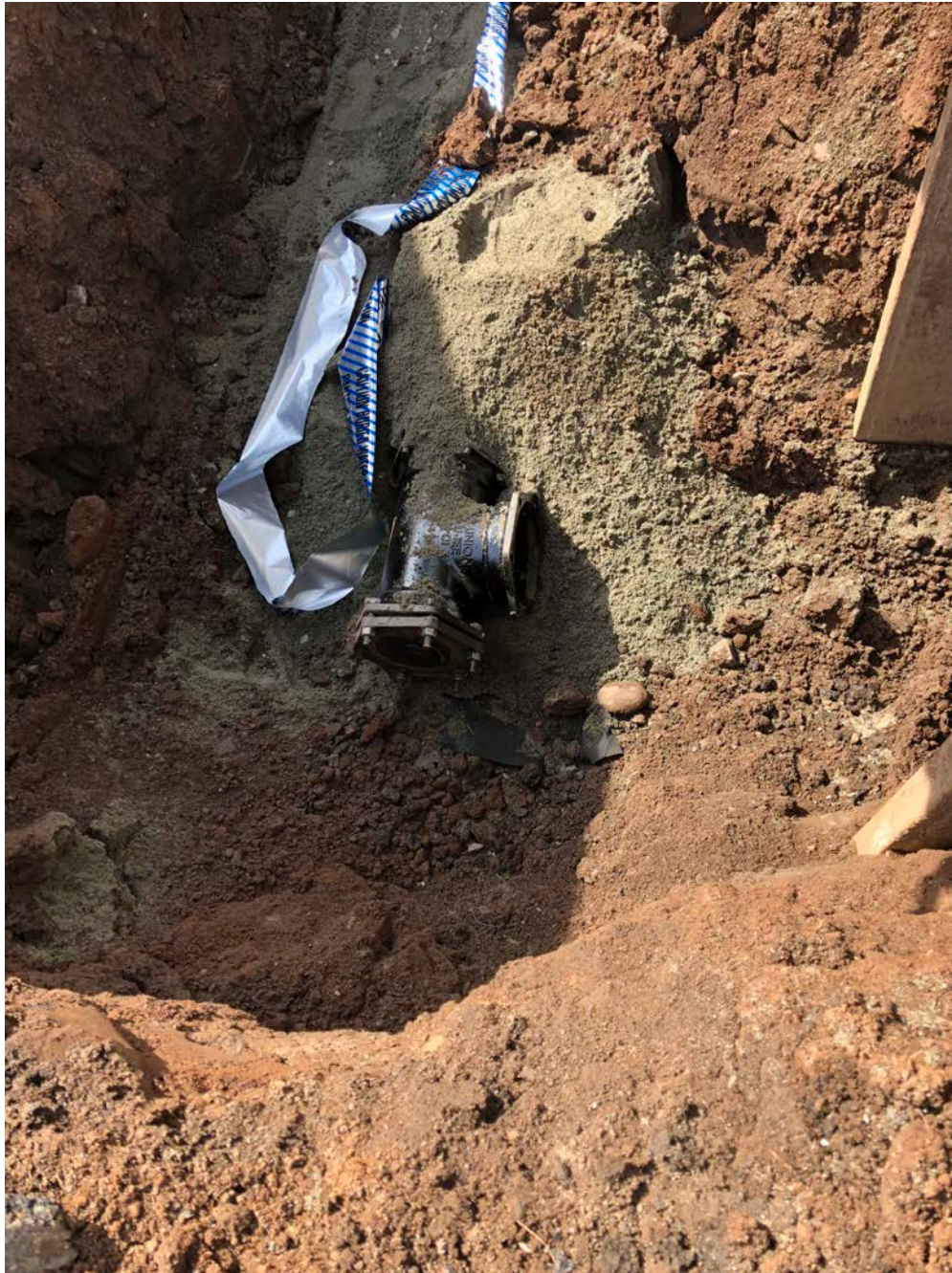
Picture 8: Tee fitting stubbed off with an M.J. cap at 750+59. View to the south.
