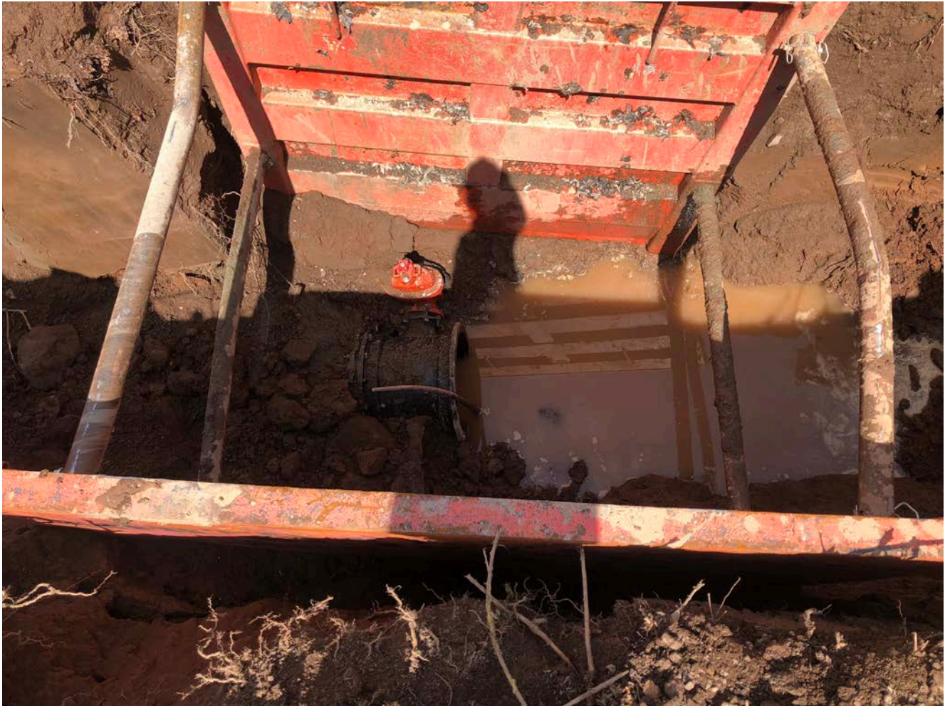
Picture 10: Water observed at bottom of trench today during the installation of 20" DIP.
