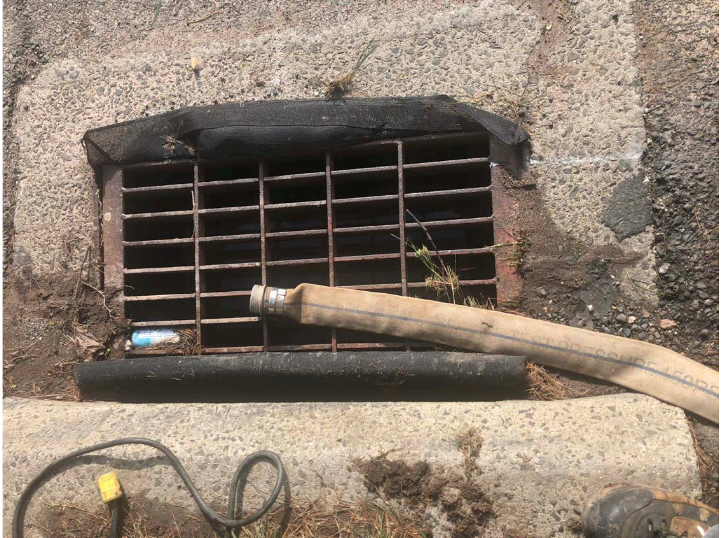
Picture 4: Catch basin with silt sock located south of excavation activities being performed at Station 751+55.
