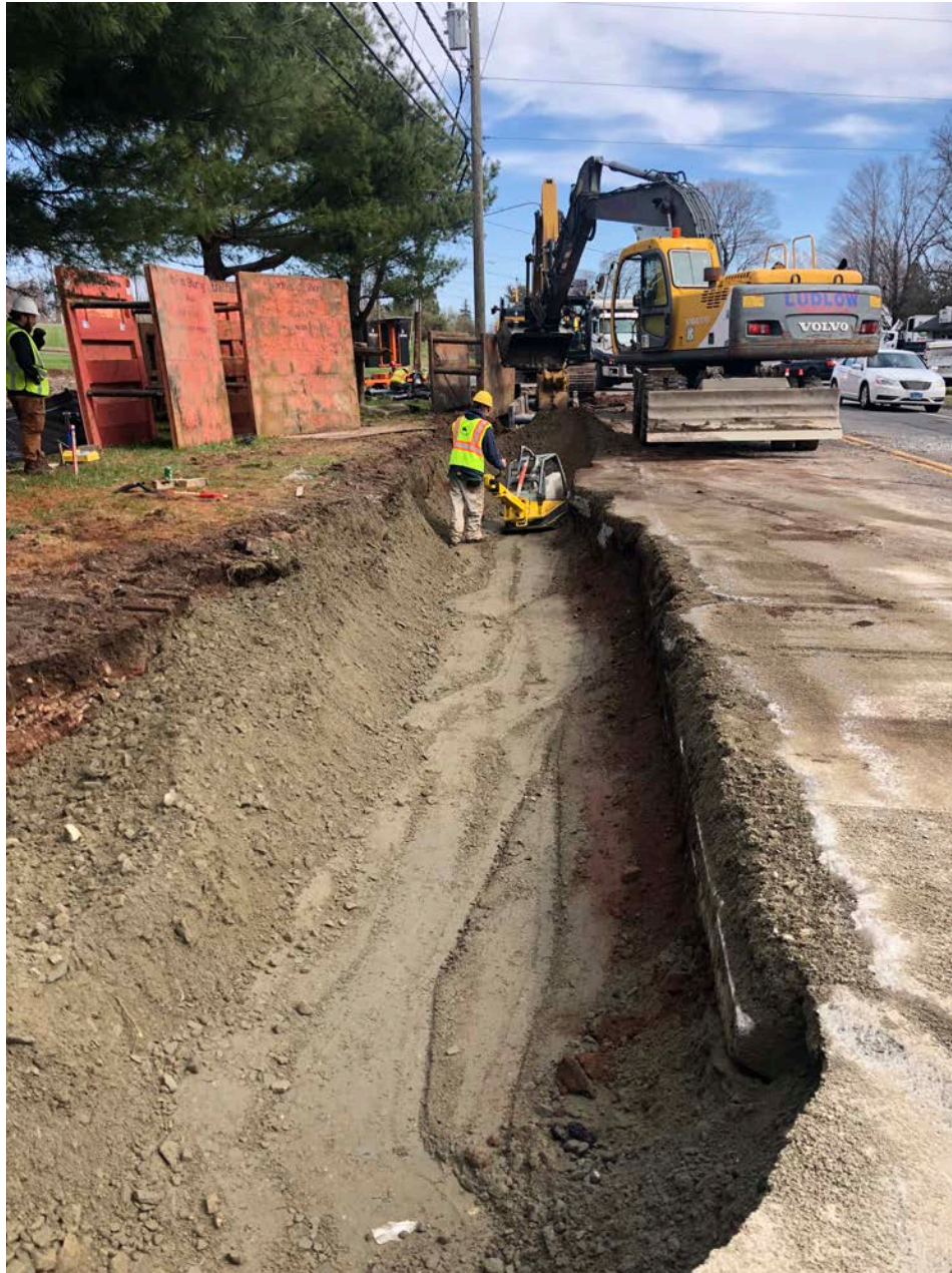
Picture 7: Ludlow compacting fill between Station 751+55 and Station 750+59. View to the north.
