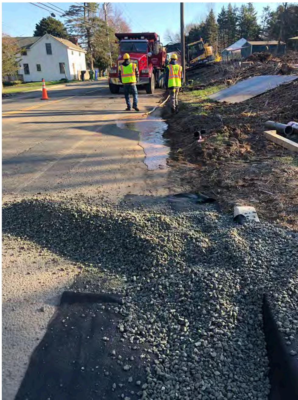
Picture 2: Ludlow pumping water from trench to catch basin covered with filter fabric and \frac{3}{4} " stone. View to the north.
