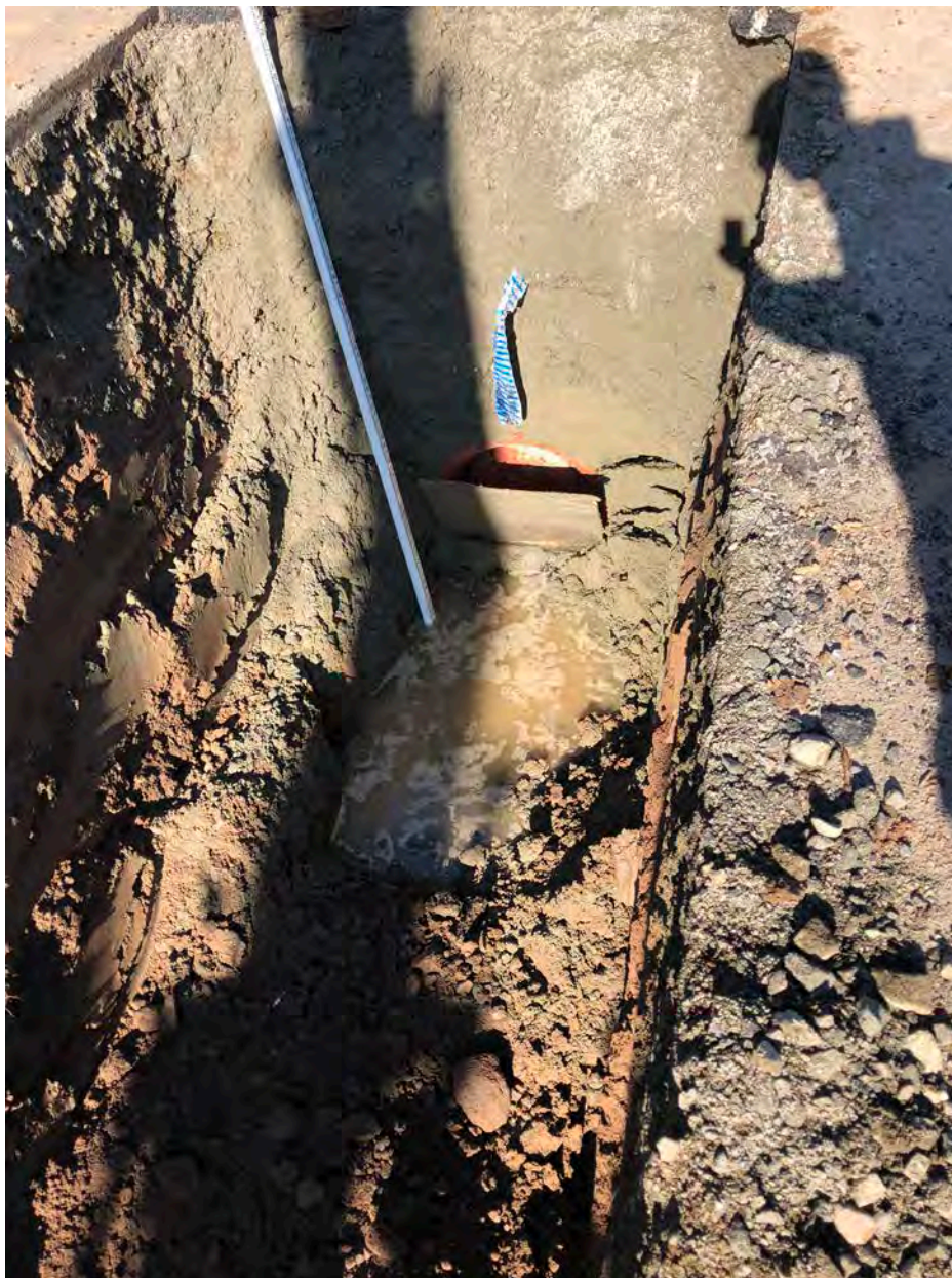
Picture 5: Water visible at 91" below surface grade at Station 124+65.
