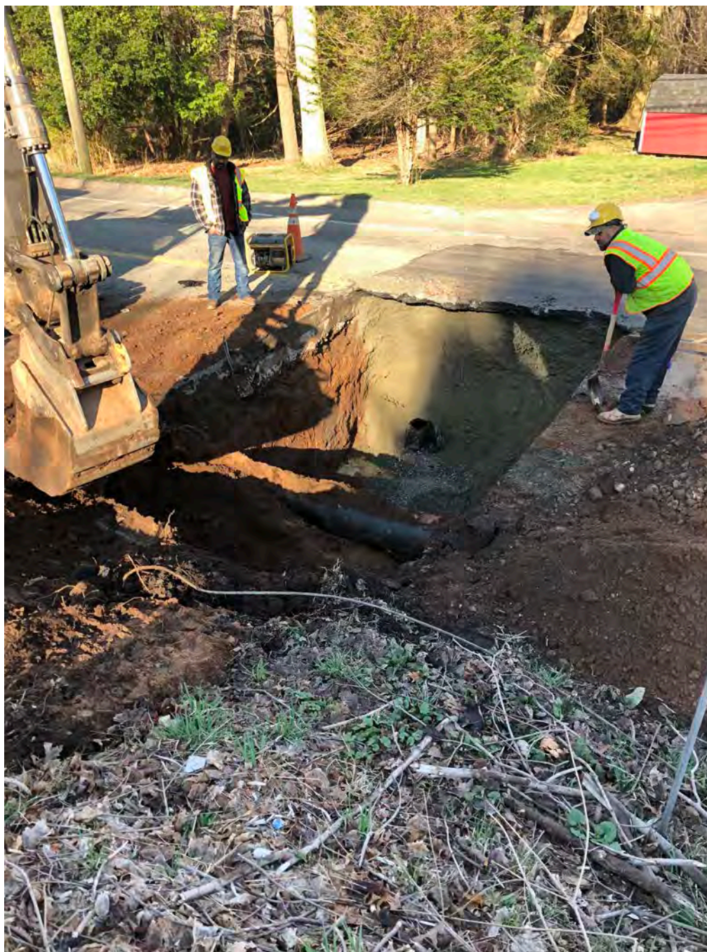
Picture 4: Excavation at Station 124+65, with high pressure gas line and existing 16" T-fitting visible
