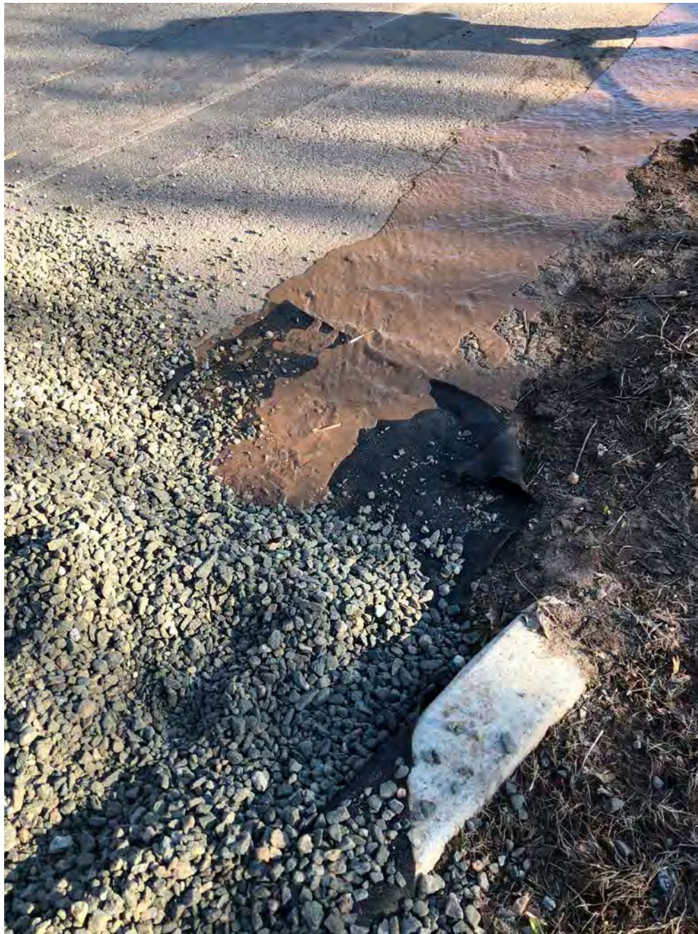
Picture 3: Close-up of catch basin covered with filter fabric and 3/4" stone, receiving water pumped from trench at Station 124+65.
