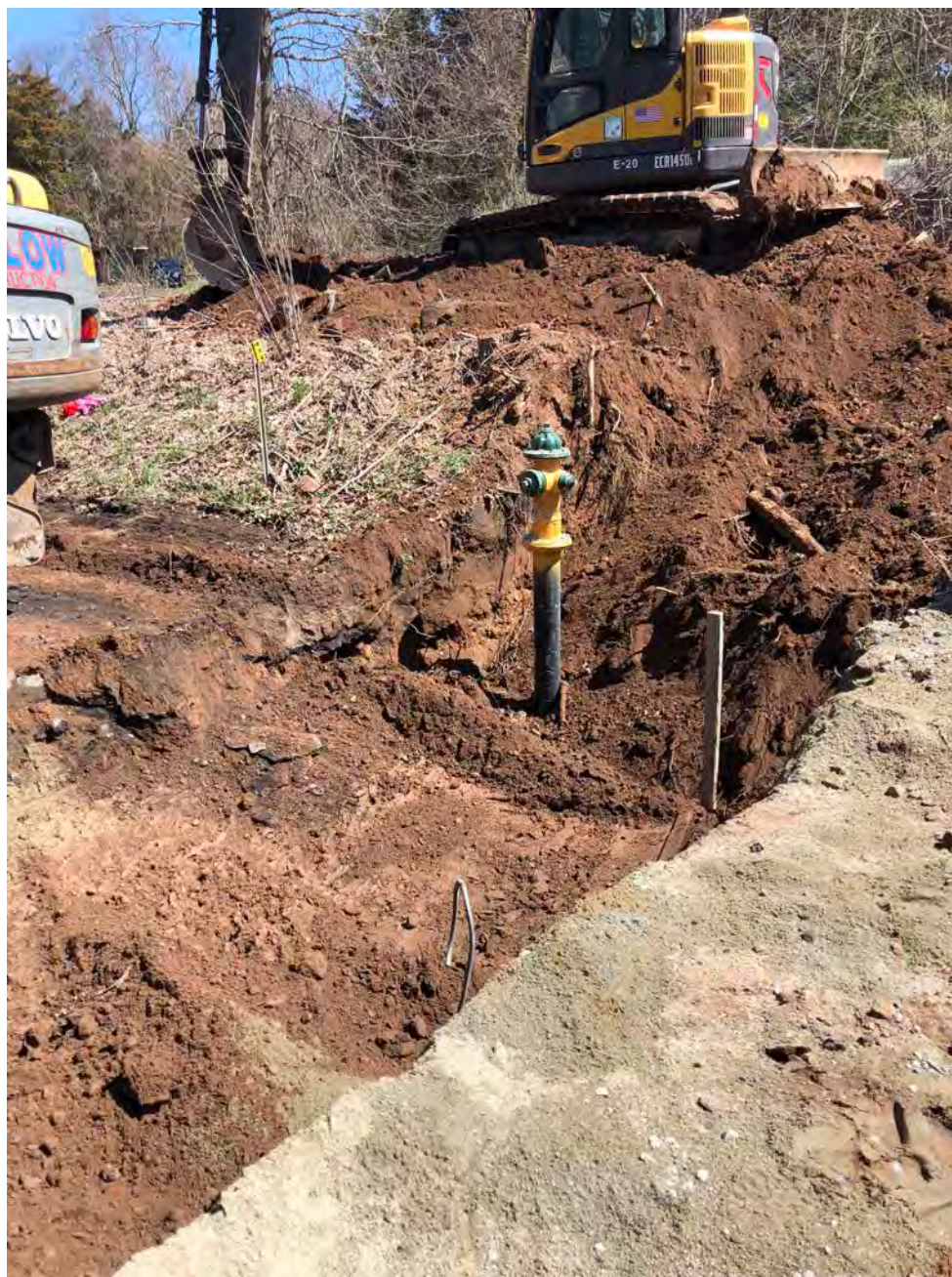
Picture 7: Fire hydrant assembly installed at Station 124+65. View to the east.
