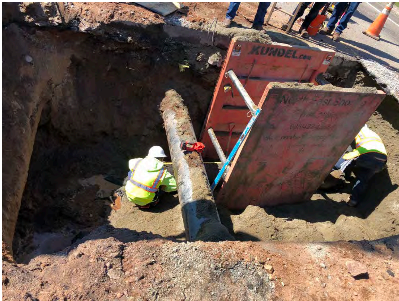
Picture 6: Ludlow installing 12' section of 16" pipe at Station 124+65. High pressure gas line visible in the center of the photo; Storm drain line visible on the very left-hand side of the picture. View to the south.
