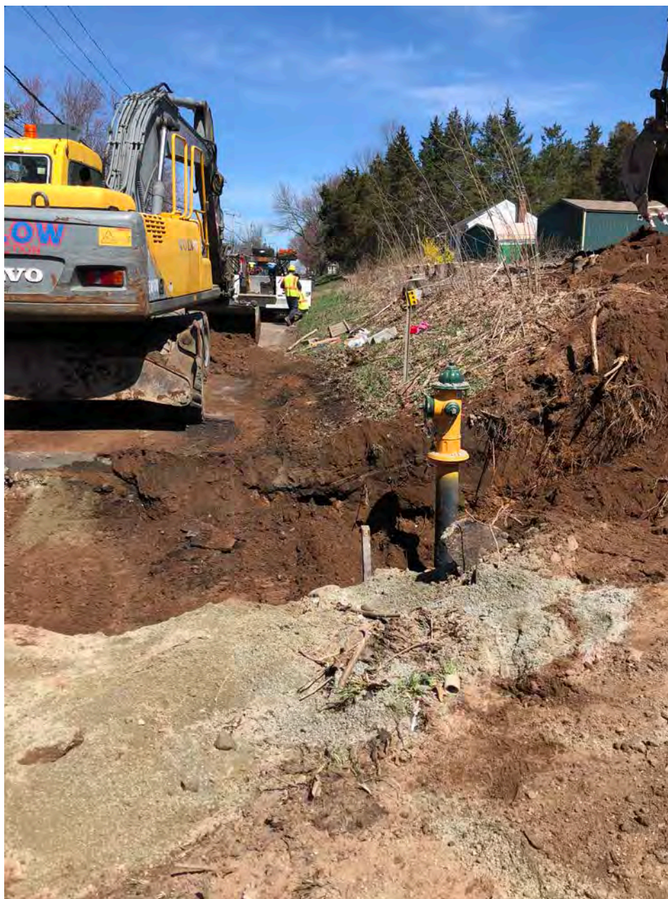
Picture 8: Fire hydrant assembly installed at Station 124+65. View to the north.
