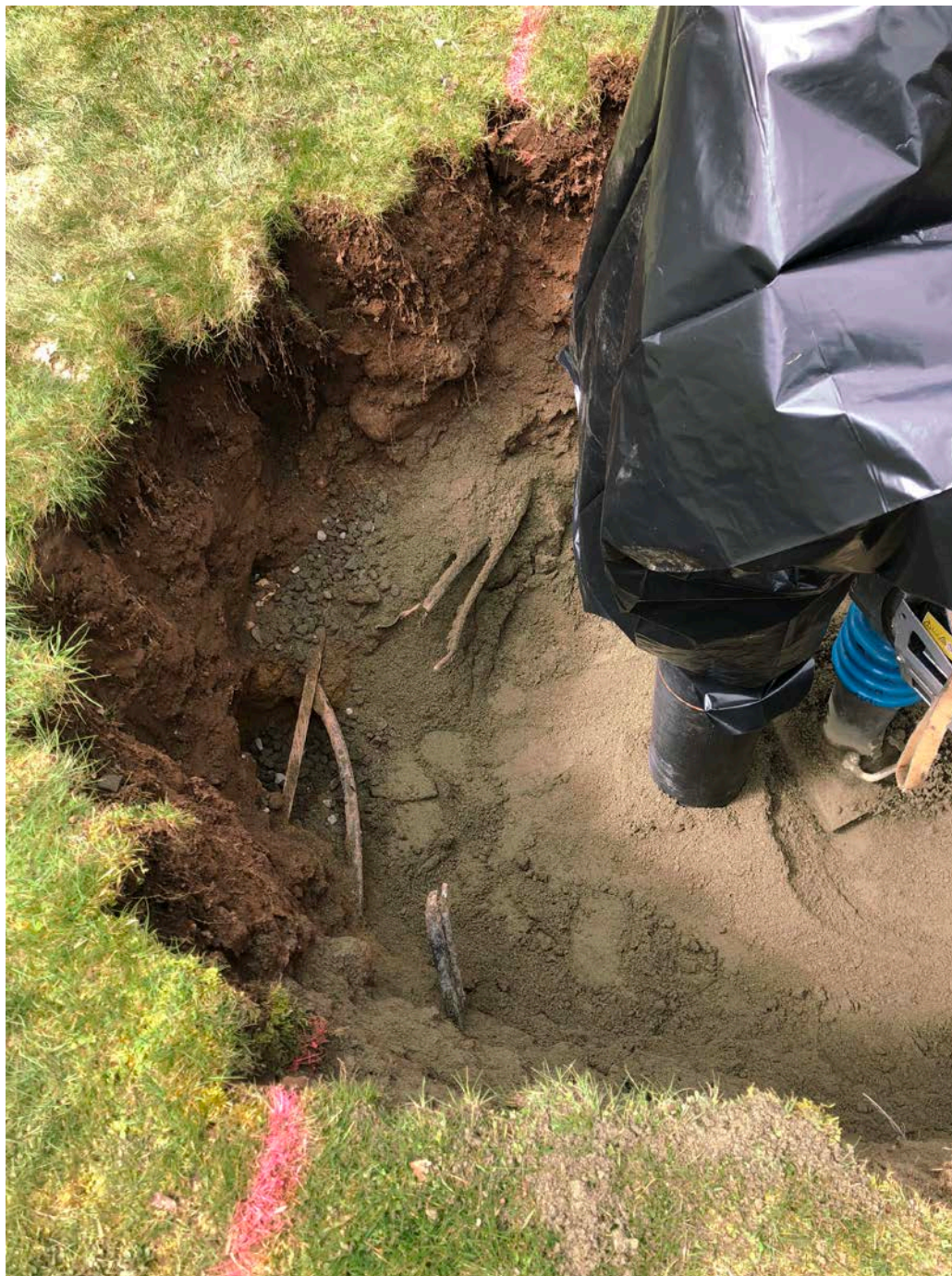
Picture 6: Another view of severed Comcast lines; installed fire hydrant assembly visible on the right-hand side of the photograph. View to the west.
