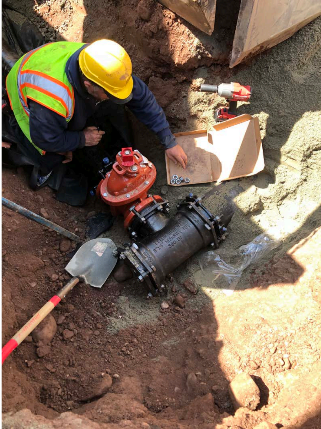
Picture 4: T-fitting and valve assembly placed at the end of 8" DIP to transition to 6" DIP.
