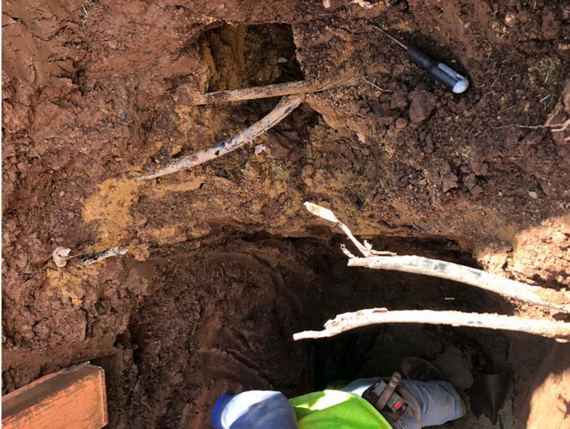
Picture 5: Comcast lines severed by Ludlow. Undamaged powerlines also visible.
