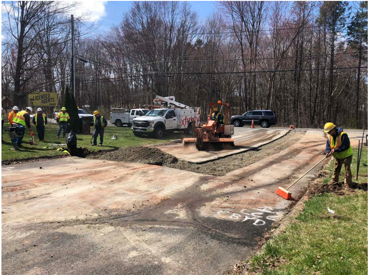
Picture 8: Overview of Royal Oak Drive work area once pipe and hydrant assembly installed; view to the west.
