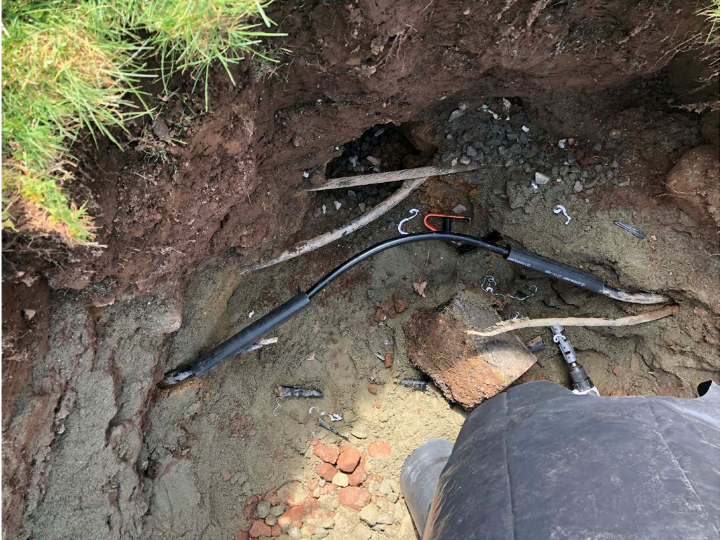
Picture 7: Damaged Comcast lines in the process of repair.
