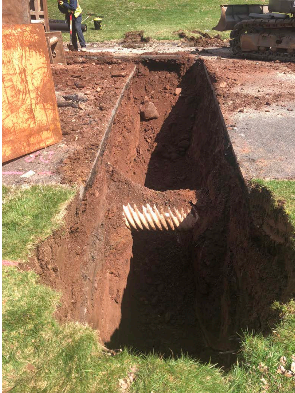
Picture 3: Corrugated storm drain pipe running down (parallel to Royal Oak Drive). View to the north.
