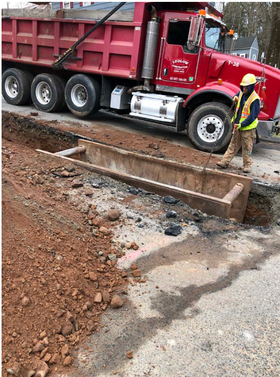
Picture 3: Trench box being deployed at Oak Terrace.
