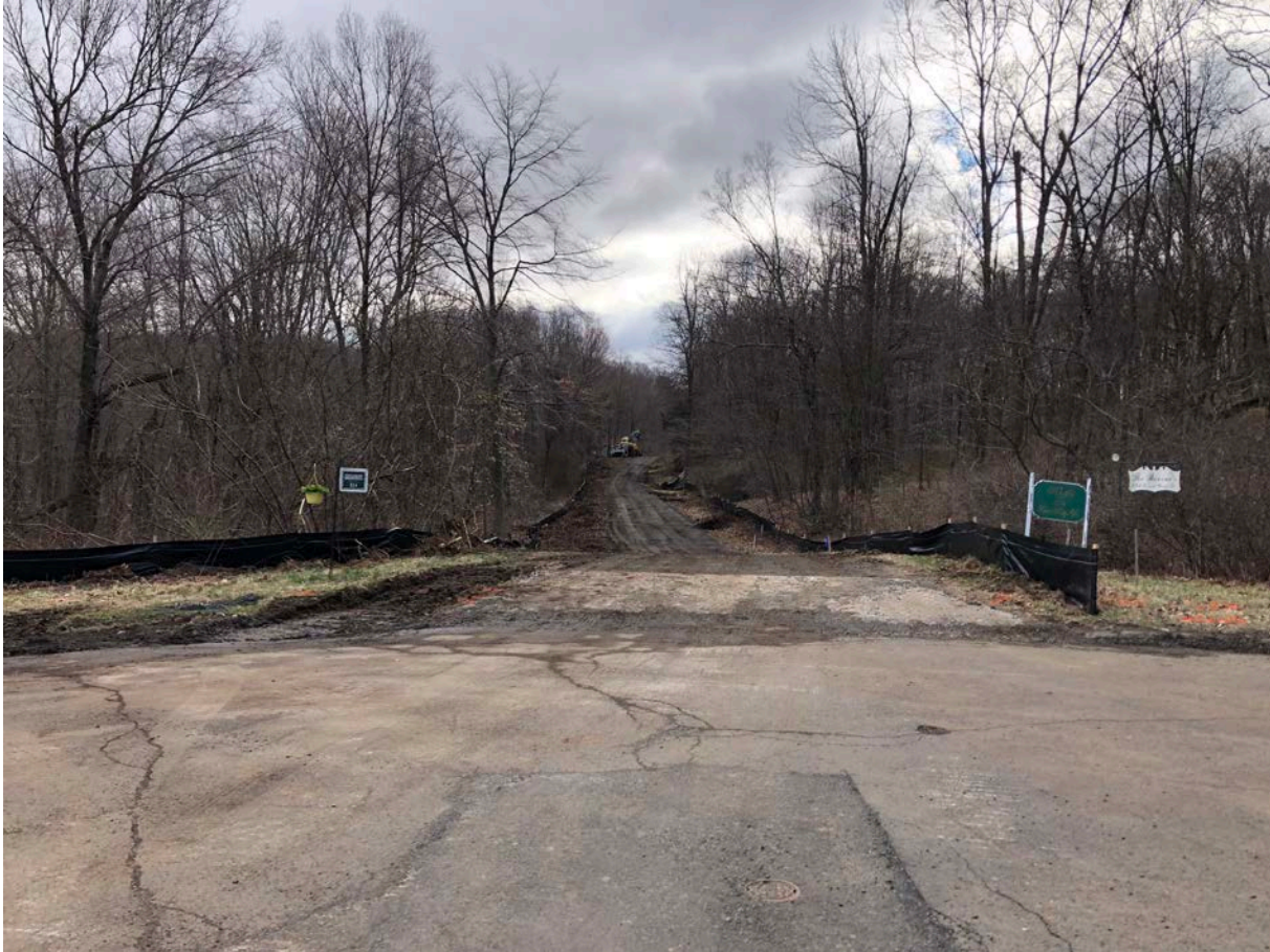
Picture 6: View of access road to future water tank from the Talcott Ridge cul-de-sac depicting erosion control View to the southeast.
