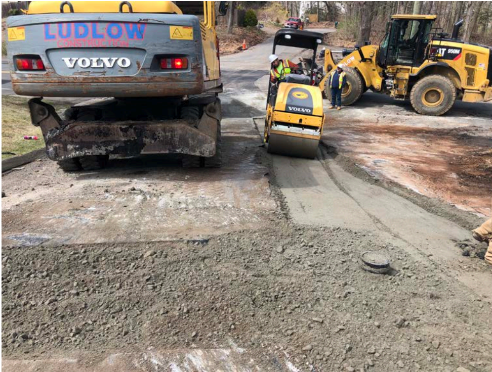
Picture 15: Compacting fill at Oak Terrace. View to the west.
