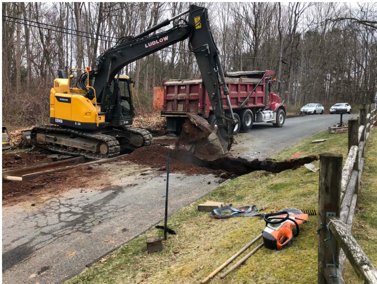
Picture 5: Ludlow excavating trench for 6" DIP.
