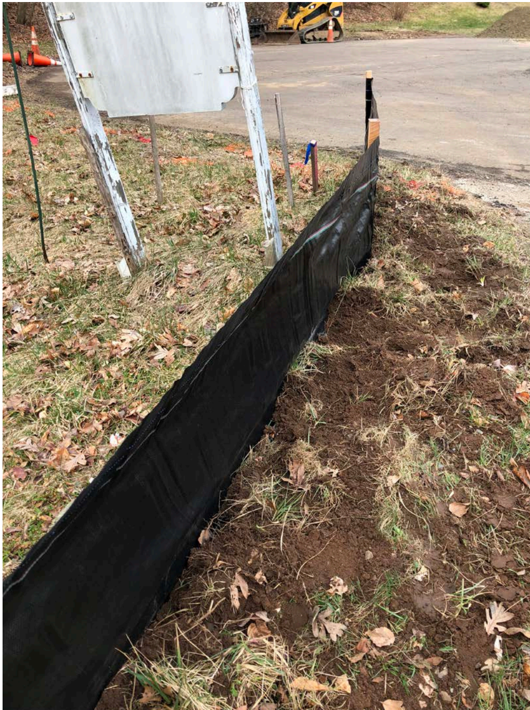
Picture 7: Close-up of erosion control fencing seated into the ground.
