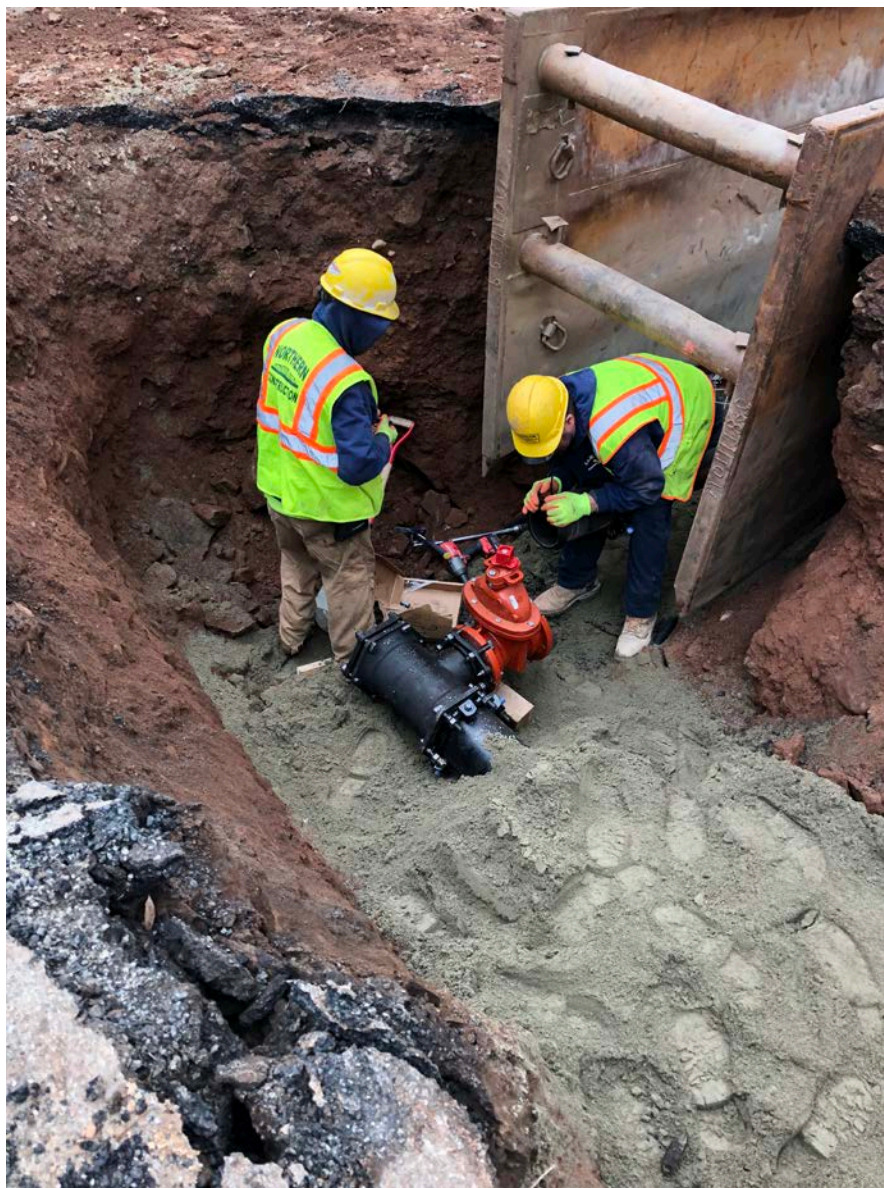
Picture 11: Installation of T-fitting and valve assembly on Oak Terrace.
