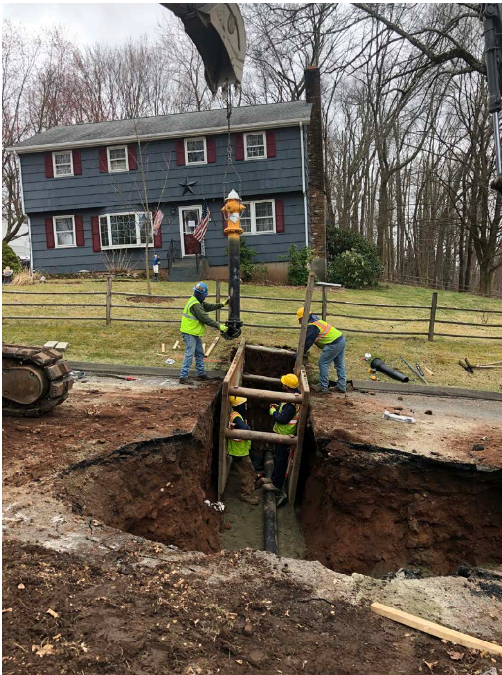
Picture 12: Installation of hydrant assembly on Oak Terrace. View to the south.
