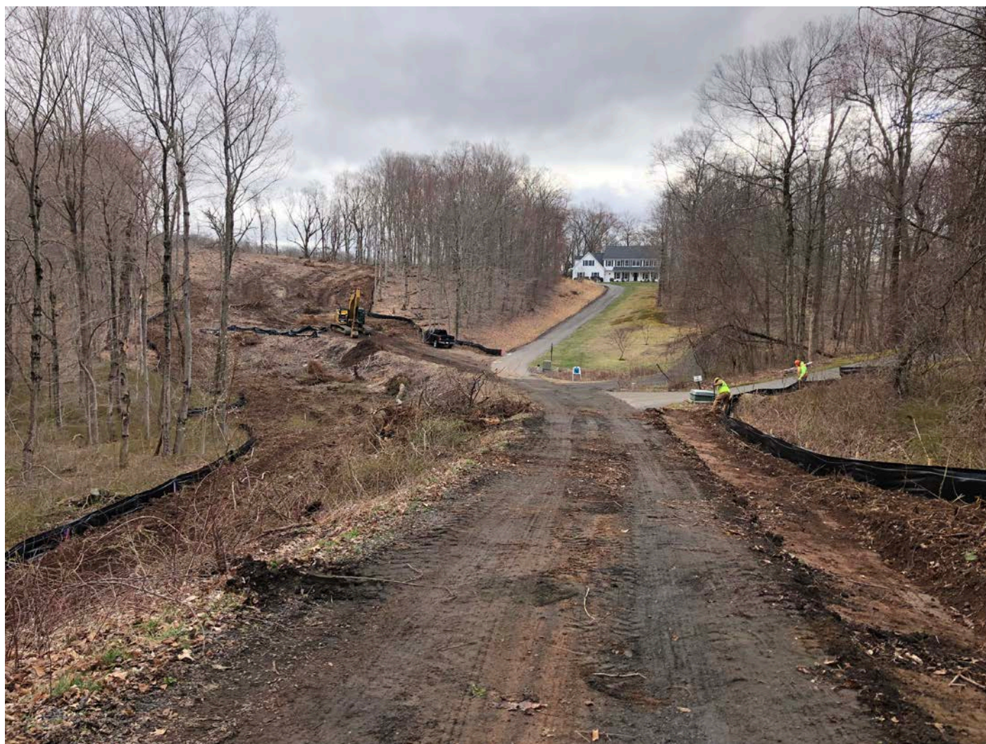
Picture 8: Access road to tank pad with erosion control in place. View to the southeast.
