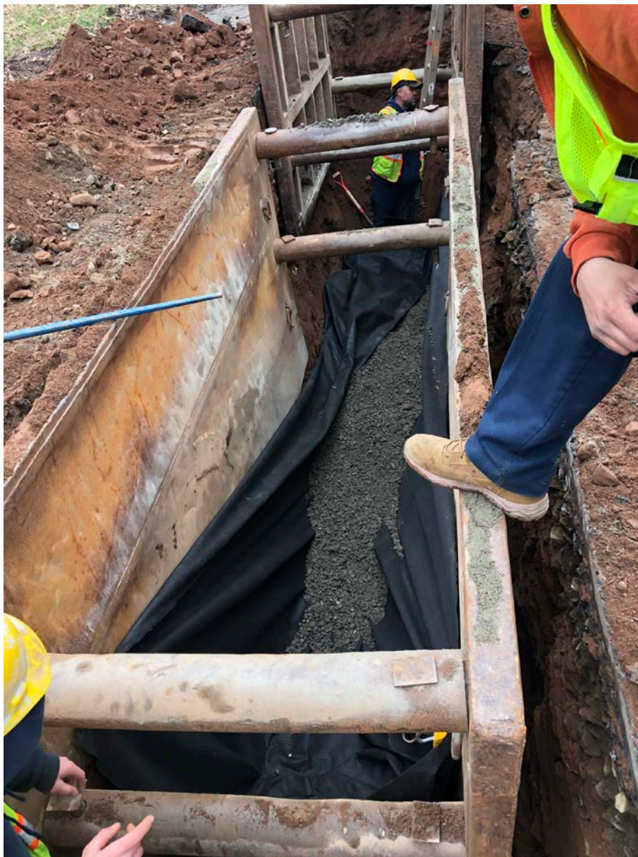
Picture 4: Ludlow preparing bedding for 8" DIP to be placed upon.
