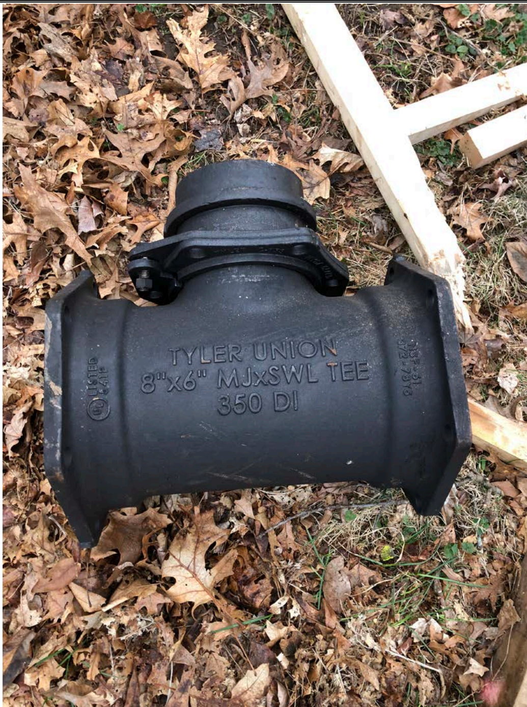
Picture 1: T-fitting used to connect 8" and 6" DIP on Oak Terrace.
