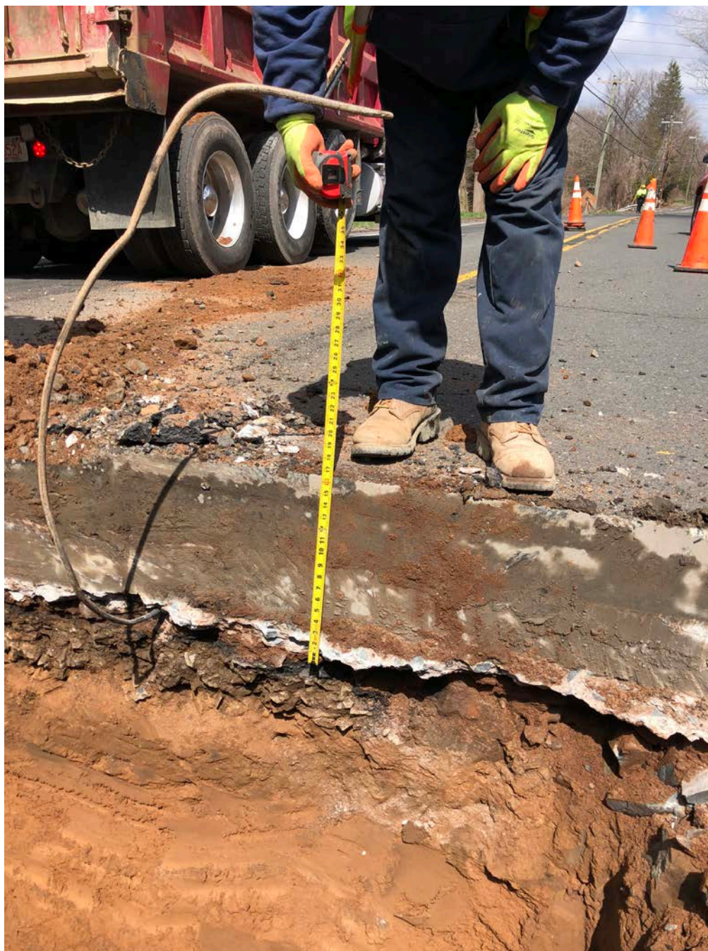
Picture 17: Thickness of asphalt and concrete on Main Street just north of Station 137+00.
