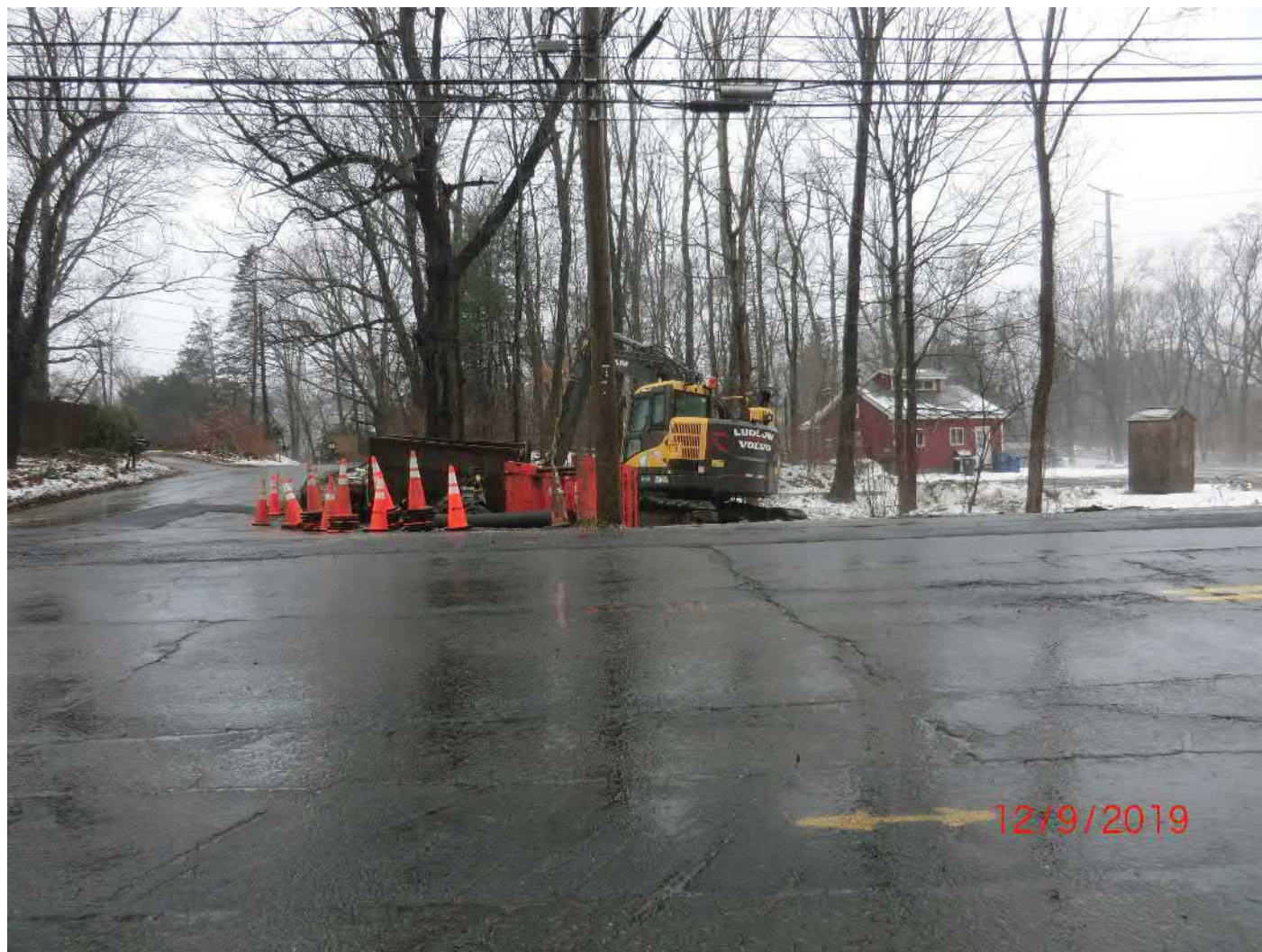
Figure 13 – Facing west at intersection of Main Street and Little Street. Mid-size excavator, trench boxes, cones, and materials. This was the last hydrant location installed.
