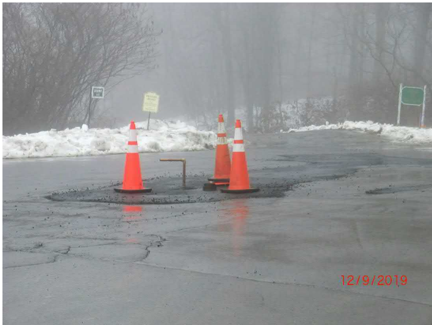
Figure 1 –Looking southeast towards private drive off Talcott Ridge cul-de-sac. Manual 1-inch air vent in open position for filling line.
