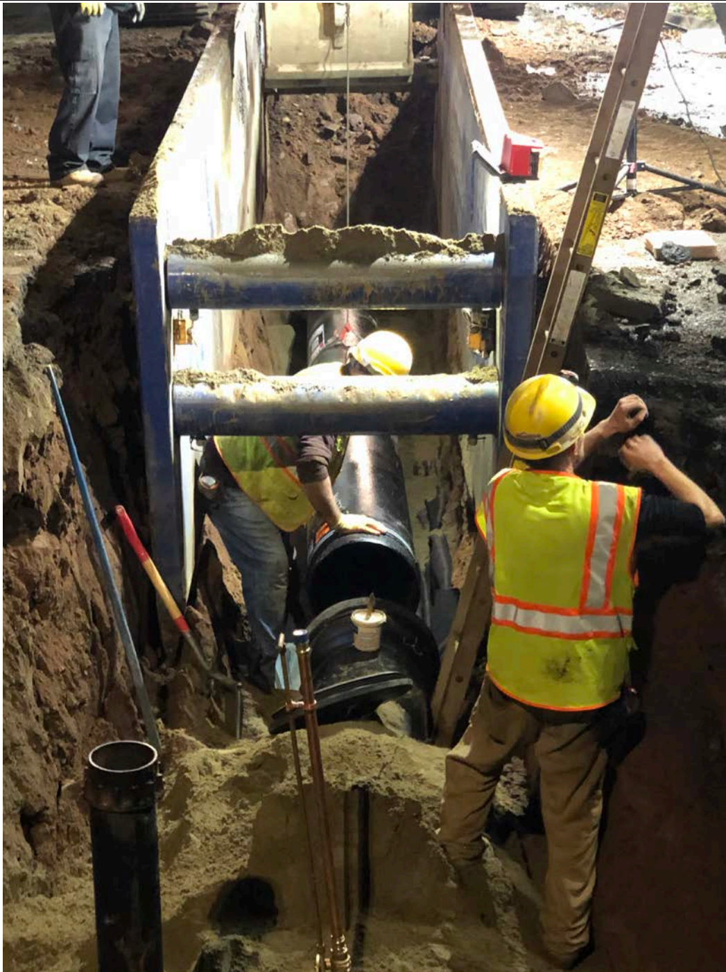
Figure 4 – Placing 2 nd pipe section (Note manual air release in foreground)
