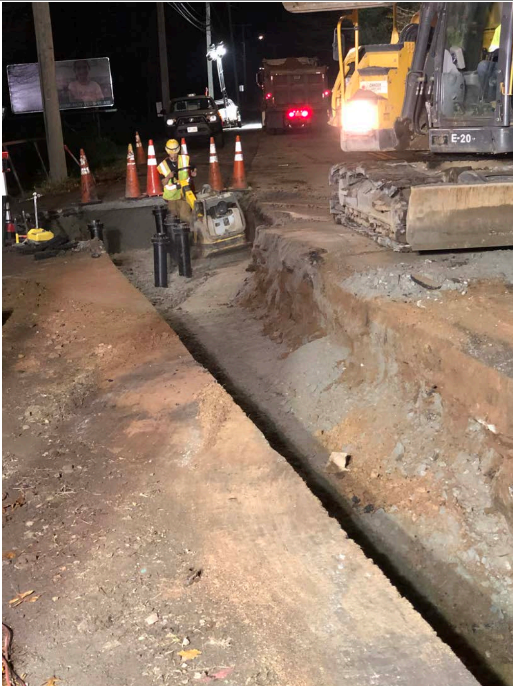
Figure 5 – Compacting 1 st backfill lift
