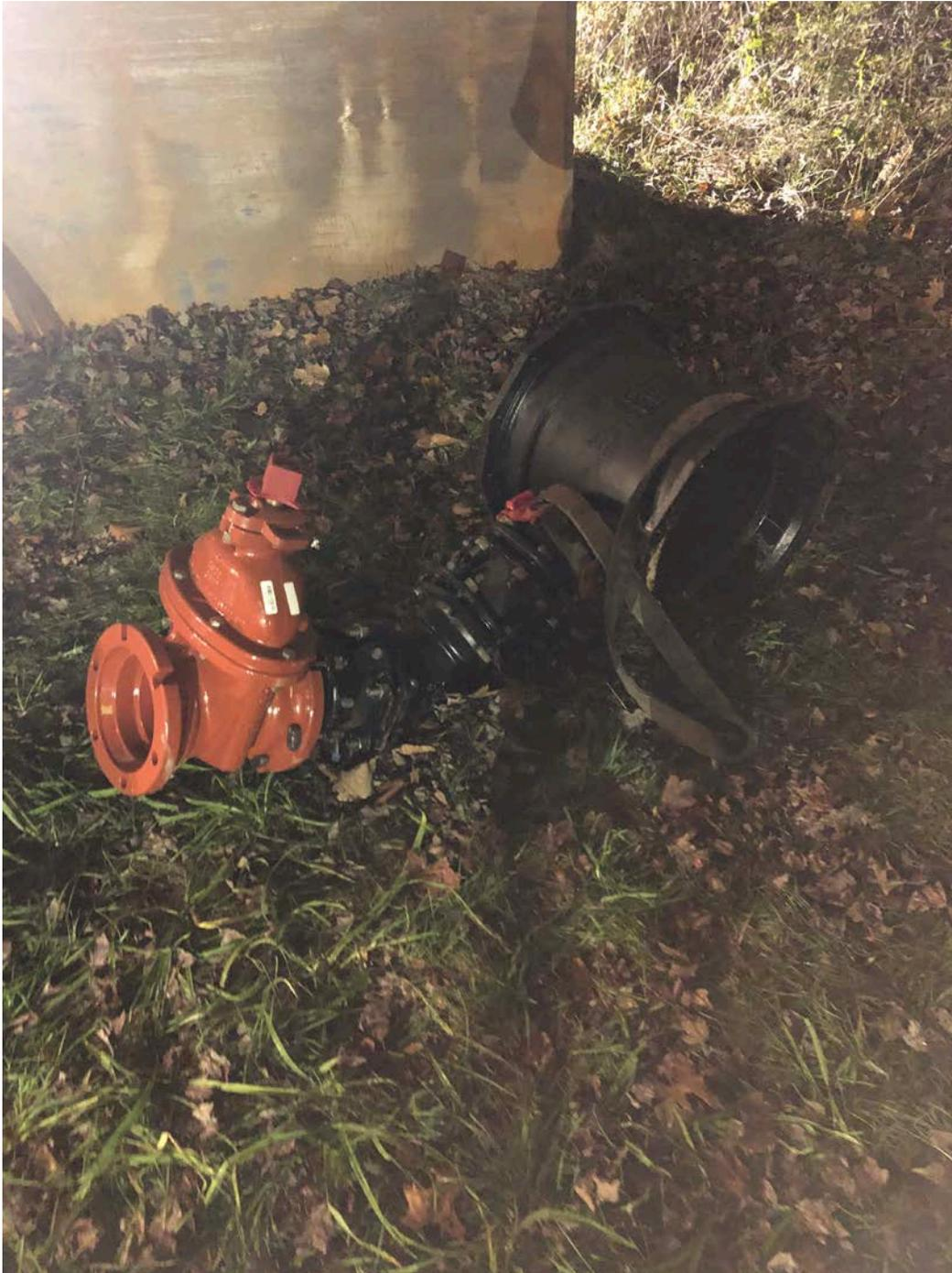
Figure 2 –Blow-off and Drain Tee section above ground
