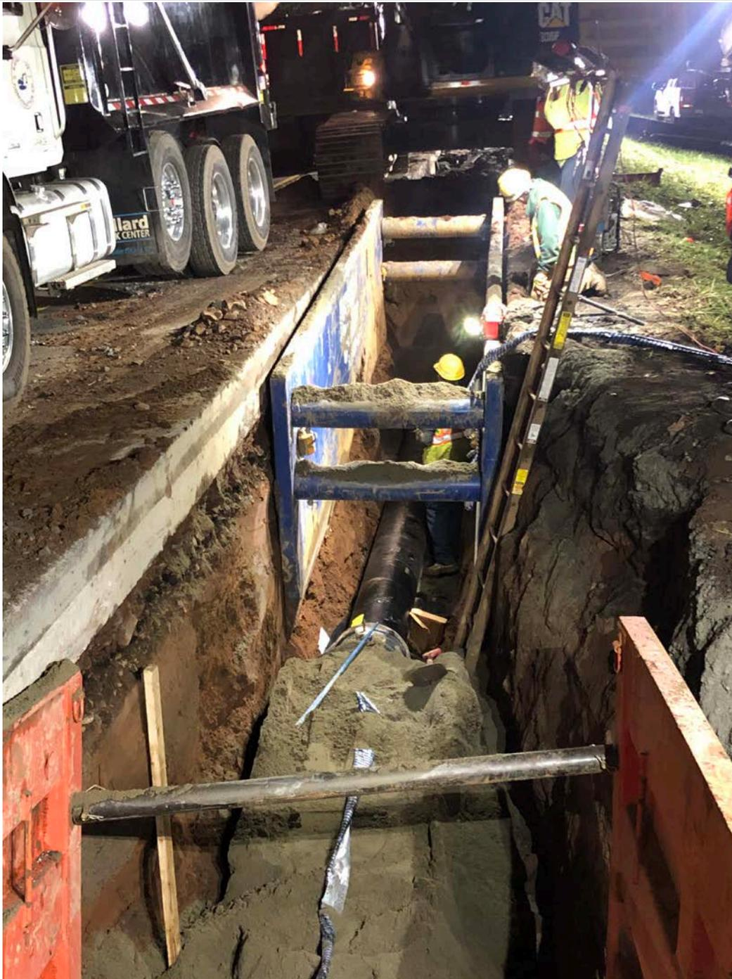
Figure 5 – 2<sup>nd</sup> pipe section attached, preparing to place, compact pipe bedding and lay warning tape
