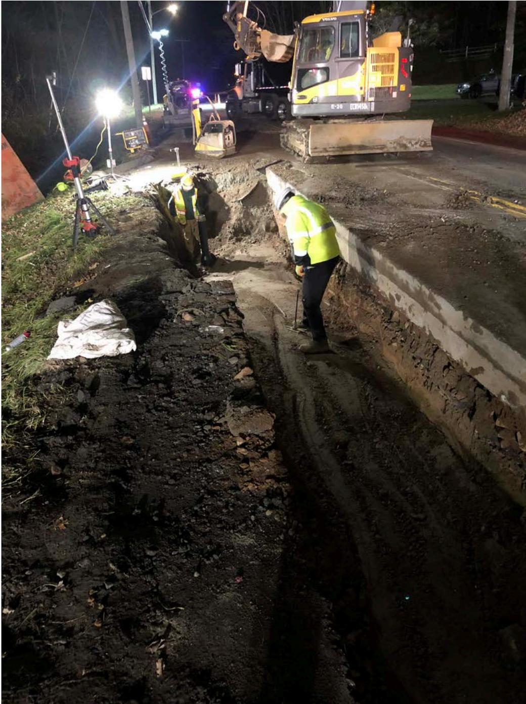
Figure 4 – Compaction testing 1<sup>st</sup> backfill lift above Tee section
