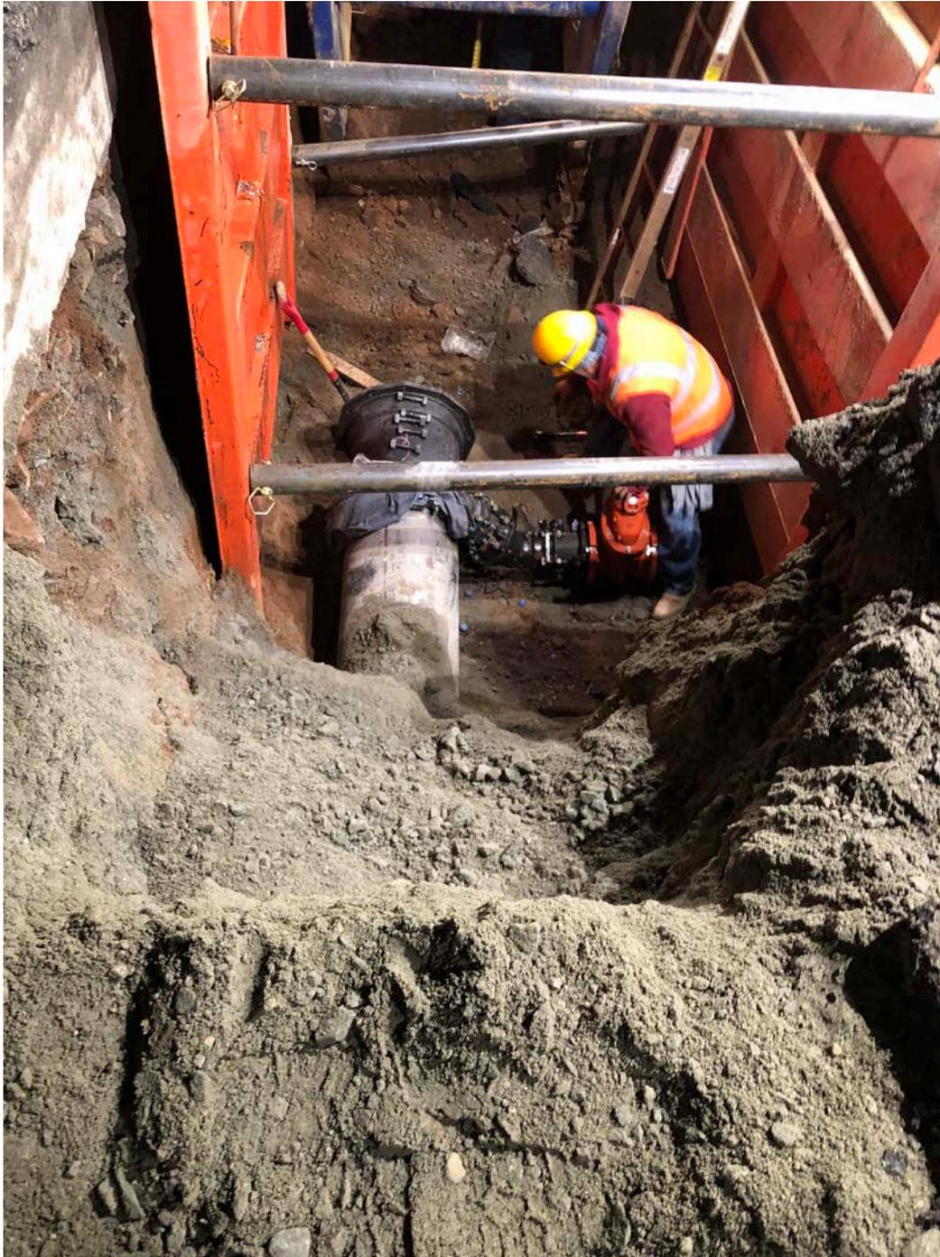
Figure 3 – Placing Tee section for blow-off and drain manhole at Sta. 137+73
