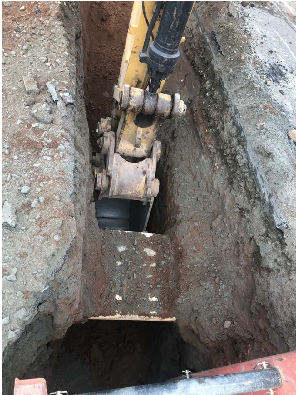
Figure 1 –Ludlow excavates soil from beneath six 4” gray PVC conduits.
