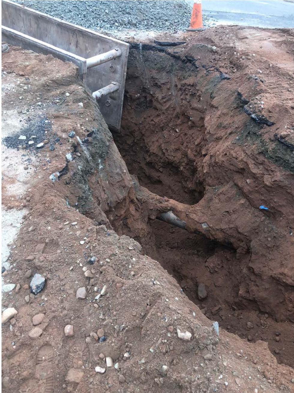
Figure 5 – Existing 8” DIP water main exposed during trenching activities.
