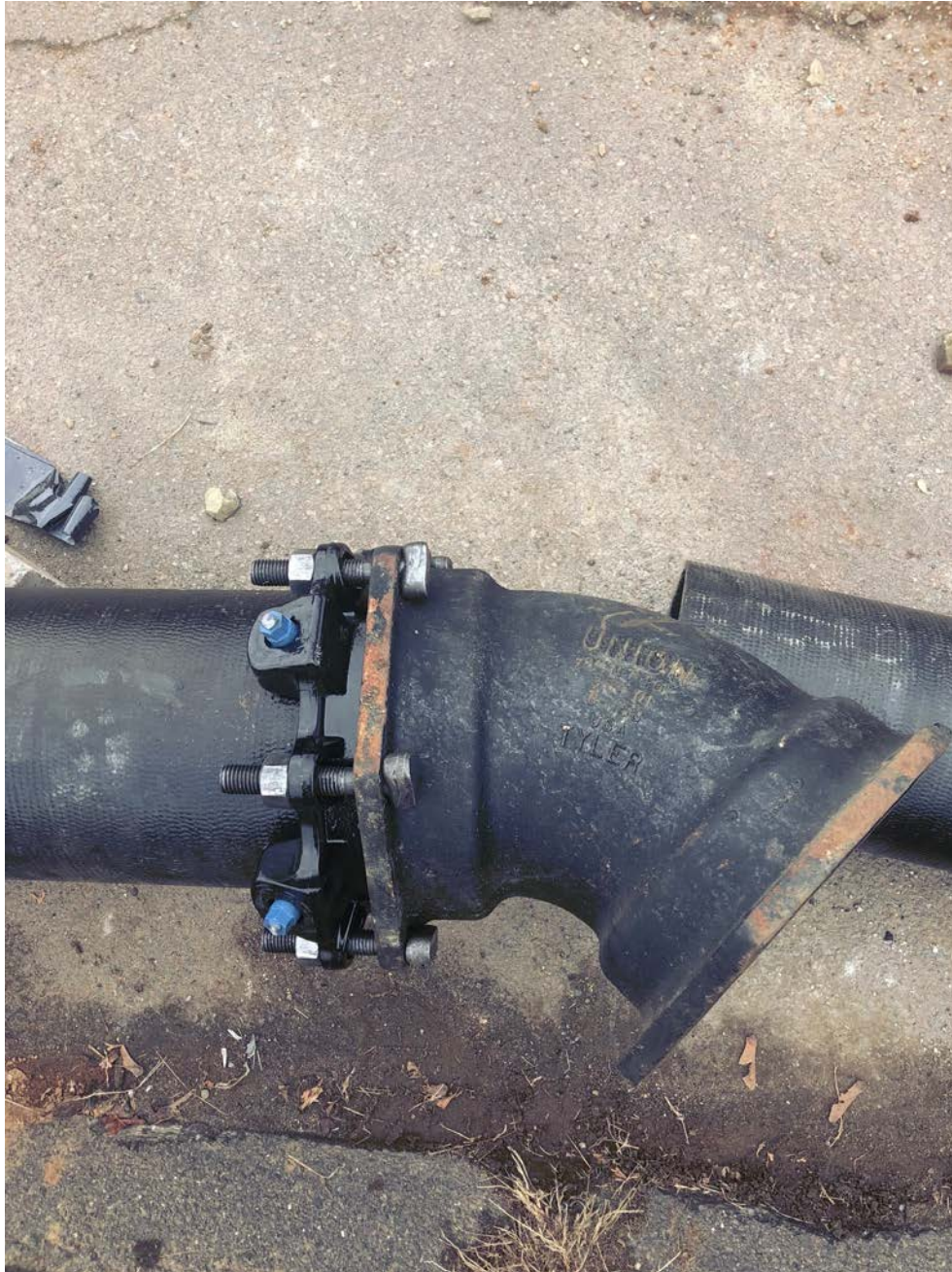
Figure 4 – One of the two 45° bend sections placed today.
