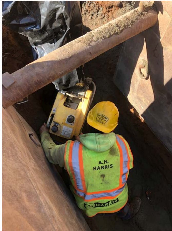
Figure 8 – Ludlow compacting sand around hydrant assembly on west side of trench.
