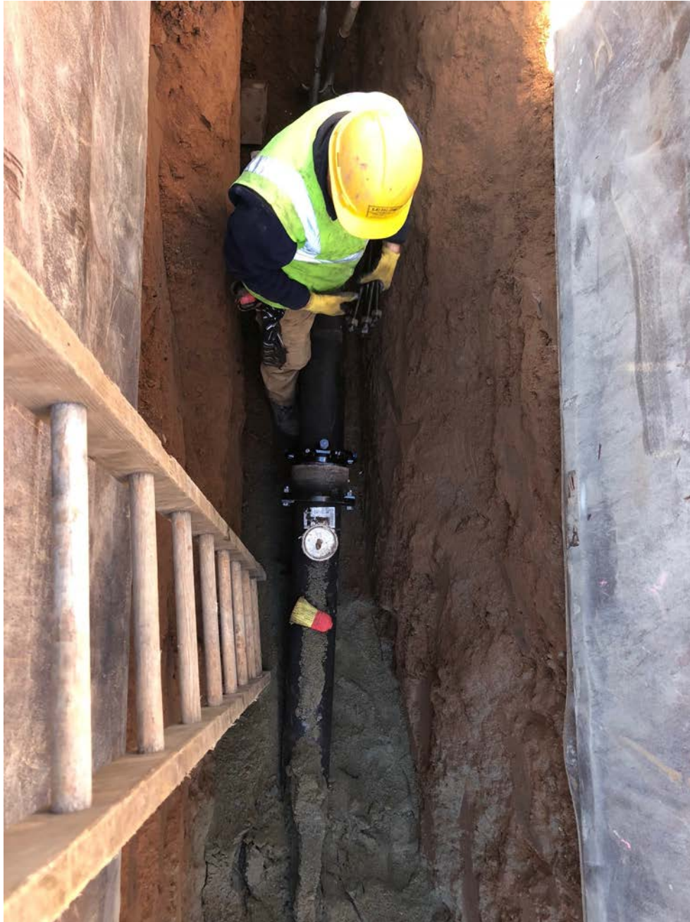
Figure 5 – Ludlow in the process of securing pieces of 6” DIP to each other using a bell clamp/megalug connection.
