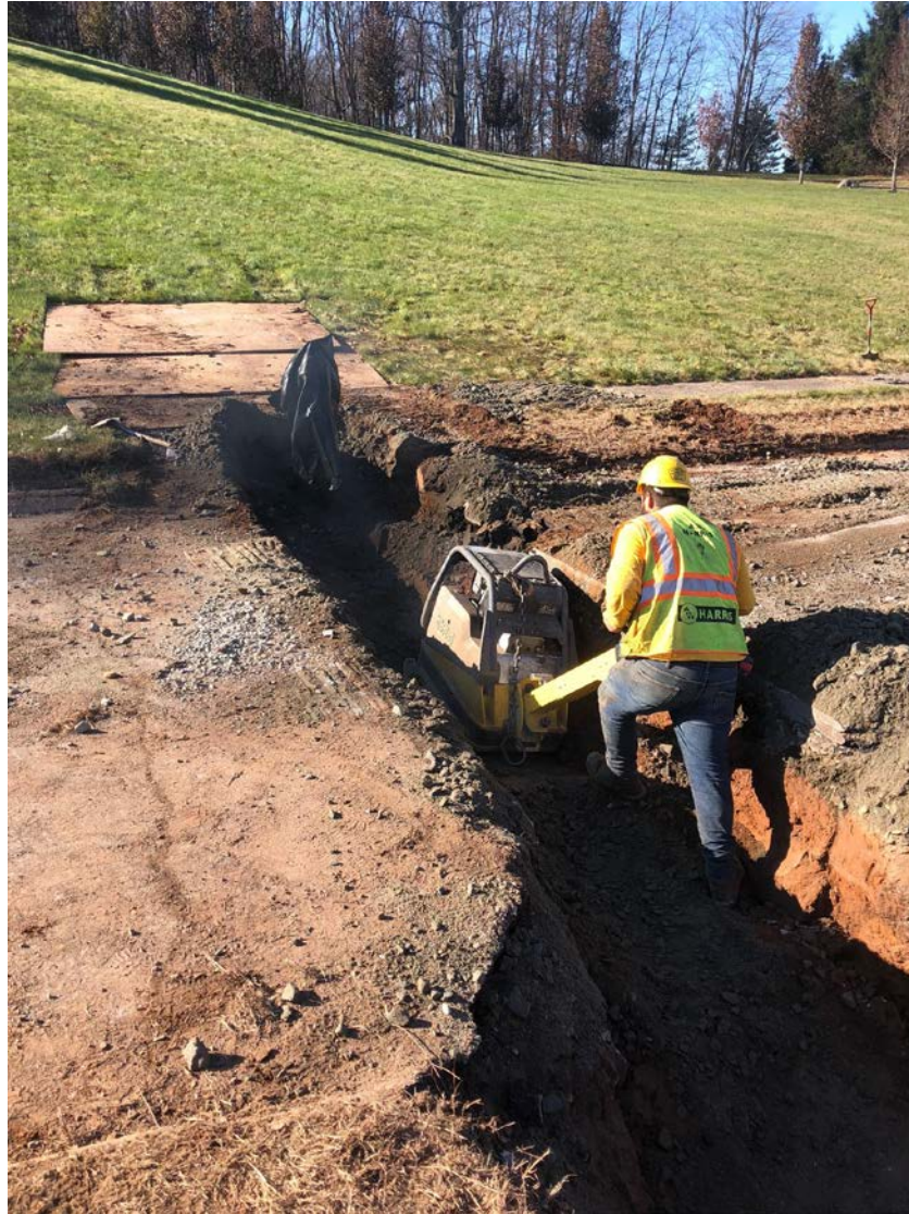
Figure 9 – Ludlow compacting 3” minus gravel backfill.
