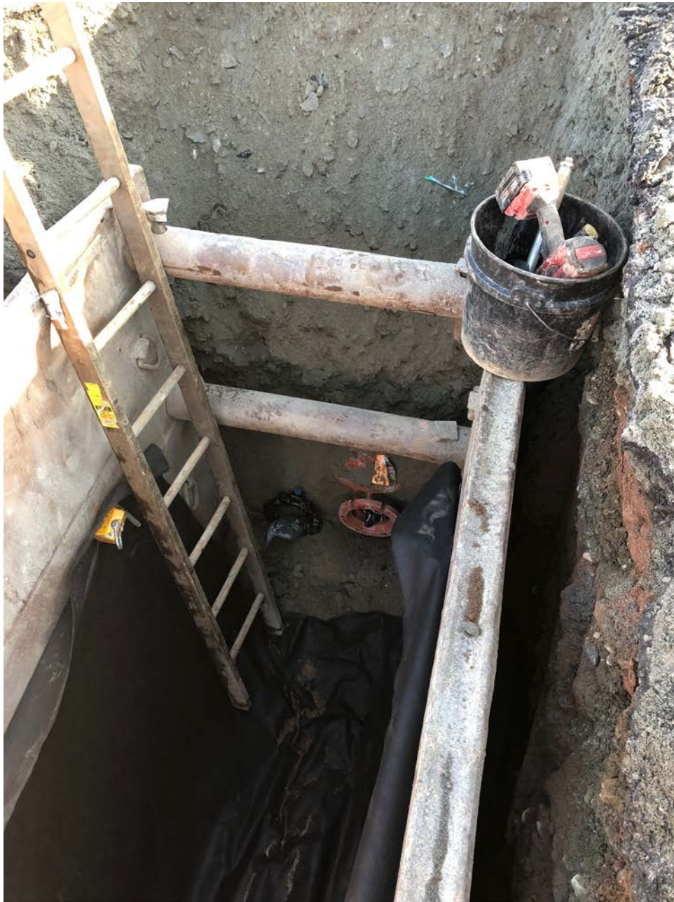
Figure 2 – Valve located on the run of 16” DIP that Ludlow recently placed on the east side of the northbound lane of Talcott Ridge Drive. View to the east.
