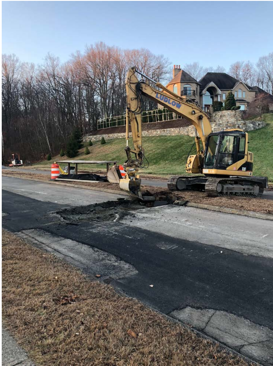
Figure 1 –Ludlow removing asphalt from Station 31+81 that will be trenched for hydrant installation.
