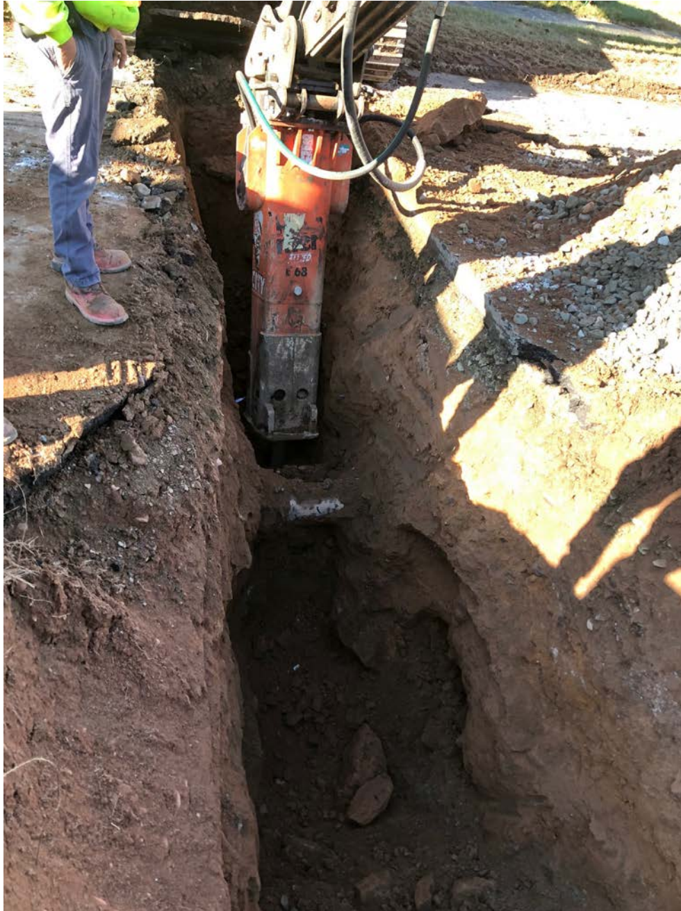
Figure 4 – Ludlow exposes an existing 8” water line that runs beneath the western (southbound) lane of Talcott Ridge Drive. View to the west.
