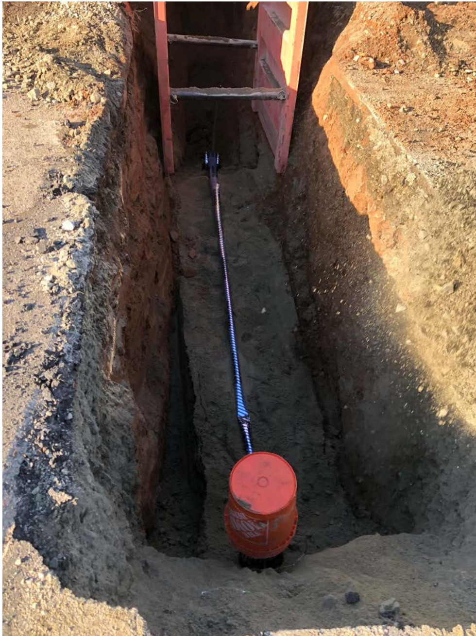
Figure 3 – Sand and caution tape placed over first stick of 6” DIP installed today. Bucket is covering the valve stem and riser that Ludlow placed on the run of 16” DIP that Ludlow recently placed on the east side of the northbound lane of Talcott Ridge Drive. View to the west.
