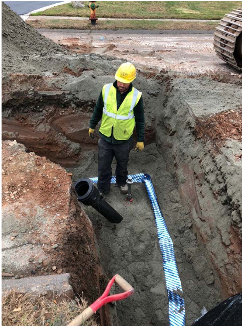
Figure 12– Ludlow installing valve operator extension and gate box onto (now buried) valve.
