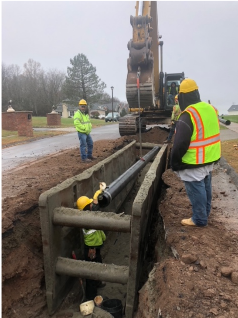
Figure 12– 8” DIP in the process of being placed.
