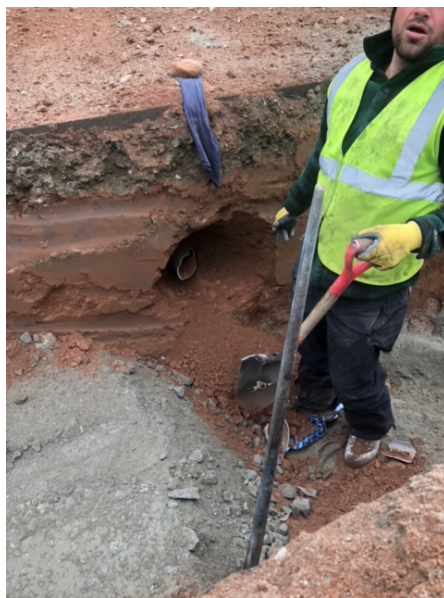
Figure 16– Remnants of 4” gray PVC conduit that Ludlow broke through just east of the eighth (and last) stick of 8” DIP installed for the day.
