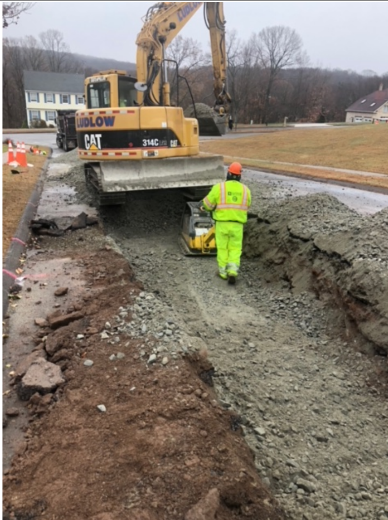
Figure 13– Ludlow compacting 3” minus gravel.
