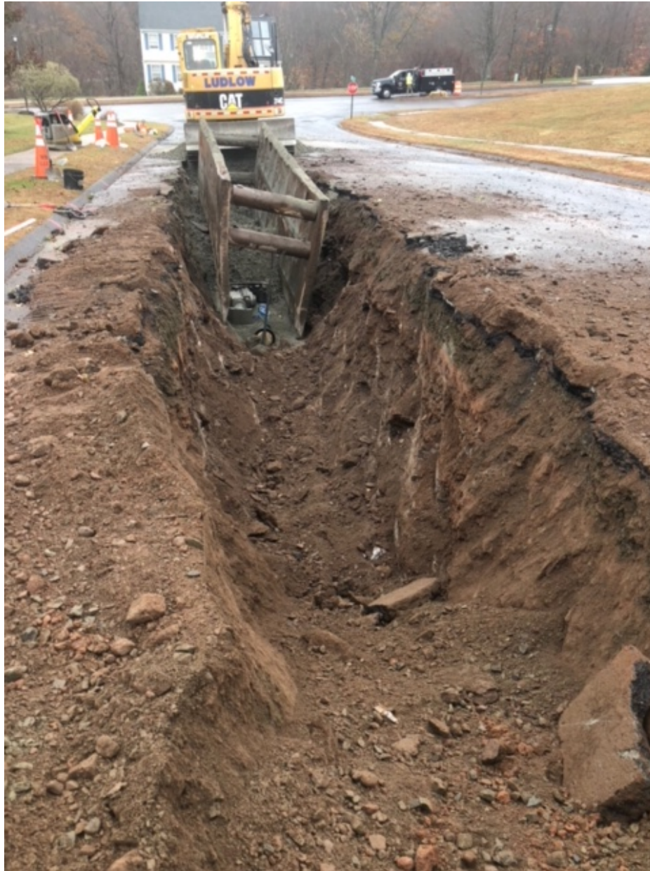
Figure 10– Bedrock visible on both sidewalls of trench. View to the east.
