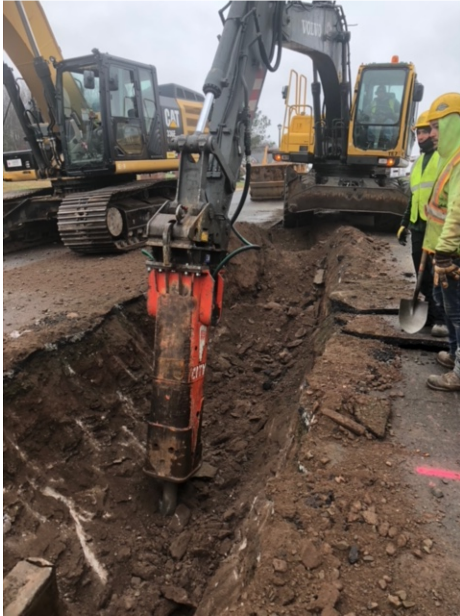
Figure 9– Ludlow hammering bedrock during trenching activities.
