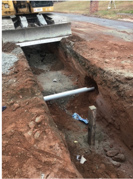
Figure 17– Repaired 4” PVC conduit.
