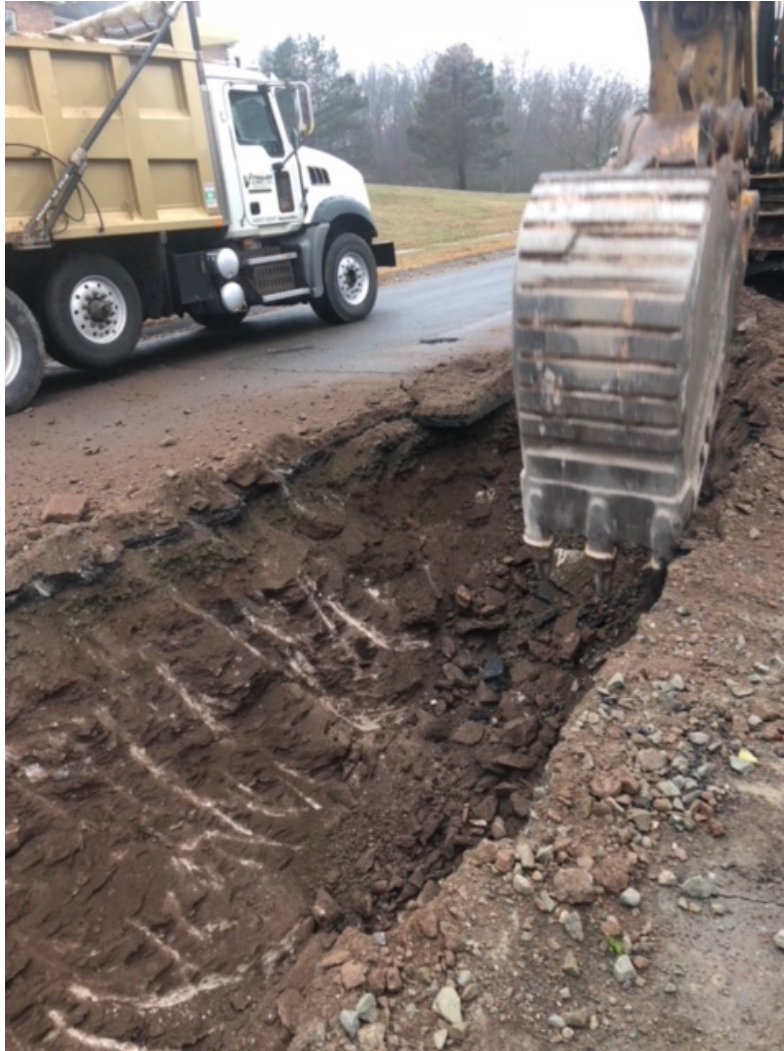
Figure 7 – Ludlow excavating through shallow bedrock prior to placing third stick of 8" DIP.
