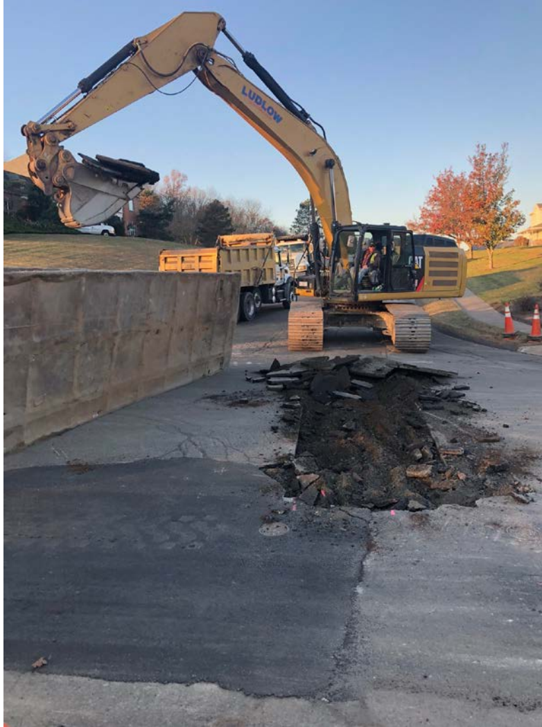
Figure 4 – Ludlow peeling back asphalt from today's work area.
