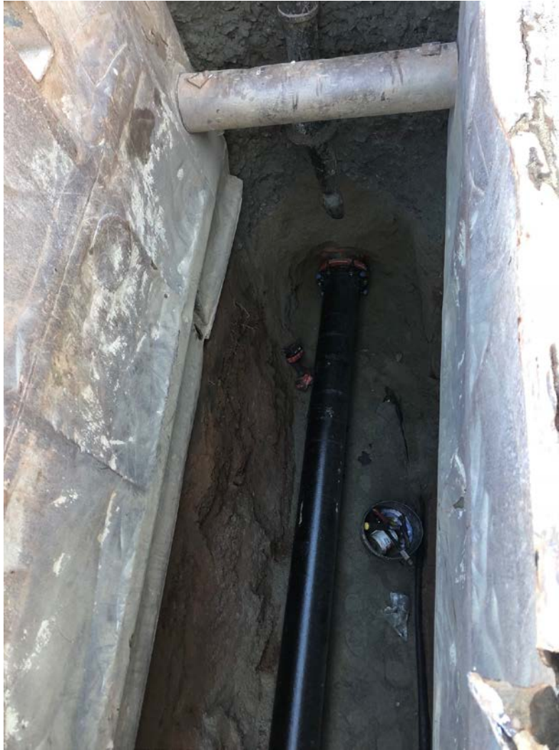
Figure 5 – Station 600+03.5, facing east. The first stick of 8” DIP attached to the new 16” water line located at the toe of the excavation.
