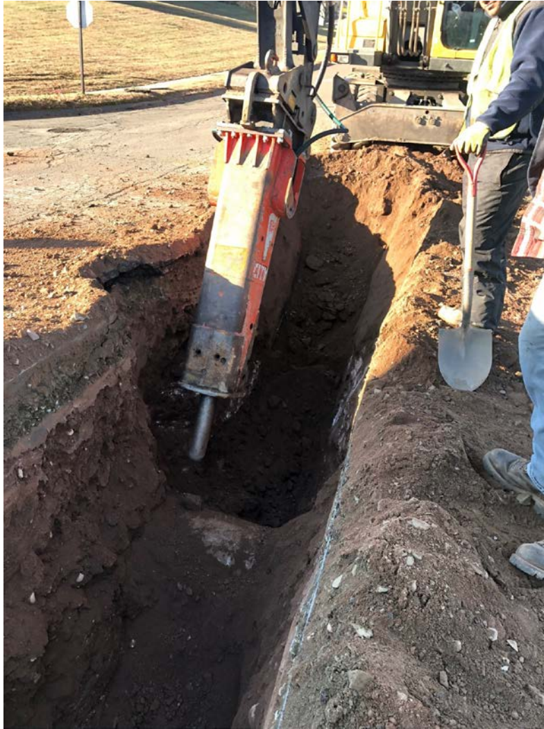
Figure 7 – Ludlow daylights an existing concrete storm drain line (~16: diameter) at ~ Station 600+30 and uses hammer to remove bedrock from beneath the pipe.
