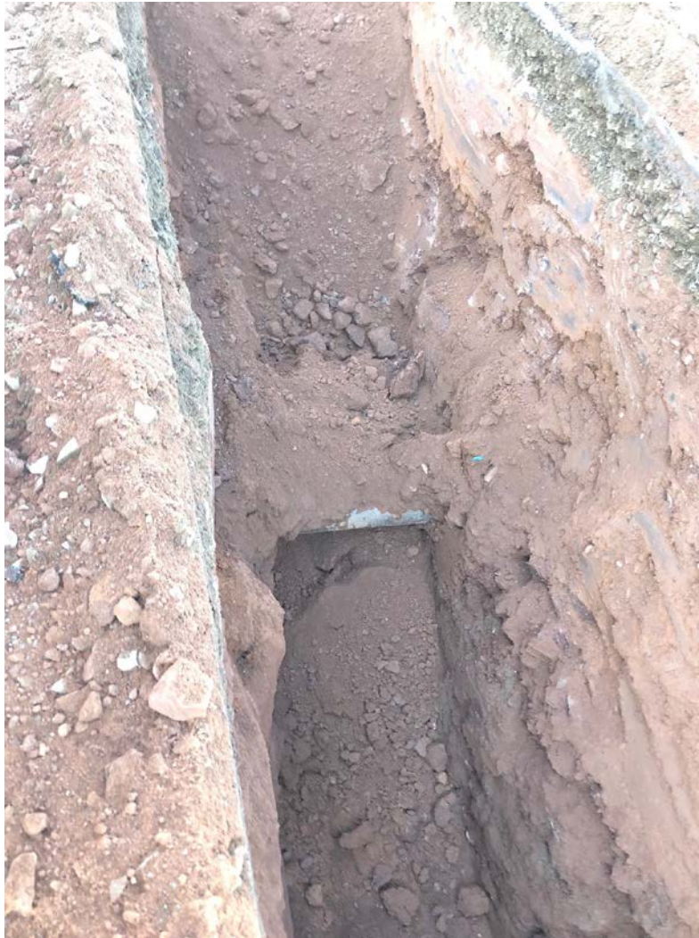
Figure 6 – Ludlow exposes an existing 8” water line at ~ Station 600+20.
