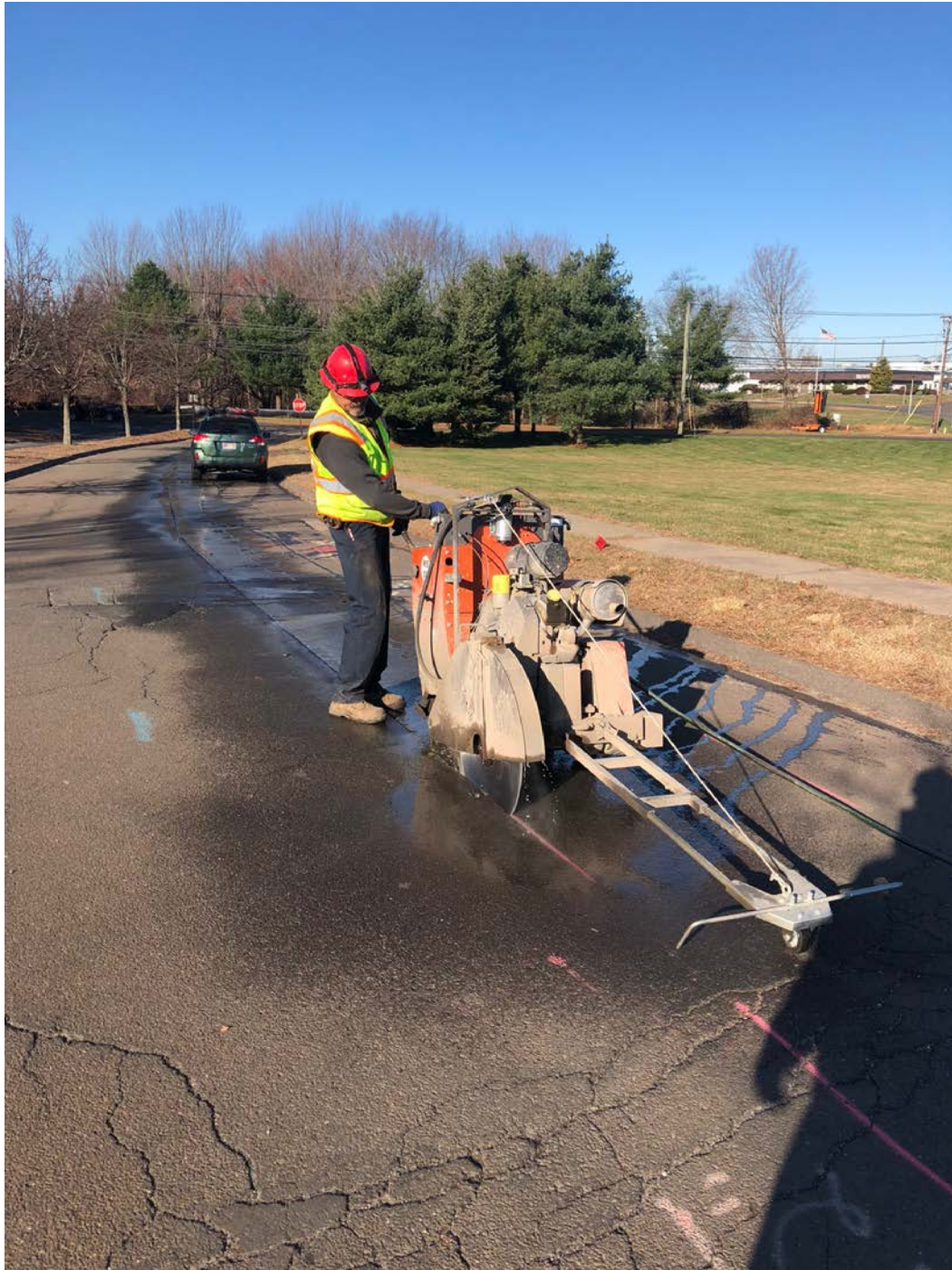
Figure 11– Ludlow saw-cutting asphalt along Talcott Ridge Drive. Route 17 in the background.
