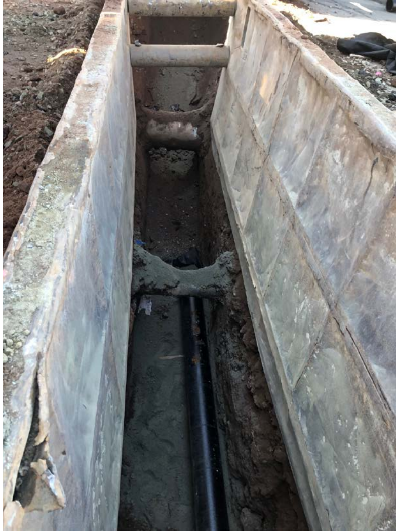
Figure 8 – 8" DIP placed beneath existing 8" water line. The existing storm drain is visible at the top of the photograph.
