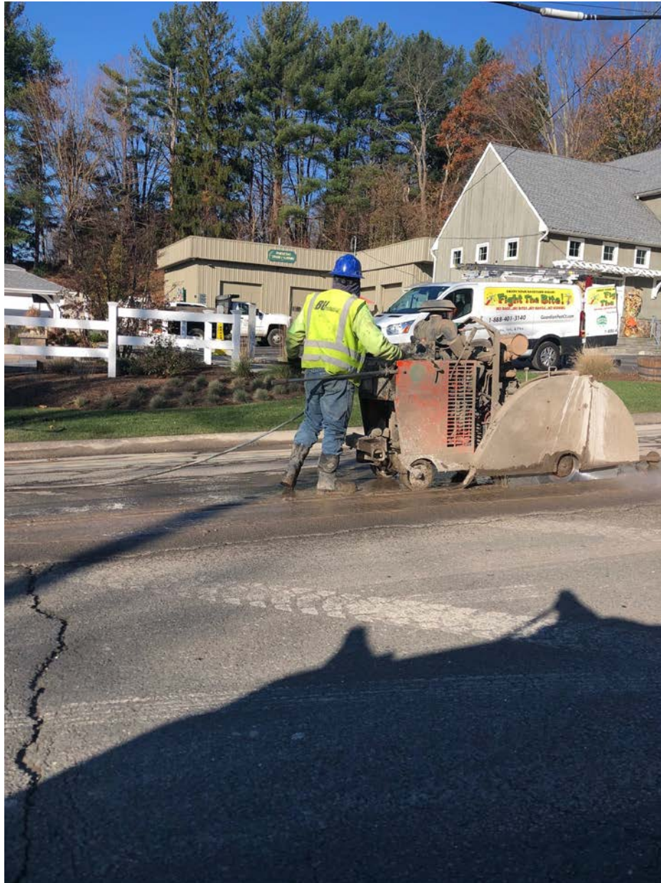
Figure 10– Ludlow saw-cutting asphalt along Route 17; southbound lane.
