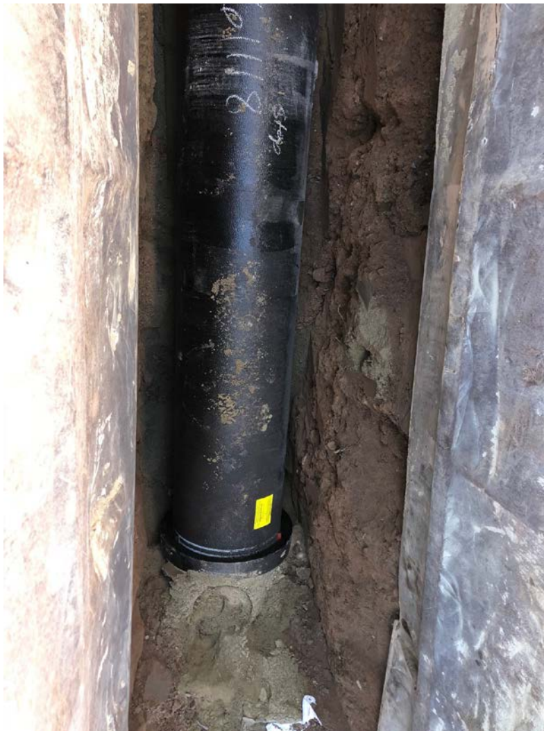
Figure 2 – Third section of 20” pipe installed.
