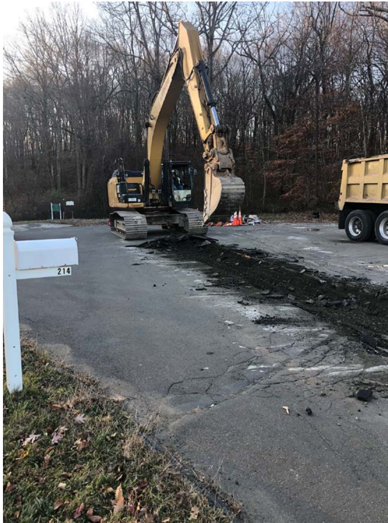
Figure 1 – Ludlow removing asphalt from top of trench.
