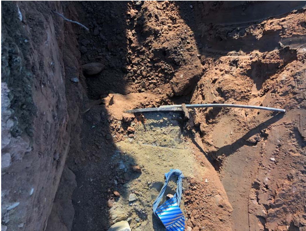
Figure 5 – 11.25° M.J. bend that was installed between 10.5' and 9.5' sections of 20" pipe.
