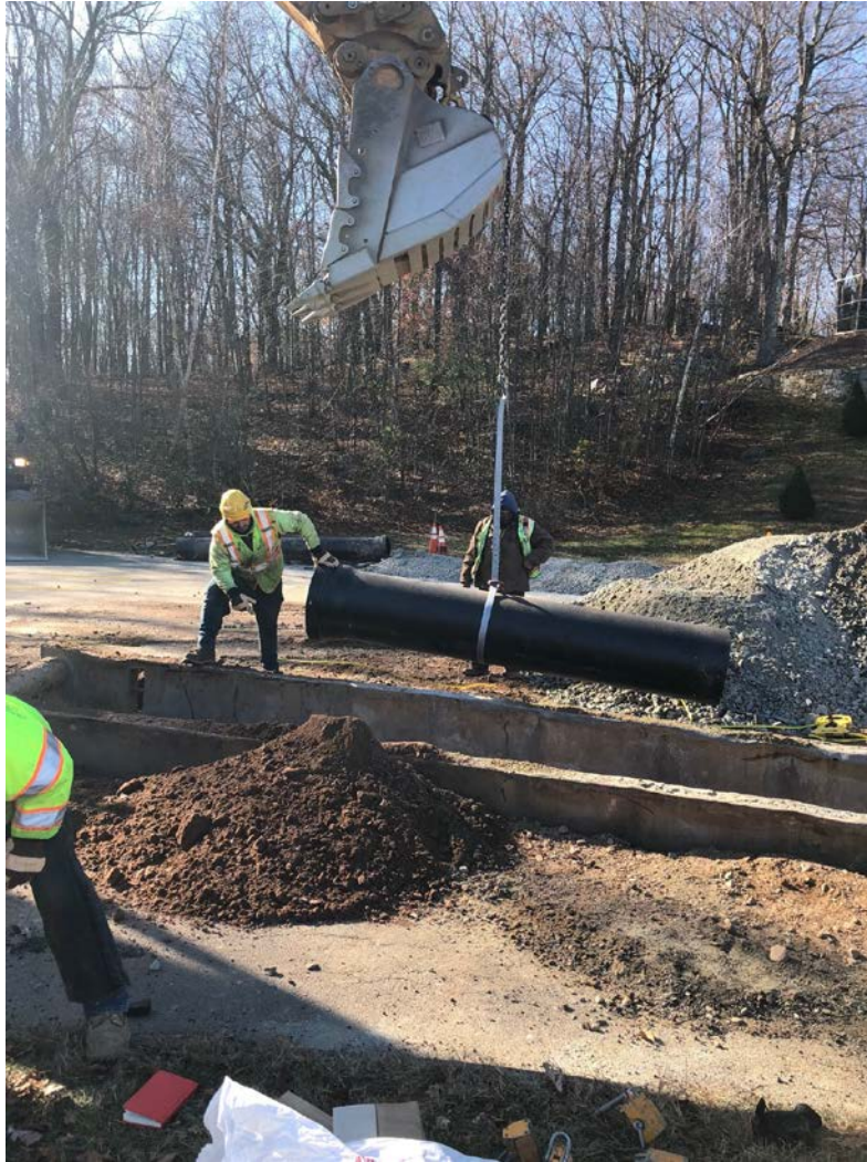
Figure 6 – Lowering 9.5' section of 20" pipe to complete 11.25° MJ bend.
