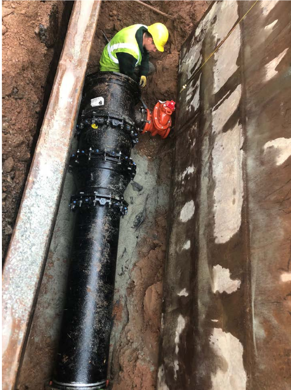
Figure 8 – Installation of 16"x20" MJ reducer and 20"x20"x6" hydrant tee. View to the south.
