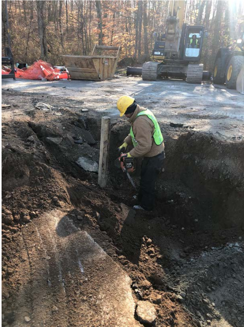
Figure 7 – 4"x4" timber placed at end of pipe run to mark its location. Talcott Ridge Road cul de sac; view to the southeast.
