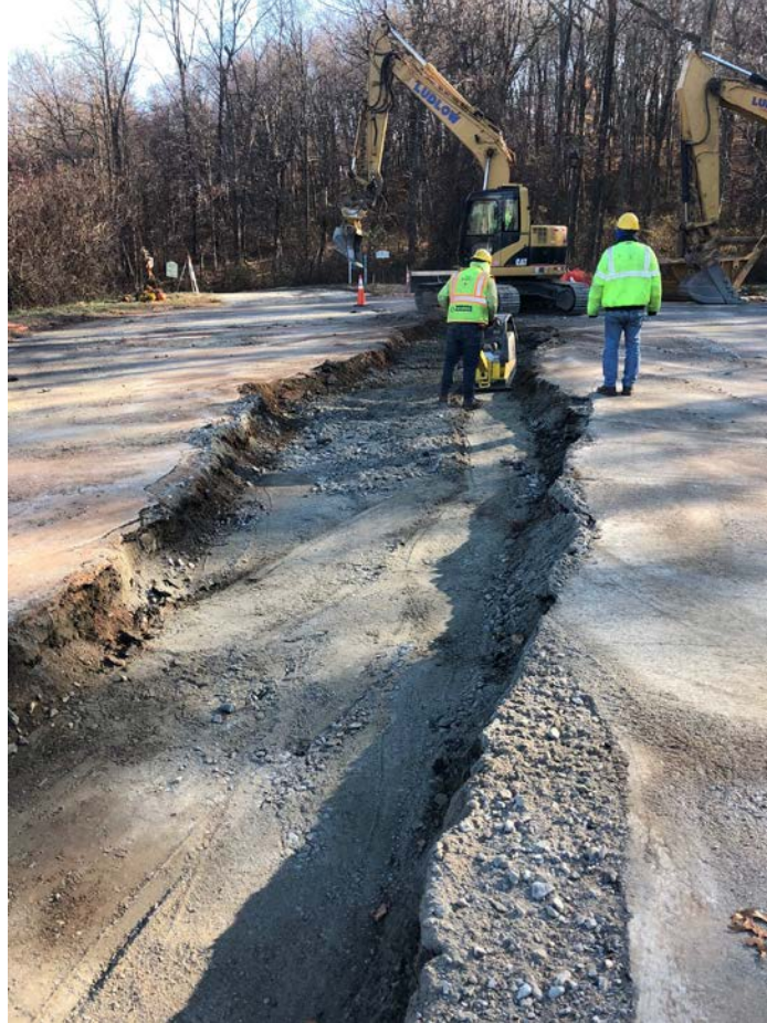
Figure 9 – Compacting 3” minus gravel prior to placement and compaction of processed stone.
