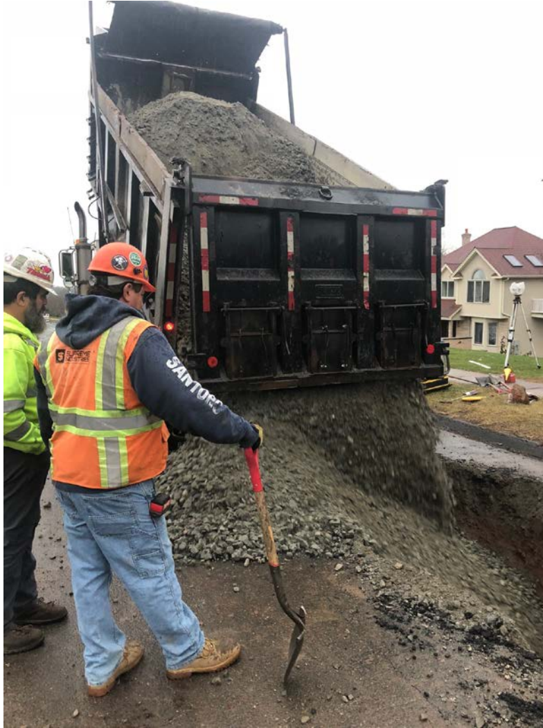
Figure 7 – 3" minus gravel being placed in trench. View to the northeast.
