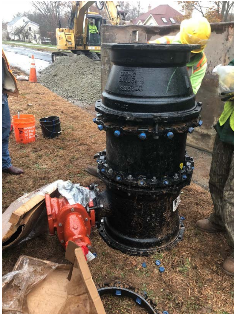
Figure 5 – 16"x20" reducer connected to 20"x20"x6" hydrant tee with a ~2-foot section of 20" pipe.
