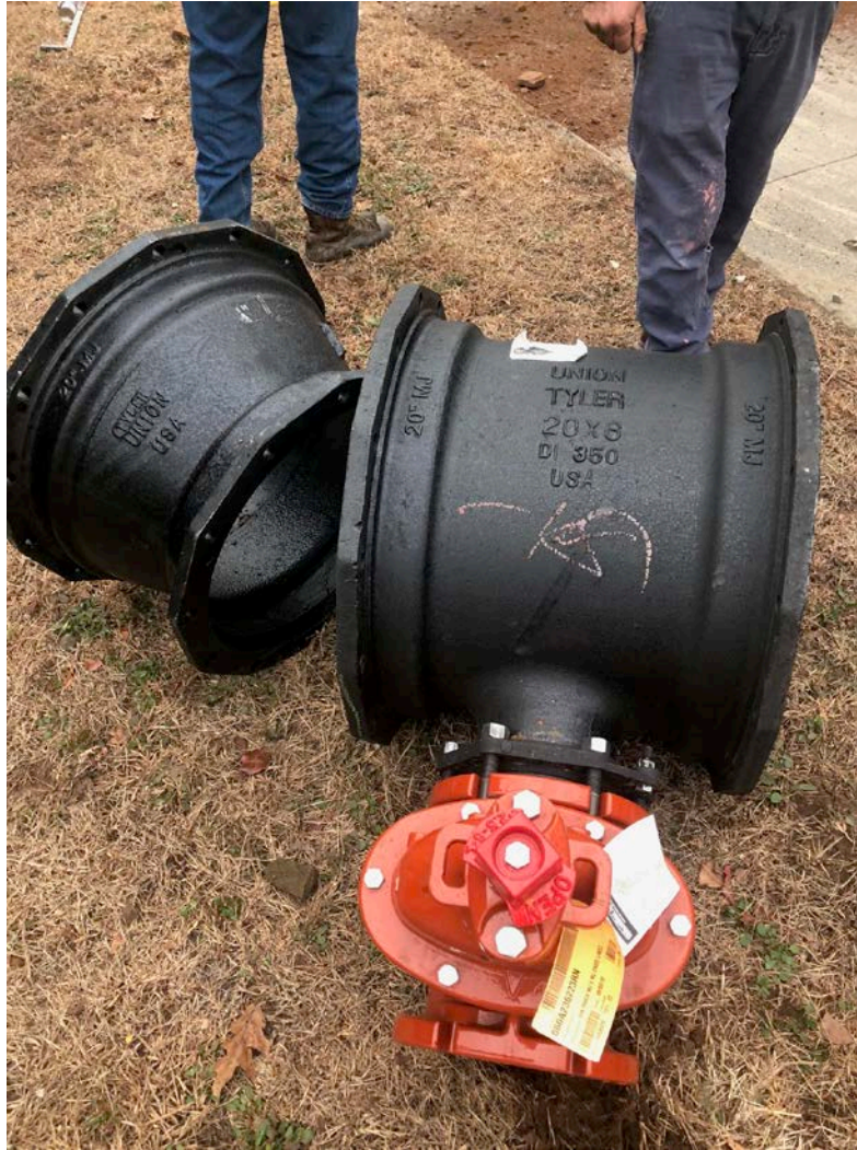
Figure 4 – 16"x20" reducer on the left and 20"x20"x6" hydrant tee on the right.
