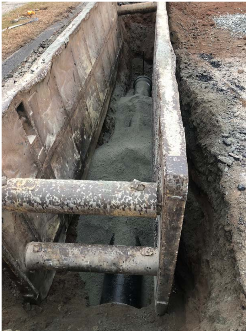
Figure 1 – First section of placed 16” pipe, view to the south.
