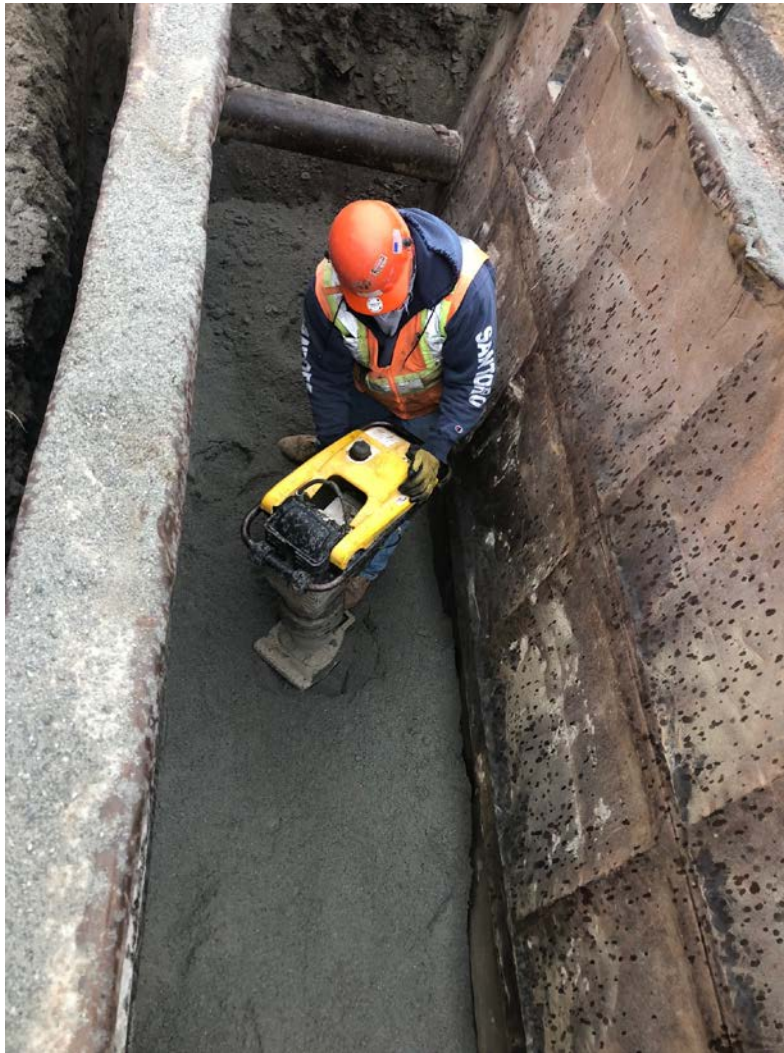
Figure 2 – Compacting sand placed over first section of placed 16” pipe, view to the south.
