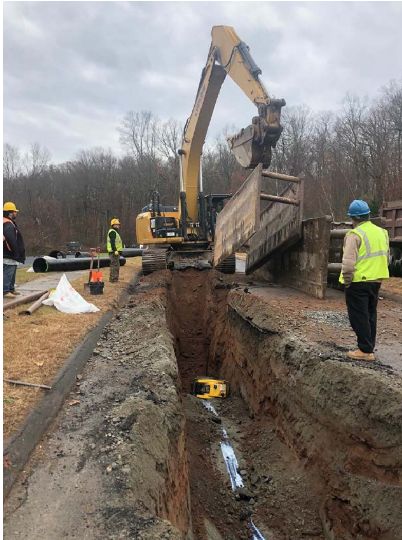
Figure 6 – Trench box being placed in trench.
