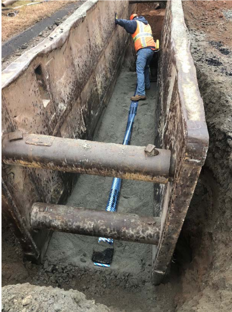
Figure 3 – Silver/blue caution tape placed over 16" pipe, view to the south.
