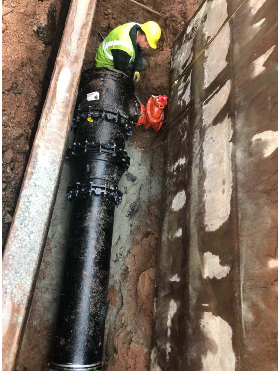
Figure 8 – Installation of 16"x20" reducer and 20"x20"x6" hydrant tee. View to the south.
