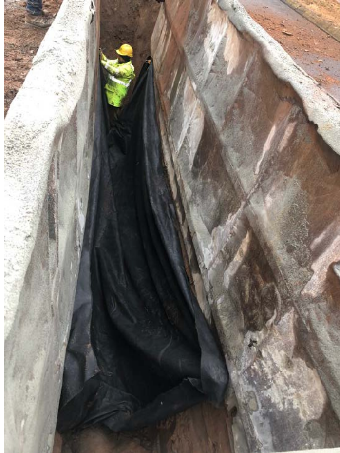
Figure 9 – Placement of geotech fabric on bottom of trench. View to the south.
