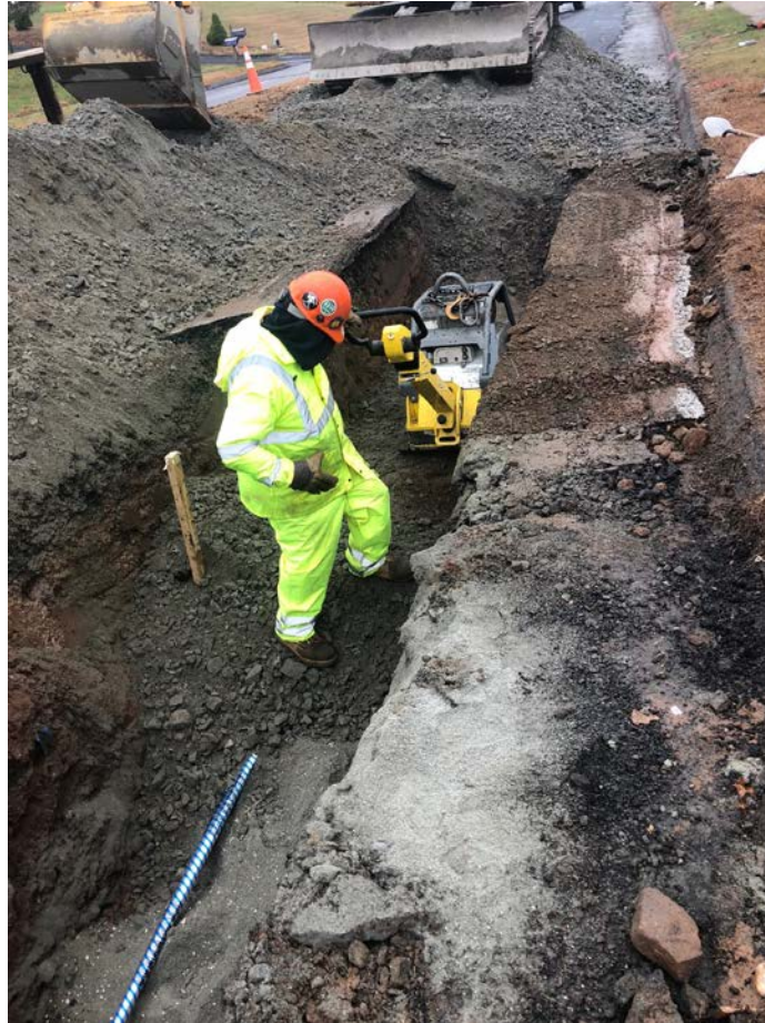
Figure 11 – Compacting 3” minus gravel in trench. View to the north.
