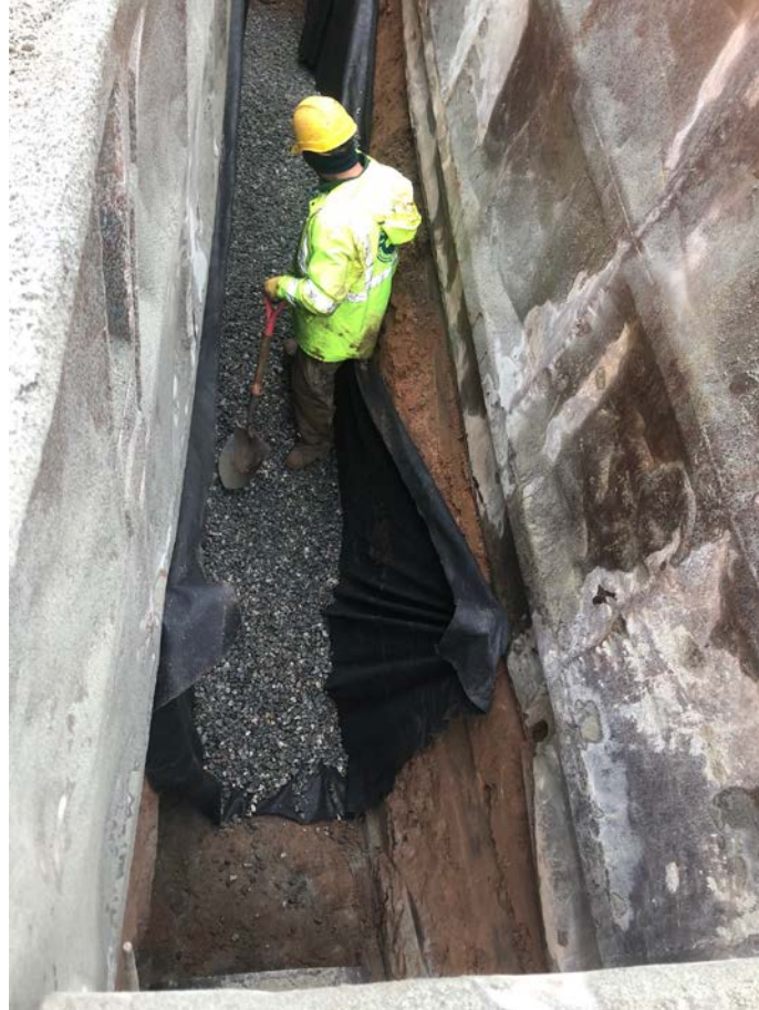
Figure 10 – ¾" minus gravel placed on top of geotech fabric. View to the south.
