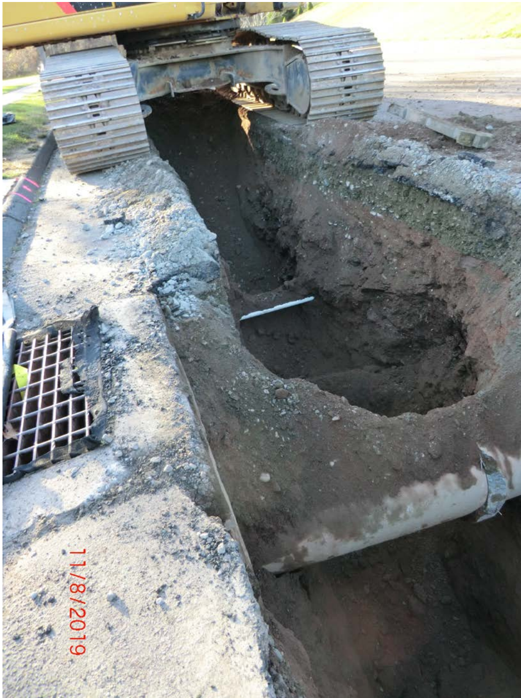
Figure 2 – Facing south and down, the only utilities crossed today. 18” catch basin drain (foreground) and electrical conduit (background).
