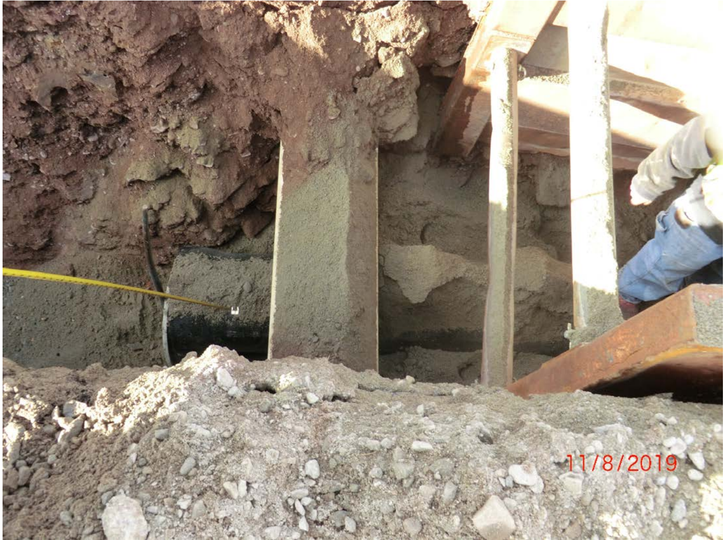
Figure 3 – End of first 20-foot run 16" DI. Depth to top of pipe roughly 6.5-7 feet.
