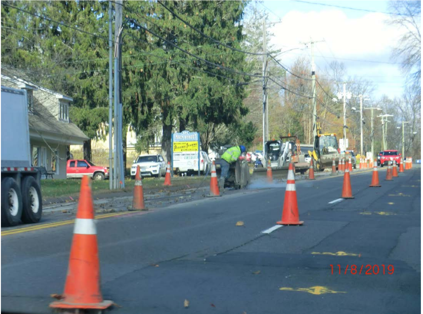
Figure 4 – Facing north, saw cutting Route 17 Main Street in Durham. Lanes fully coned.
