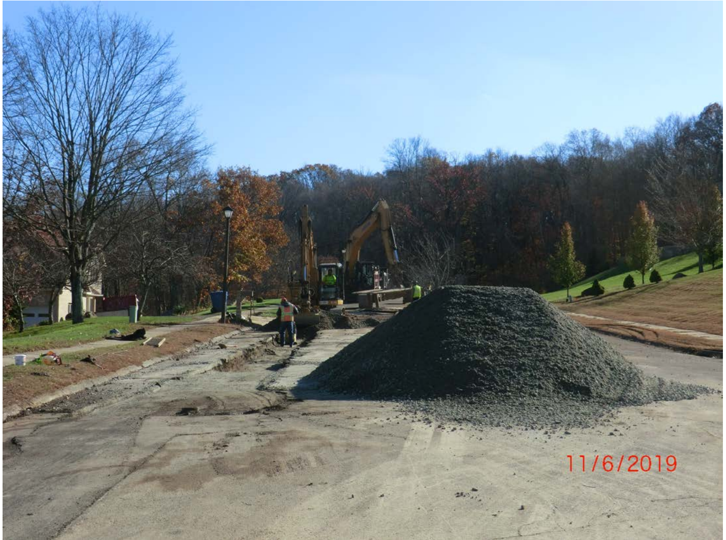
Figure 11 – Facing south, pile of 1” process waiting to be installed in the final lifts of trench.
