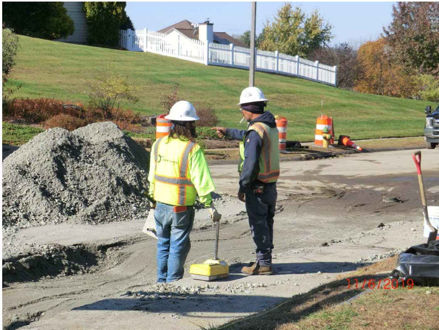
Figure 6 – Compaction testing. Upper two lifts done today, bottom three lifts done yesterday.
