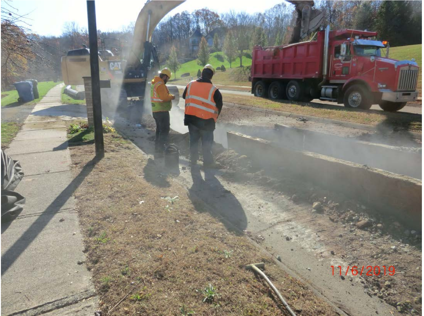
Figure 3 – Facing southwest. Running into ledge along the trench – indicated by the ‘smoke’. Slows progress due to the need to dig it out.
