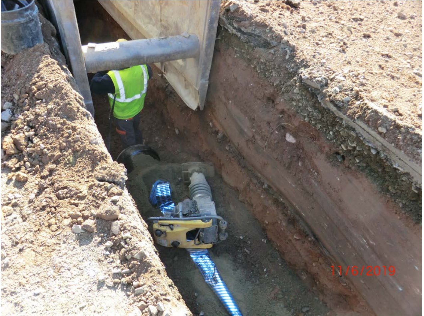
Figure 8 – Typical. Preparing for next stick of 16” DIP to be installed.
