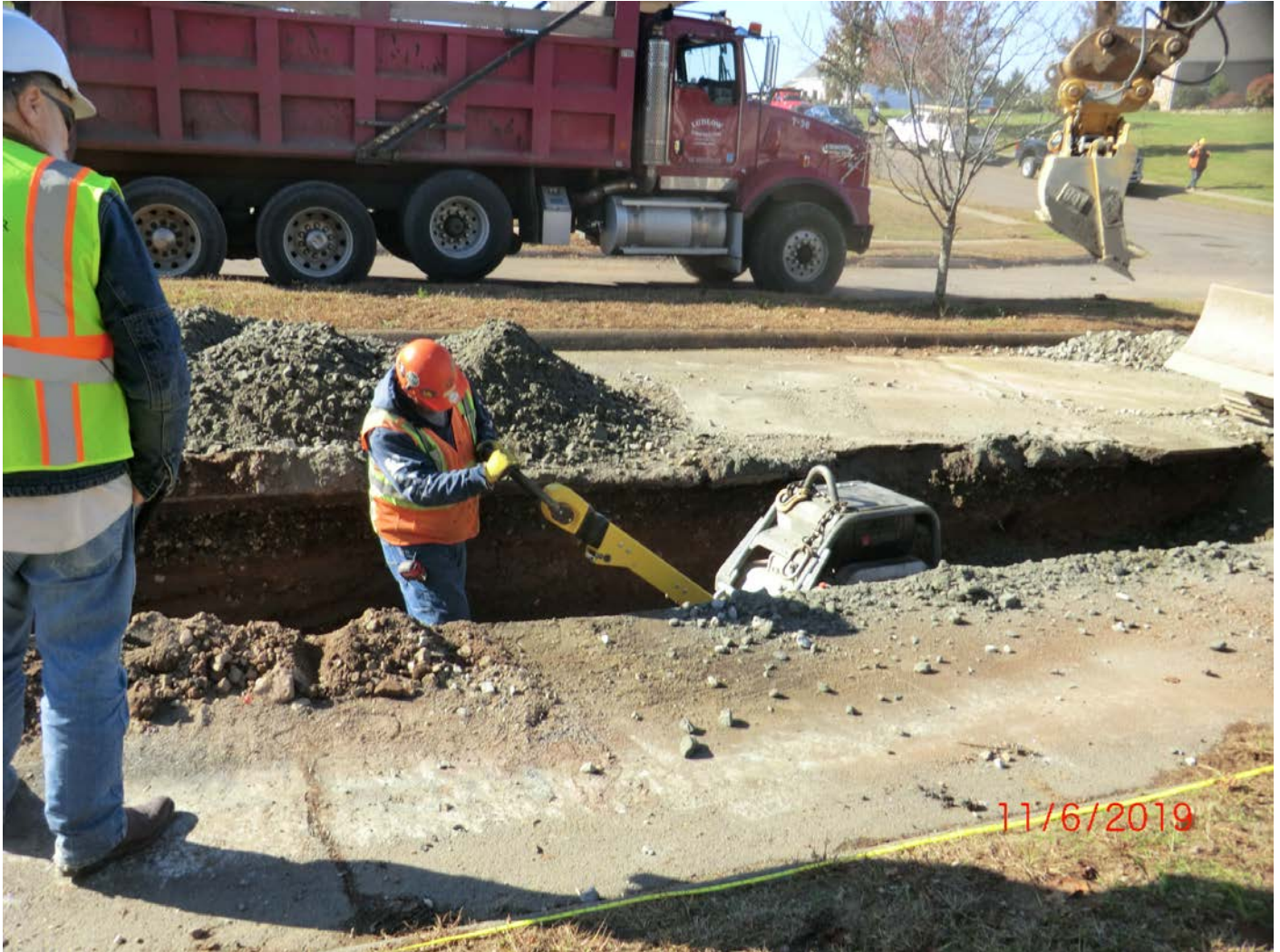
Figure 7 – Facing west. Running the Wacker compaction plate. Upper right of the photo is ‘upper’ Watch Hill Drive.
