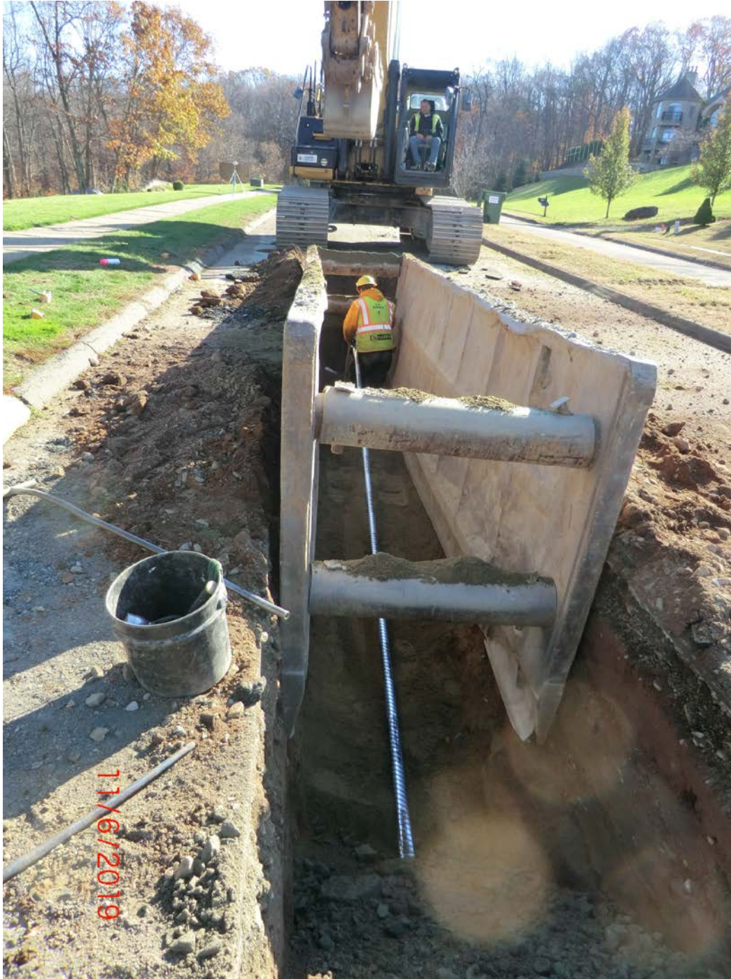
Figure 10 – Facing south, last run of pipe for the day ending at Sta. 34+04.62. Running Water Line Caution tape over top of 16" DIP
