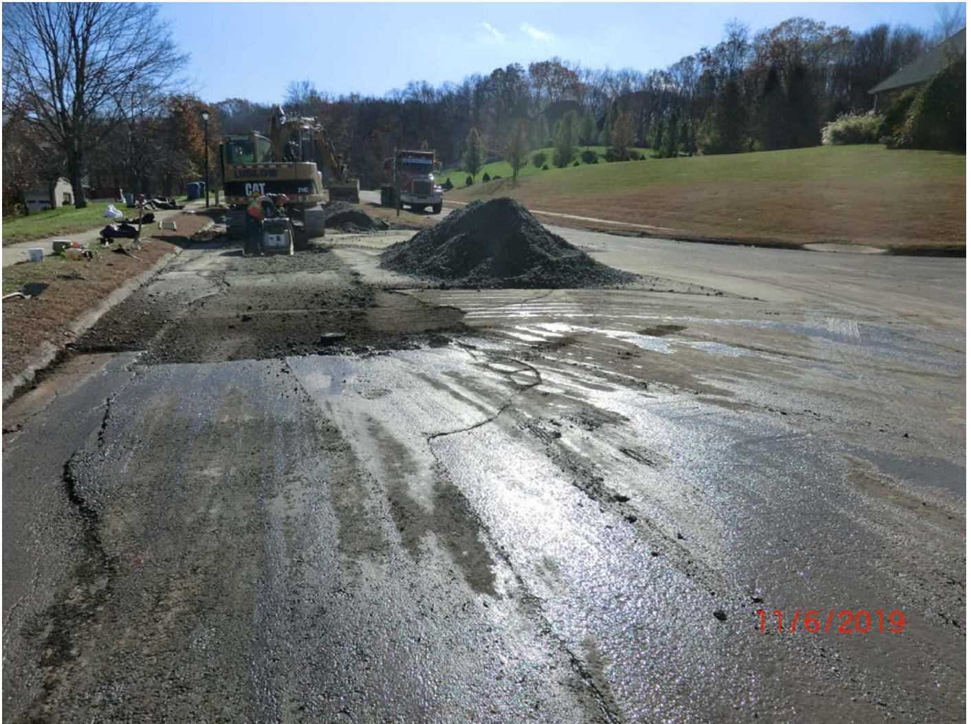
Figure 1 – Facing south, today's starting station 35+63.95 on Talcott Ridge. To the right of the photo is 'upper' Watch Hill Drive. Cap seen at start of road cut is the valve access to a 16" butterfly valve, one of two in the 16x8" tee assembly, which was the final install yesterday 11/5. The tee will connect an 8" line up Watch Hill to a hydrant replacement.
