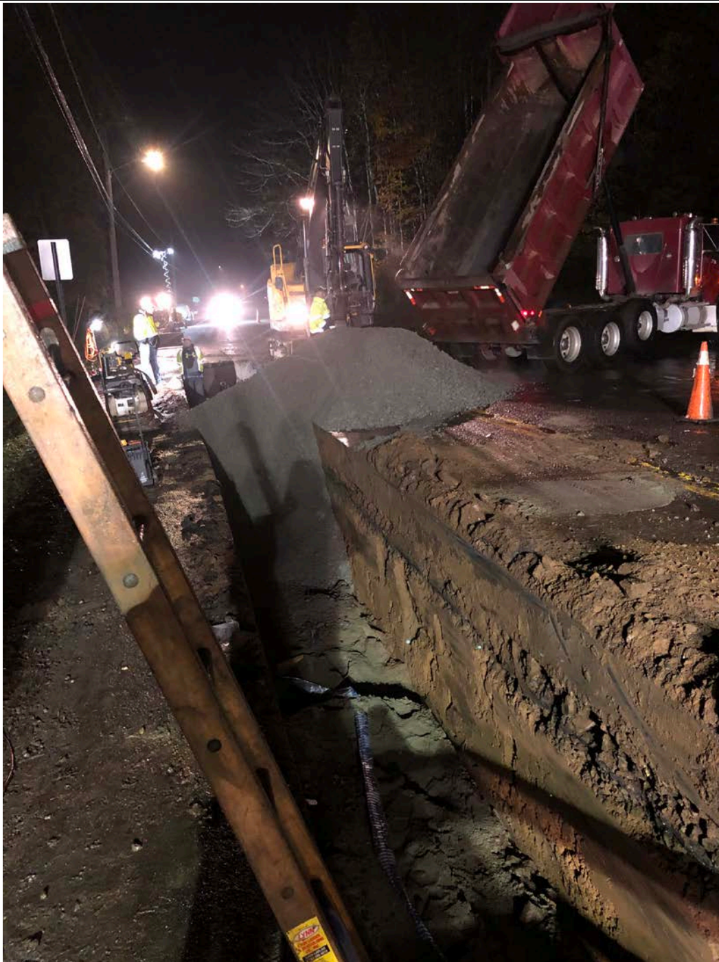
Figure 4 – Backfill pile dumped, will be 1 st lift
