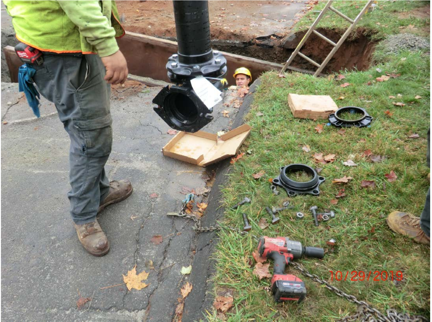
Figure 6 – Hydrant connection with manufacturer gland removed – on grass with bolts. In upper right of picture is the Mega-Lug restraint with check lugs (blue).
