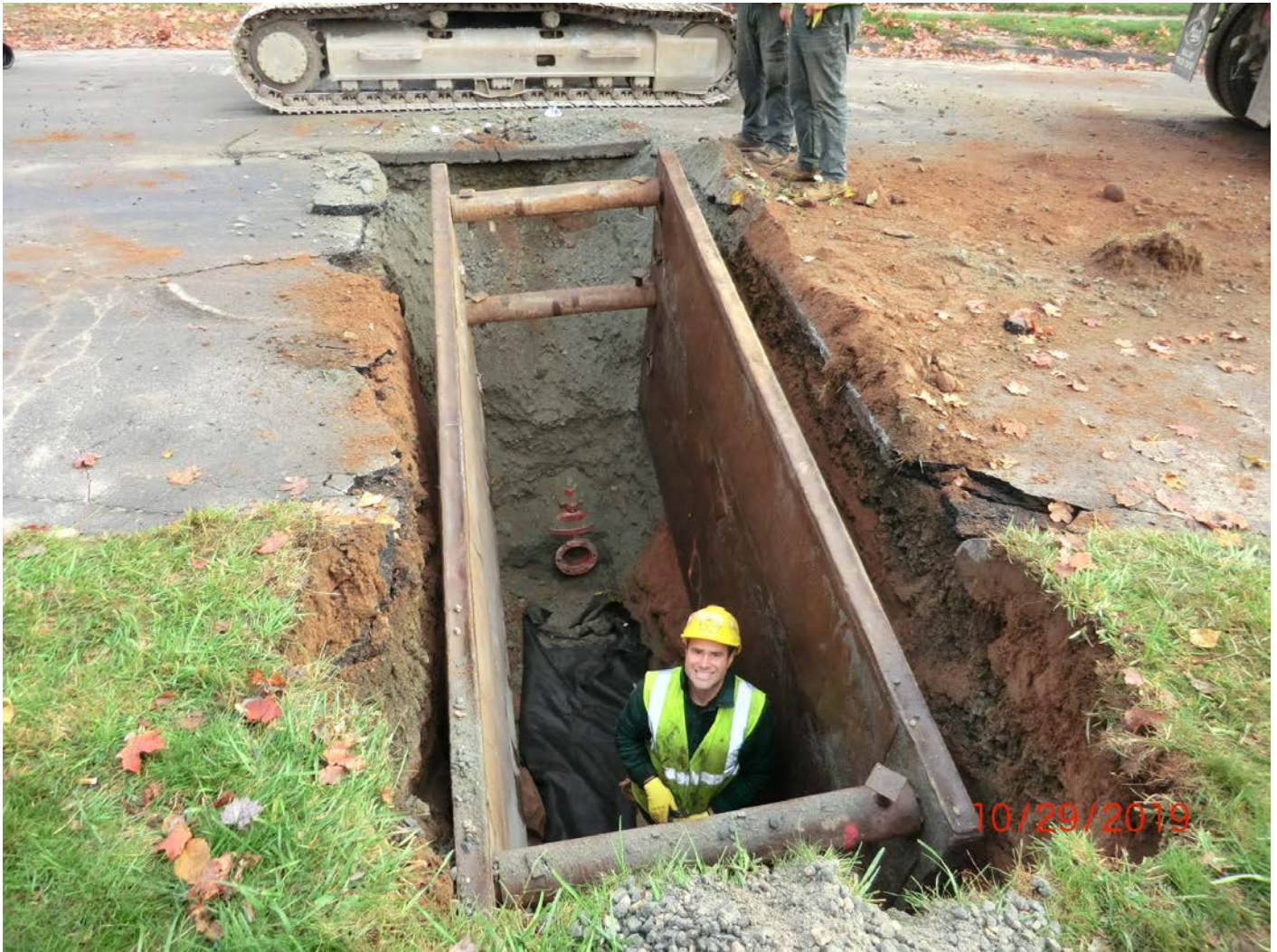
Figure 2 – The man in the box. Preparing base for hydrant line. 6" gate valve (red) seen in center of picture.
