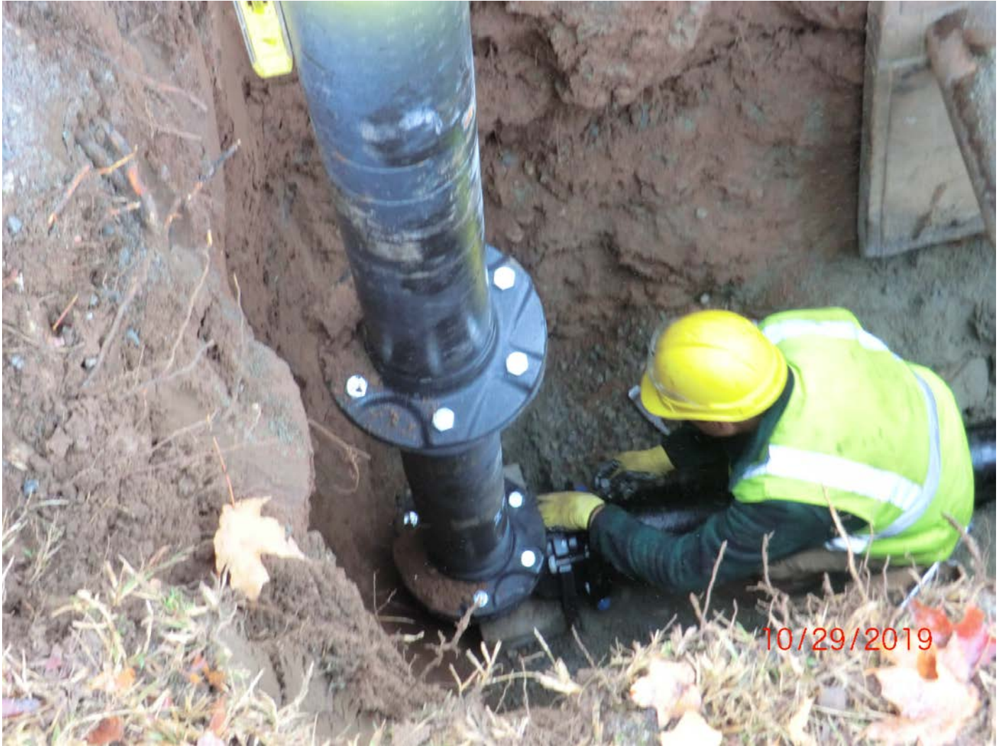
Figure 15 – Attaching hydrant assembly to 6” line with Mega-Lug restraint.
