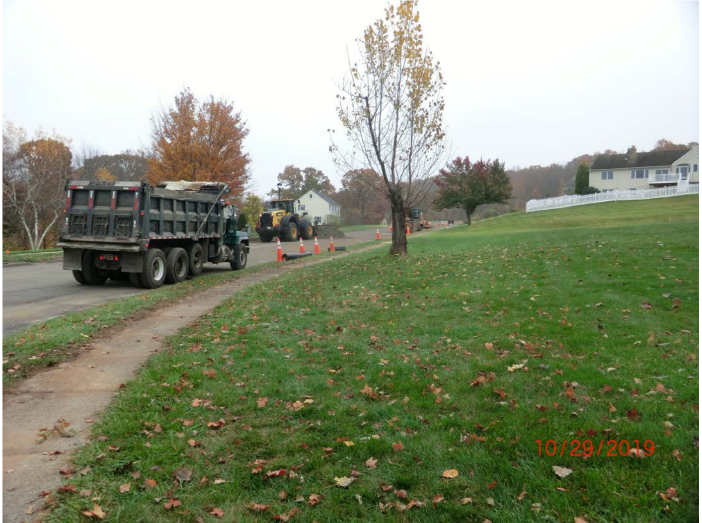
Figure 11 – Mis-communication. Processed fill dropped up the street near yesterdays ending point. Driver unaware that water main pipe was not being installed today. Fill was bucket loaded and delivered to the hydrant installations. Created a wider spread area to clean at the end of the day.
