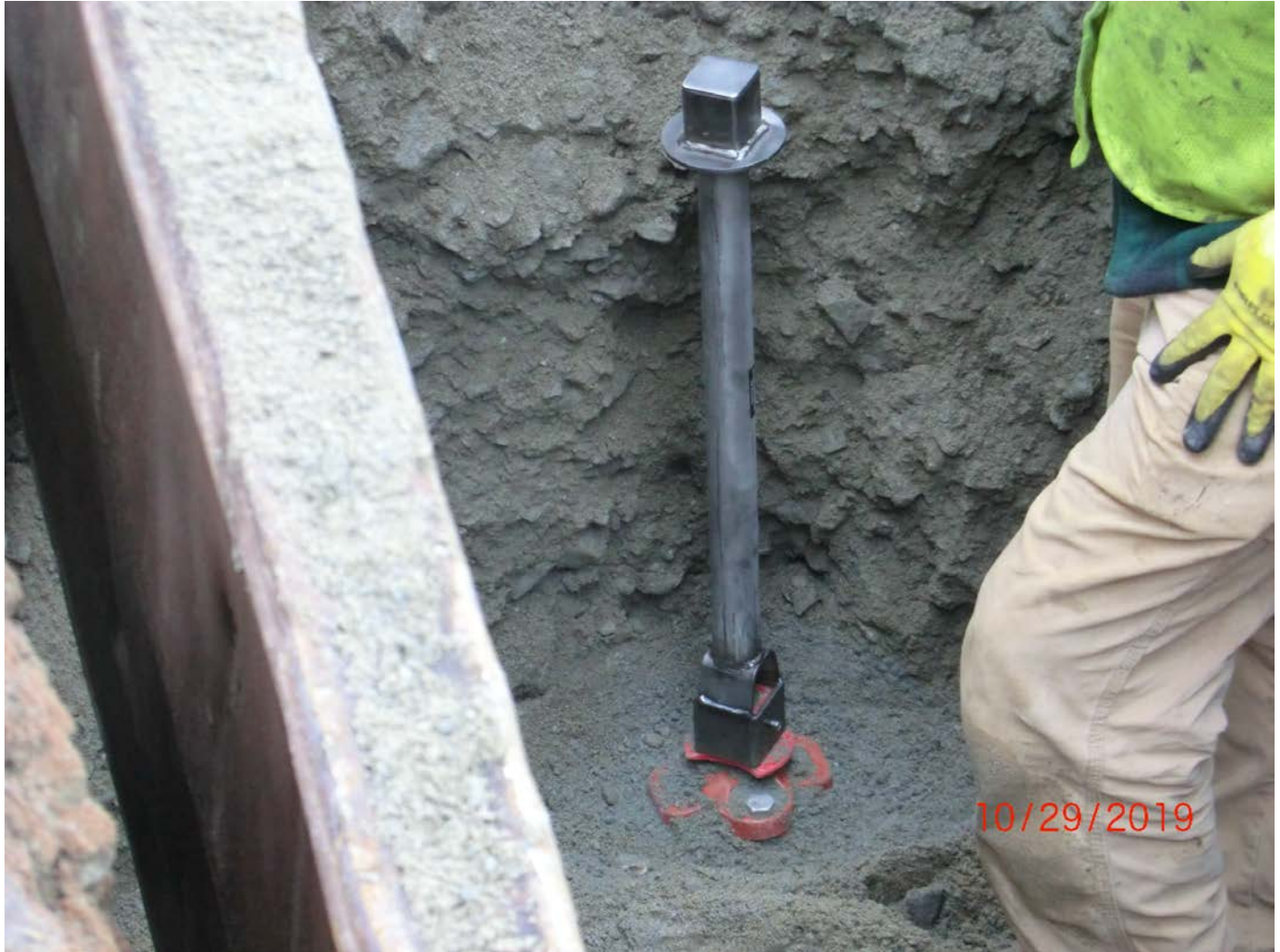
Figure 8 – Street valve connector. Top of gate valve.
