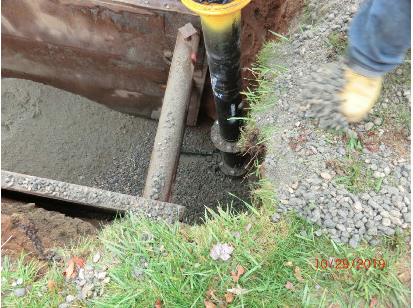
Figure 10 – Crushed stone backfill around base of hydrant and stone dust over pipe. Crushed stone covered by geotextile fabric and entire length covered in stone dust. Compacted and then covered with processed fill compacted in lifts.
