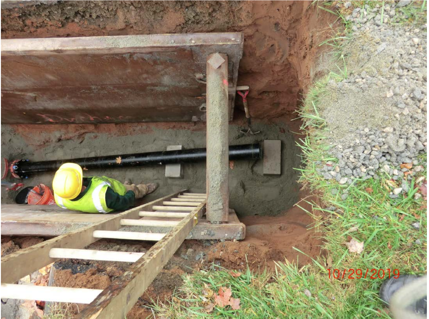
Figure 4 – Awaiting Hydrant Assembly
