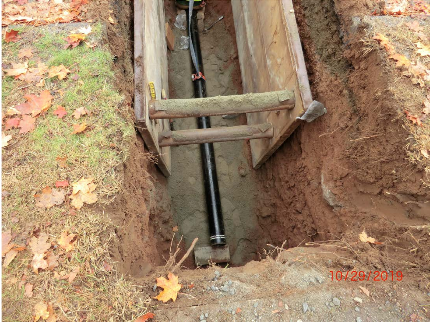
Figure 14 – Awaiting hydrant assembly. Note 8” block for elbow to set on (bottom of picture).
