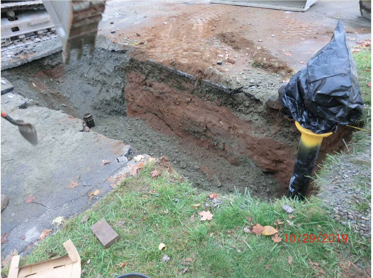
Figure 12 – Backfilling with processed backfill. On right side of picture note bag over hydrant to indicate not in use. Left side of picture is valve extension and riser pipe; note cap on upside down to prevent processed fill from getting into riser.
