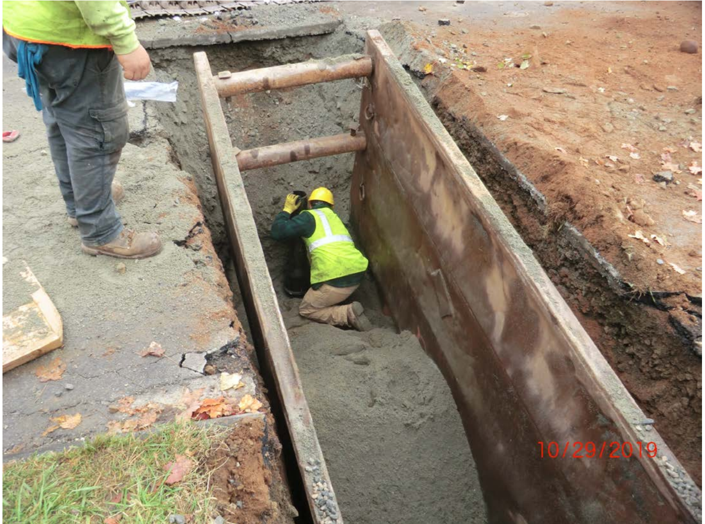
Figure 9 – Valve box placed over street valve connector (pictured in previous figure).
