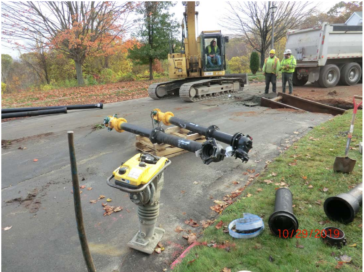
Figure 1 – Hydrant Assemblies. First location on Talcott Ridge. Station Old 40+44.38 / New 40+49.21
