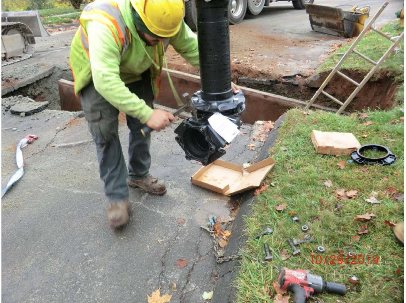
Figure 5 – Removing manufacturer gland. Note bolts already removed, laying on grass.
