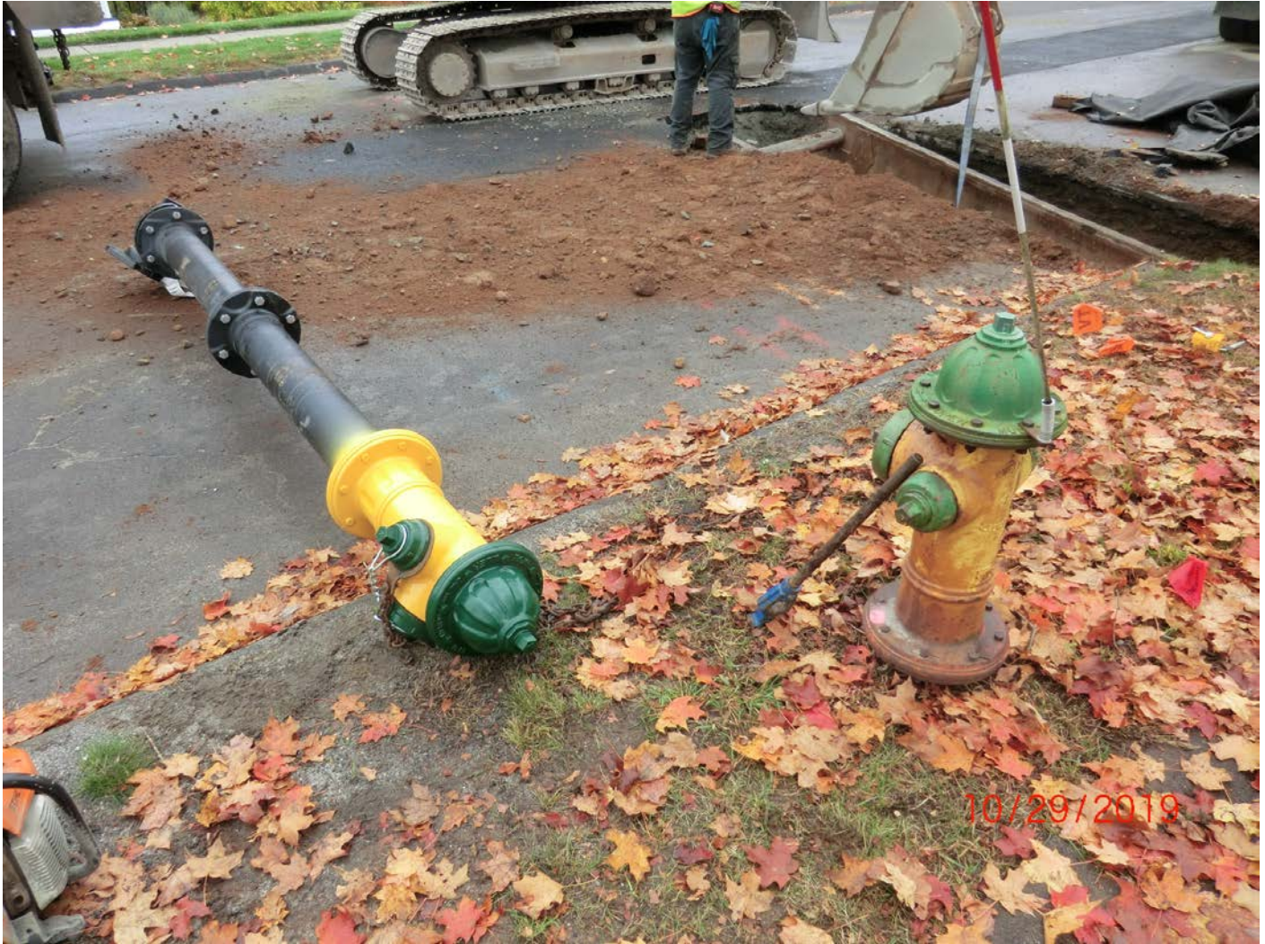
Figure 13 – Existing fire hydrant and new fire hydrant to be installed. Second location at Station Old 41+42.34 / New 41+47.17.
