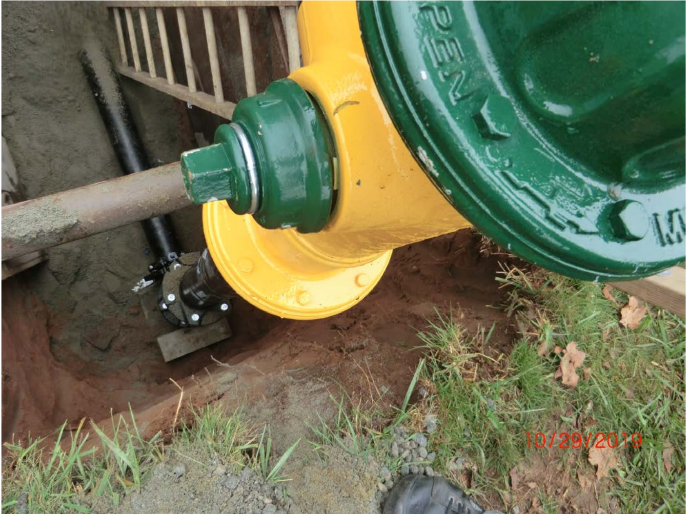
Figure 7 – Completed hydrant assembly connection. Note one 8” thrust block set behind elbow and one 8” block set under the elbow for support (mostly hidden by stone dust, only edge visible).
