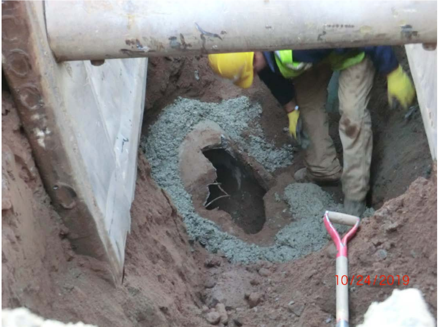
Figure 4 – Cement 'gasket' set completely around hole in drain.
