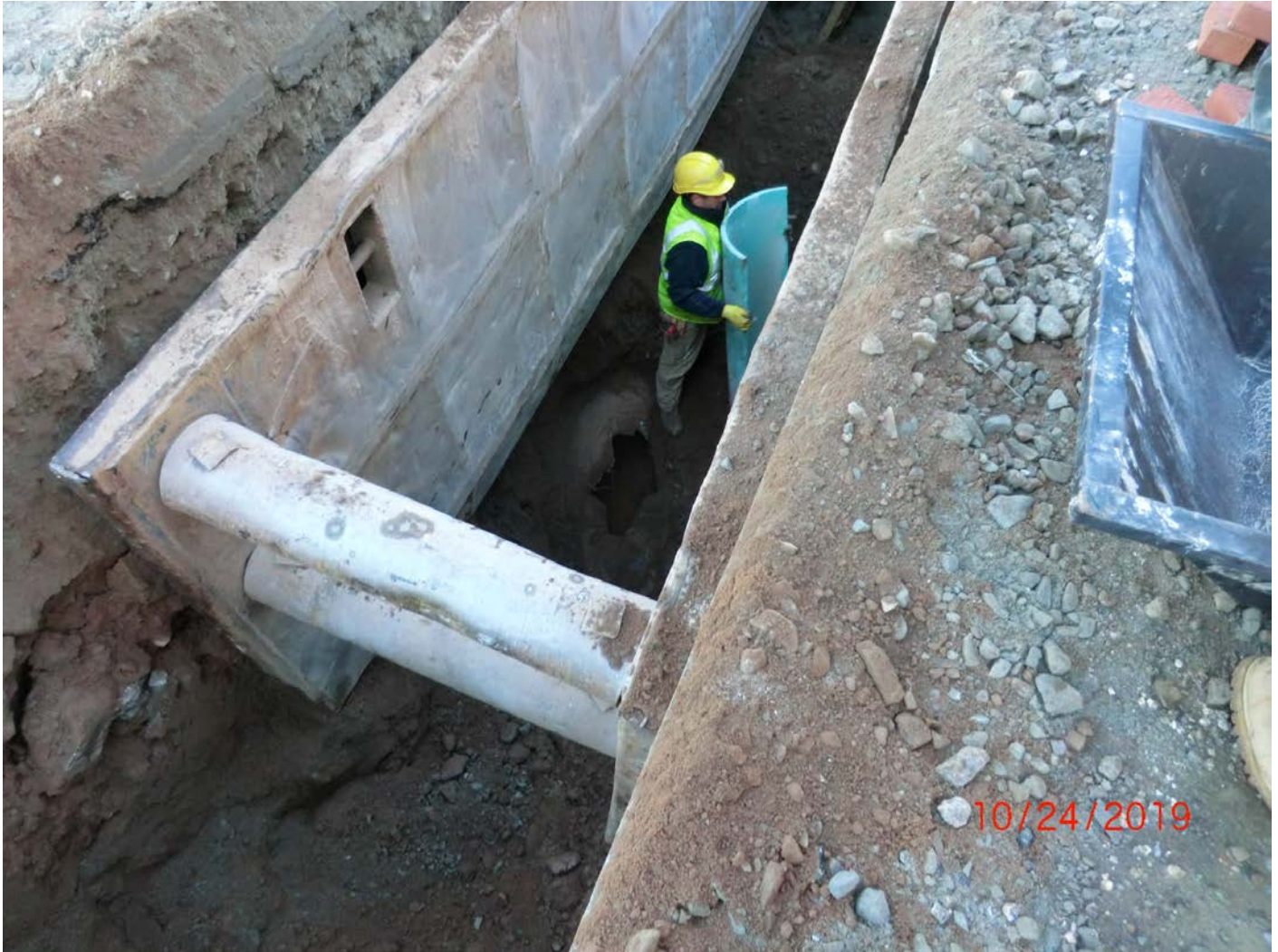
Figure 3 – A partial segment of ADS pipe to be fitted over hole.
