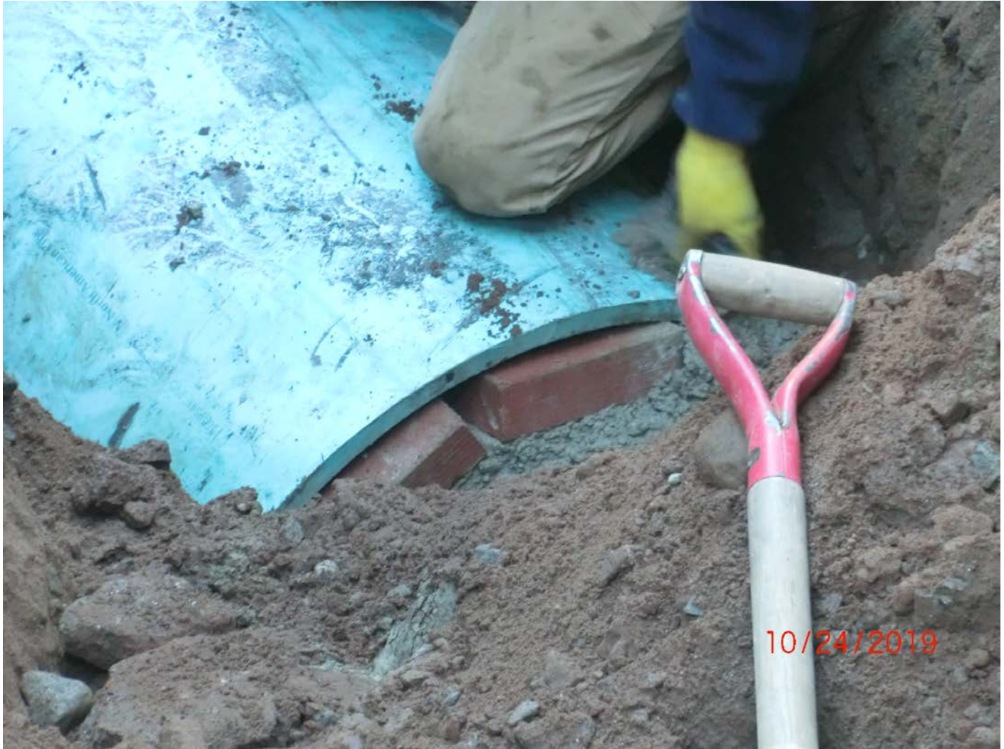
Figure 6 – Ends bricked in for added support and strength.
