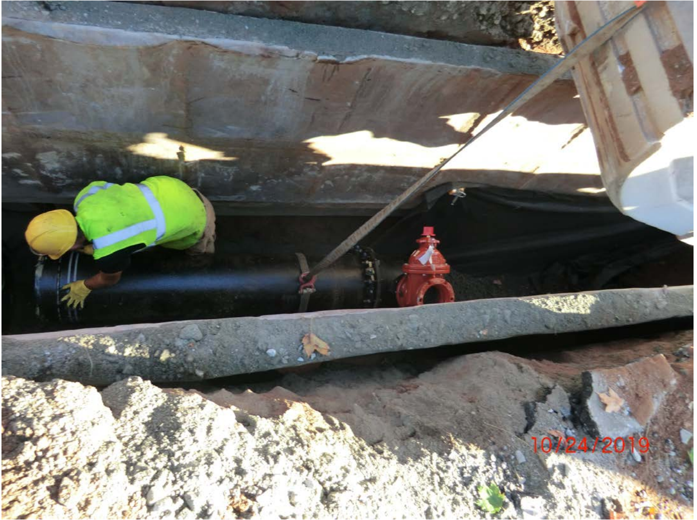
Figure 11 – Installation of Hydrant T section. Note that the T points up at first to fit through the trench box and is then rotated into the proper position once pipe is laid down.
