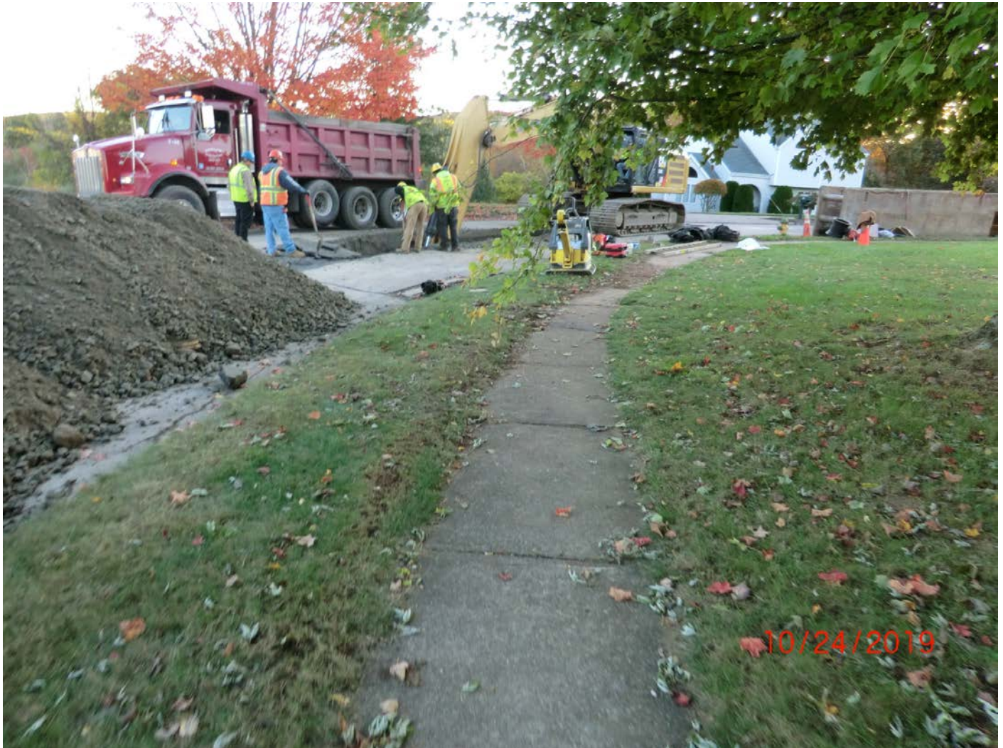
Figure 1 – Facing NE (124 Talcott Ridge seen in upper right of photo). Start of day. Excavating from 22.5-degree bend installed at Sta. 40+71.71 to 18" broken drainage line.
