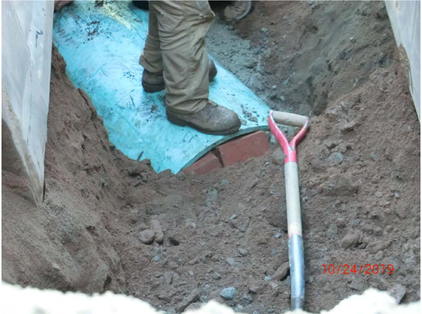
Figure 8 – Final brick face. This was done on both sides of pipe.
