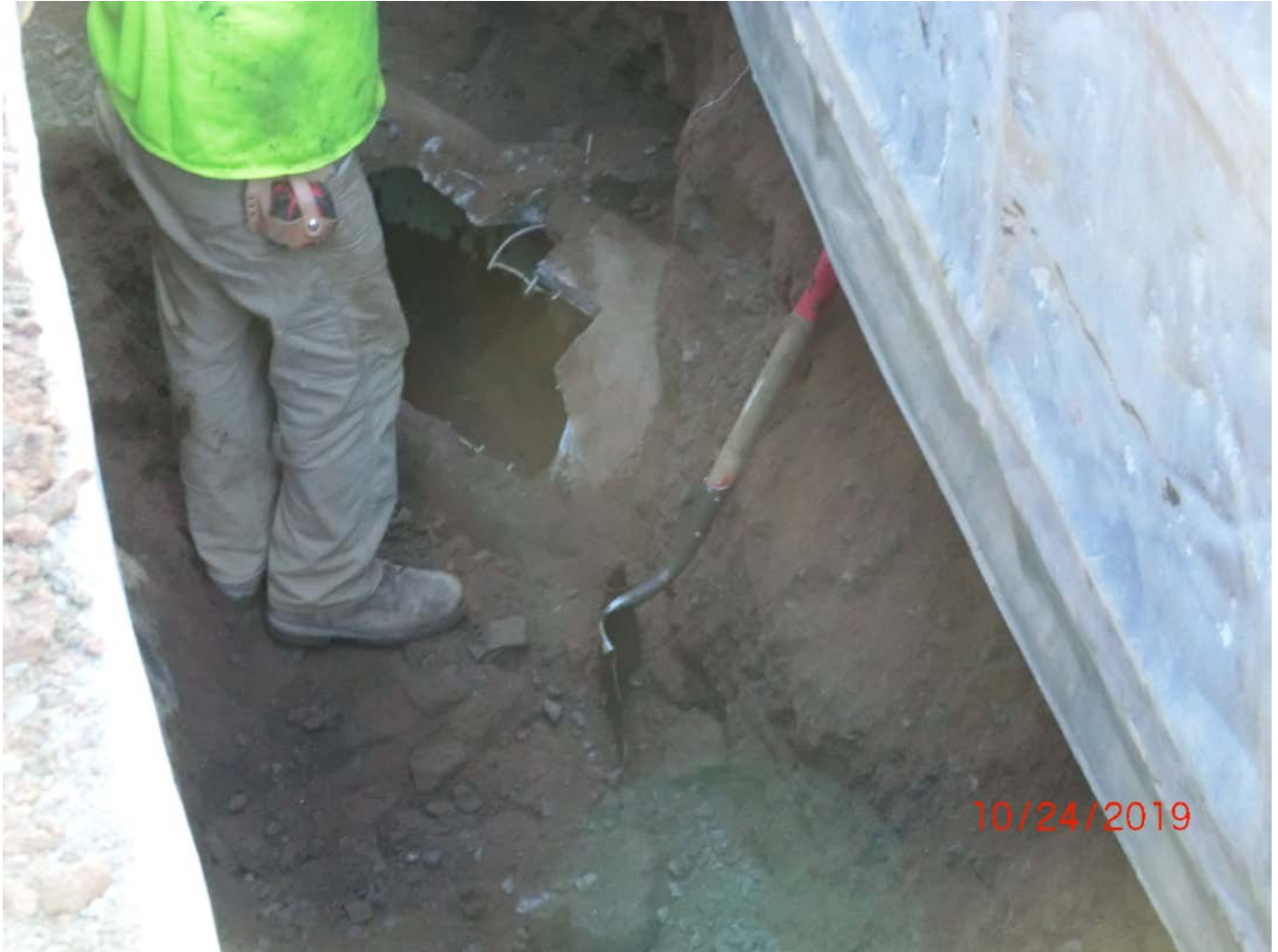
Figure 2 – Excavated to broken drain line. Cleaning up and exposing line so as to repair the hole.
