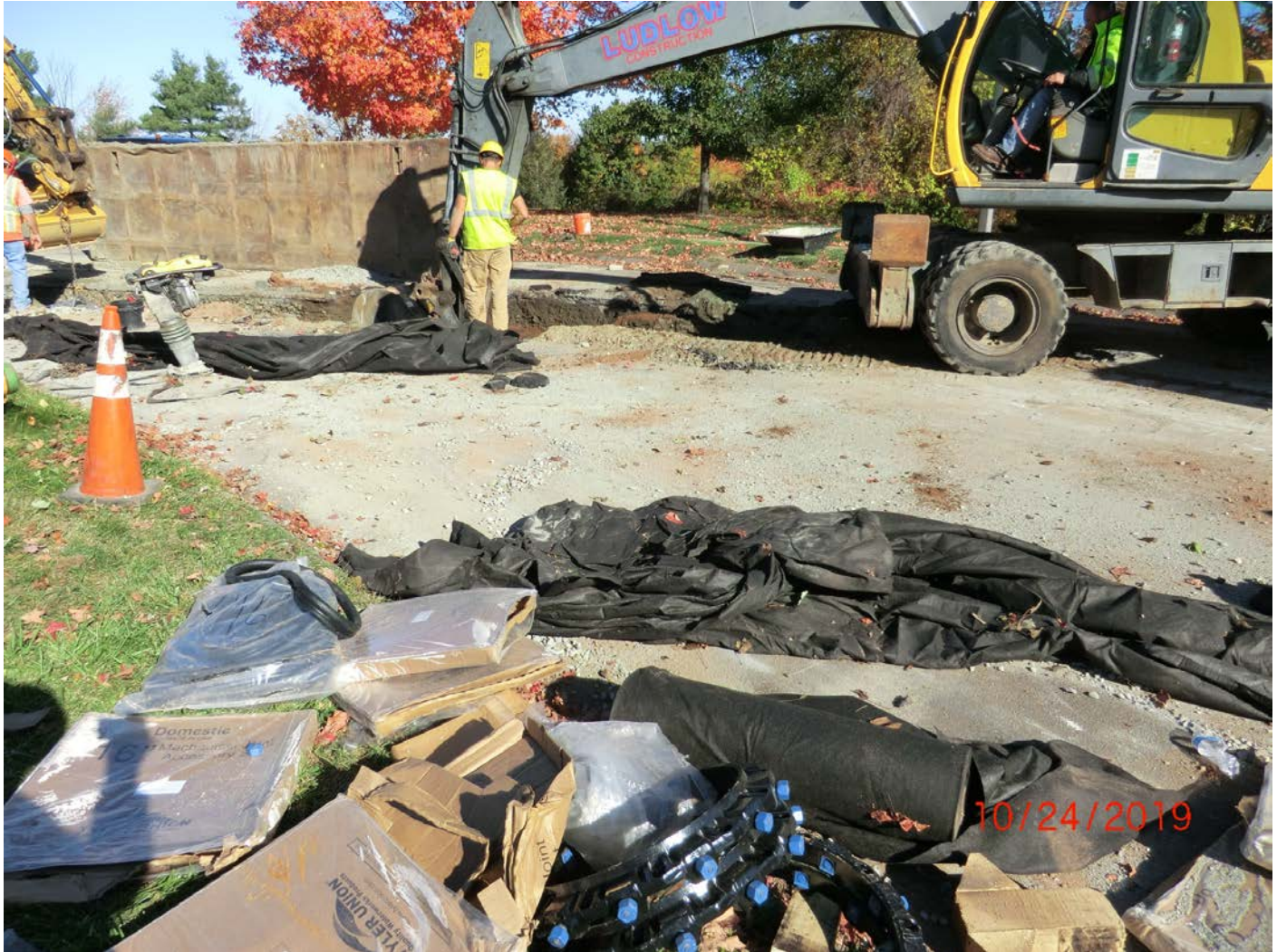
Figure 12 – Excavating a slightly larger hole for the installation of the 12” water line Tee. The existing 12-inch water line will be connected at a later time. Note that the Large Excavator has been switched out for the smaller Rubber Wheeled Excavator. This was done to avoid damaging the driveway of 124 Talcott Ridge, which is located behind the excavator to the right of this picture. Also note that the town ROW and existing valve assembly is located on the other side of this trench to the north side. Picture is taken facing north.
