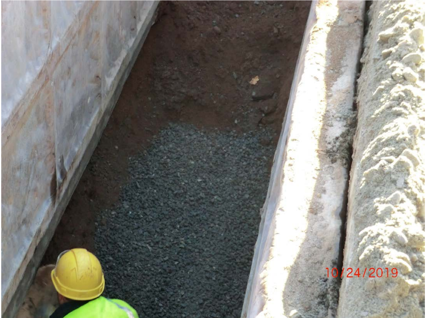
Figure 10 – Not shown, is geotextile fabric placed over the entire patched hole, then covered by 12 inches of gravel to raise the bed to the elevation needed to lay the 16" DI pipe over this section.
