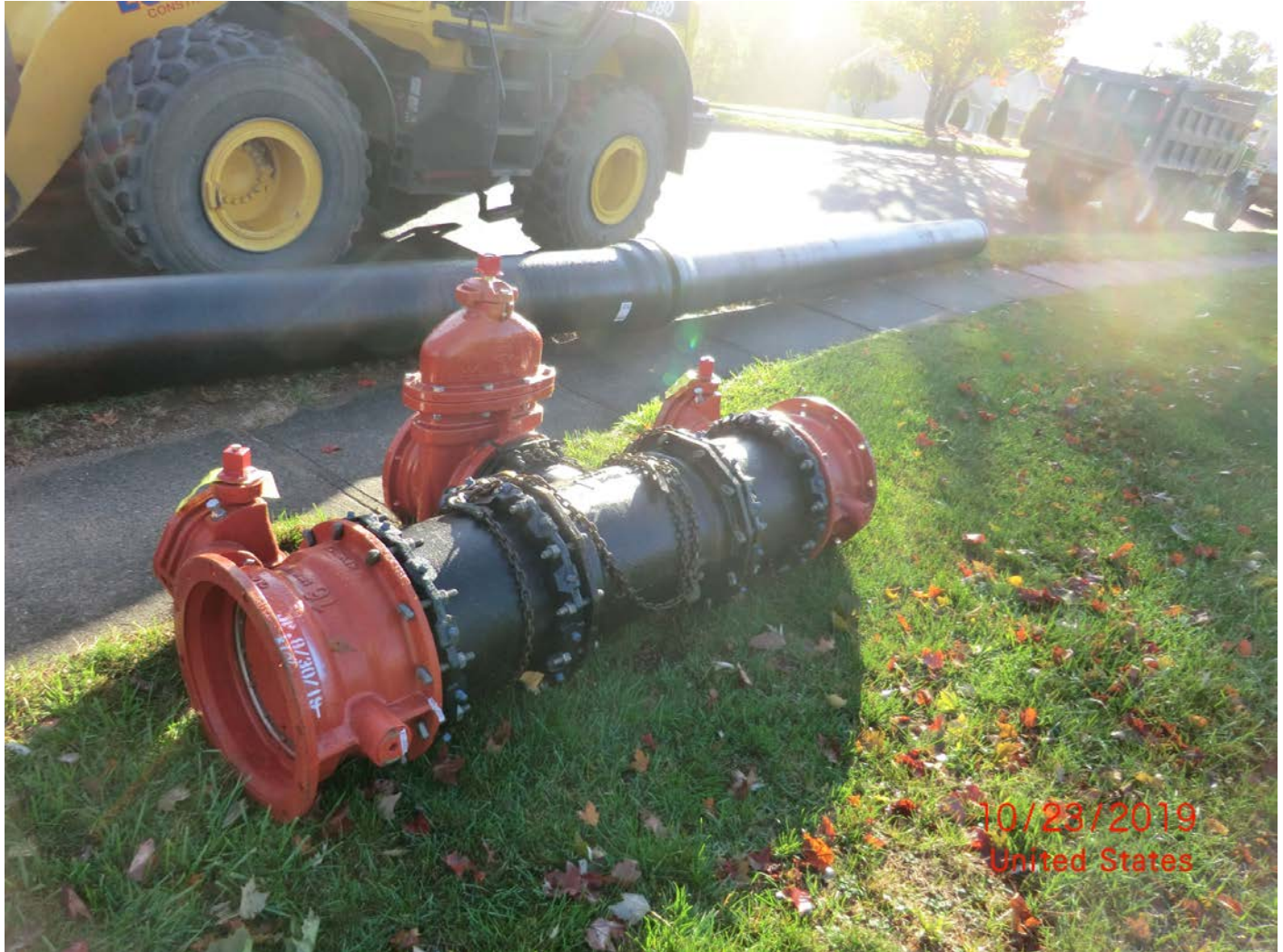
Figure 13 – Three valve assembly to be installed at location shown in Figure 12. Includes 2x16” Butterfly valves on either side and a 12” Gate valve in the center attached to a 16x12 Tee-section. Pipe length is 6.34 feet, physical length is approximately 7 feet.
