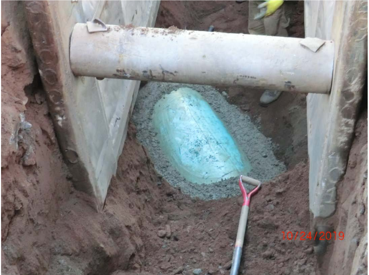
Figure 9 – A second ‘gasket’ of cement set around entire cover. Note that the ends were fill in over the bricks.
