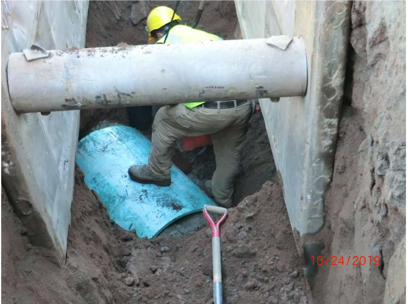
Figure 5 – Segment of ADS pipe set over ‘gasket’ of cement.
