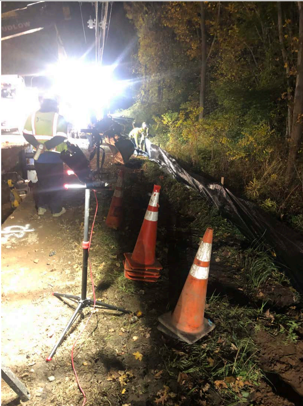
Figure 4 – Setting up sedimentation fence along road shoulder
