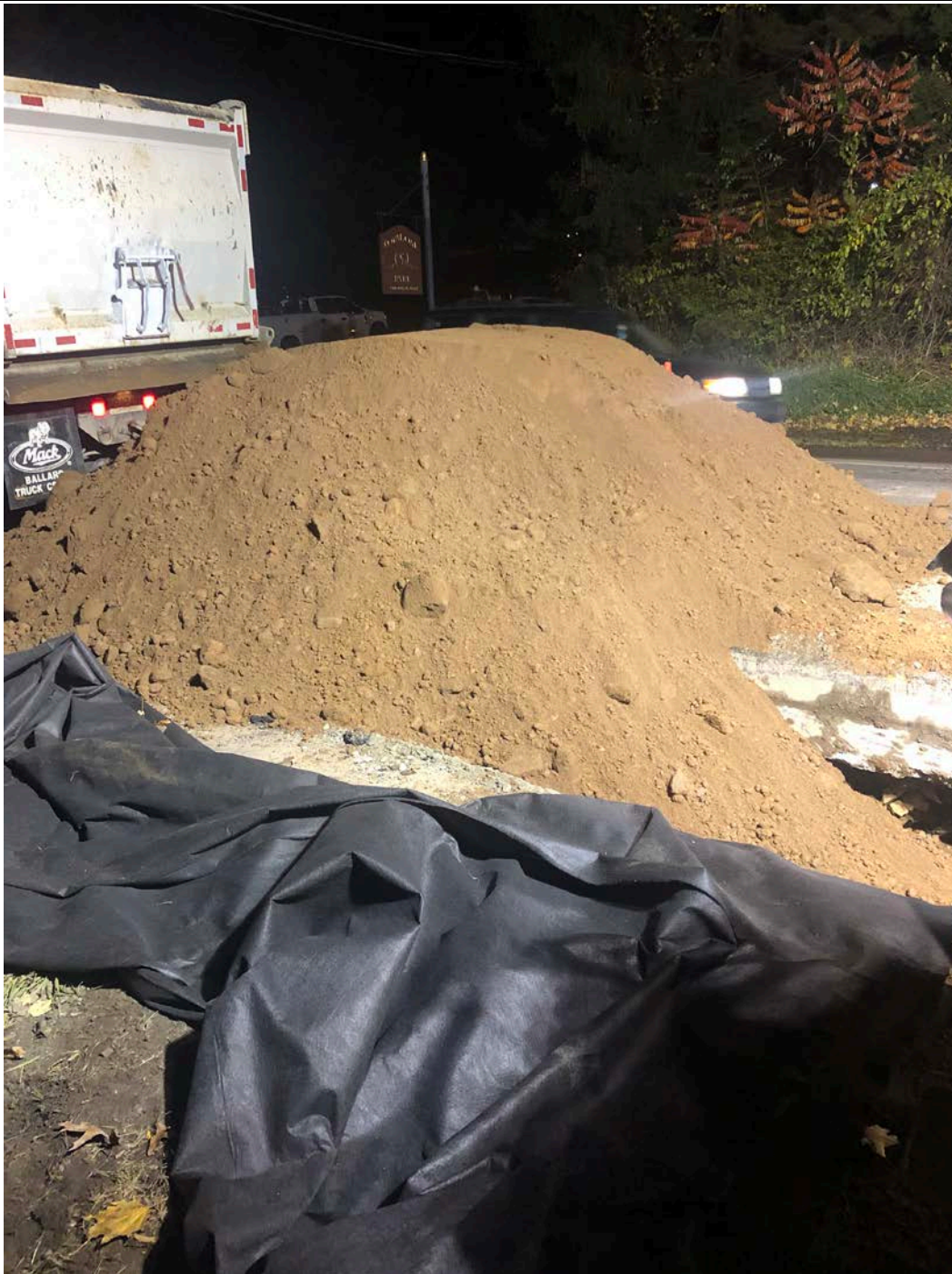
Figure 3 – Backfill pile at Sta. 126+74
