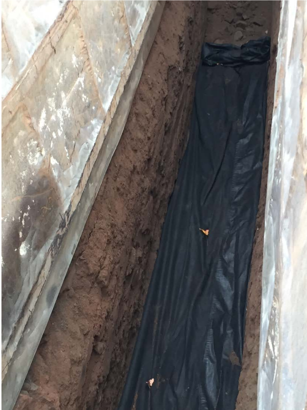
Figure 4 – Picture facing east into trench. The so called ‘gravel burrito’.
