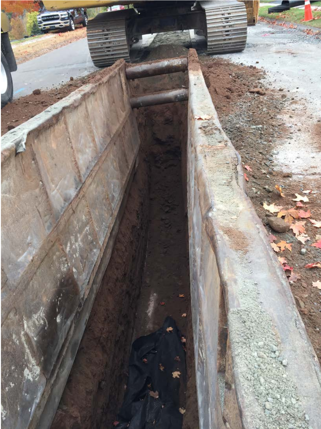
Figure 2 – Facing east into trench. Setting fabric in base of trench.
