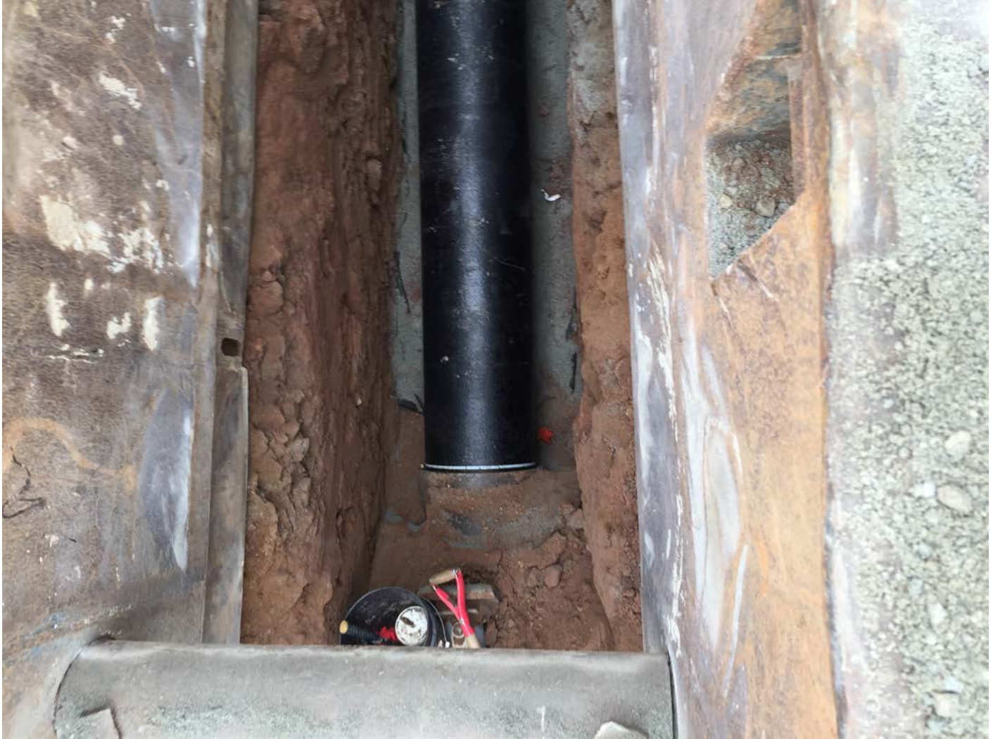
Figure 8 – Facing into trench. Unrestrained connection. Pipe seated in bell of previous section.
