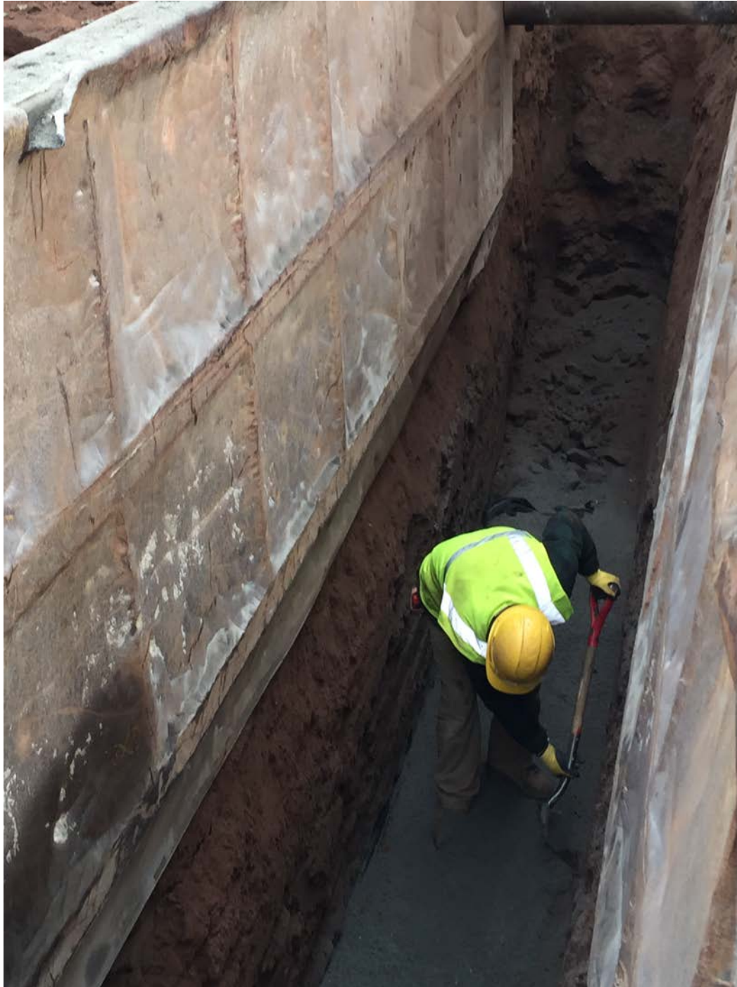
Figure 5 – Facing east into trench. The ‘burrito’ covered by approximately 3”-4” of stone dust and rough leveled.
