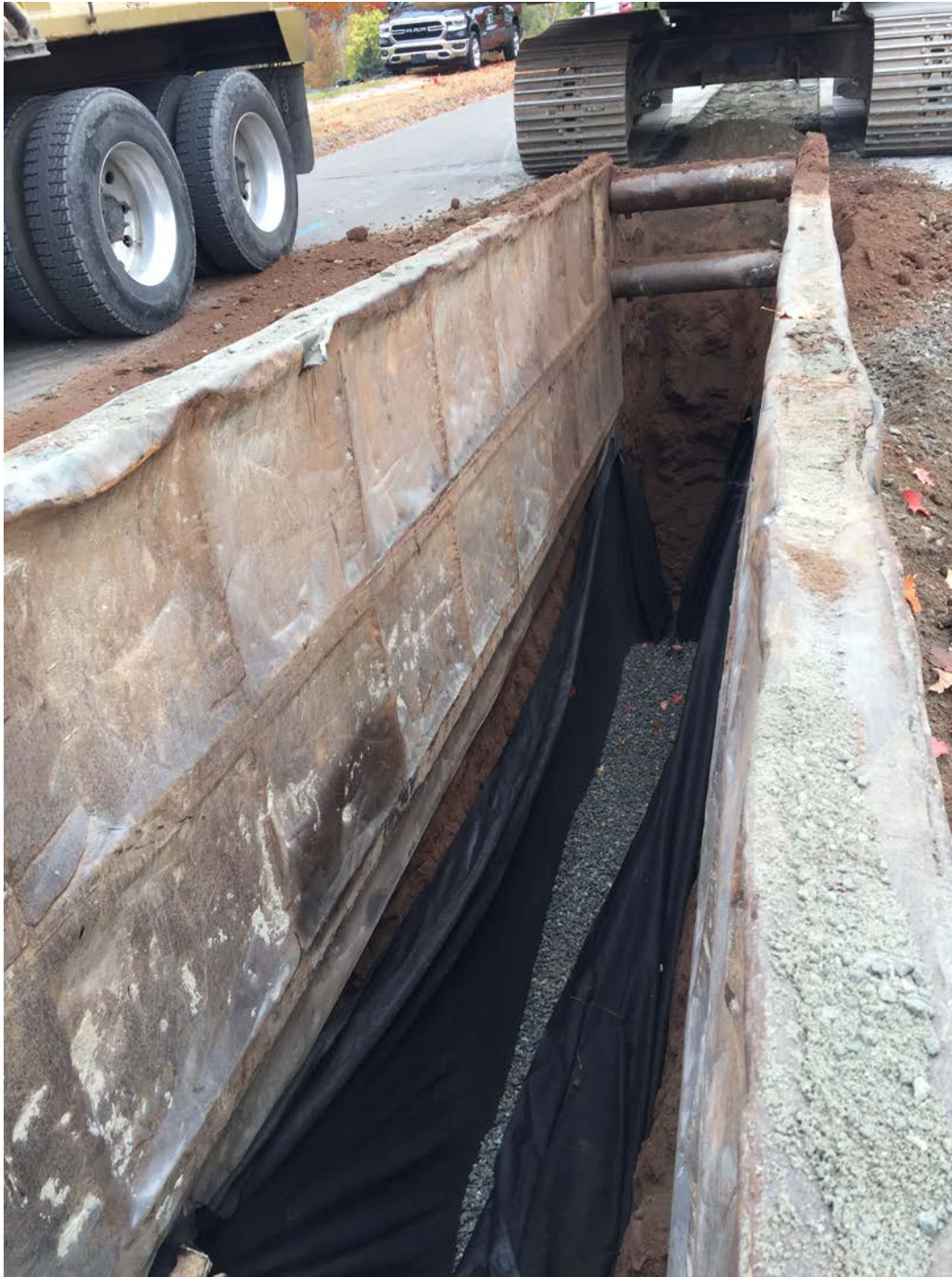
Figure 3 – Looking eastward into trench. Geotextile fabric with 1 foot of stone. Note trench box magnets used to hold fabric in place while stone is put into trench (magnet can be seen in bottom left corner of shot).
