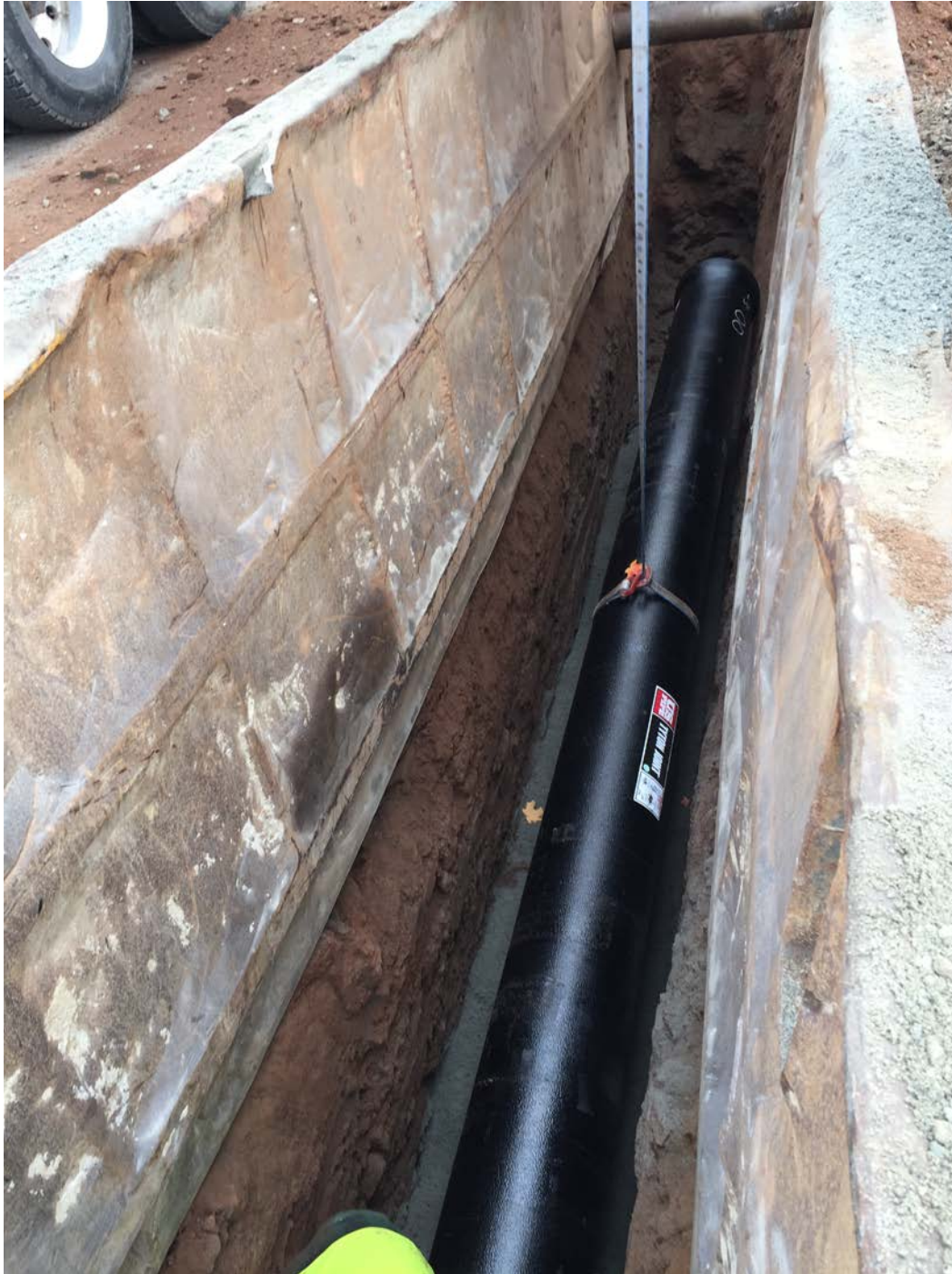
Figure 6 – Facing east into trench. Pipe set into trench.
