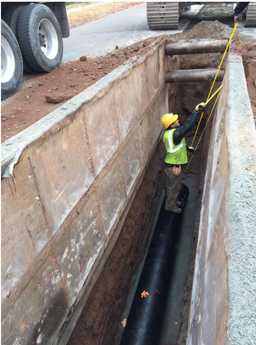
Figure 7 – Facing east into trench. Depth of pipe checked and adjusted as necessary.
