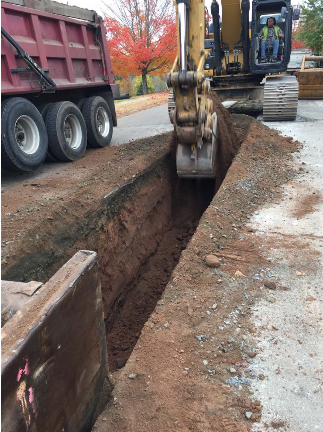
Figure 1 – Facing east. Digging trench for pipe.
