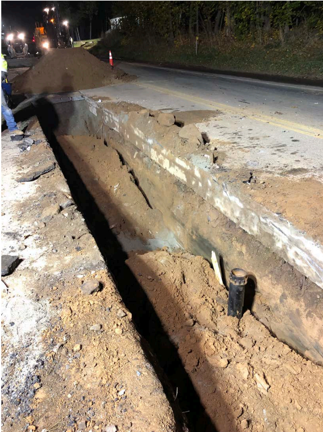
Figure 4 – Tee section covered with backfill, not yet compacted
