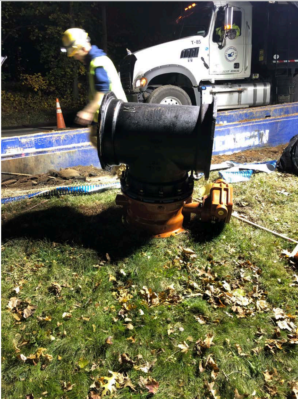
Figure 2 –T section to be placed at Sta. 125+20 (water meter vault connection)
