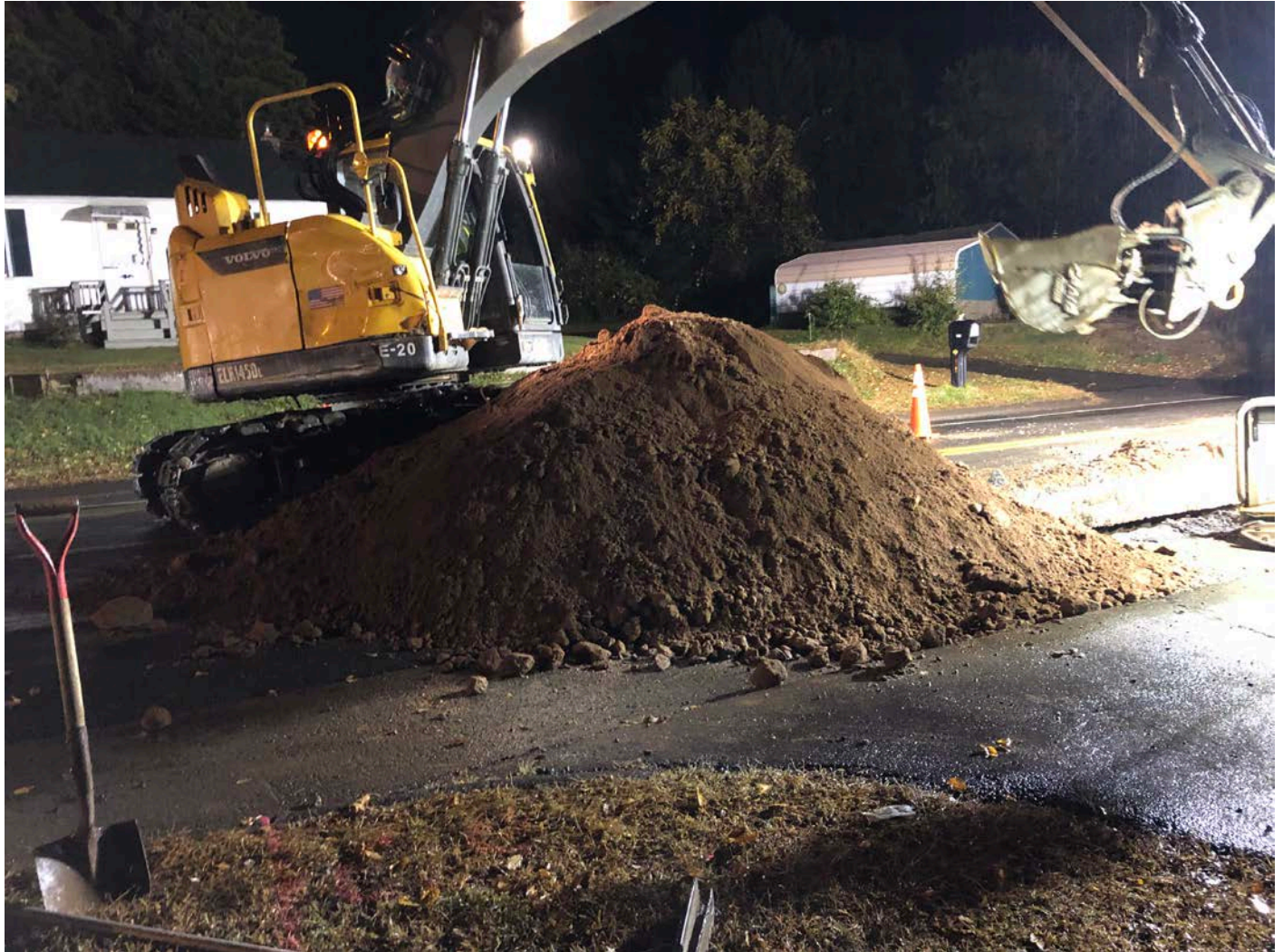
Figure 1 – Backfill pile before Sta. 122+92
