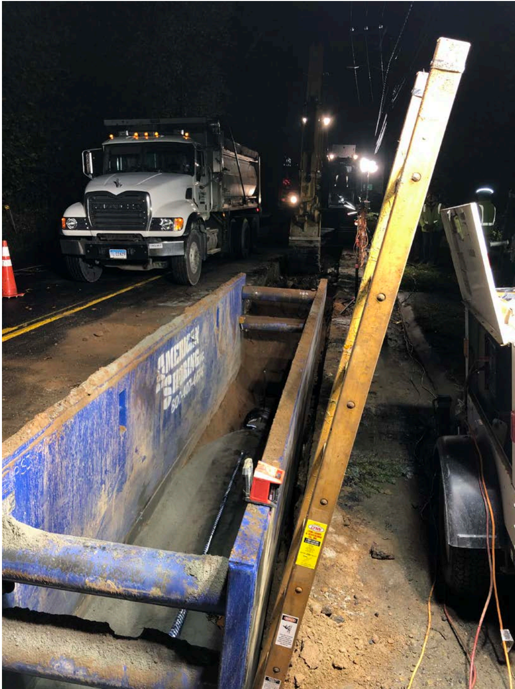
Figure 5 – 8 th section with bedding and warning tape laid overtop
