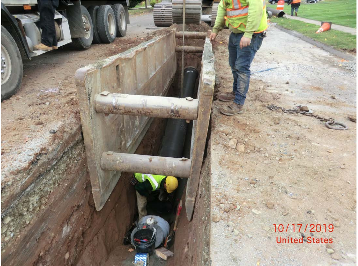
Figure 7 – Facing east, final 20-foot section of pipe installation.
