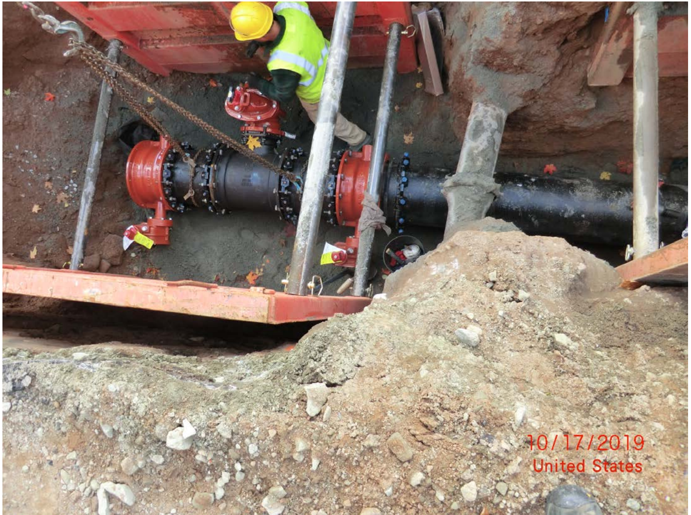
Figure 2 – Facing down into trench from north side. Note 8" existing line to right side crossing over first 11 feet of 16" DI installed. This is followed by the assembly currently being lowered into the trench – two 16" butterfly valves (red) either side of a 16x16x8 Tee-section (centered) with an 8" gate valve (red) 20" off the center line of the T to the south side.
