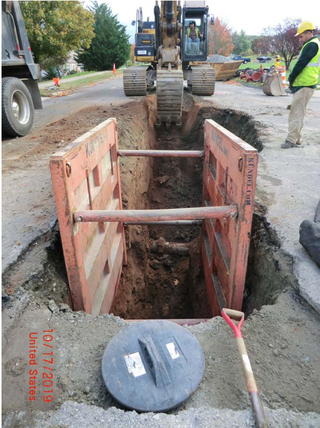
Figure 1 – Start Station 47+27.67. Note existing 8" restrained water line just beyond end of trench box. 16" DI will eventually run 0.5 feet under this line. First section installed – 11 feet to 47+16.67 Picture taken facing east.
