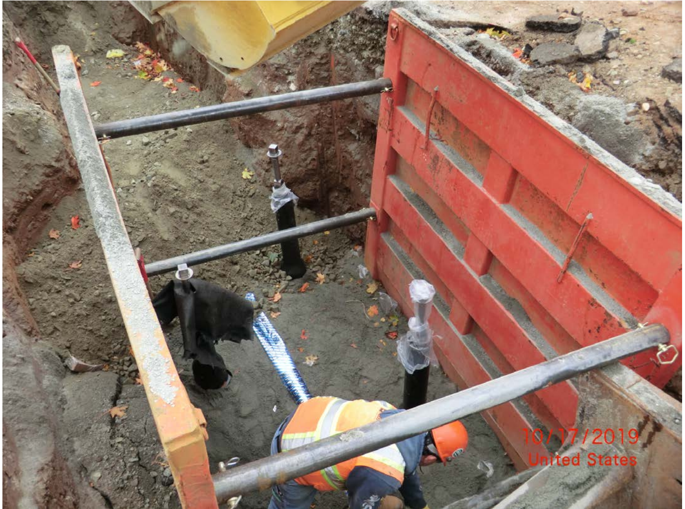
Figure 5 – Facing west into trench. Installing valve extension stems and raising grade. Note shiny water line marker tape.
