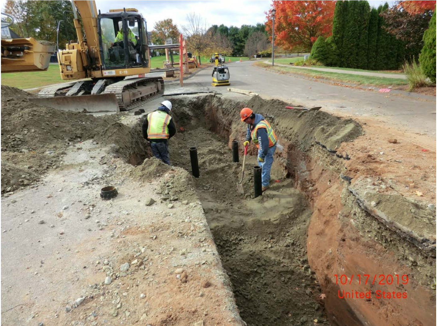
Figure 6 – Facing west, compacting lifts with Jumping Jack around valve box risers.
