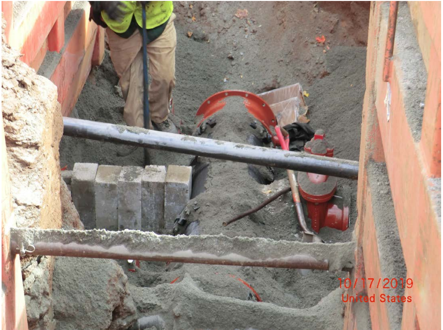
Figure 3 – Picture taken facing east. Thrust blocks installed on north side of Tee-section across from 8" gate valve.
