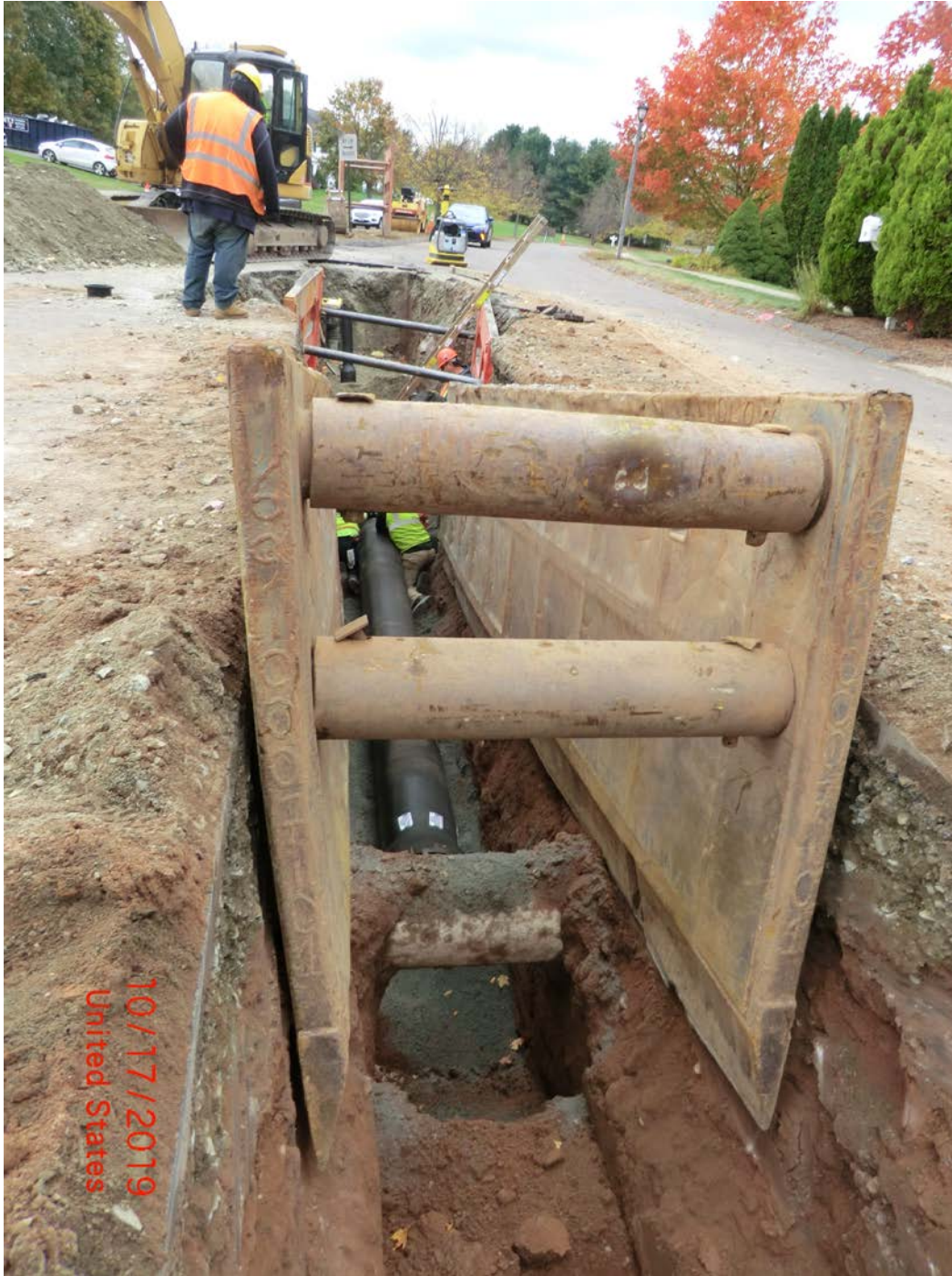
Figure 4 – Picture facing west. First 20-foot section of 16" DI installed to 46+90.34, just short of crossing under 18" catch basin drainage pipe. Next section of pipe will cross approximately 1.5 feet below the drain pipe..
