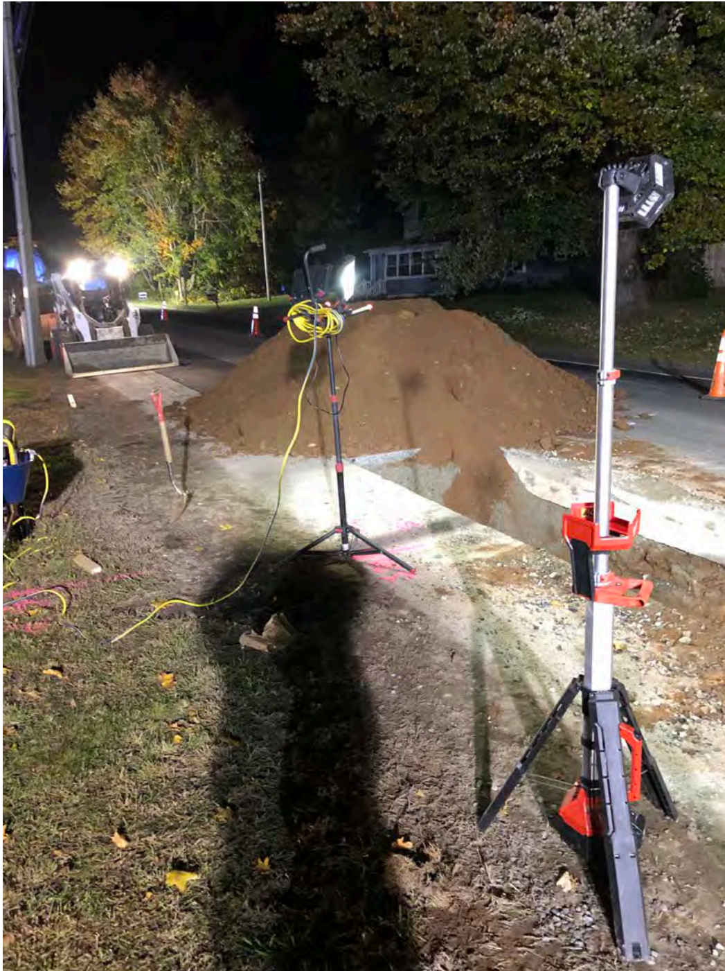
Figure 3 – Backfill pile before Sta. 118+31
