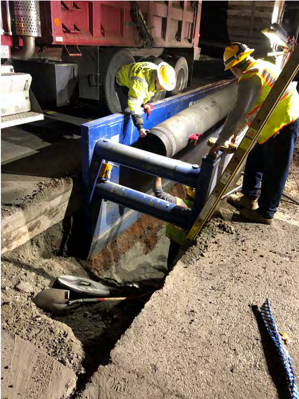
Figure 1 – Attaching 1 st pipe section at Sta. 118+31
