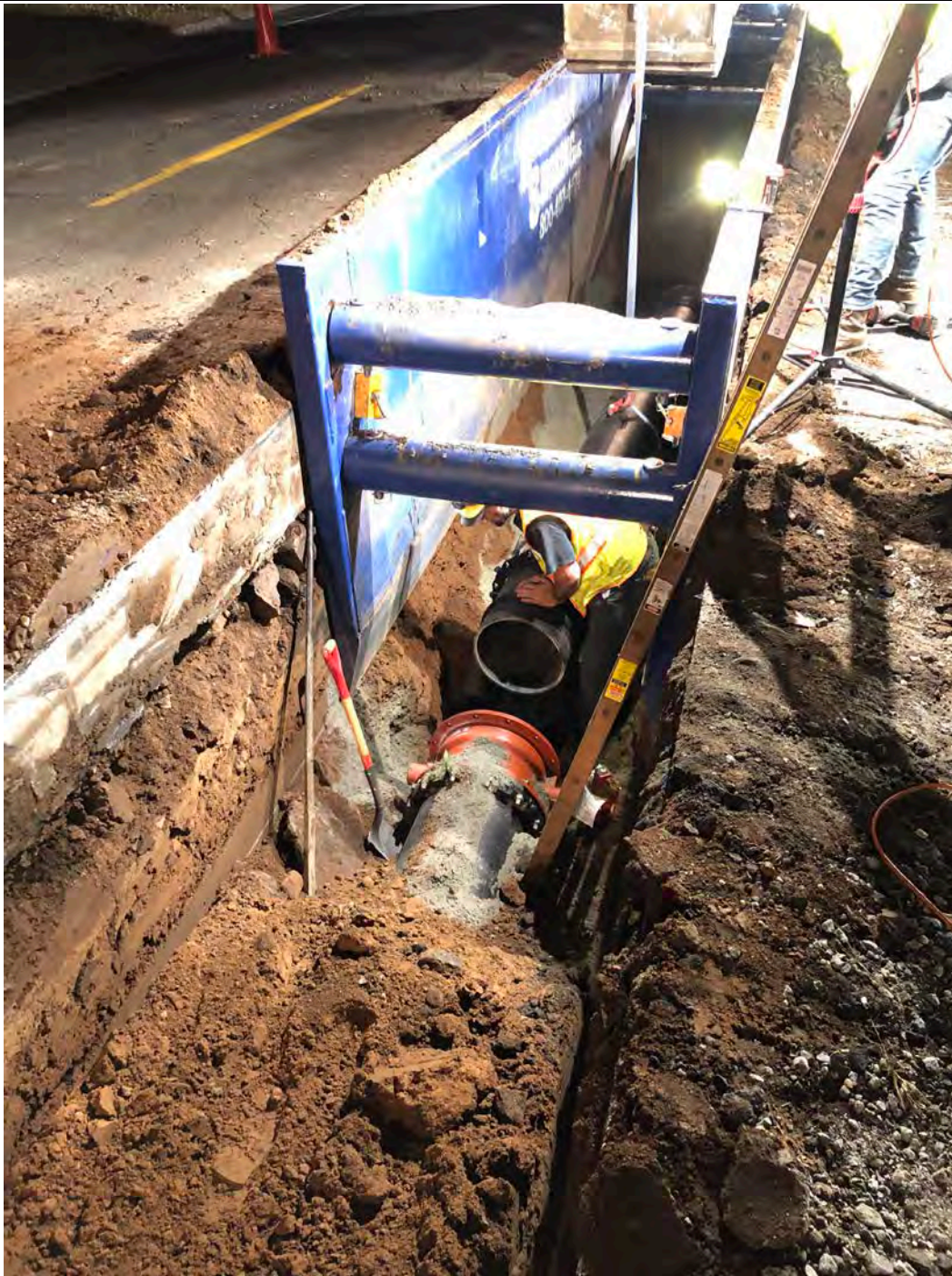
Figure 5 – Attaching 7 th pipe section to 16” butterfly valve at Sta. 119+37
