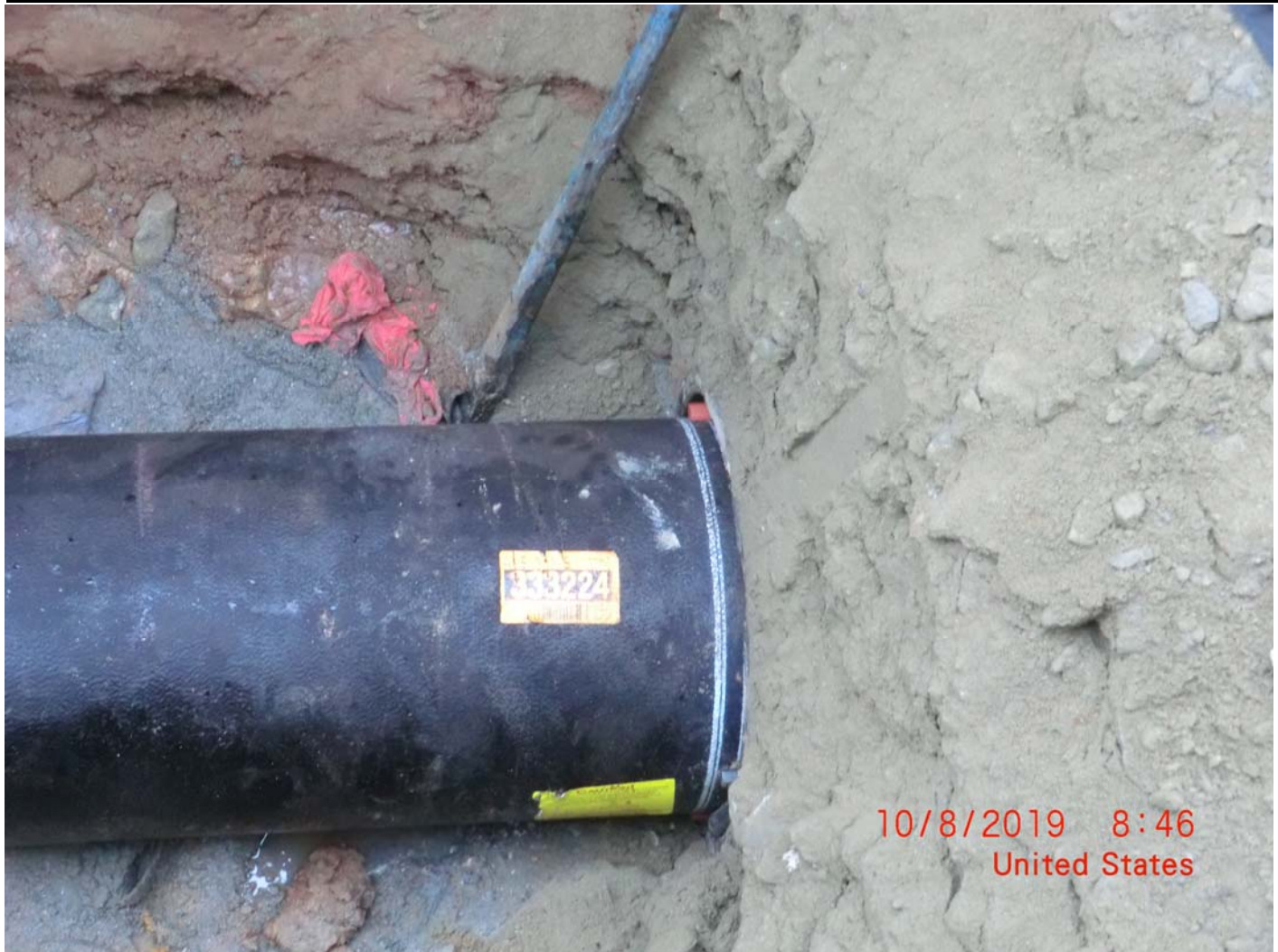
Figure 6 – Typical pipe seating. 16” DI Pipe to left - pipe bell to right (not shown in picture due to fill). Note the orange (top) and black (bottom) lock wedges seated in connection to bell.
