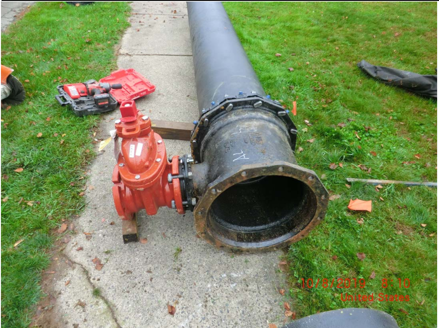
Figure 4 – Fire Hydrant Tee assembly preparation. Pipe cut at approximately 14 feet to insert Tee. Remaining 6 feet at bottom right of picture.
