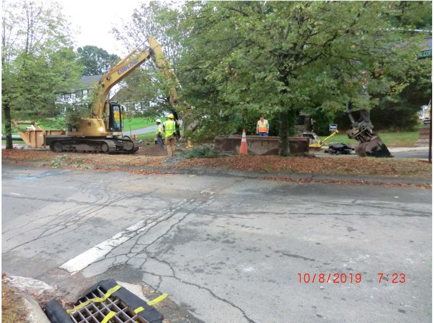
Figure 1 – Start of first run at 51+72. Note excavator to left digging and excavator to right backfilling (not currently active). Also note double catch basin to front left of picture – typical liner installed to catch sediment runoff. Picture taken facing south.
