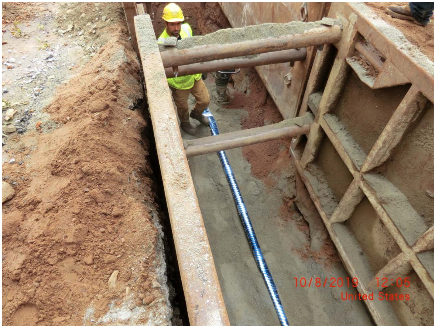
Figure 9 – Top of compacted 12-inch lift of pipe bedding. “Caution Water Line Below” tape on top.
