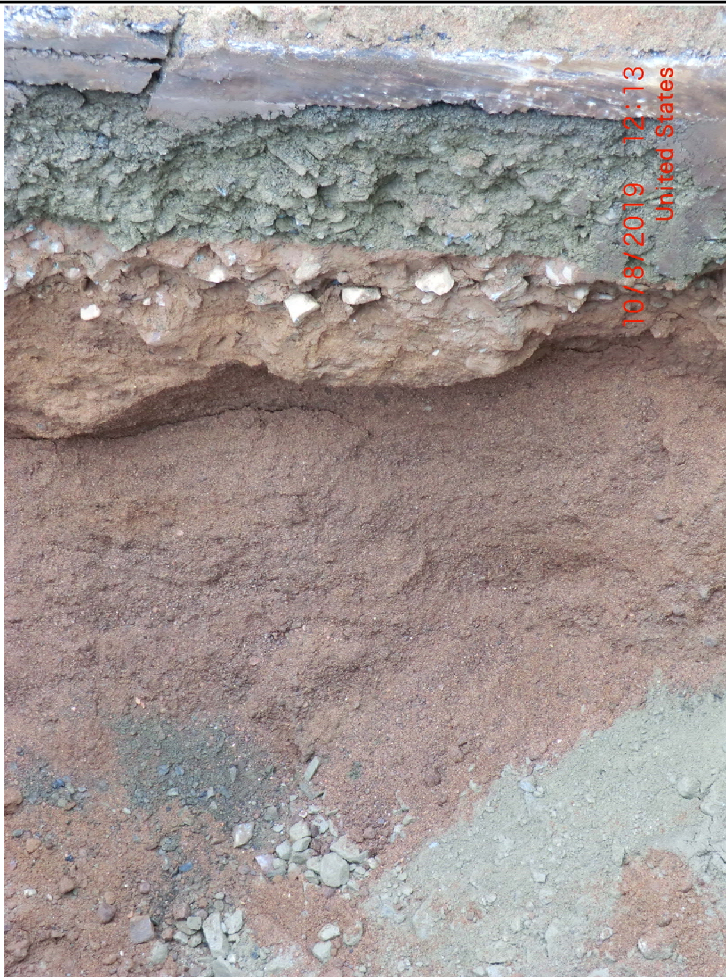
Figure 10 – Typical soil profile section located roughly at 51+00. From top, asphalt, road base, medium-fine sand, sandy silt (not shown – below pipe bedding backfill at bottom of picture).
