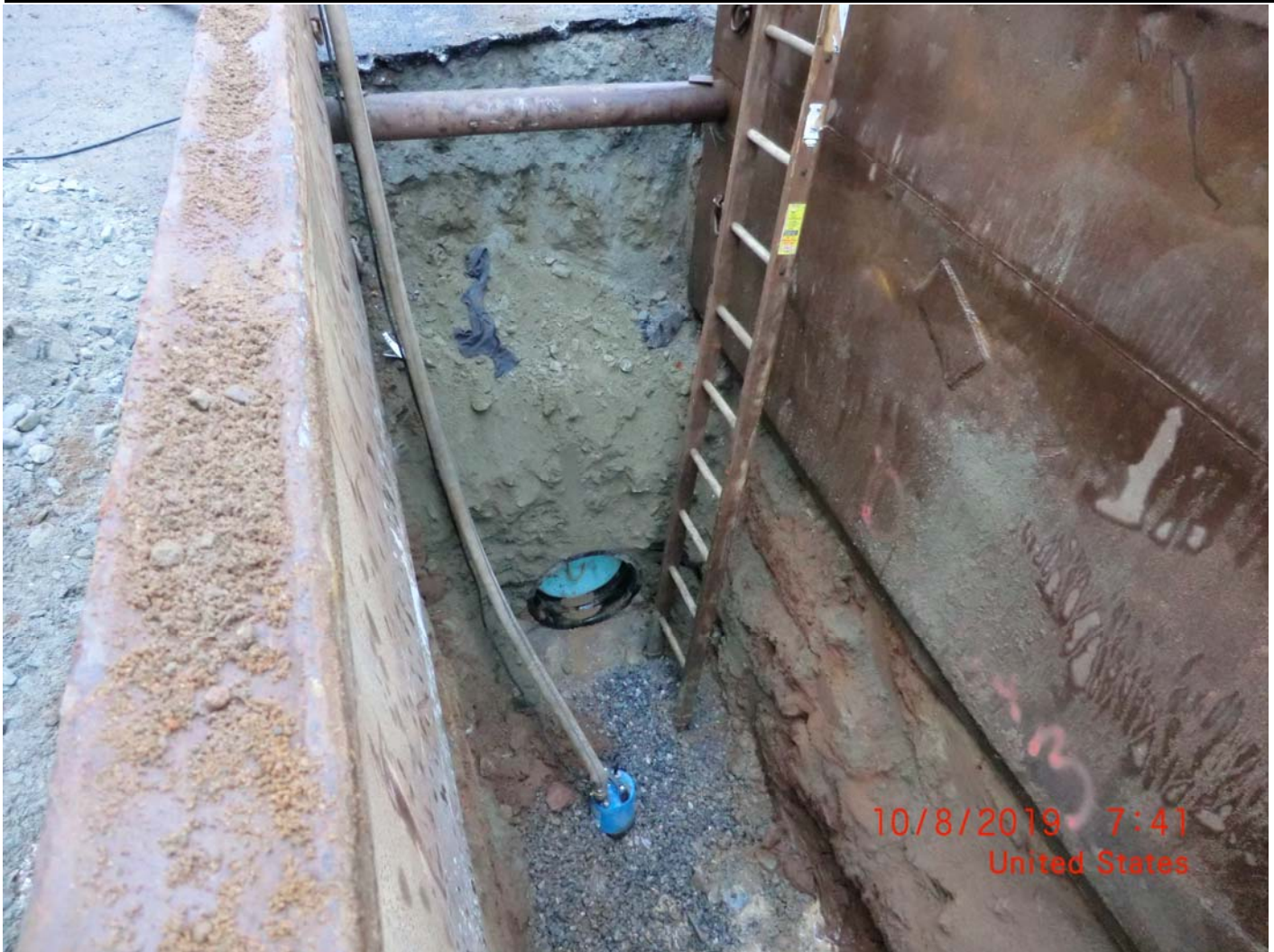
Figure 2 – Start of operations – Plugged pipe end from 10/7/19 at 51+72. When this plug was removed approximately 20 gallons water spilled out. Gate valve at other end of pipe (Tee-section with So. Main Street line) is closed at time of this picture. Picture taken facing west into road cut.
