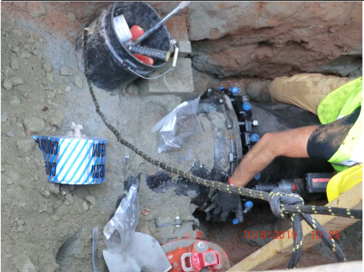
Figure 8 – Installation of remaining 6 feet of 18-foot 16" DI pipe, with Megalug restraining gland.
