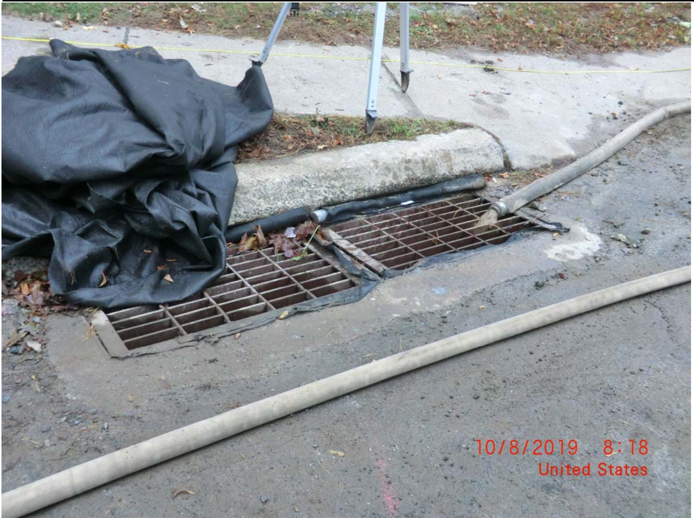
Figure 5 – Sump discharge to double catch basin (south side of Talcott Ridge Dr. at South Main St.). Note that catch basins have been lined.
