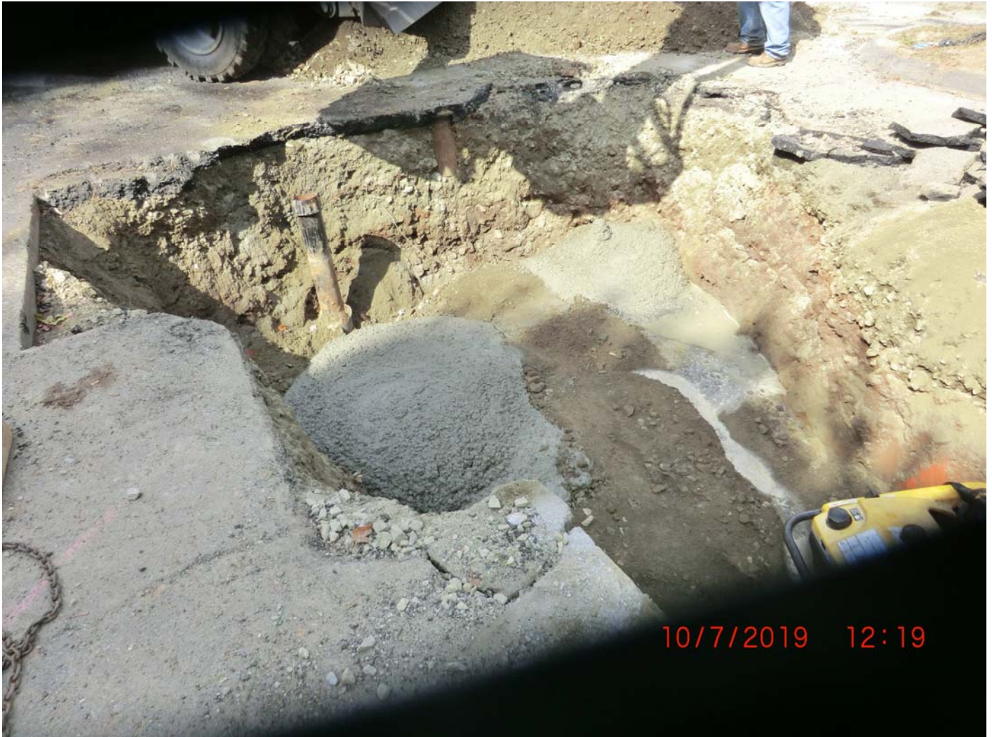
Figure 11 – Cement cover over stormwater drain connections and T-connection. Note valve boxes.
