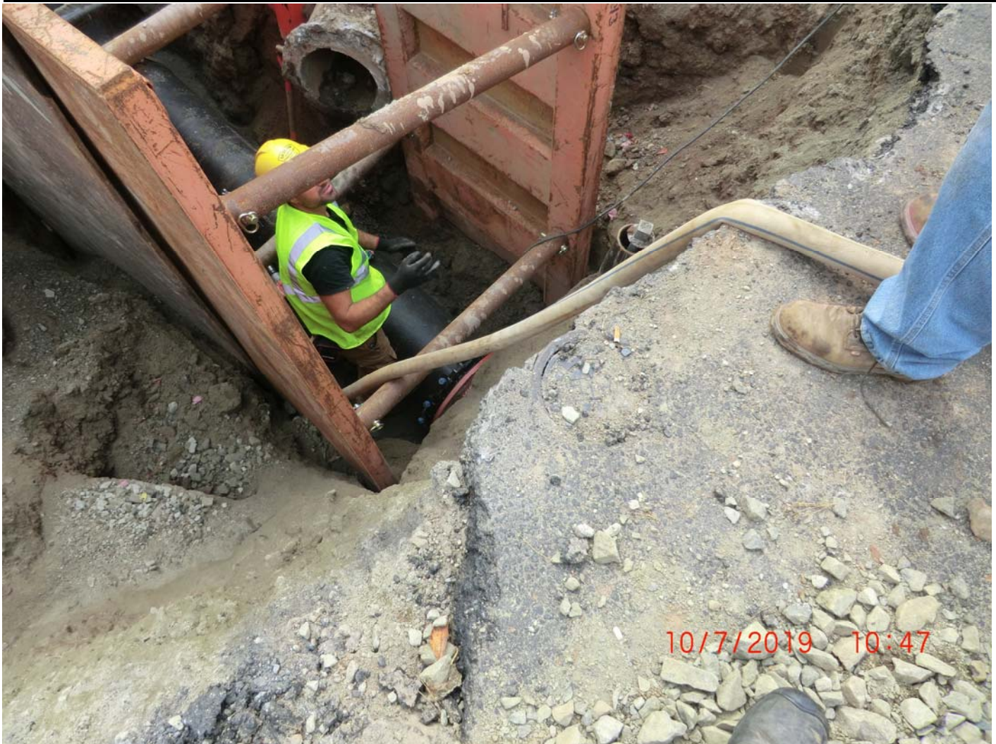
Figure 8 – Connection with MJ retainer gland. Note sump line hose.
