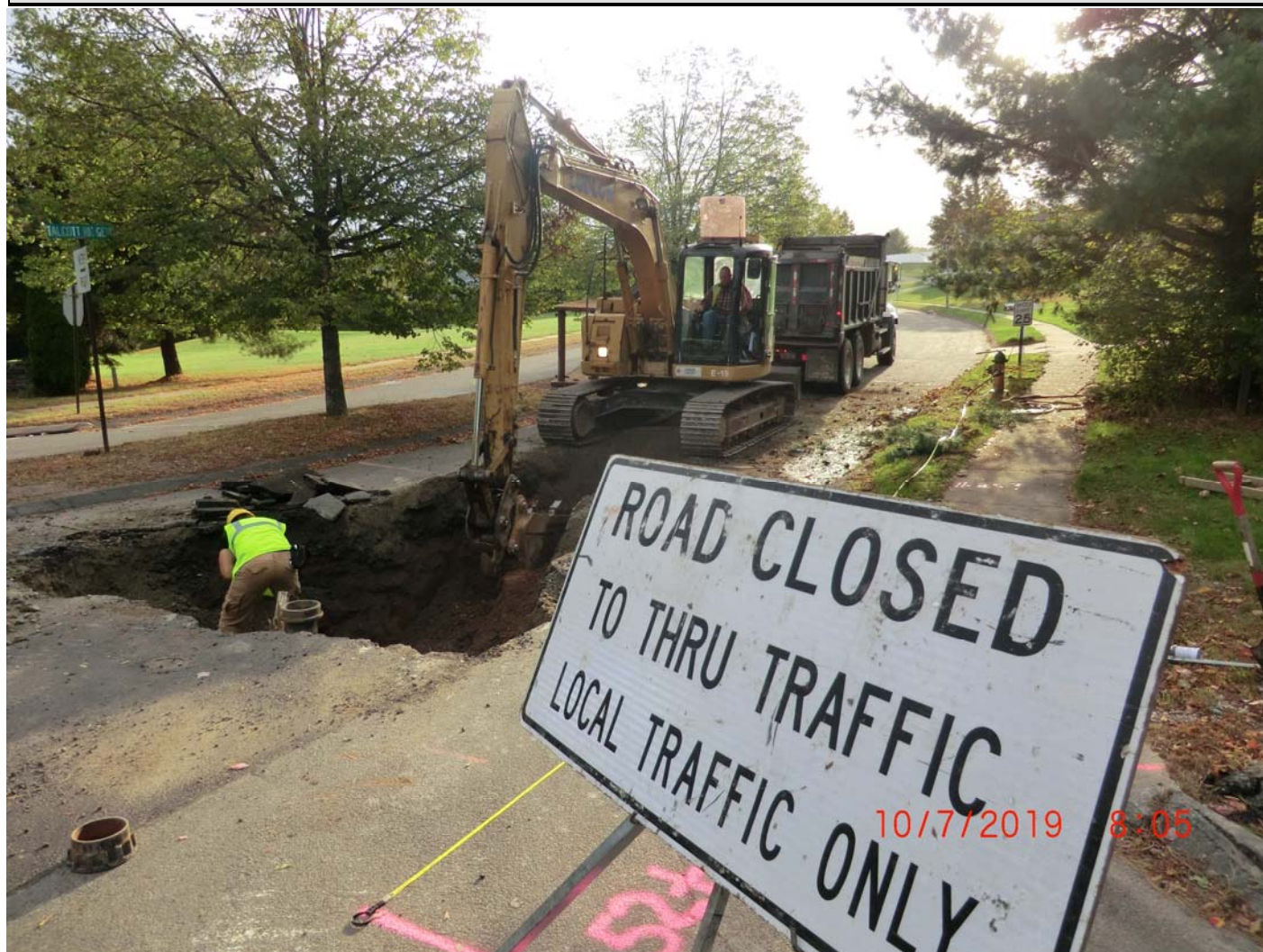
Figure 2 – Start of operations. Note 52+00 in foreground. START 51+93 – Tee-connection.
