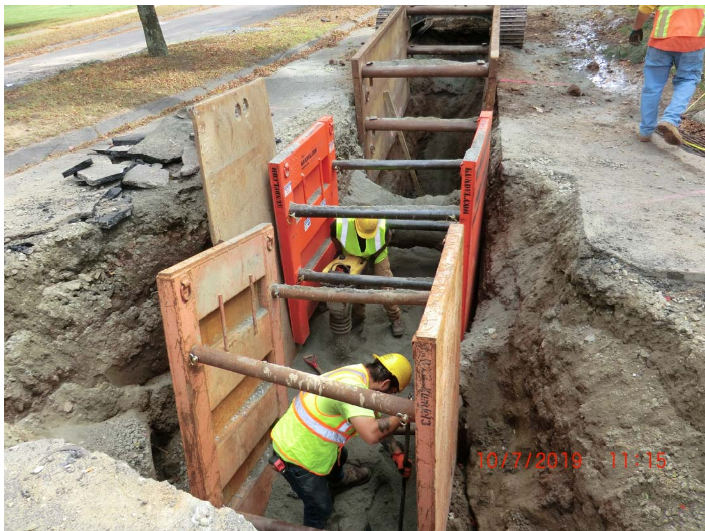
Figure 9 – Compacting pipe bedding lifts
