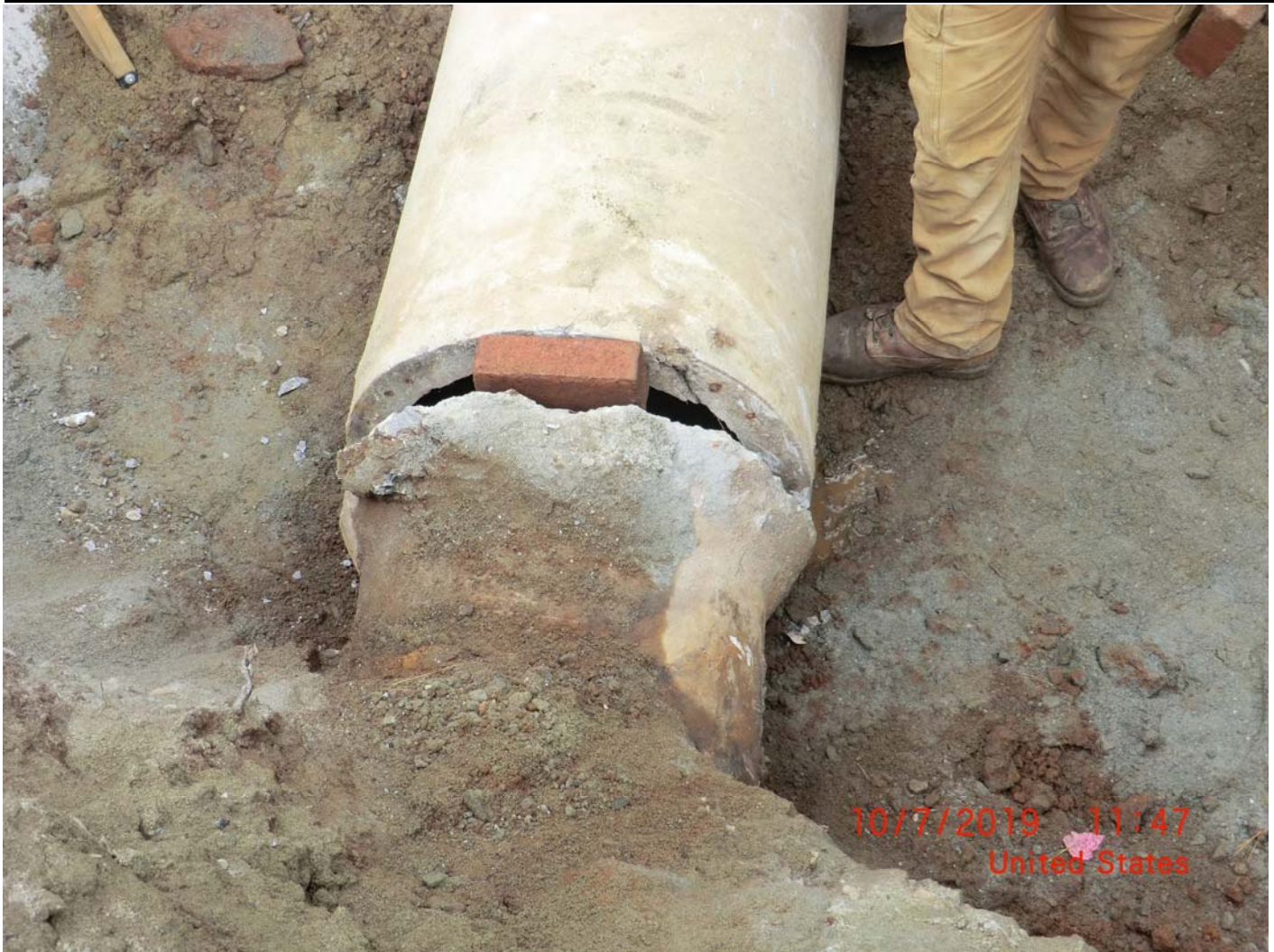
Figure 10 – Using bricks to fill gap at 15"/18" stormwater pipe connection. Gap filled with brick pieces, followed by wrapping in geotextile fabric, and duct tape ends.
