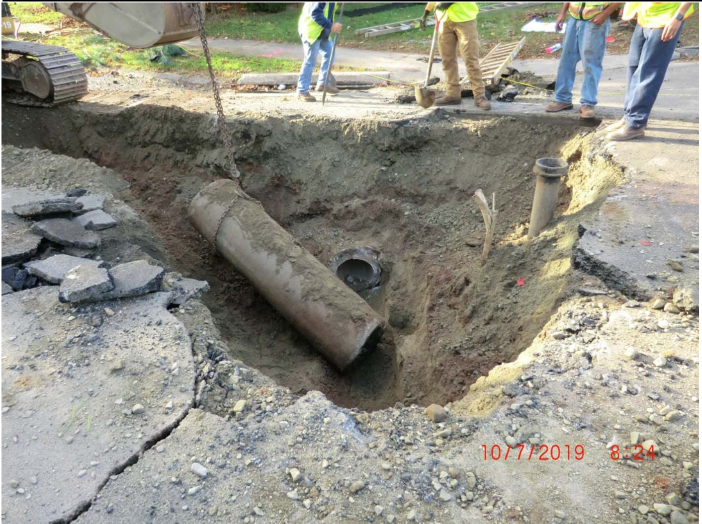
Figure 4 – Stormwater drain section removed. Looking up flow at 15” opening. Pipe on chain is 18”. Catch Basins top center of picture.
