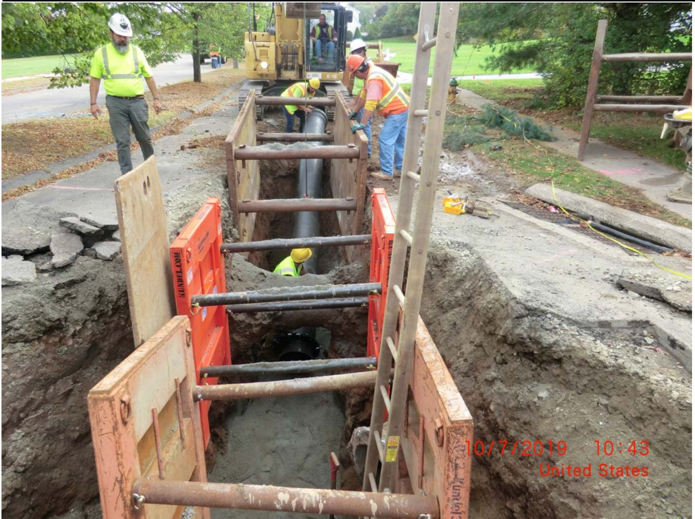
Figure 7 – 16" DI pipe installation
