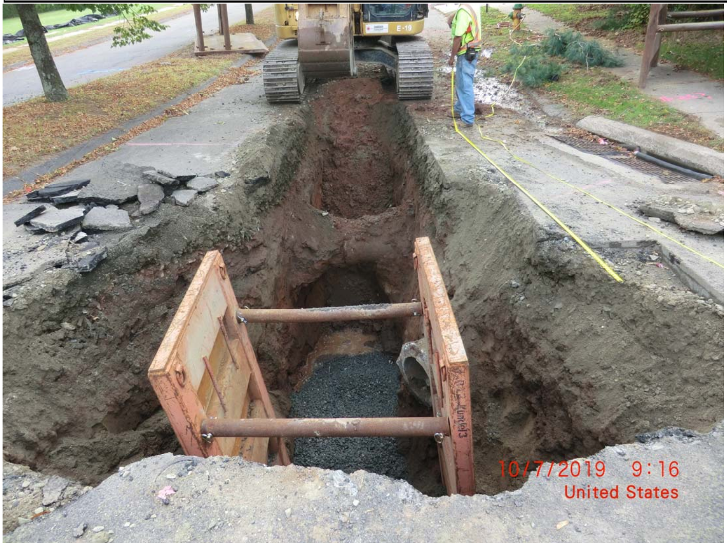
Figure 5 – Second storm drain center of picture. Note gravel in pit placed because of water infiltrations. 15" drain behind road-box.
