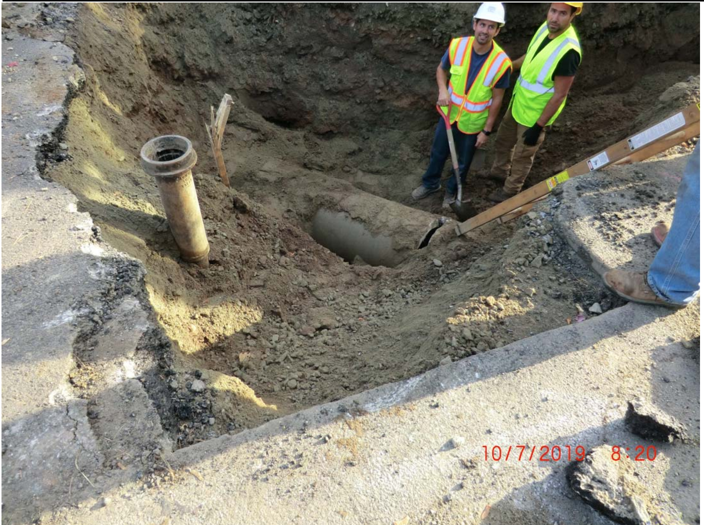
Figure 3 – Mis-matched 18" (left) to 15" (right) stormwater drain.
