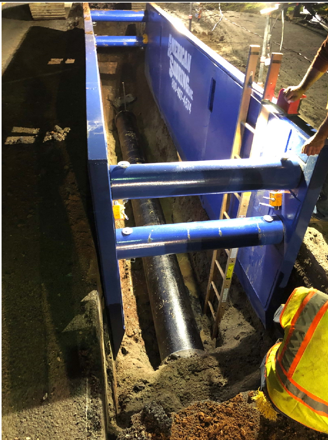
Figure 1 – First pipe section attached at Sta. 111+88
