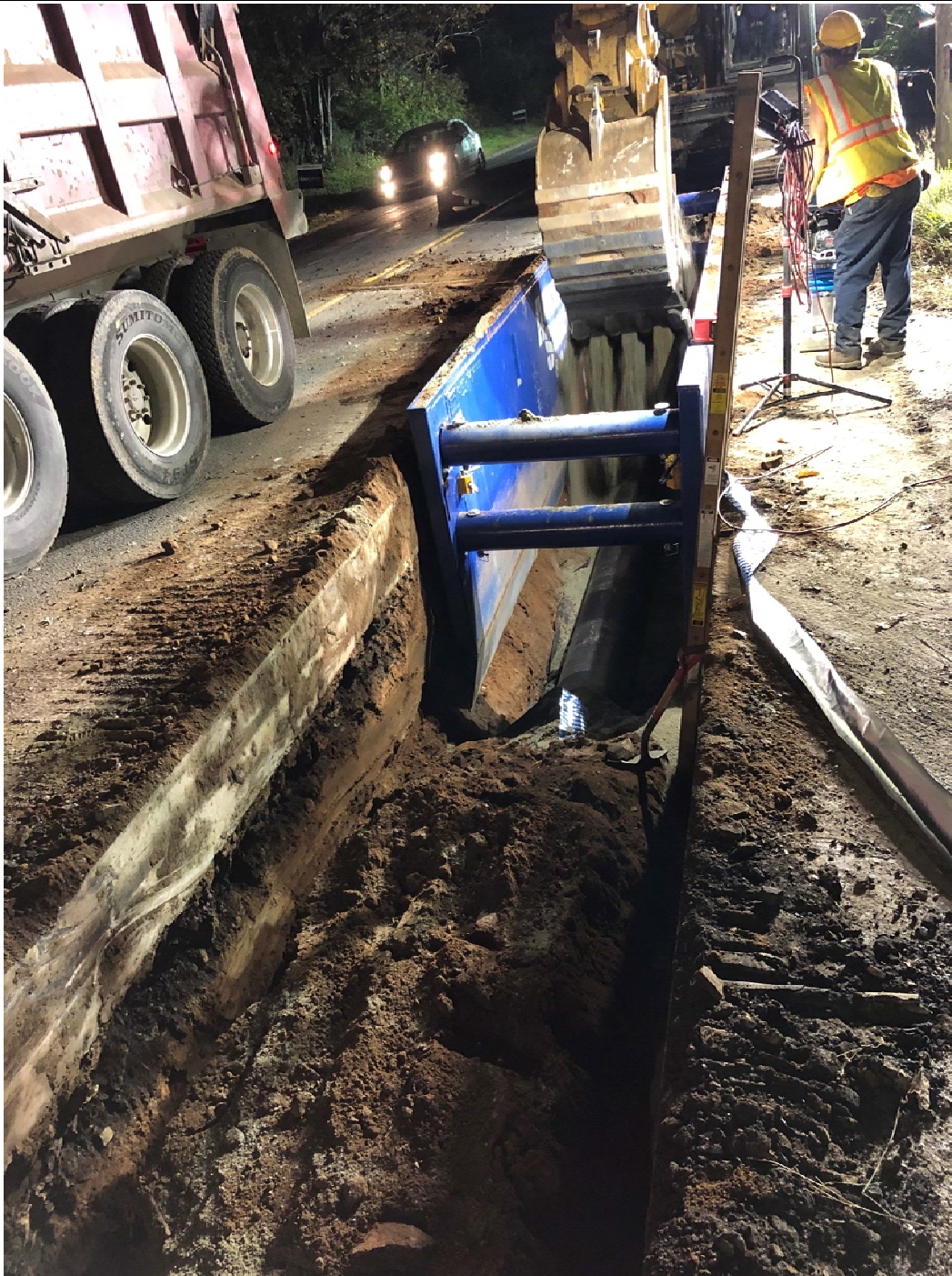
Figure 4 – Bedding being placed over 6 th section of the night
