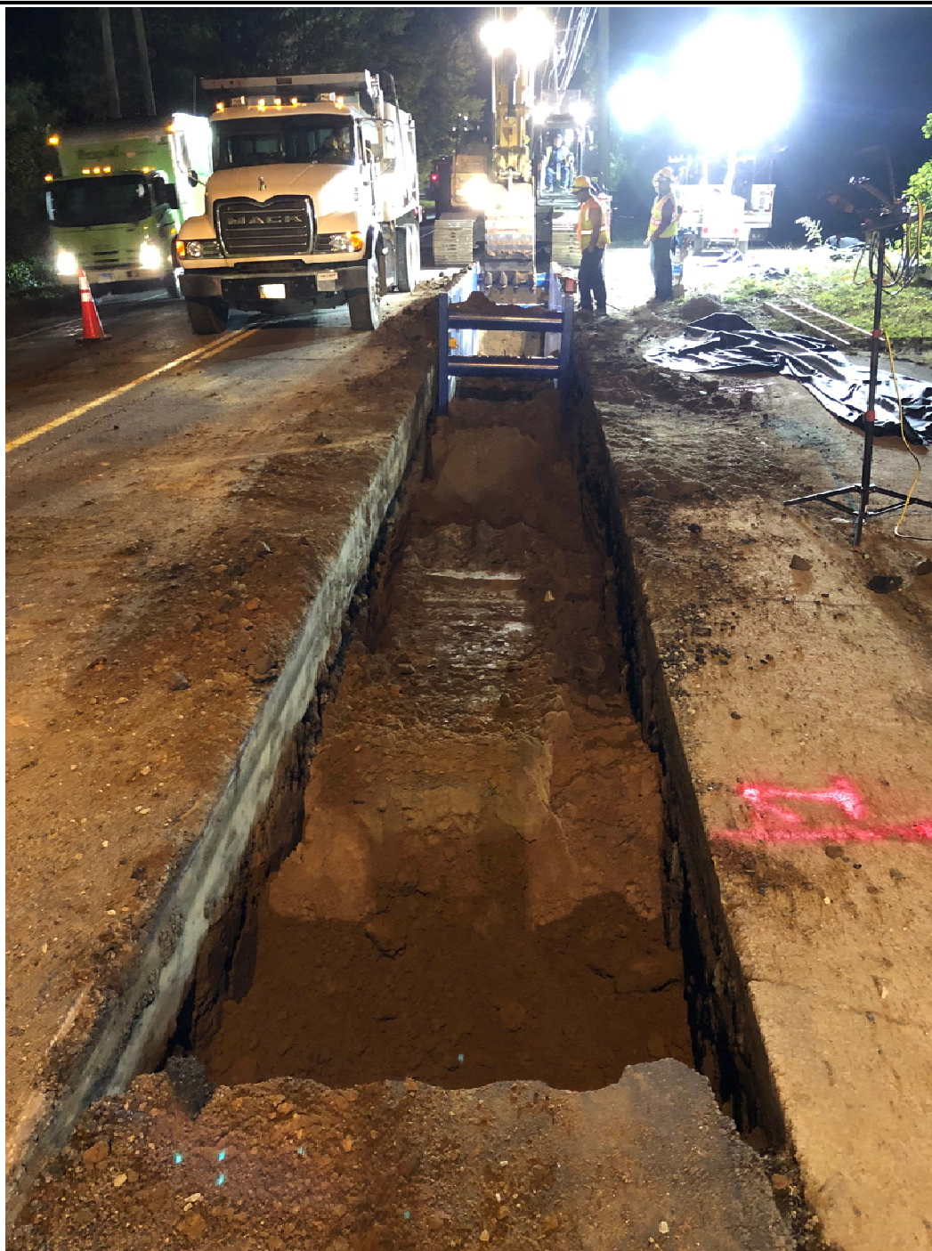
Figure 2 –Uncompact backfill over sections 1 and 2 of the night
