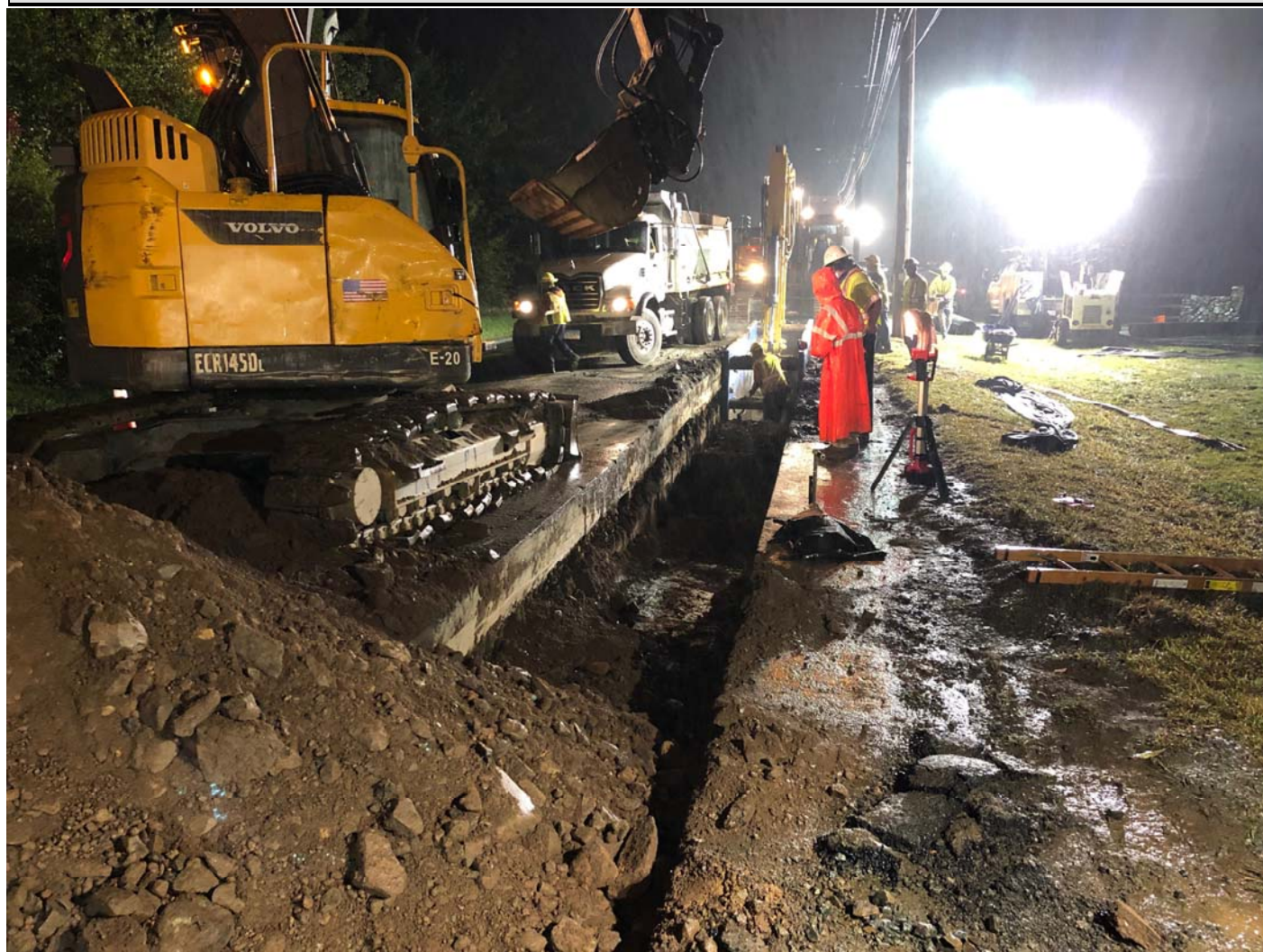
Figure 2 –Uncompacted backfill pile, looking southwest
