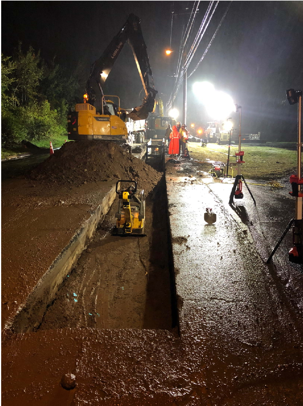
Figure 3 – Compacted top backfill lift standing at Sta. 109+49
