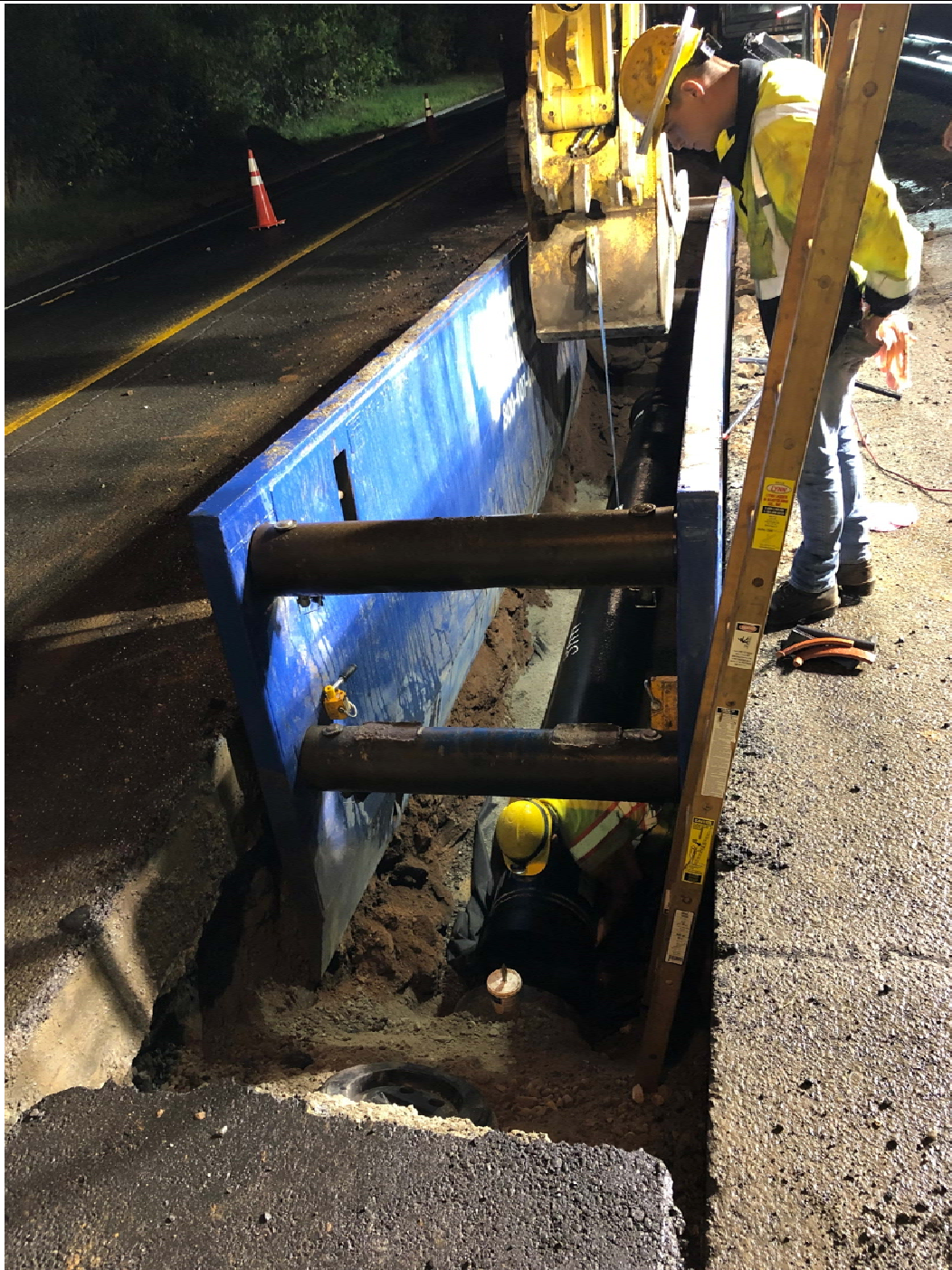
Figure 1 – Lowering first pipe section to attach
