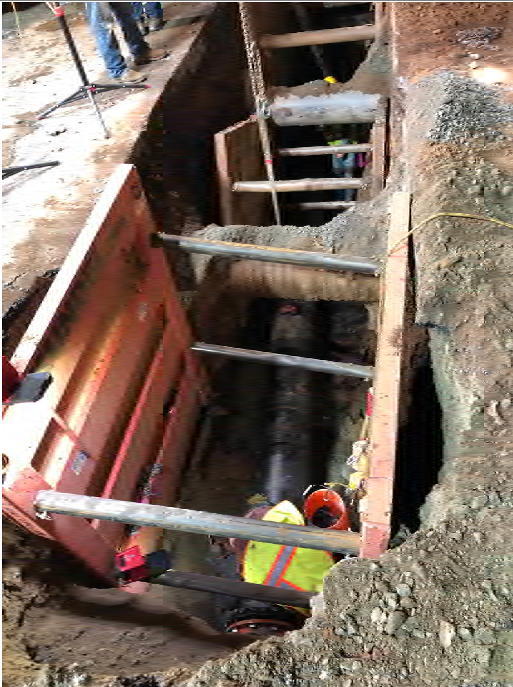
Figure 2 – Placing pipe section, attached to tee section and butterfly valve
