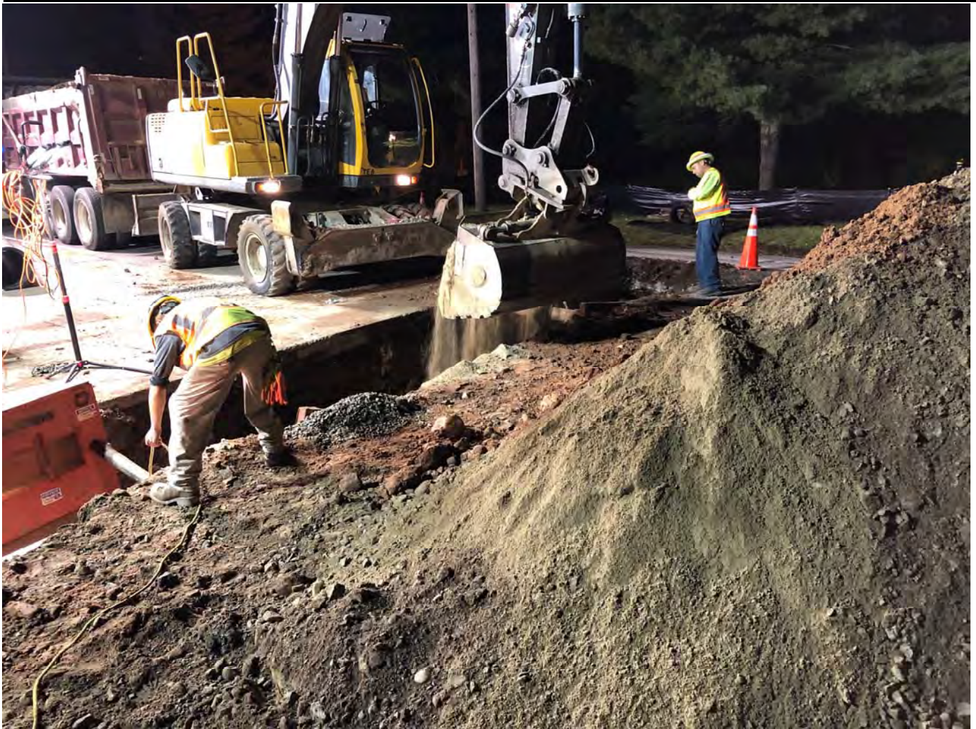
Figure 3 – Placing pipe bedding over pipe section
