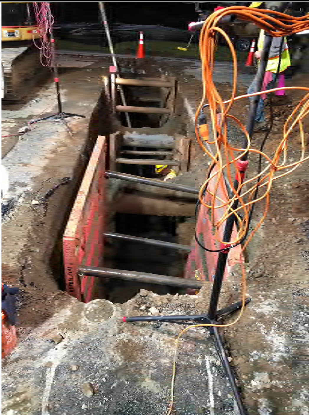
Figure 1 – Storm drain (near) and natural gas (far) lines in trench, facing west (across road) from Tee section
